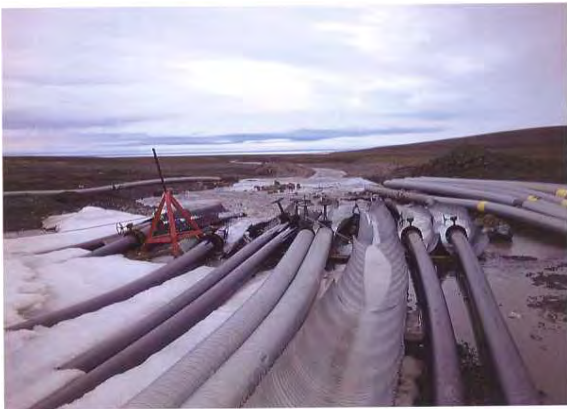
Figure 6. Siphoning of Garrow Lake surface water across the outlet dam into Garrow Creek (looking downstream).
