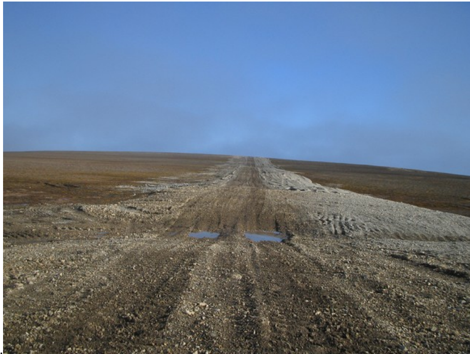
View to southwest looking up gently sloping section approximately 800 m from the water intake causeway. Roadway is in good condition, with only minor erosion of loose material at drainage crossing.
