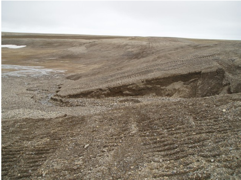
View adjacent and immediately to west of view shown above showing significant erosional down cutting of what appears to be quarry strippings of silty sand and gravels.
