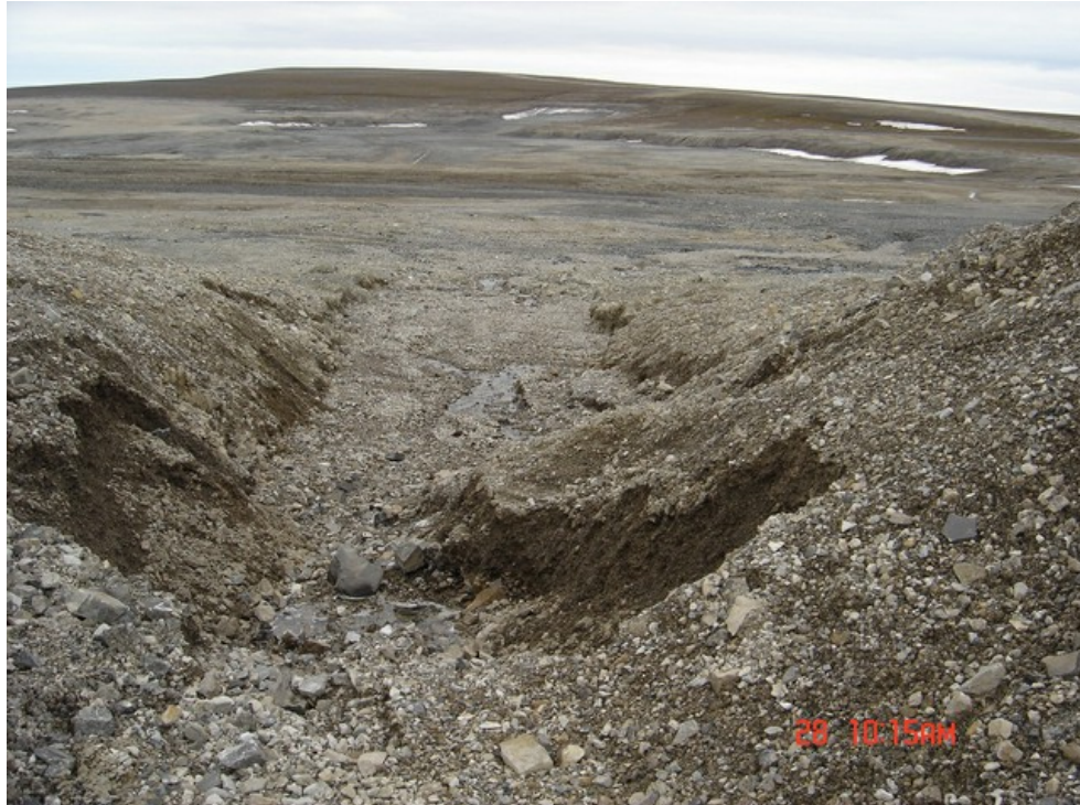
Photo looking downstream from waypoint NQG2CUL, where there is an existing collapsing culvert. While channel appears to self-armouring, the culvert should be removed and sideslopes flattened.
