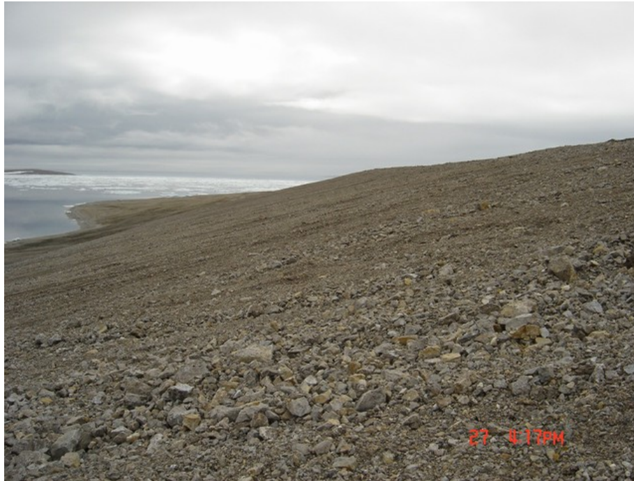
View southwest along main sideslope of the Operational Landfill from waypoint OLF3, again showing slopes in good condition, free of any erosion or deformation.
