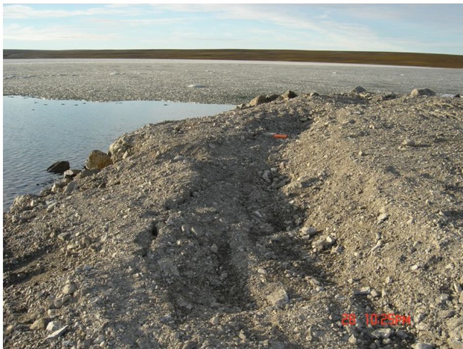
View from waypoint FL2 looking across northern end of causeway – note slight subsidence in foreground, with vertical separation of about 0.3 m over a width of 2 m possibly from melting of snow/ice buried within the fill.
