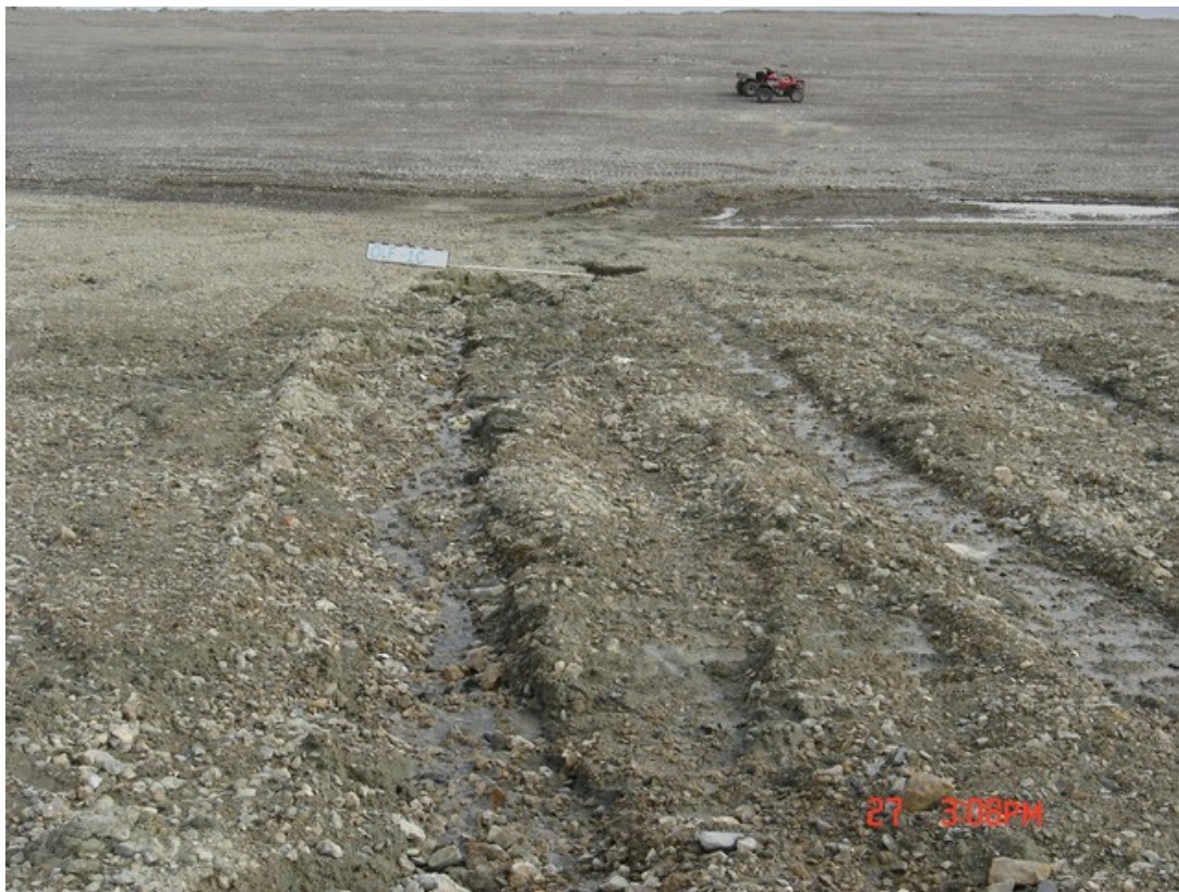
View downslope from waypoint LO SPR TOP. The degree of erosion is not serious and appears to be gradually self-armouring.
