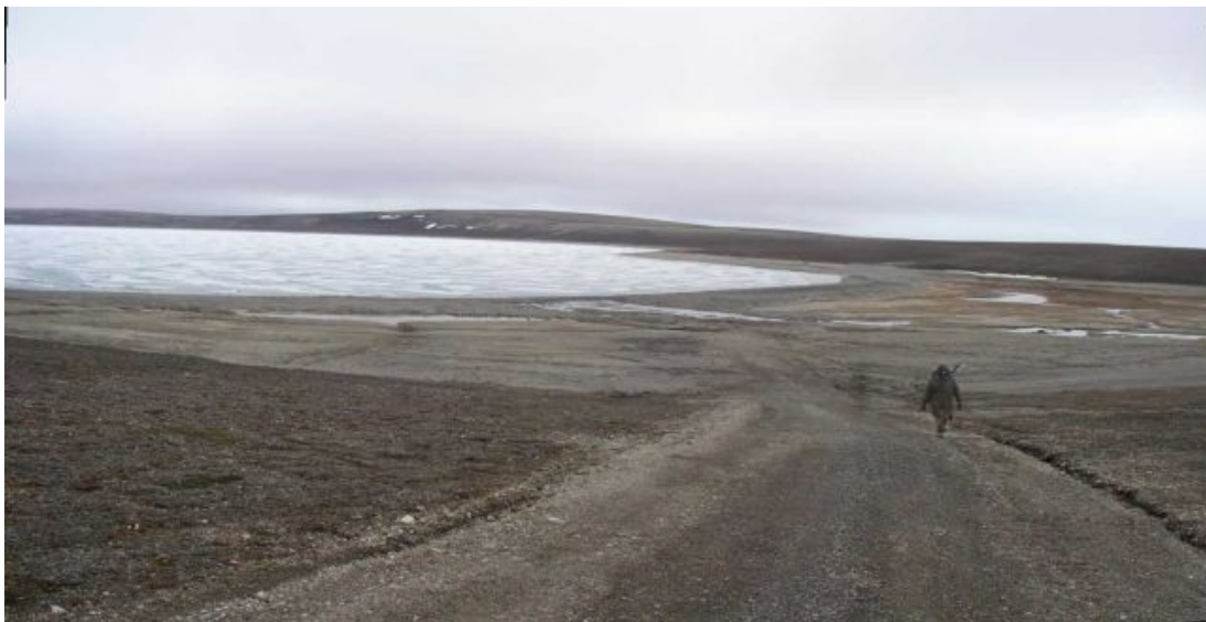
2006 – Panoramic view of Garrow Lake at left and wave break structure in the centre from waypoint GLWB1 on the access road on the western valley side slope. Note that outlet channel has filled in with a 0.4 m thick ridge of beach gravel. Otherwise no major changes have occurred since last inspection in 2005.
