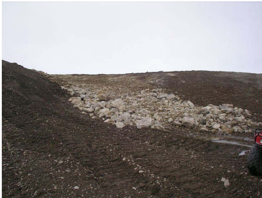
View of toe area of erosion gully showing coarse material placement.
