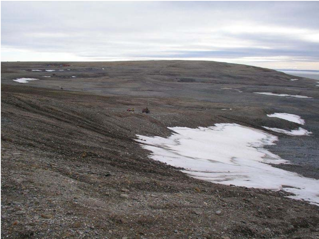
2006 – View looking down west sideslope of New Quarry Extension, where stripped organic surficial soil has been spread. Occasional cracks but no signs of mass movement presenting any hazard to humans or wildlife, with no significant change since last inspection in 2005.
