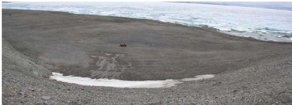
2006 – Slope above Main Portal area is inclined at about 26 degrees, locally steepening to 35 degrees. Minor slumping was observed, but not considered to present hazard to humans or wildlife.
