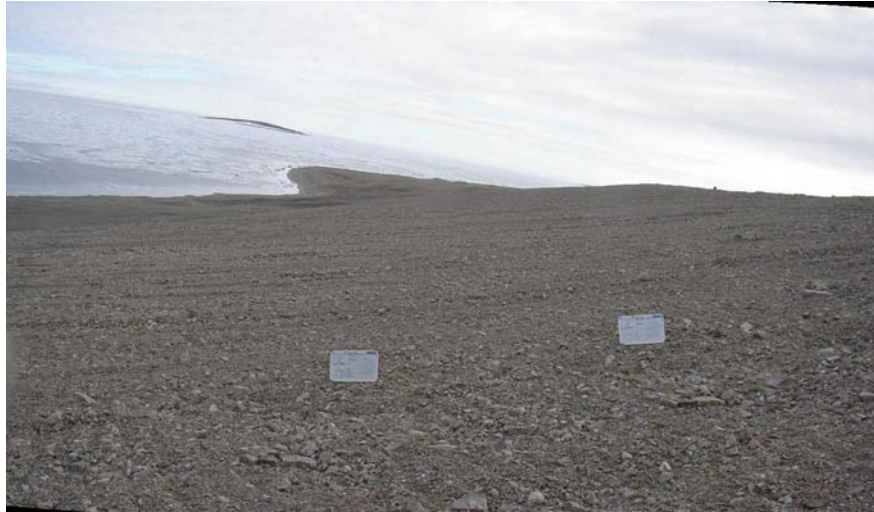
View southwest along main side slope of the Operational Landfill from waypoint OLF3, again showing slopes in good condition, free of any erosion or deformation, as previously observed in 2005.
