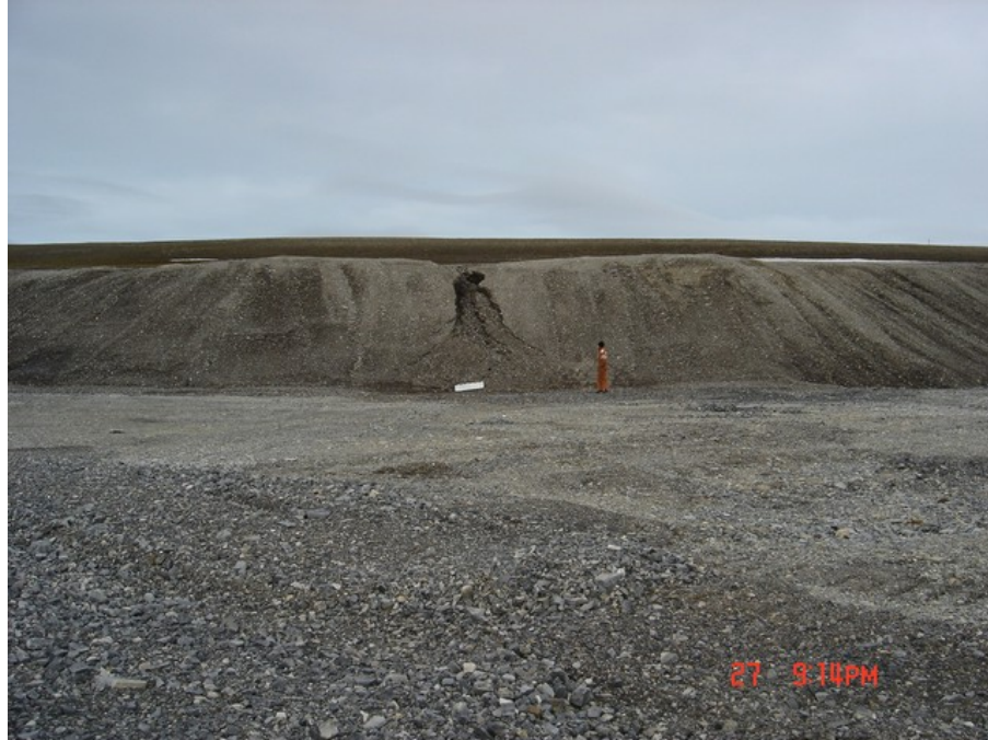
2005 – Isolated erosion gully at waypoint NQ2 PH1.
