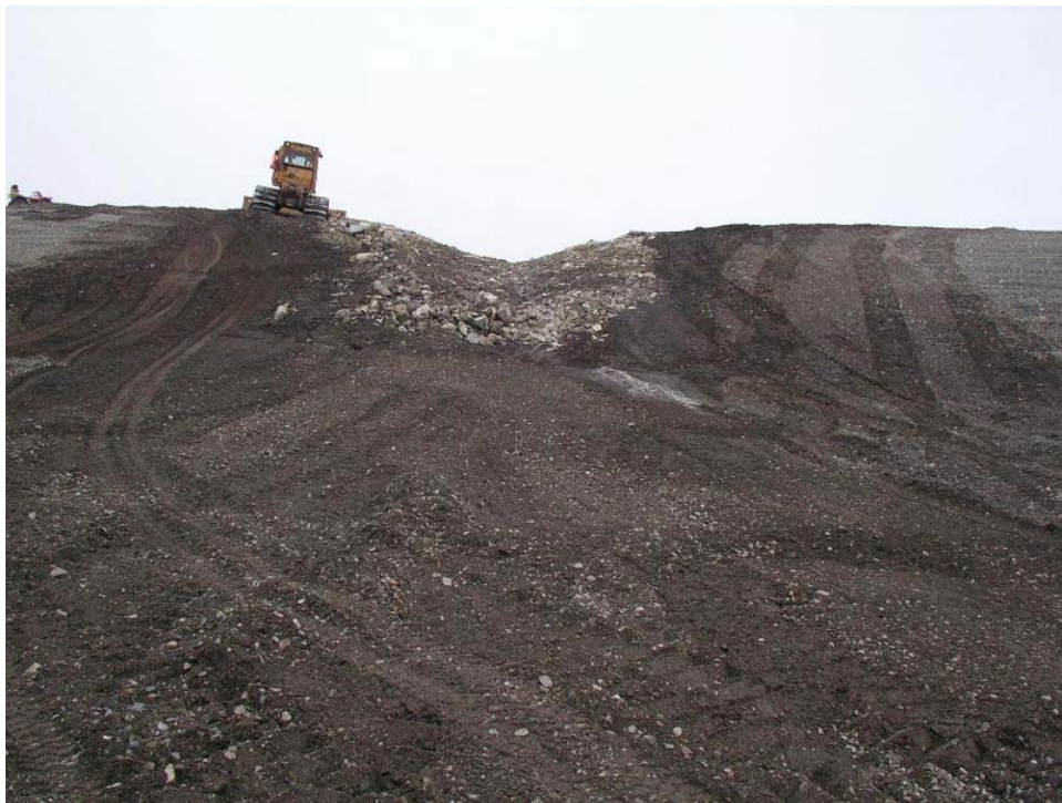
View upstream of waypoint NQ0602 showing v-shaped armoured swale.
