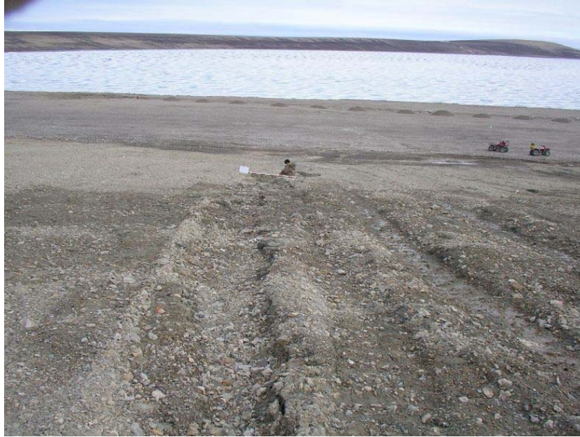
View down slope from waypoint LO SPR TOP. The degree of erosion is not serious and appears to be gradually self-armouring, and is virtually identical to observed conditions in 2005 .
