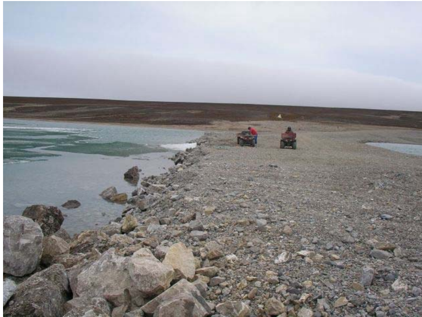
2006 – View from waypoint FL1 looking east towards shoreline. Conditions appear virtually unchanged since observed in 2005, with some minor loss of finer material exposing coarse rockfill.
