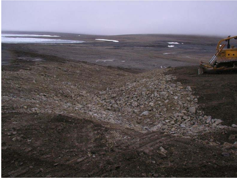
View downstream from waypoint NQ0603 showing wide swale of armoured channel.
