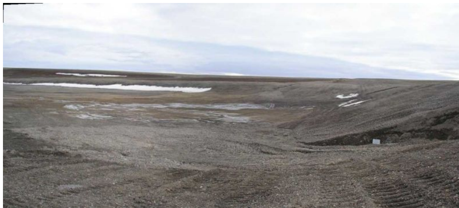
2006 – Debris fanning across floor of New Quarry from erosion gully where Loon Creek drains across a fill embankment. Little change was observed in the overall nature of this feature since inspected in 2005.
