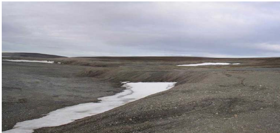
2006 – Area above waypoint NQ5 view looking northeast across area of disturbed surficial soil bordering edge of quarry side slope. Illustrates typical pattern of surficial deformation caused by seasonal thaw of disturbed surficial soils. This poses no threat to humans or wildlife, and no discernible changed observed since last inspected in 2005.
