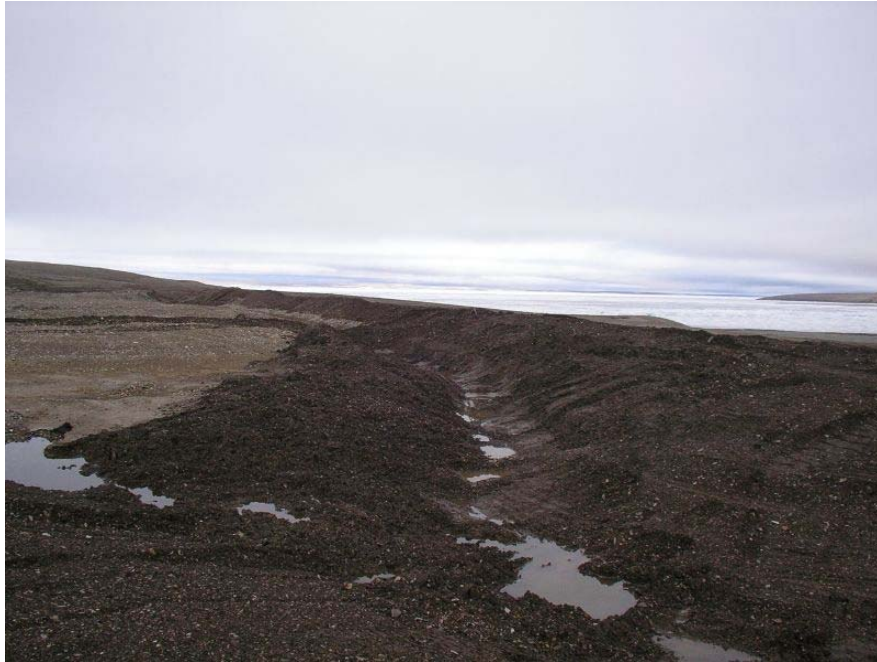
View west showing area between two erosion gullies where, as part of remediation swale has been cleaned out and material raised and rounded off to deter over-topping of any ponded water in future runoff events.
