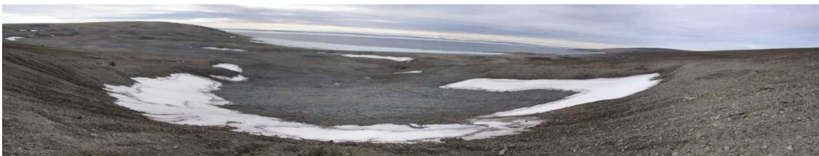
2006 – Panoramic view looking west down slope into extension of New Quarry, from waypoint NQ1 PH2, shows area of disturbed soil, which appears to be stable, with no discernible change since inspected in 2005.
