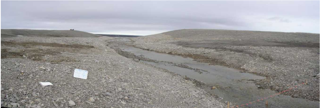
View looking upstream from waypoint GLD4 of overall breached dam and rip-rapped channel. No significant changes are discernible since the previous inspection in 2005.
