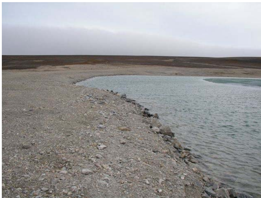
2006 – View from waypoint FL2 looking towards shoreline along west side of causeway. No sign of deformation observed along this side. Some loss of fines has occurred at waters edge, but no signs of major instability.
