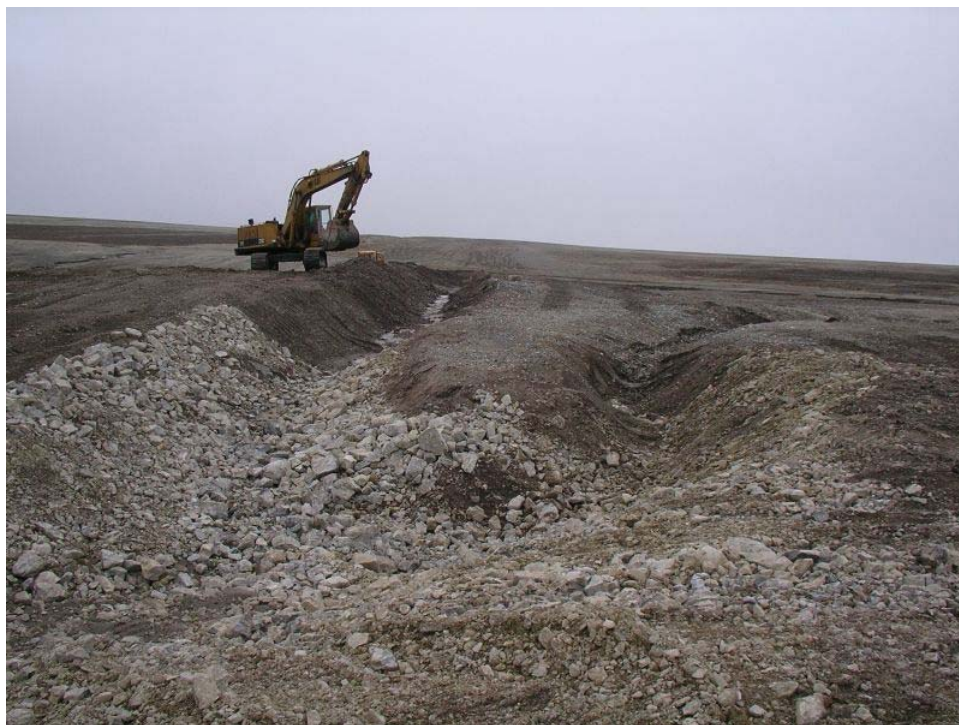
View upstream of waypoint NQ0603 showing broad extent of placement of rockfill armouring.
