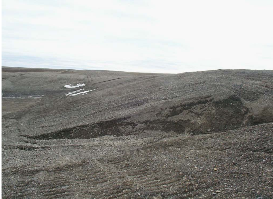
2006 – View adjacent and immediately to west of view shown above showing significant erosional down cutting of what appears to be quarry strippings of silty sand and gravels.
