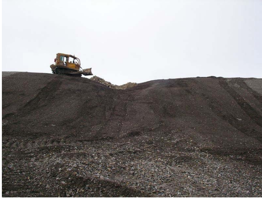
Placement of well graded rockfill in a v-shaped swale after sides-slopes re-shaped.
