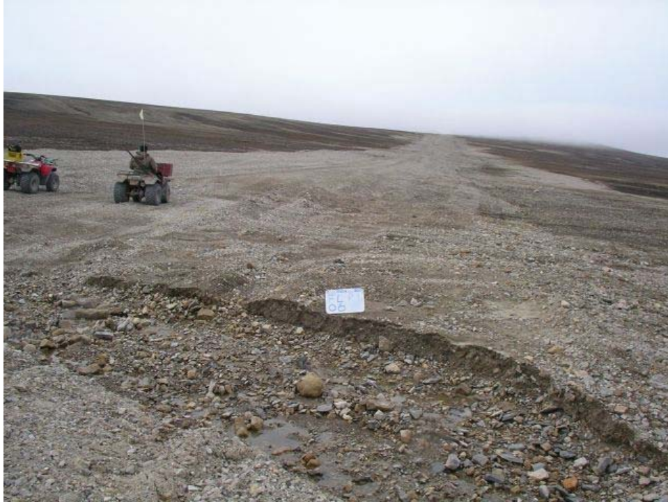
2006 – Access roadway at waypoint FLR 06 1 view to the southwest at about 200 m distance from intake causeway. Erosion is localised, shallow, and appears to be self armouring.
