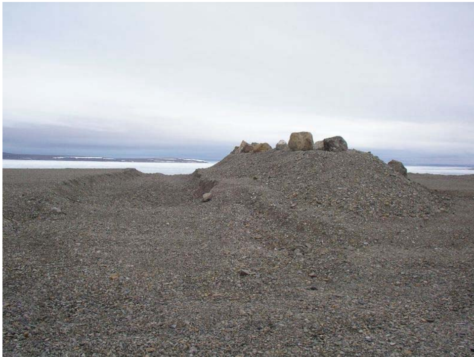
View of the terrain adjacent to the north end of the airstrip, and of the safety berm around the upper edge of the LRD quarry slopes. The berms are in good condition.
