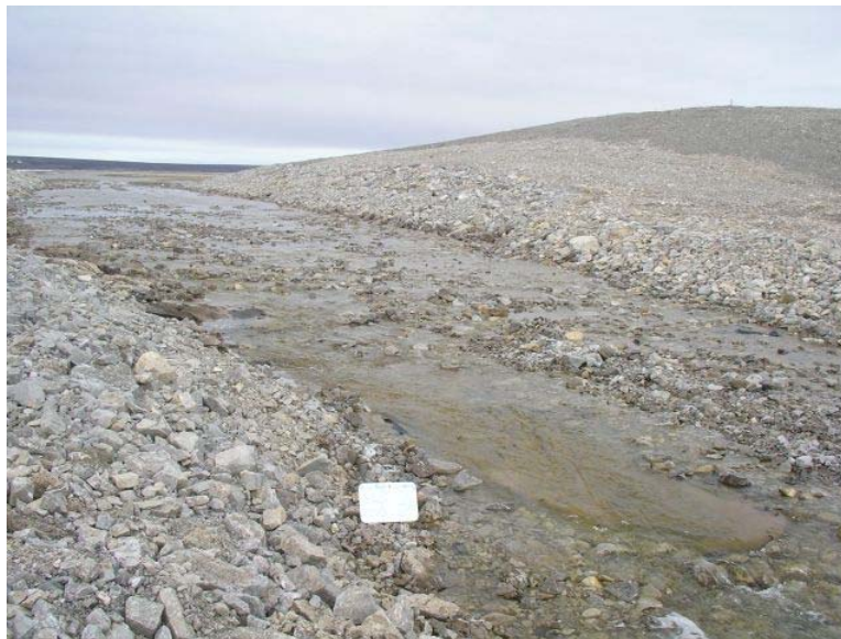
View from 30 m downstream of waypoint GLD3 at a point where channel gradient increases. Filter fabric underlying the rip-rap material was observed in 2005 to be exposed over a width of 3 to 4 m and over a length of about 10m. Conditions appear not to have changed significantly since then. The integrity of surrounding rip-rap does not appear to have been affected. Remedial action to replace rip-rap is recommended as a precaution in 2007.
