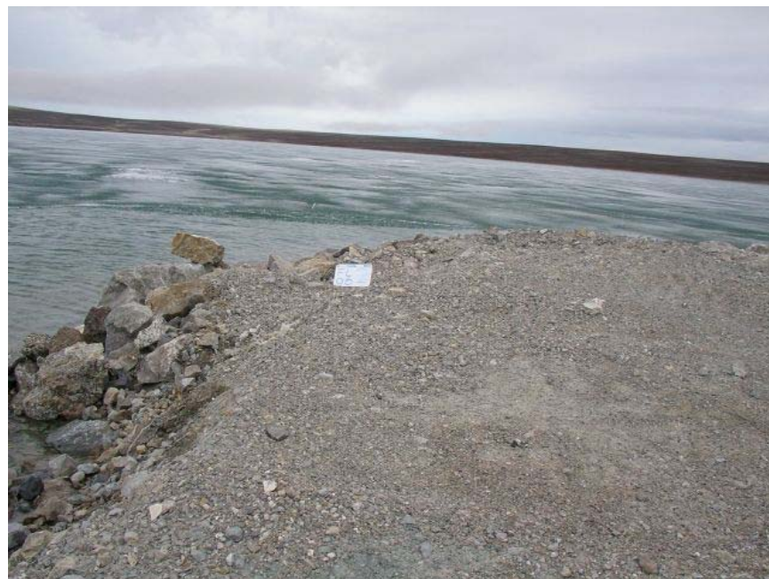
2006 – View from waypoint FL2 looking across northern end of causeway – previously observed subsidence in 2005 near sign remains unchanged, with vertical separation of about 0.3 m over a width of 2 m. As shown in photo from waypoint FL1, corner at lower left has been eroded exposing coarse rockfill. Surrounding fill across crest of causeway appears unaffected and stable.
