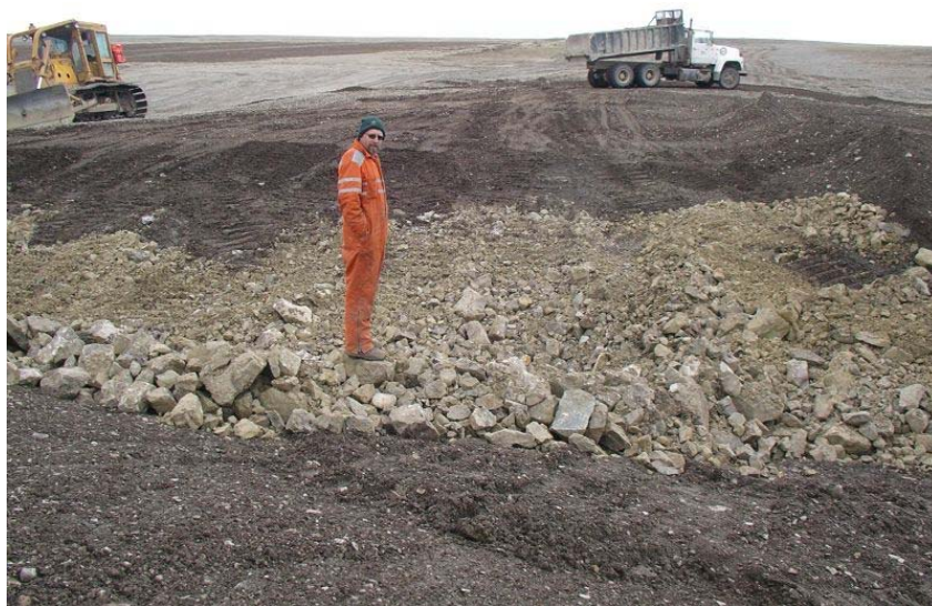
Limestone rockfill being place in the upper part of the erosion gully.
