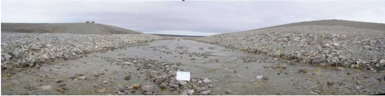
View northwards at waypoint GLD3, looking upstream along creek channel, showing rip-rap lining, which is in good condition. Flow is moderately uniform across channel, with high clarity. Conditions appear to be unchanged since previously inspected in 2005.
