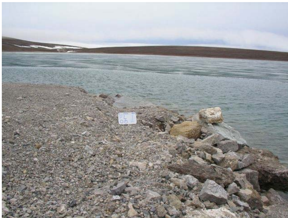
2006 – View from waypoint FL1 looking across end of causeway – note slight subsidence in foreground and significant erosion of finer material at far corner.
