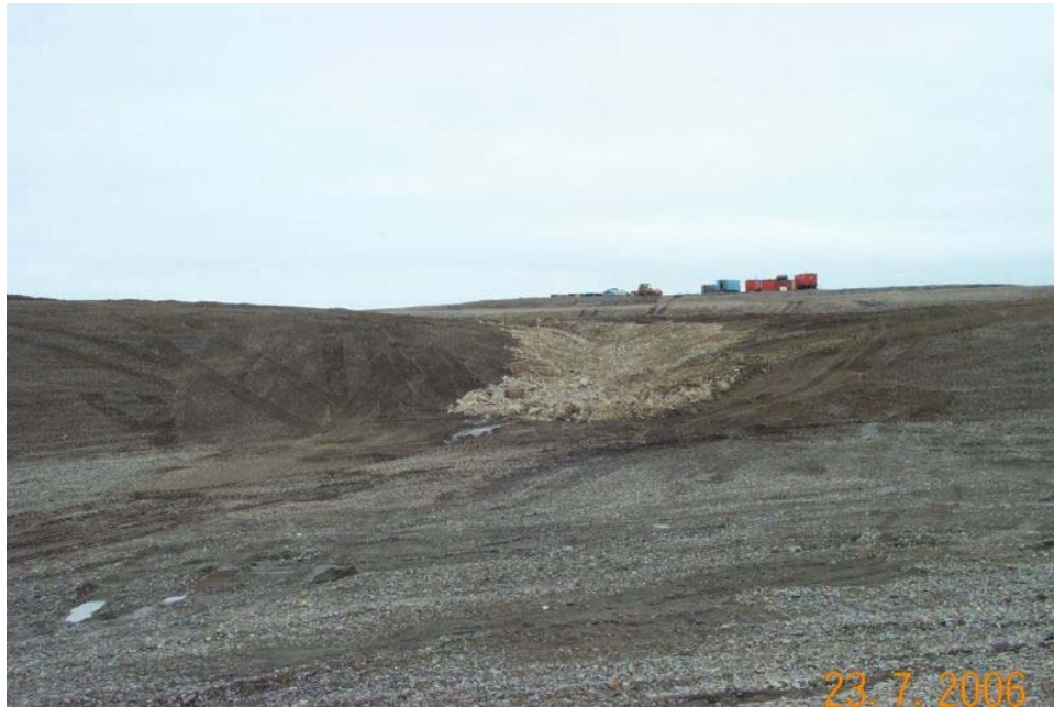
View of westernmost erosion gully after completion of remedial works with coarse material extending beyond toe of embankment fill.
