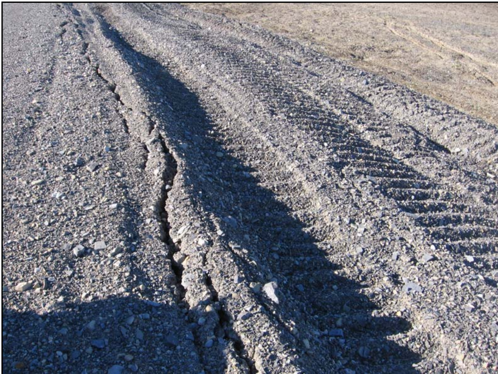
Photo 14 - Northing: 8367721 Easting: 560837 Elevation: 57 m. Tension crack along road
