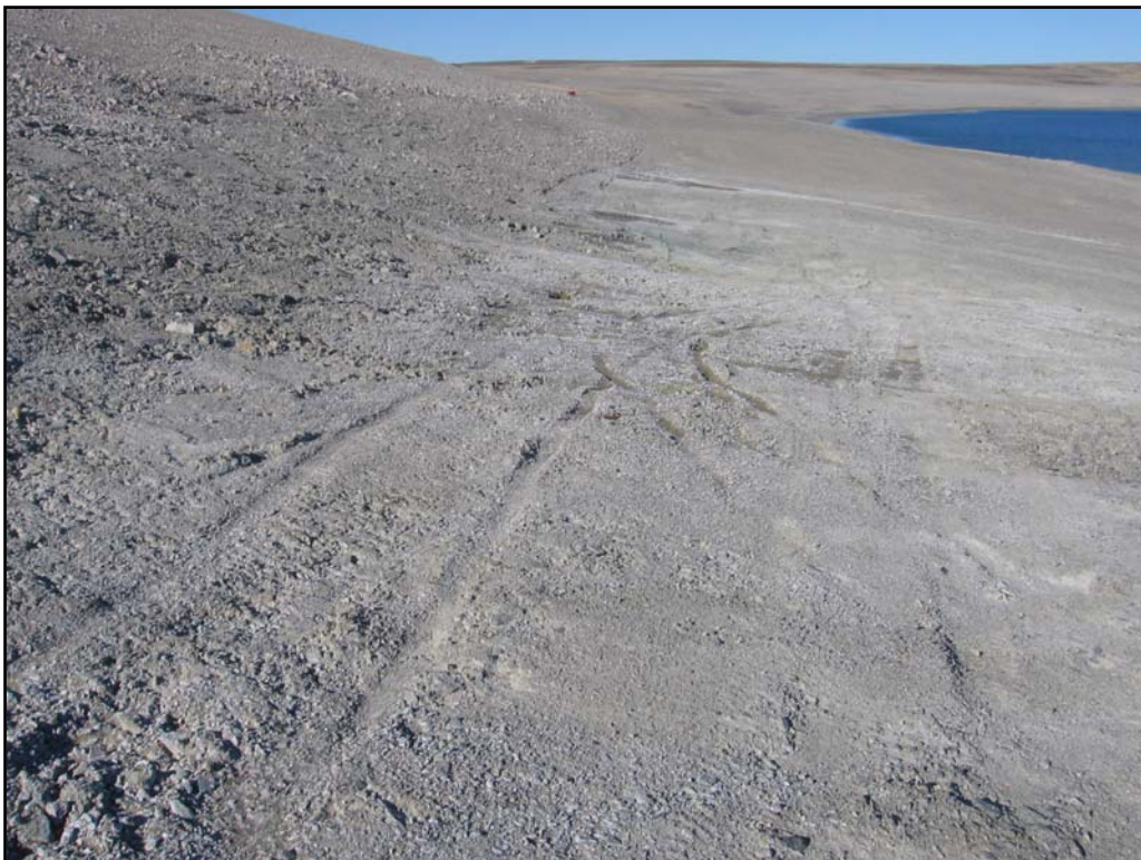
Photo 10 - Northing: 8367408 Easting: 558917 Elevation: 9 m. Operational landfill; Seepage from toe and white precipitate
