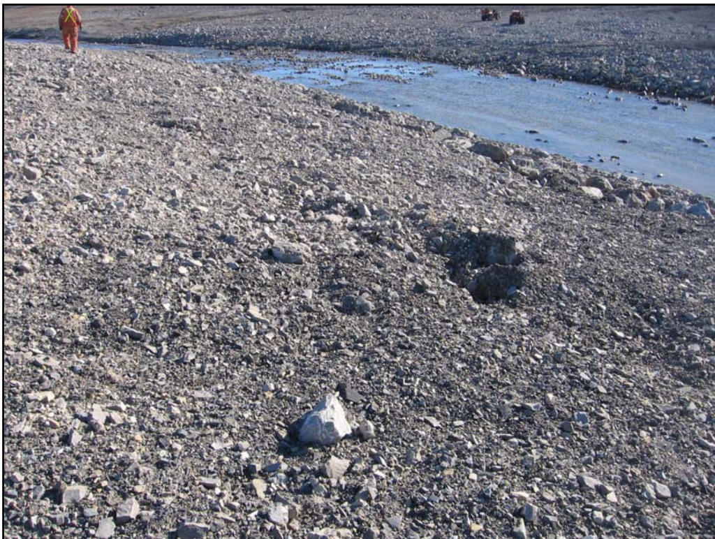
Photo 24- Northing: 8366999 Easting: 561646 Elevation: 15 m. Garrow dam; loose evidence of settling / movement on Southeast abutment above rip-rap
