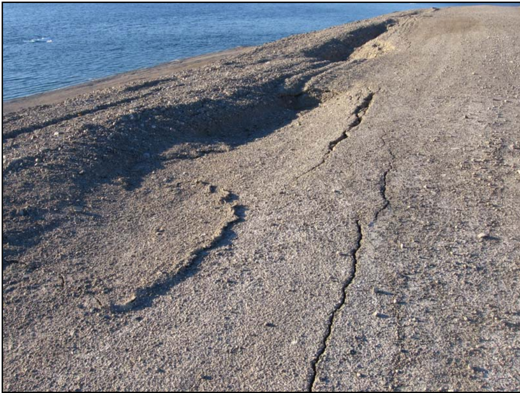
Photo 29- Northing: 8368863 Easting: 557713 Elevation: 38 m. Subsidence/slumping along road to Little Red Dog Quarry
