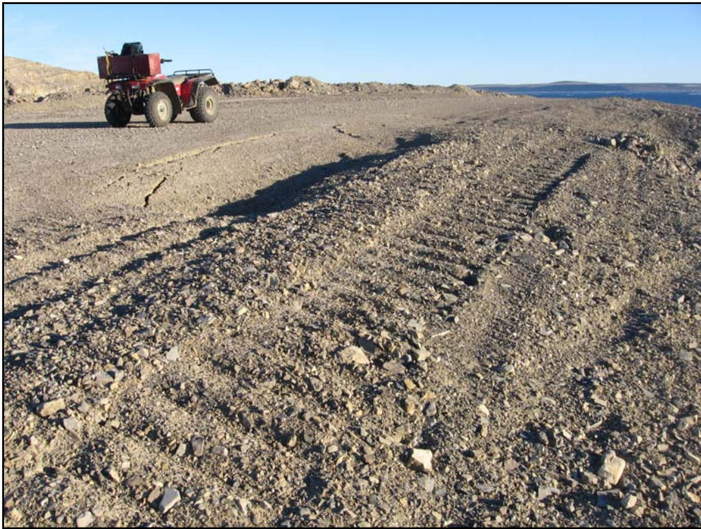
Photo 31- Northing: 8368863 Easting: 557713 Elevation: 38 m. Subsidence/slumping along road to Little Red Dog Quarry
