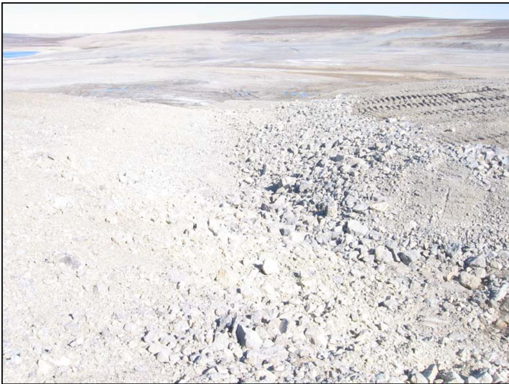
Photo 69- Northing: 8368702 Easting: 558670 Elevation: 36 m. New quarry; rip-rap repaired gully
