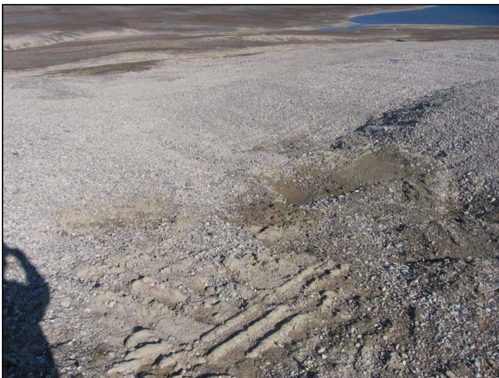
Photo 54- Northing: 8371151 Easting: 560166 Elevation: 52 m. Frustration Lake access road; repaired erosion gully
