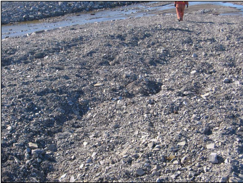
Photo 23- Northing: 8366999 Easting: 561646 Elevation: 15 m. Garrow dam; hummocky / bumpy crest of Southeast abutment
