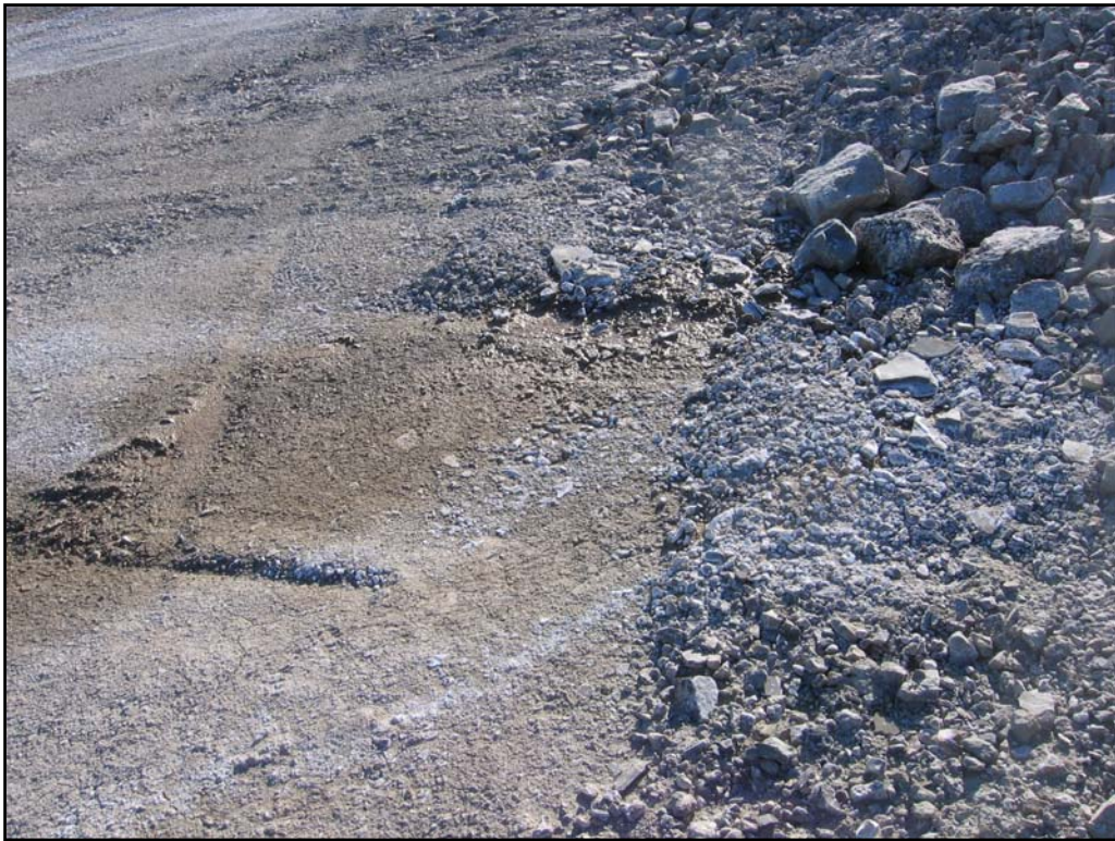
Photo 9 - Northing: 8367408 Easting: 558917 Elevation: 9 m. Operational landfill; Seepage from toe and white precipitate
