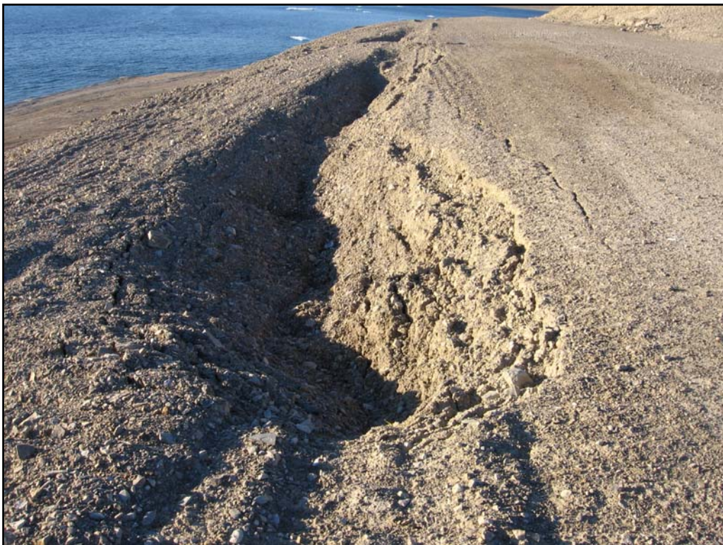
Photo 30- Northing: 8368863 Easting: 557713 Elevation: 38 m. Subsidence/slumping along road to Little Red Dog Quarry
