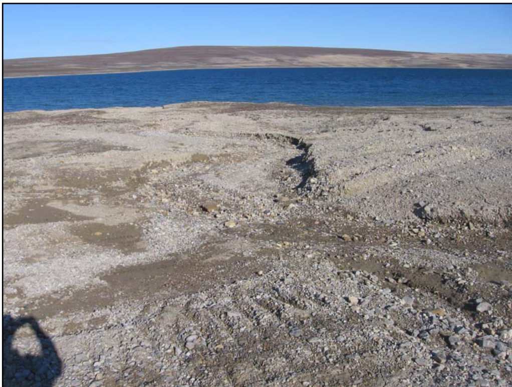
Photo 53- Northing: 8371827 Easting: 560363 Elevation: 22 m. Frustration Lake access road; erosion gully facing downstream of road
