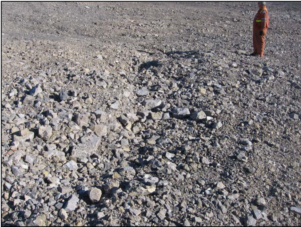
Photo 25- Northing: 8366999 Easting: 561646 Elevation: 15 m. Garrow dam; lower bumpy slope from snow / ice fill or slope movement
