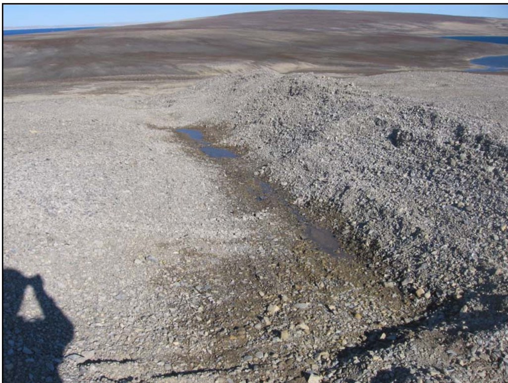
Photo 56- Northing: 8371018 Easting: 560120 Elevation: 57 m. Frustration Lake access road; repaired erosion gully with water bar
