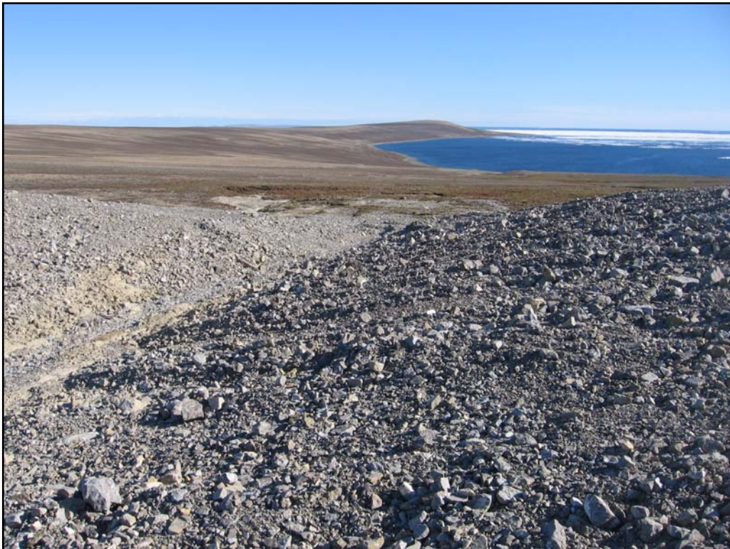
Photo 12 - Northing: 8368751 Easting: 559743 Elevation: 46 m. Drainage crossing through road with downstream erosion
