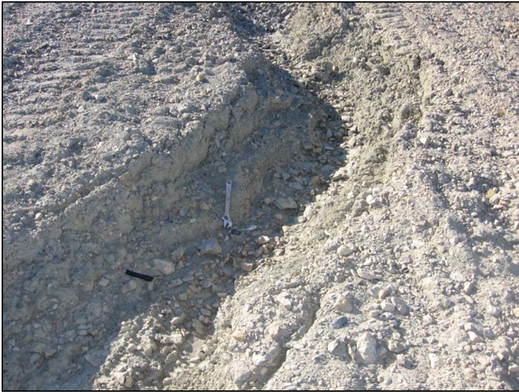
Photo 7 - Northing: 8367615 Easting: 558780 Elevation: 33 m. Operational landfill; View of erosion gully on slope above the landfill (Scale: Wrench is 0.3 m)
