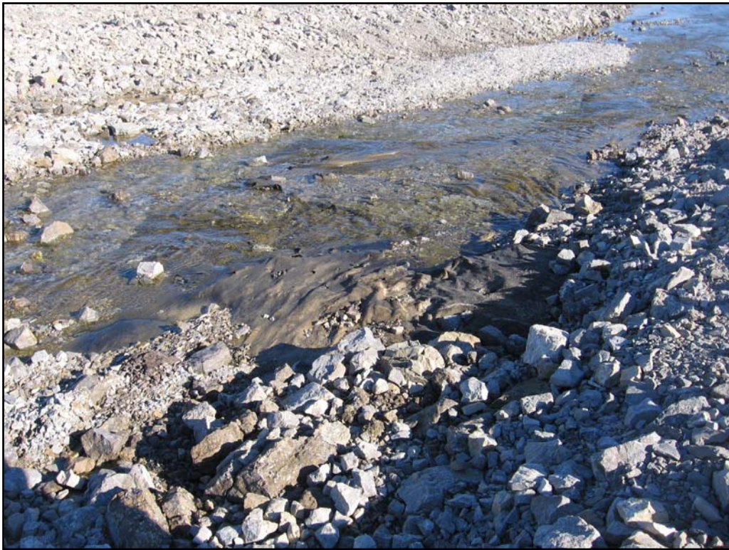
Photo 19- Northing: 8366909 Easting: 561646 Elevation: 15 m. Garrow dam; exposed geotextile
