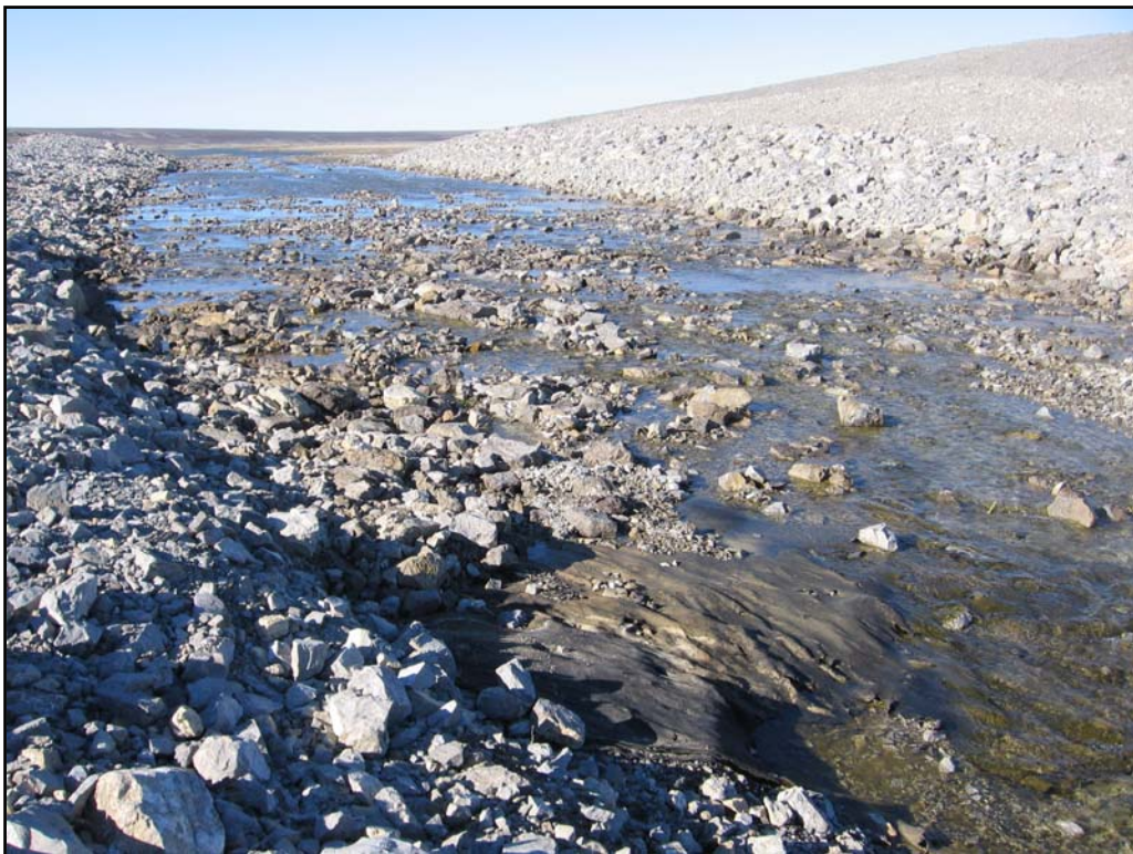
Photo 18- Northing: 8366909 Easting: 561646 Elevation: 15 m. Garrow dam; exposed geotextile
