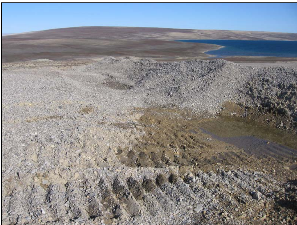
Photo 58- Northing: 8370930 Easting: 560085 Elevation: 61 m. Frustration Lake access road; repaired erosion gully with water bar
