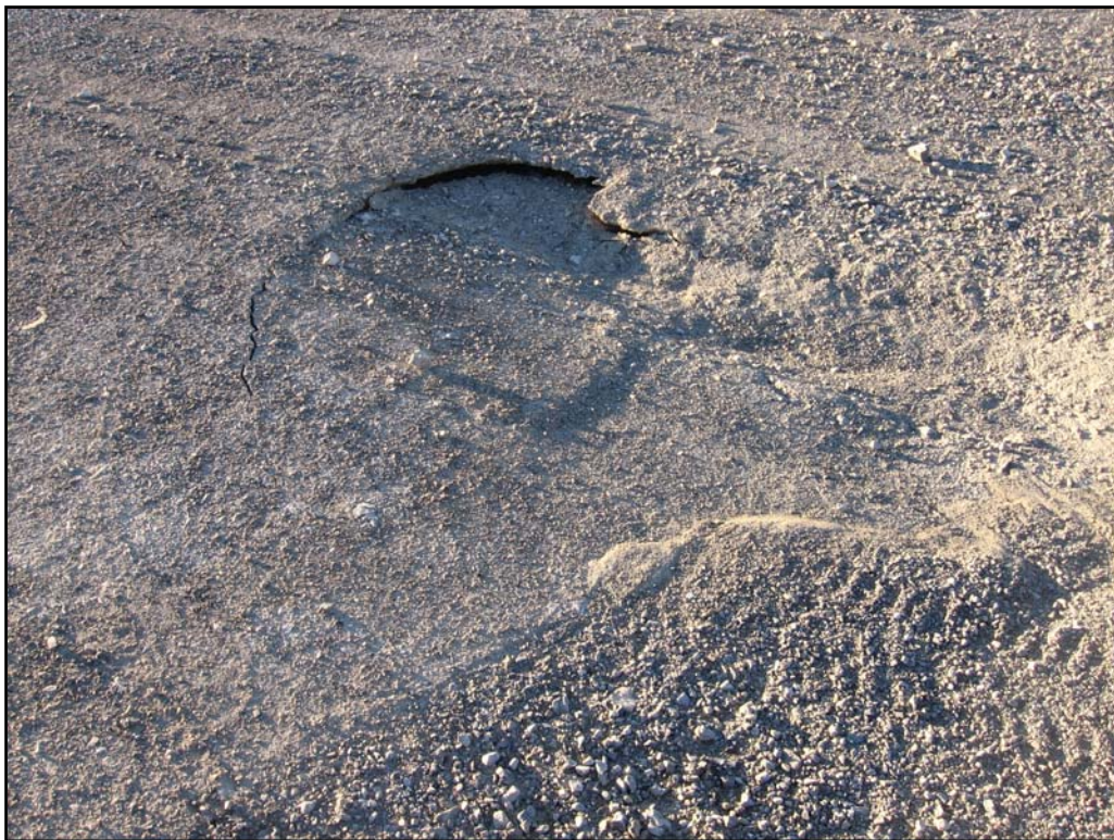
Photo 35- Northing: 8368499 Easting: 558491 Elevation: 49 m. Crack / settlement in middle of road likely from melting of entrained snow or ice
