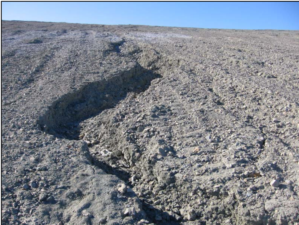
Photo 6 - Northing: 8367615 Easting: 558780 Elevation: 33 m. Operational landfill; View of erosion gully on slope above the landfill
