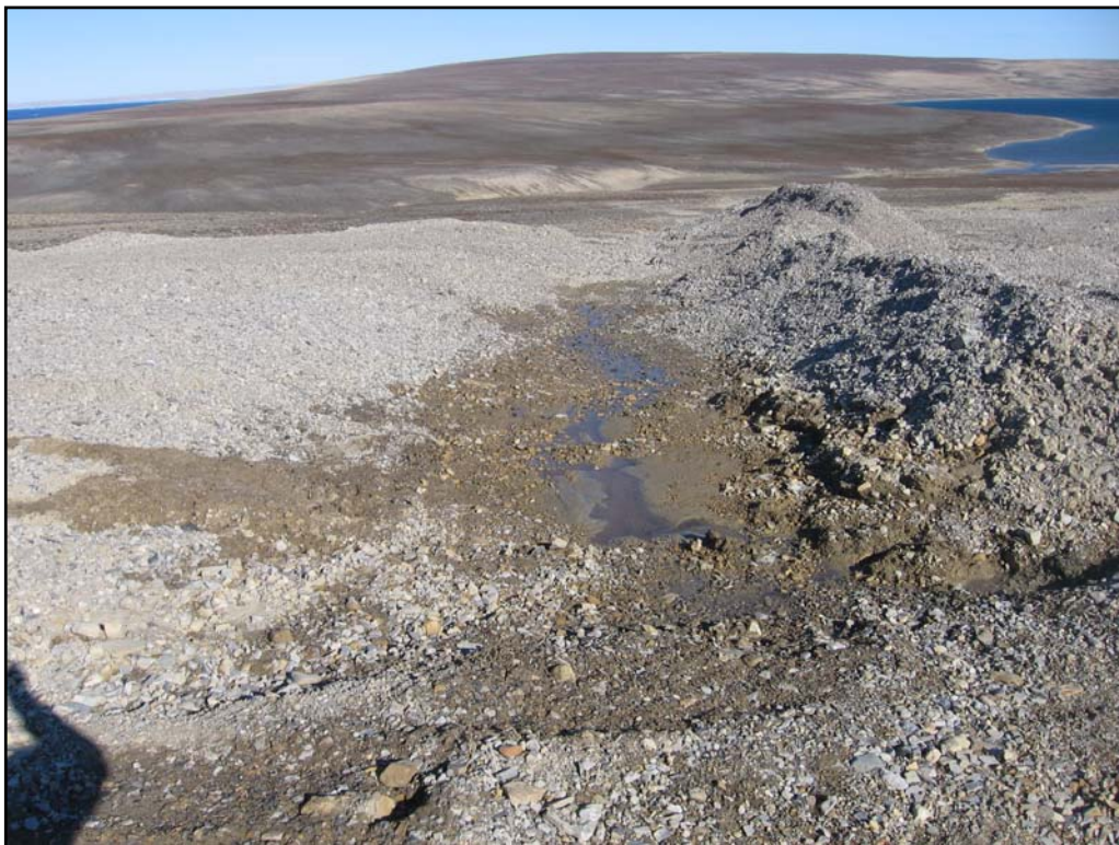
Photo 57- Northing: 8370978 Easting: 560105 Elevation: 60 m. Frustration Lake access road; repaired erosion gully with water bar
