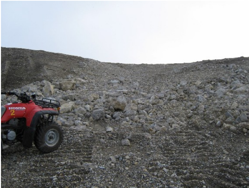
Photo 109- Northing 558699 Easting 8368752 Elevation 28 m New quarry area: rip-rap lined drainage ditch
