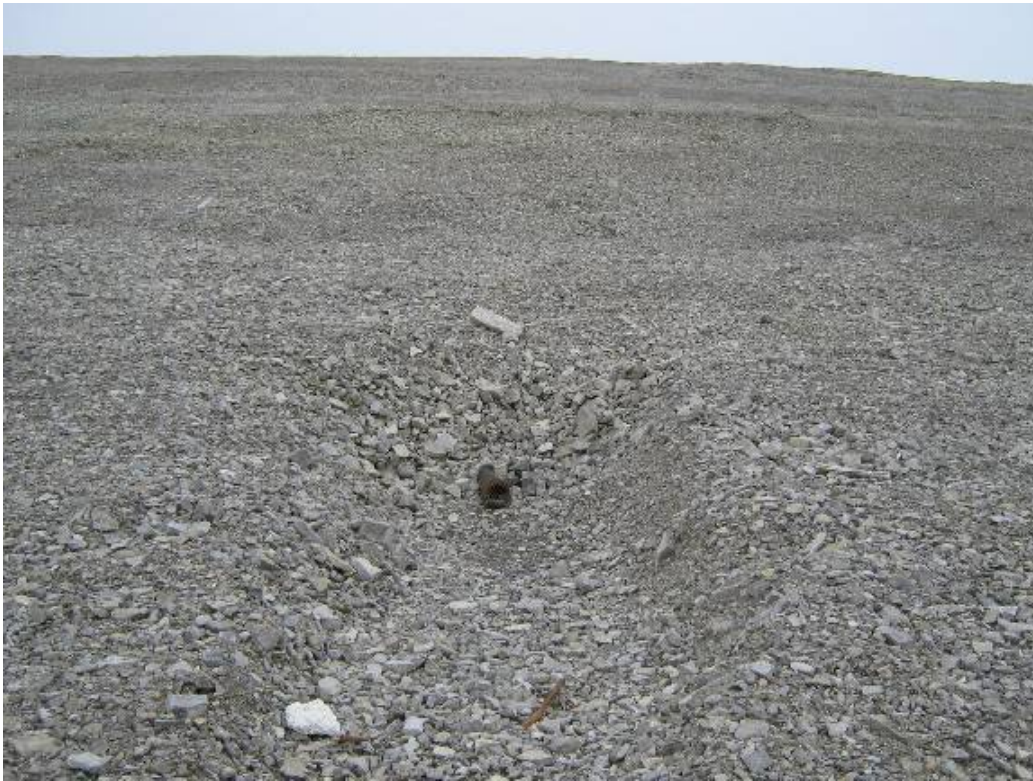
Photo 34- Northing 557829 Easting 8368182 Elevation 23 m Exploration portal: black hole pipe drain covered with wire mesh
