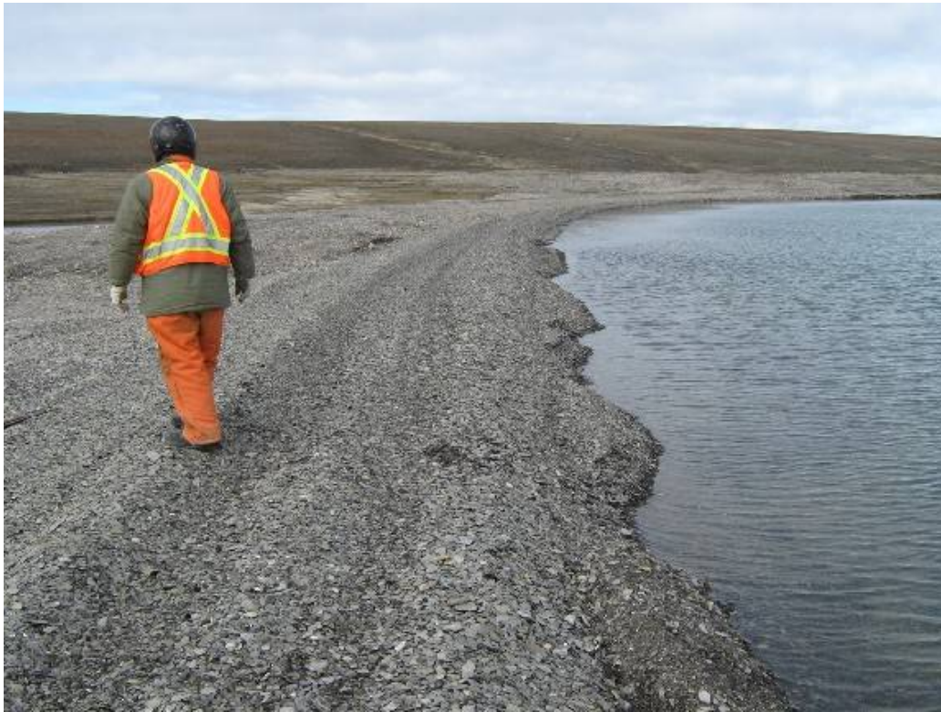
Photo 80- Northing 561569 Easting 8367440 Elevation 8 m Crest of deposited gravel berm along wave break structure
