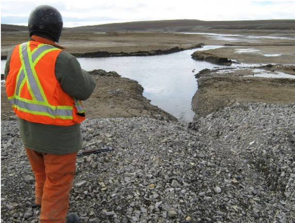
Photo 82- Northing 561569 Easting 8367440 Elevation 8 m Seepage through wave break structure causing some settlement from piping
