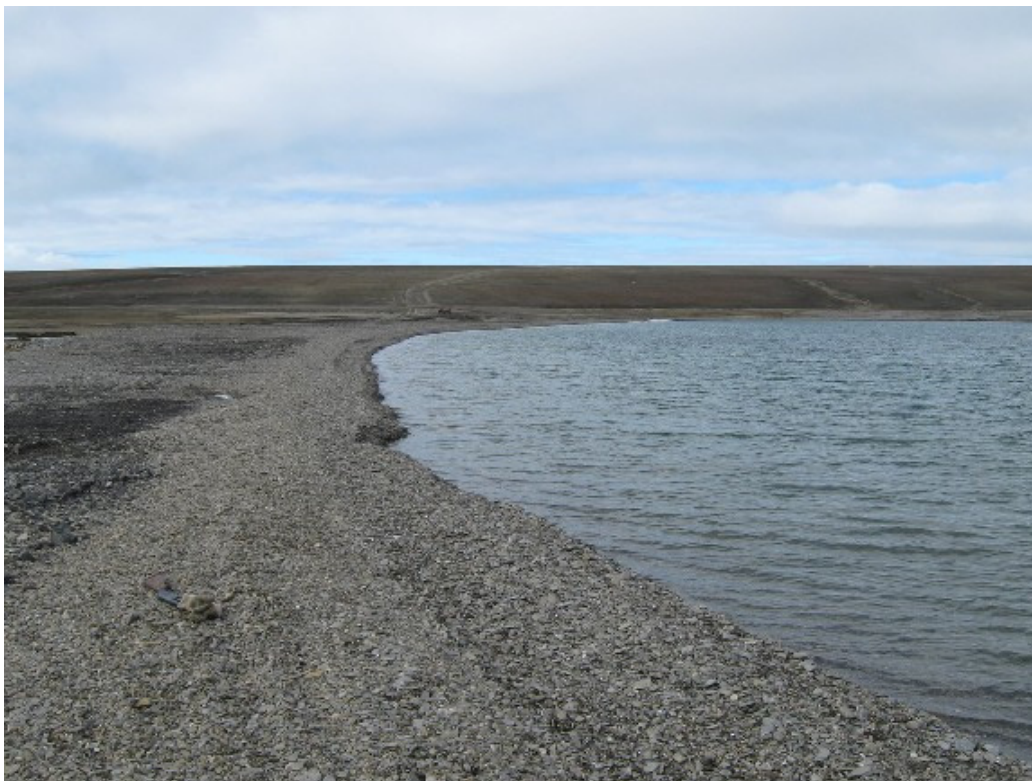
Photo 81- Northing 561569 Easting 8367440 Elevation 8 m Crest of deposited gravel berm along wave break structure
