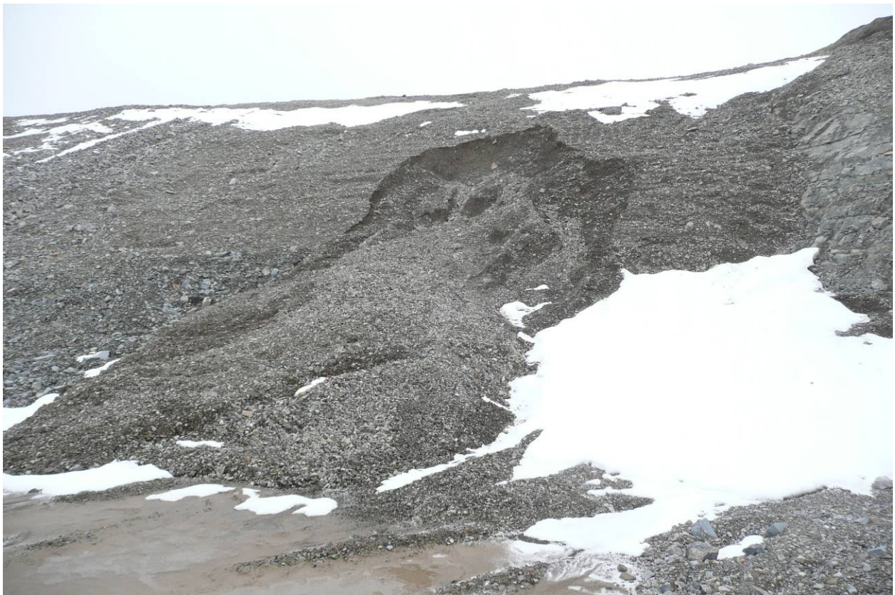
Main Portal Slope Failure (Close-up) – August 24, 2008
