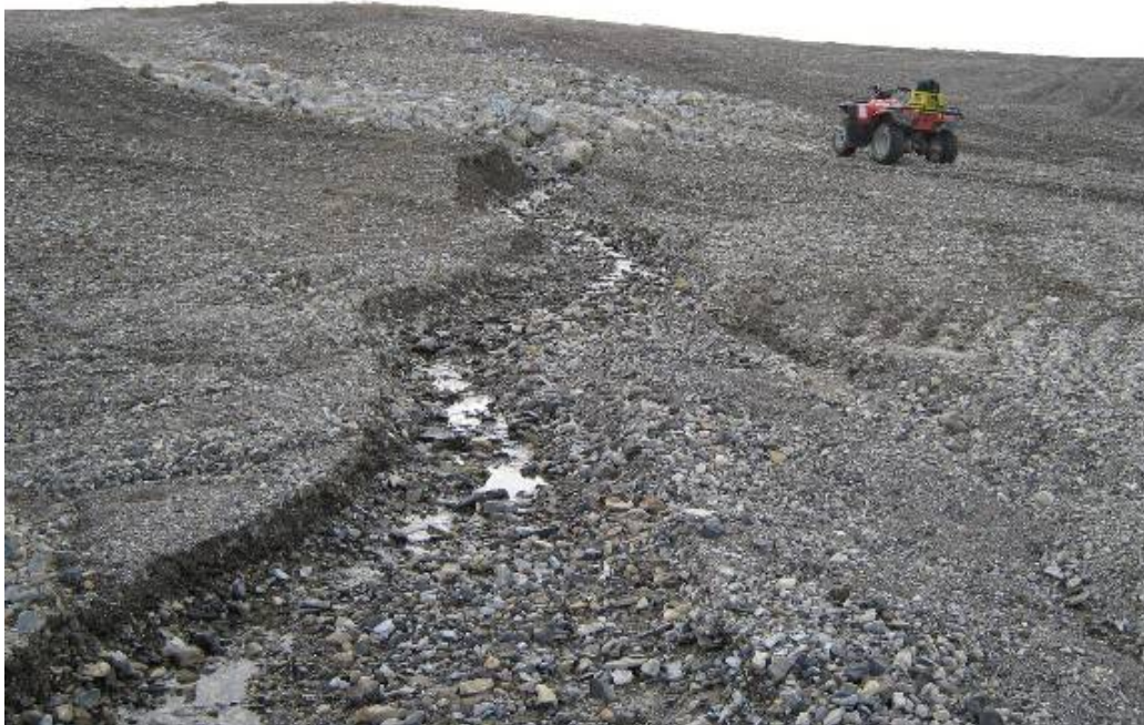
Photo 110- Northing 558699 Easting 8368752 Elevation 28 m New quarry area: erosion gully below rip-rap lined ditch
