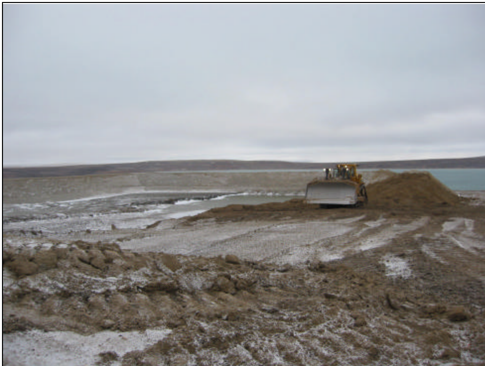
Photo 30 – Bulldozer decommissioning the Tailing Thickener berm
