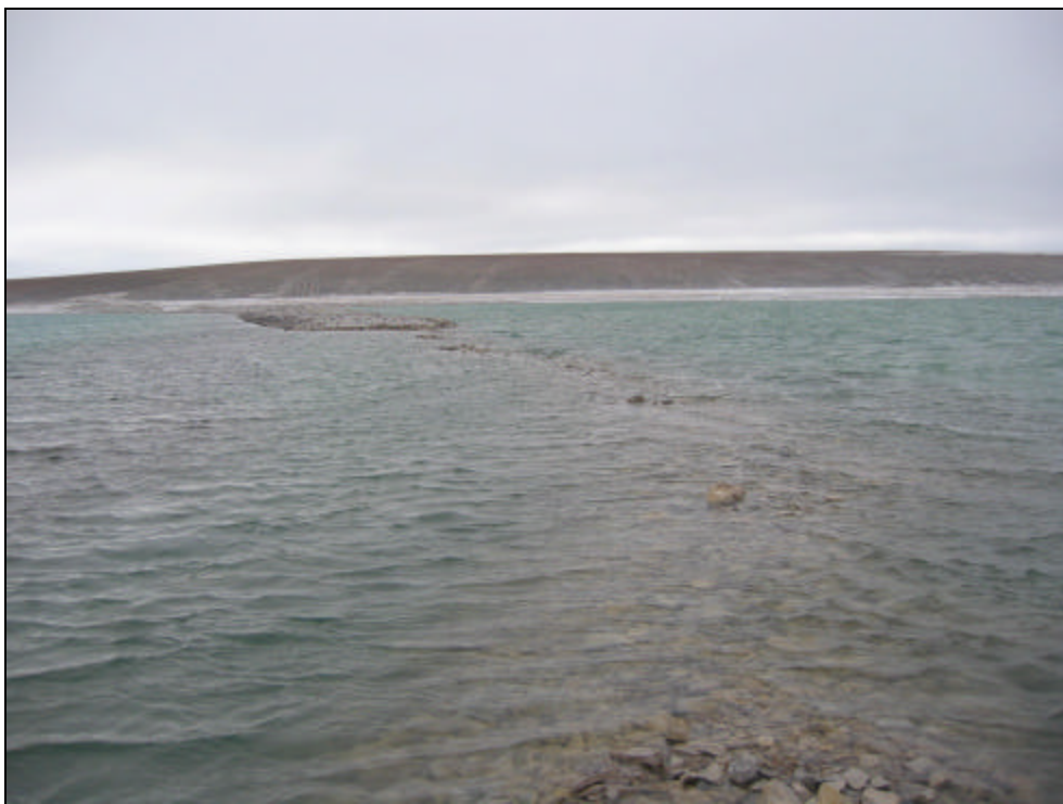
Photo 28 – Wave break structure; the structure has become more apparent as the lake level has dropped
