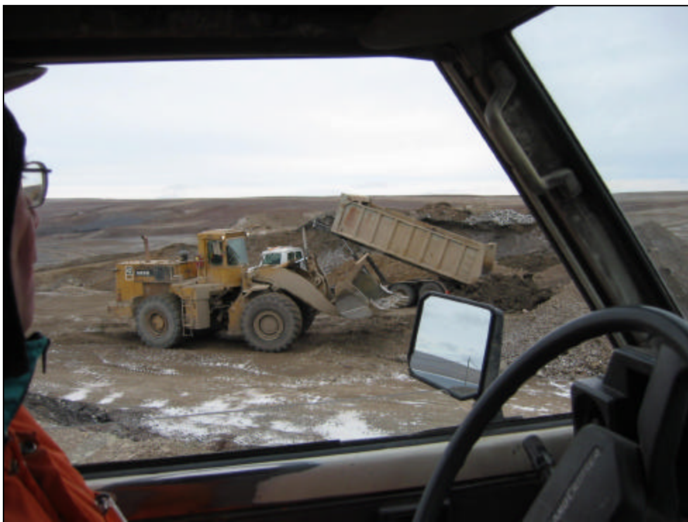
Photo 42 – Front end loader preparing to push contaminated soil underground
