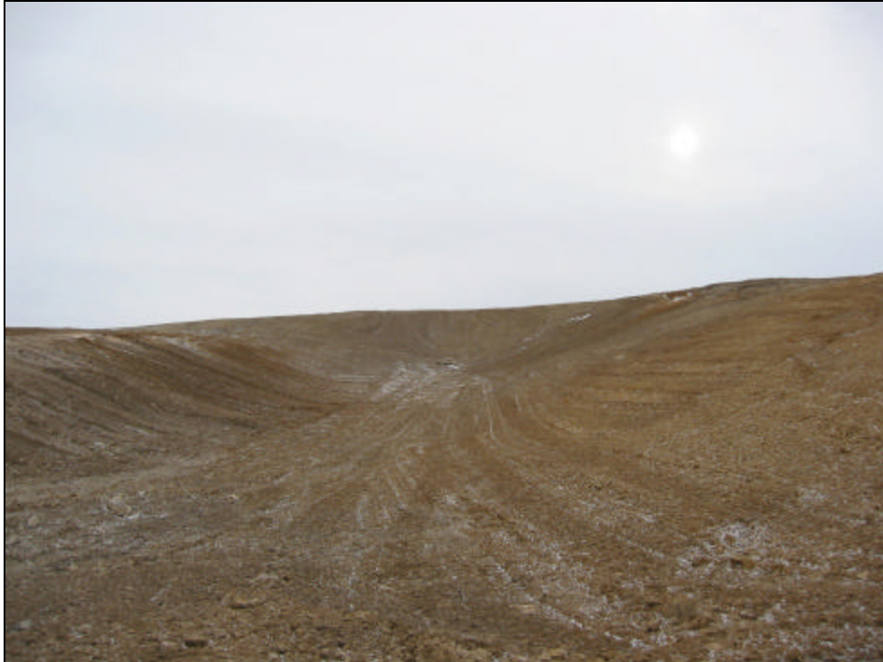
Photo 43 – The sides of the North Pit have been smoothed and recontoured
