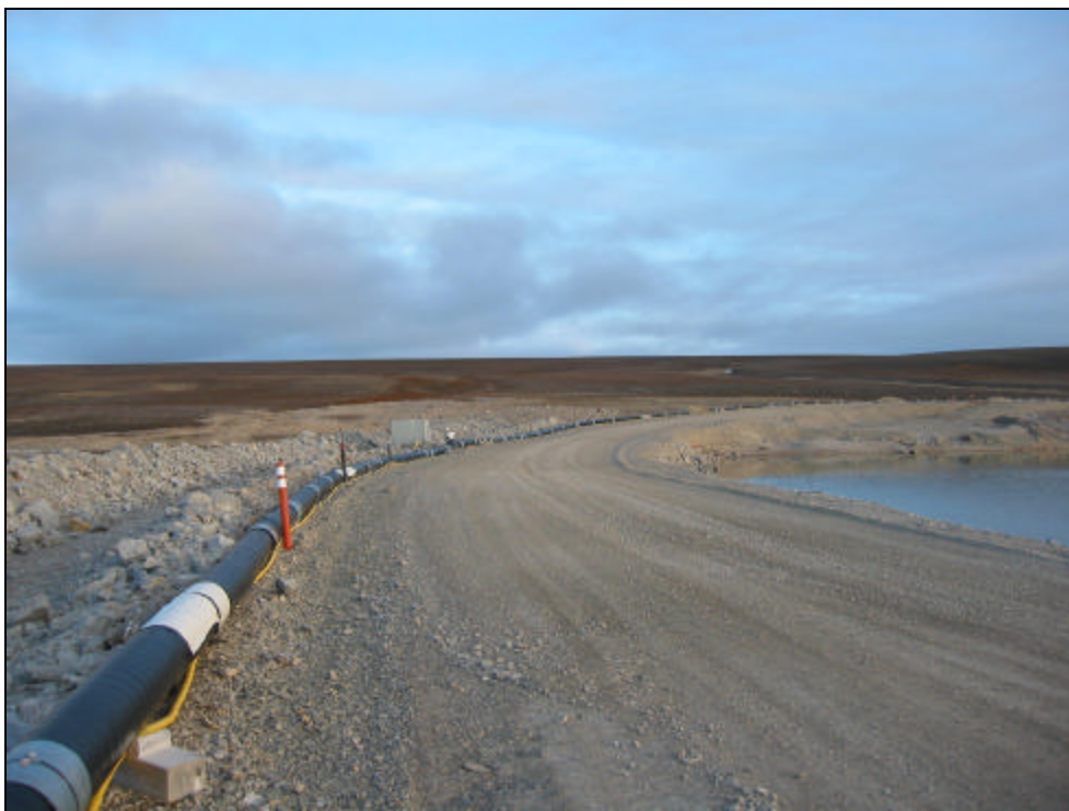
Photo 10 – Insulated water pipe from Frustration Lake to mine
