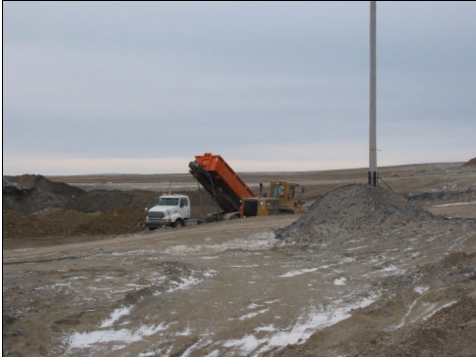
Photo 41 – Dump truck depositing contaminated soil in front of raise borehole
