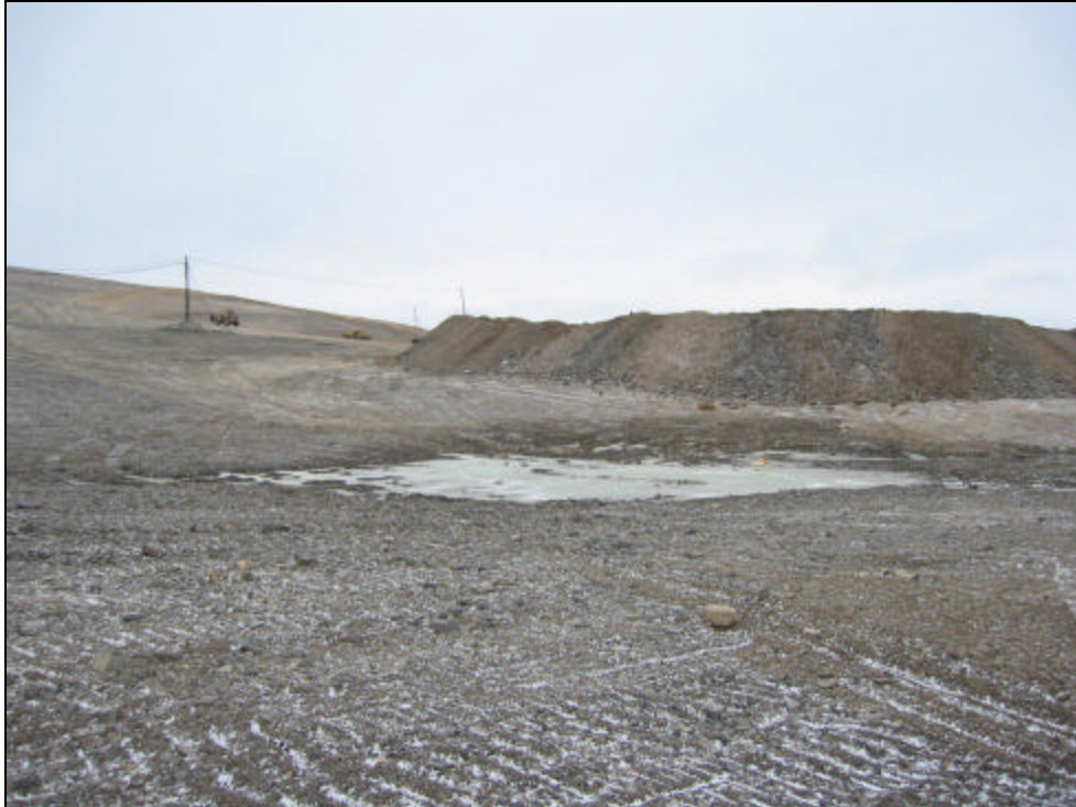
Photo 37 – Water pooling over subsidence zone
