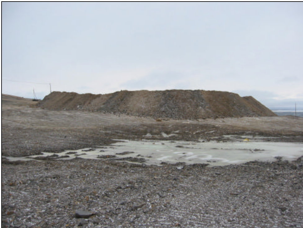
Photo 38 – Close-up of water pooling over subsidence zone
