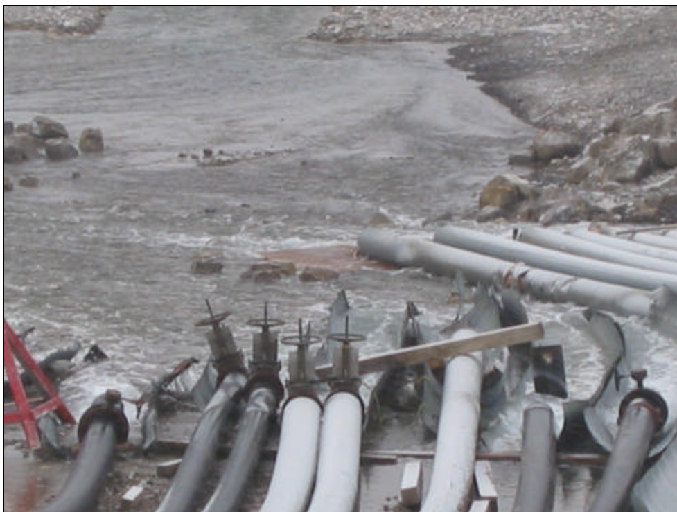
Photo 26 – Close-up of siphons draining lake water into Garrow Creek
