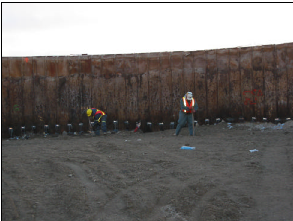
Photo 20 – Workers digging out glycol pipes behind dock pilings
