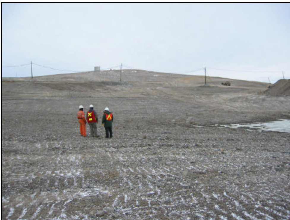
Photo 36 – Inspection group on top of subsidence zone; Teck Cominco has placed shale gravel on top of the site
