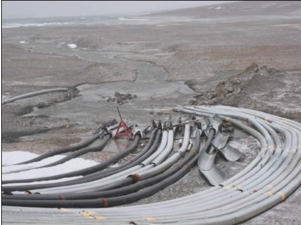
Photo 25 – Siphons draining lake water into Garrow Creek
