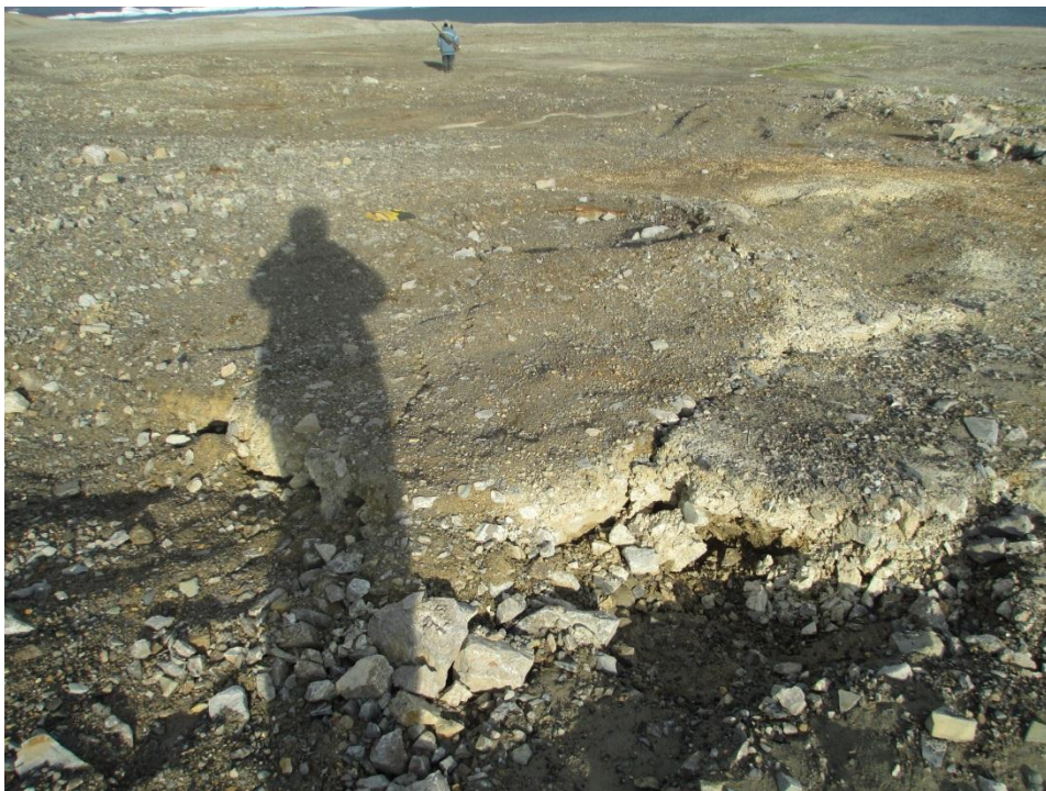
Photo 16, Subsidence Area, thaw settlement adjacent to Vent/Backfill Raise (WP#15)
