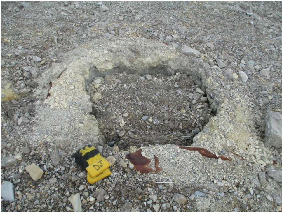
Photos 30, Subsidence Area, Vent/Backfill Raise with ~0.3 m internal settlement (WP#27)
