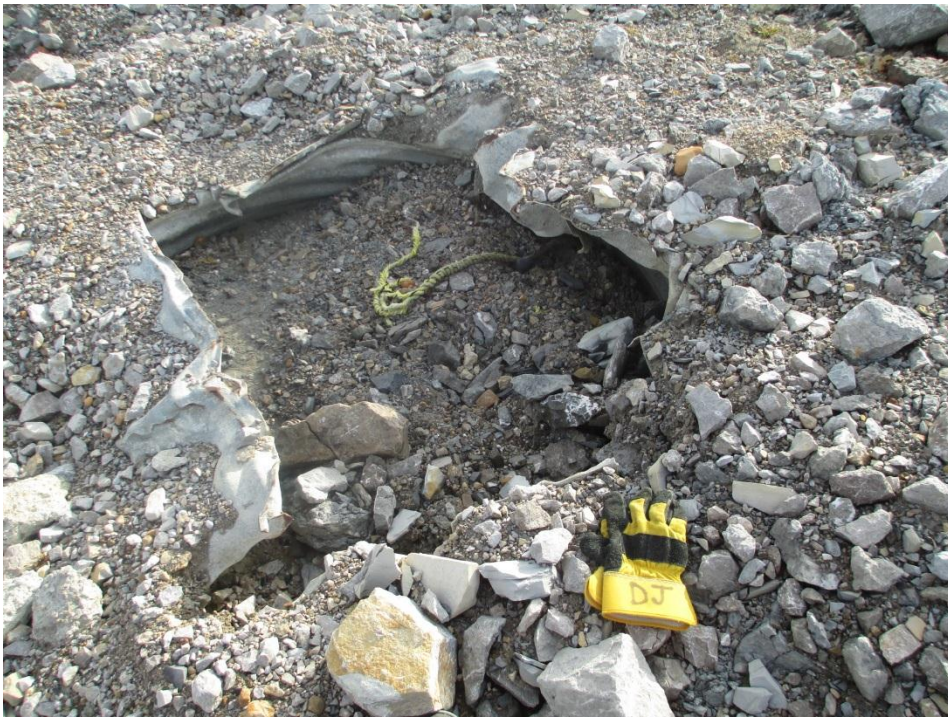
Photo 47, Subsidence Area, Vent/Backfill Raise (WP#40)
