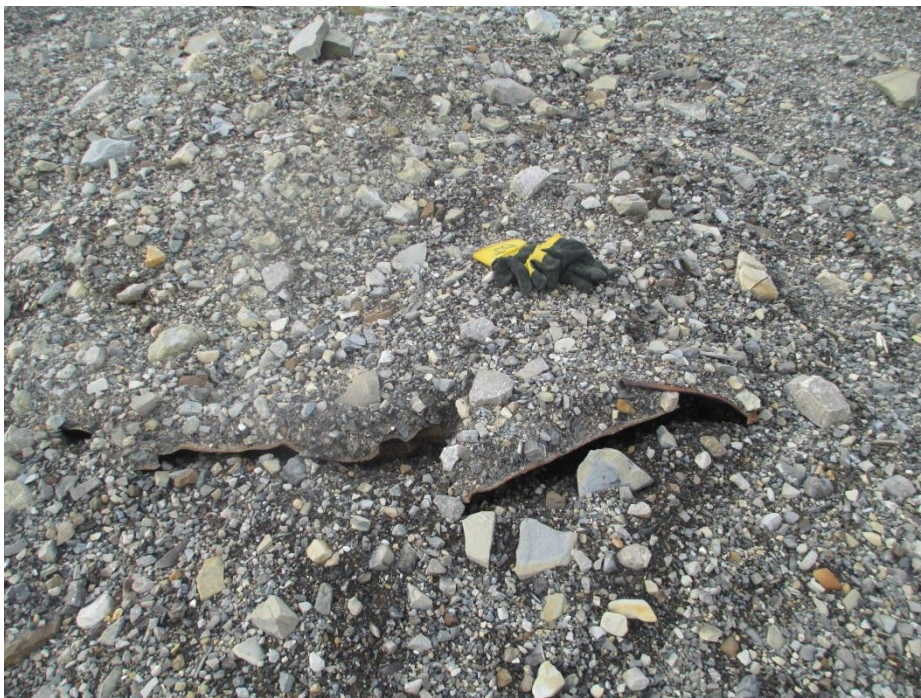
Photo 14, Subsidence Area, Vent/Backfill Raise (WP#13)
