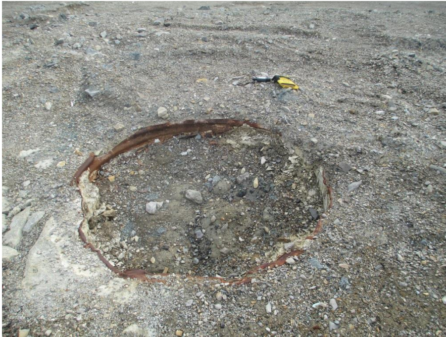
Photo 1, Subsidence Area, Vent/Backfill Raise (WP#1)
