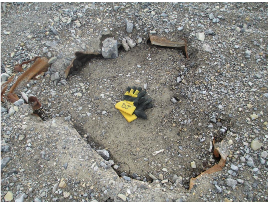
Photo 22, Subsidence Area, Vent/Backfill Raise (WP#20)
