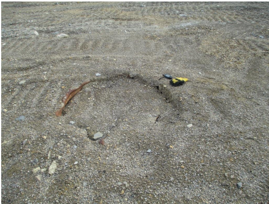
Photo 2, Subsidence Area, Vent/Backfill Raise (WP#2)
