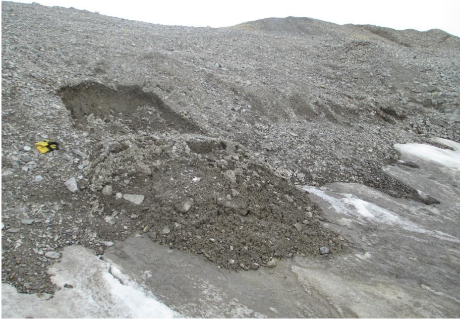
Photo 113, Main Portal, minor slumping of slope above portal (WP#82)
