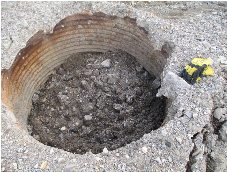
Photo 57, Subsidence Area, Vent/Backfill Raise with ~0.7 m internal settlement (WP#48)
