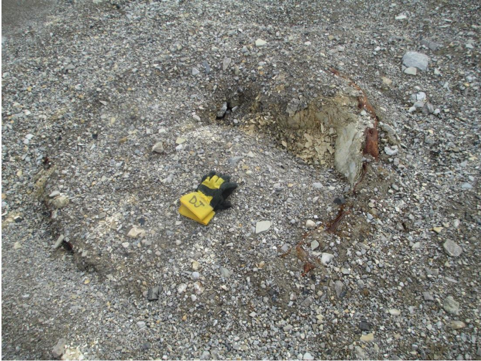
Photo 65, Subsidence Area, Vent/Backfill Raise (WP#55)
