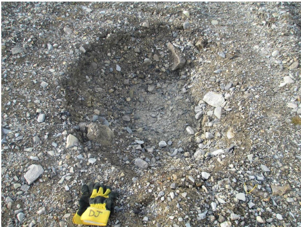
Photo 50, Subsidence Area, Vent/Backfill Raise (WP#43)
