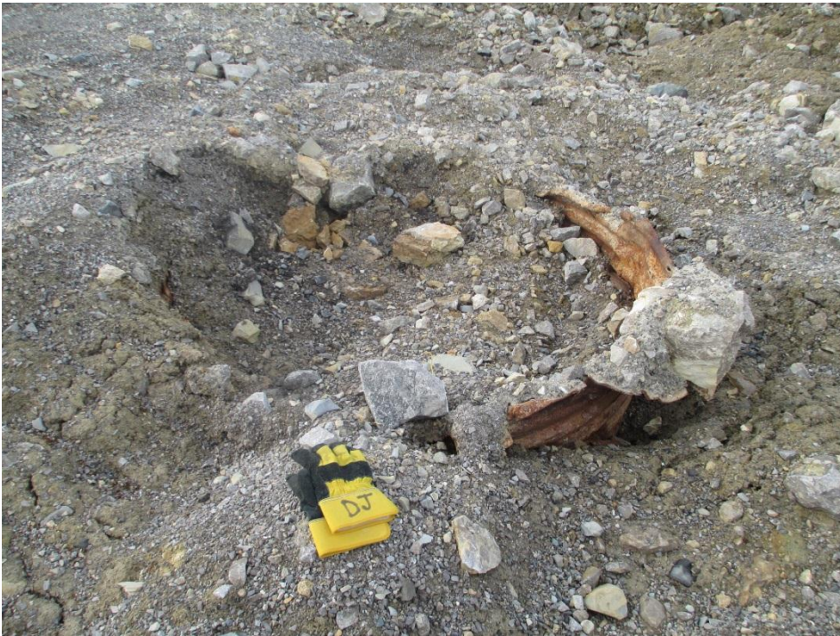
Photo 11, Subsidence Area, Vent/Backfill Raise with exposed CSP (WP#10)
