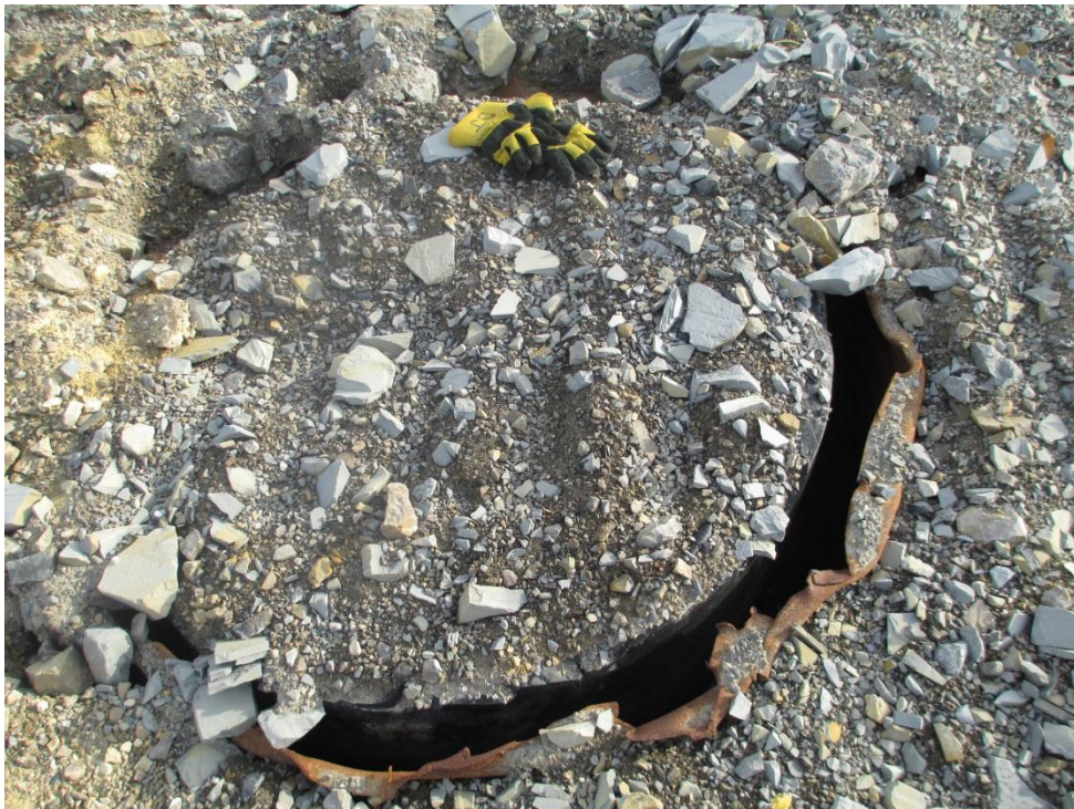
Photo 46, Subsidence Area, Vent/Backfill Raise with internal HPDE liner (WP#39)
