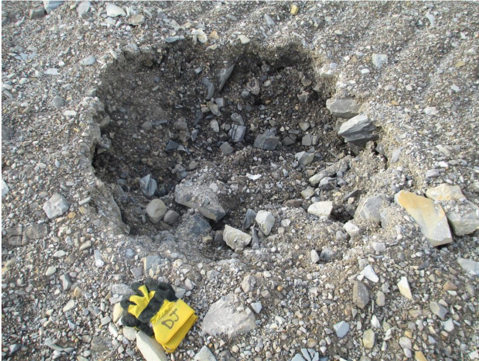
Photo 49, Subsidence Area, Vent/Backfill Raise (WP#42)
