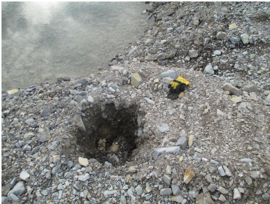
Photo 32, Subsidence Area, Vent/Backfill Raise with ~0.3 m internal settlement (WP#28)
