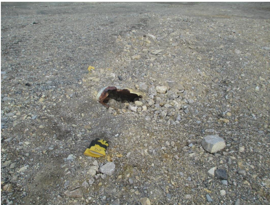
Photo 10, Subsidence Area, Vent/Backfill Raise (WP#9)
