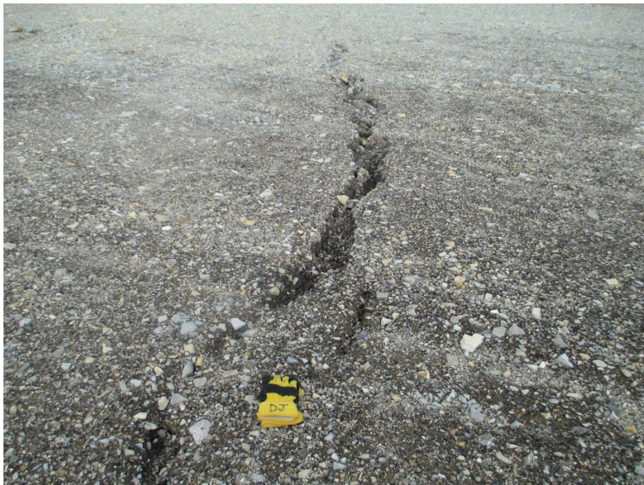
Photo 70, Subsidence Area, old tension crack (WP#59)
