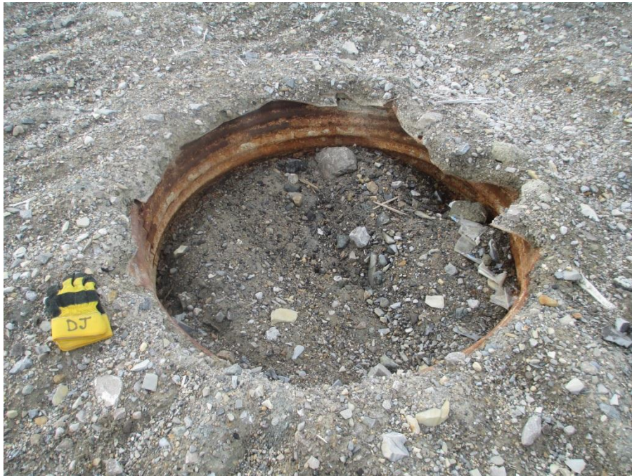
Photo 25 , Subsidence Area, Vent/Backfill Raise with 0.3 m internal settlement (WP#23)
