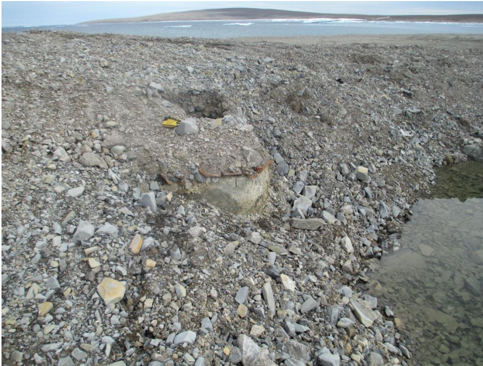
Photo 31, Subsidence Area, Vent/Backfill Raise beside ponded water (WP#28)
