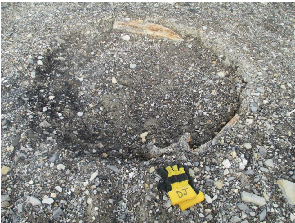
Photo 62, Subsidence Area, Vent/Backfill Raise (WP#52)
