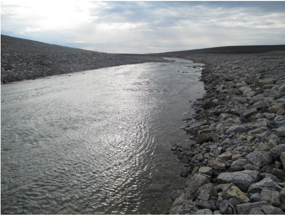
Photo 93, Garrow Lake Dam, dam breach channel (WP#72)
