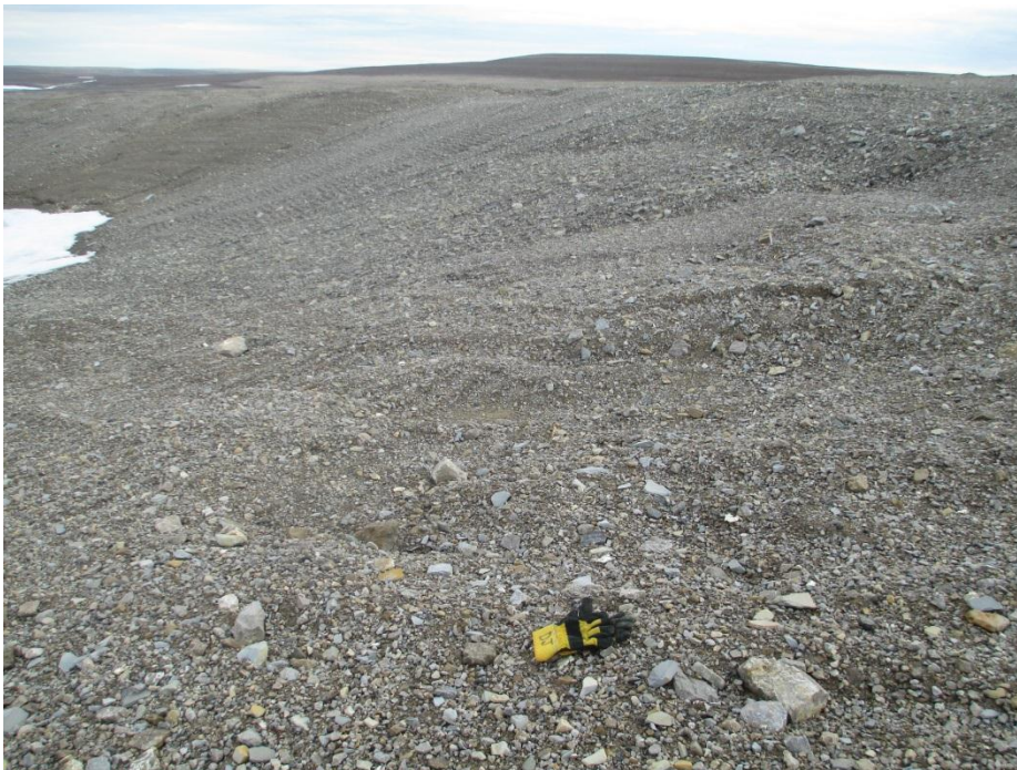
Photo 6, Subsidence Area, graded slope with some thaw settlement (WP#5)
