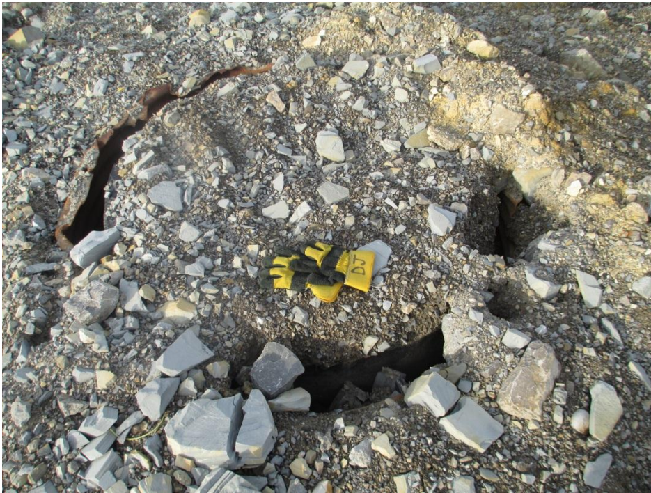
Photo 45, Subsidence Area, Vent/Backfill Raise with internal HPDE liner (WP#39)
