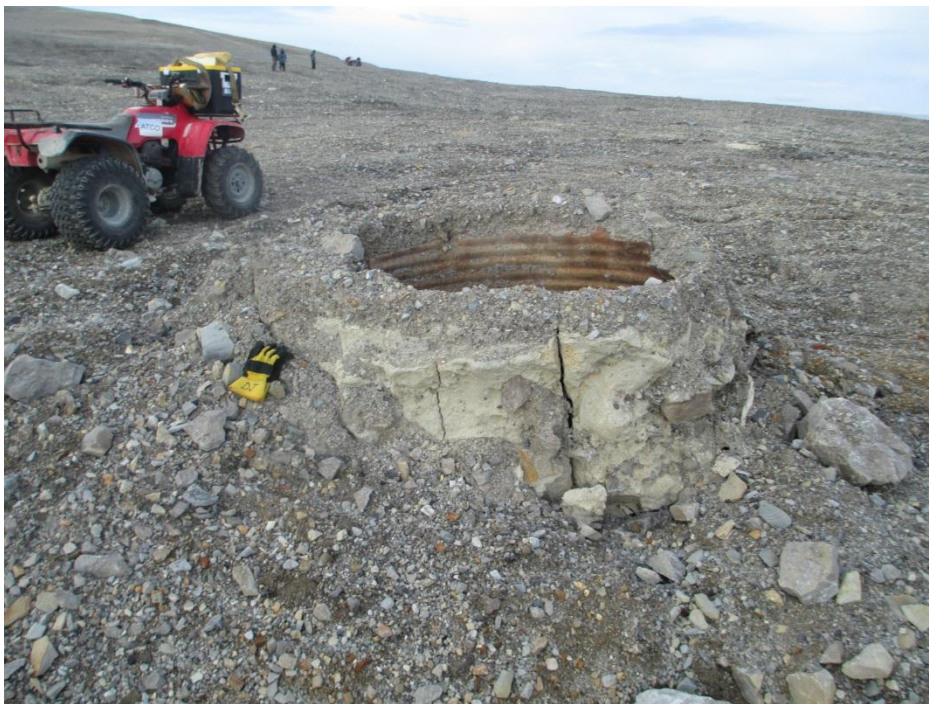
Photo 56, Subsidence Area, Vent/Backfill Raise (WP#48)
