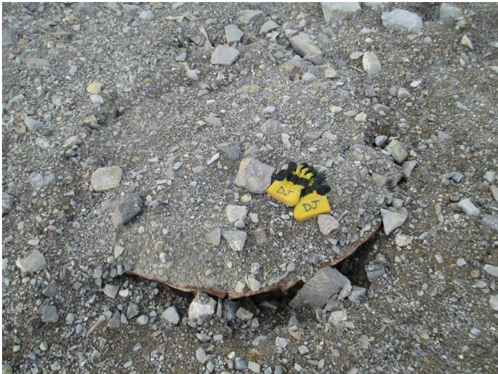
Photo 54, Subsidence Area, Vent/Backfill Raise (WP#47)
