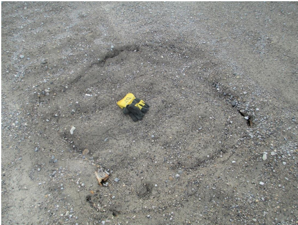
Photo 20, Subsidence Area, Vent/Backfill Raise (WP#18)
