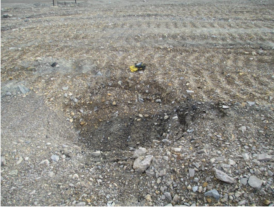
Photo 3, Subsidence Area, Vent/Backfill Raise (WP#3)
