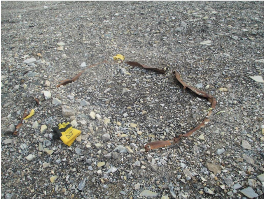
Photo 13, Subsidence Area, Vent/Backfill Raise (WP#12)
