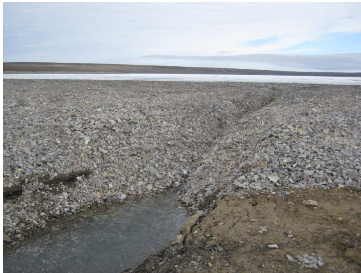
Photo 6, Garrow Lake Wave Break, Thaw Settlement at East End
