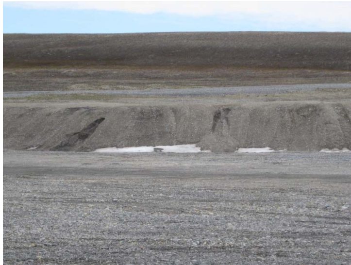
Photo 33, New Quarry, Minor Erosion and Slumping on East Slope
