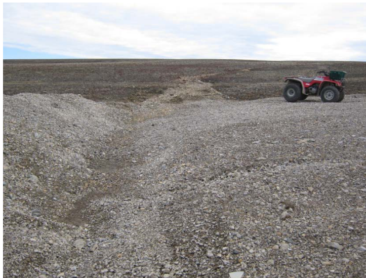
Photo 22, Frustration Lake, Typical Road Drainage Crossing
