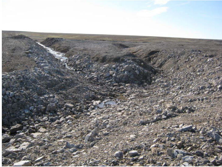
Photo 81, Drainage Ditches, Rip-Rap Lined Slope Below Drainage Ditch
