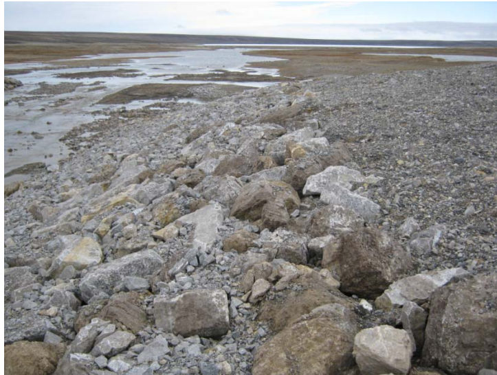
Photo 11, Garrow Lake Dam, Channel Rip-Rap on East Breach Slope
