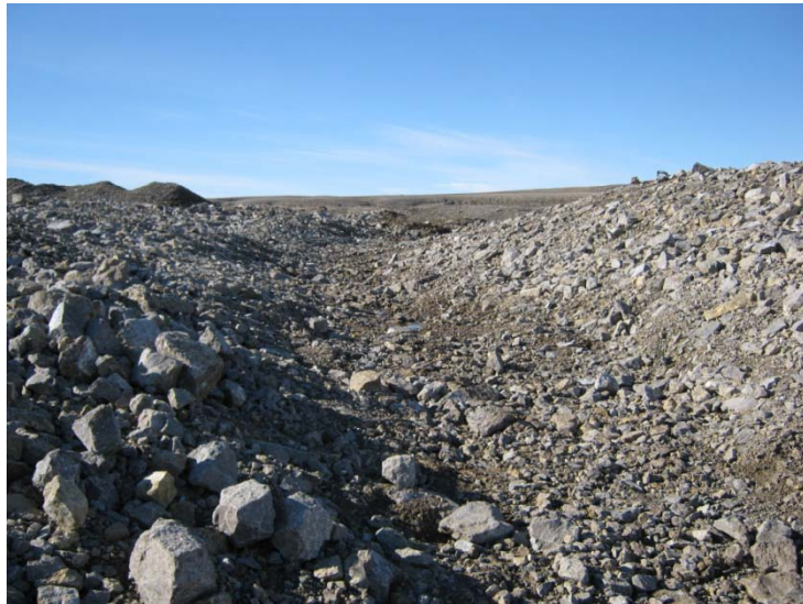
Photo 80, Drainage Ditches, Rip-Rap Lined Ditch Across Road Near Camp
