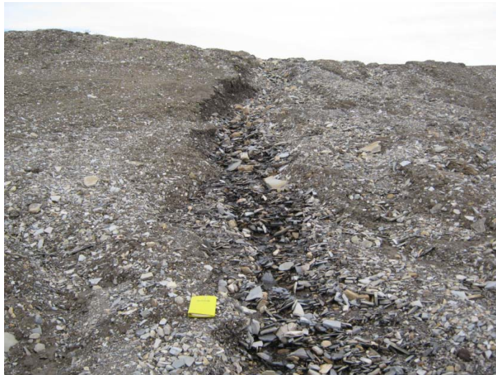
Photo 32, New Quarry, Minor Erosion Gully on North Slope
