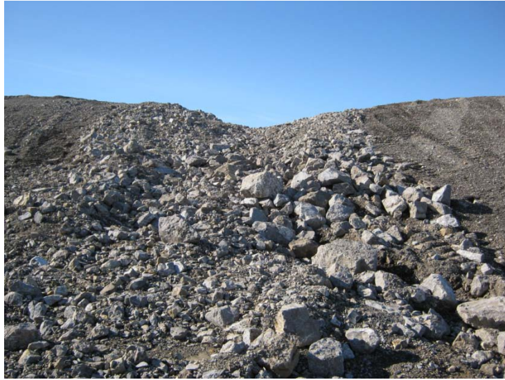
Photo 79, Drainage Ditches, Rip-Rap Lined Slope Below Drainage Ditch
