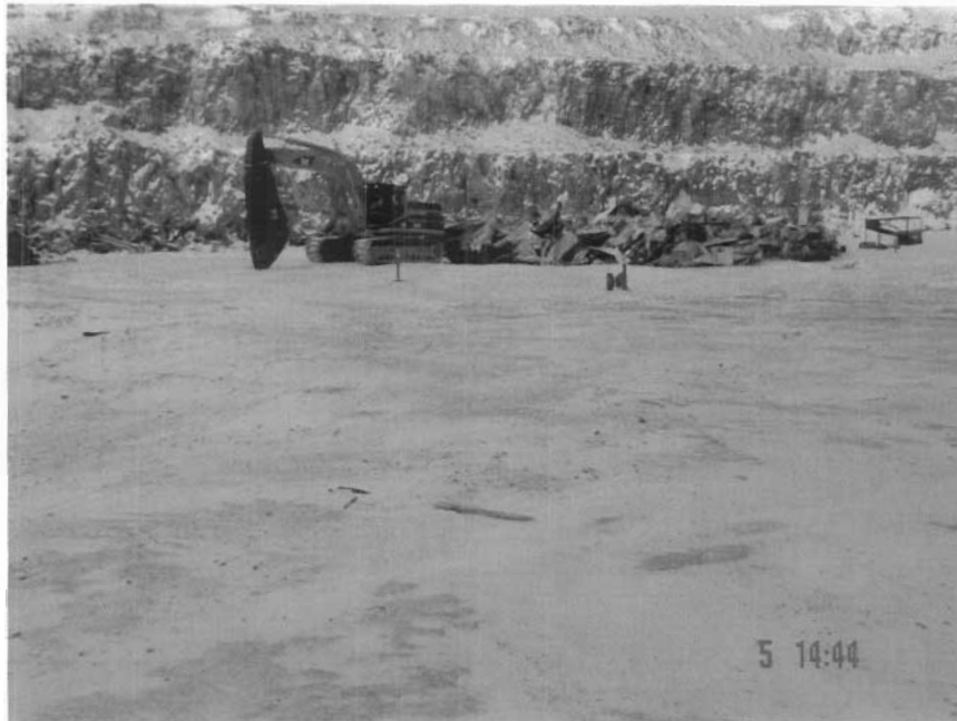
Photo # 11. Mechanical shear on back-hole in Red Dog Pit for consolidation of demolition debris.
