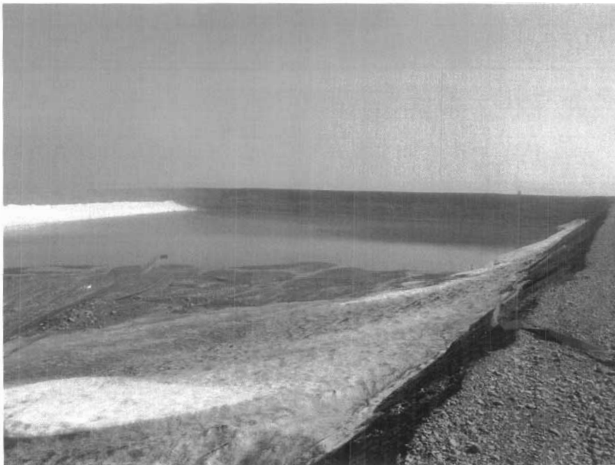
Photo # 18. Sludge Thickening Facility emergency dump pit. All berms in good condition with no leaks.
