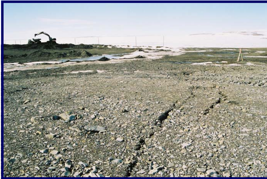
Subsidence area, looking north. Note cracks in backfill material.
