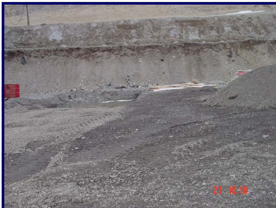
Backslope of product storage area. Some metals contaminated soils remain to be removed from this area.
