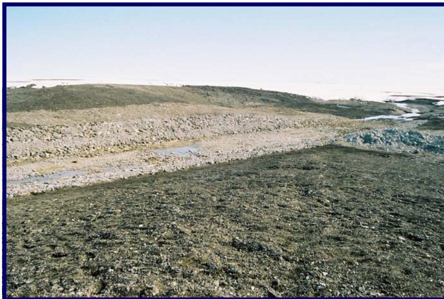
Garrow Lake Dam, riprap lined channel.
