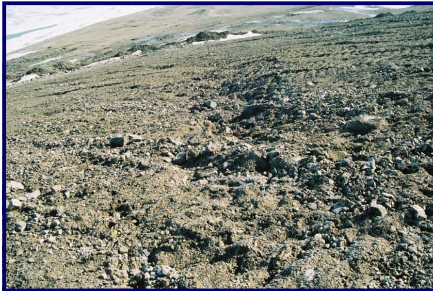
Operational Landfill - minor gully erosions/ subsidence in cover material on seaward facing slope.
