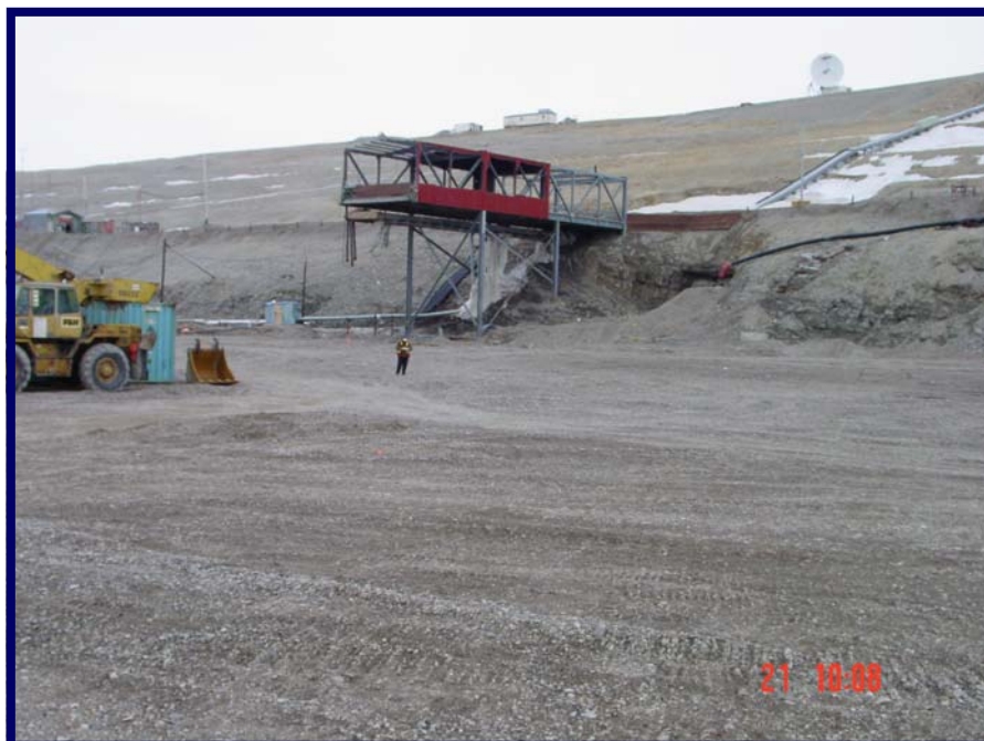
Beach gravel backfill over mill/barge and product storage shed area.
