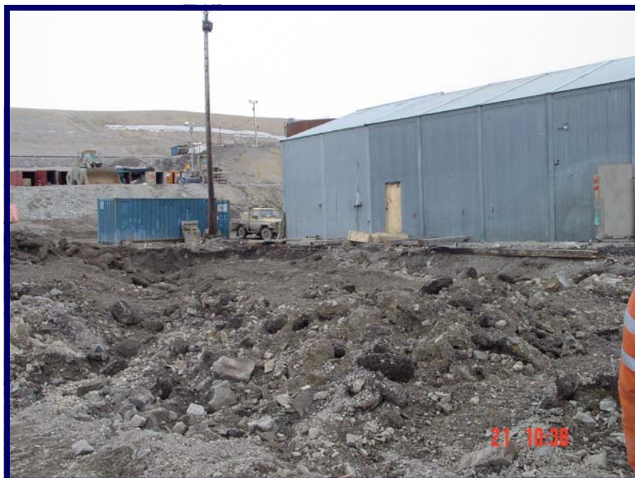
Excavation of hydrocarbon contaminated soils from footprint of north foldaway buildings.
