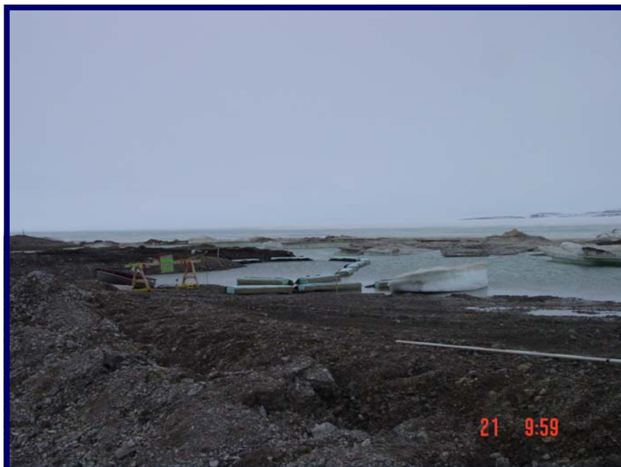
Sorbent boom in dock cell area to contain minor hydrocarbon contamination.
