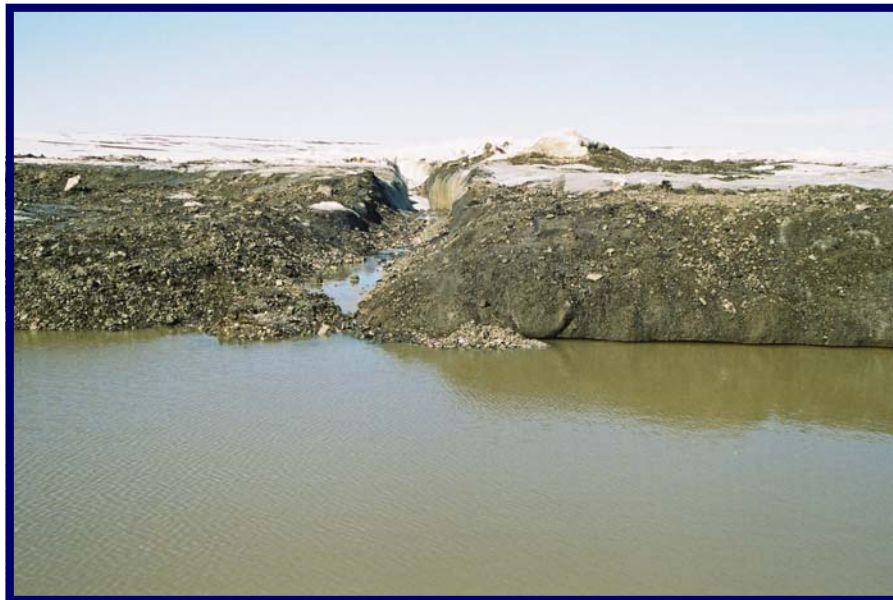
Channel cut into ice of Garrow Lake upstream of dam to channel flow towards breach.
