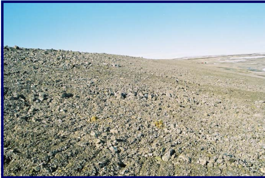
Operational Landfill, seaward sloping aspect of cover. Note finer grained nature compared with cover at the top of the slope.
