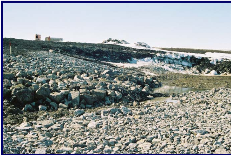
View of upstream face of dam with drifted snow and spoil. This area needs to be re-graded after the snow melts.
