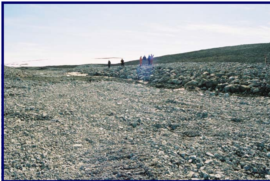
View looking downstream along riprap lined channel through Garrow Lake Dam.
