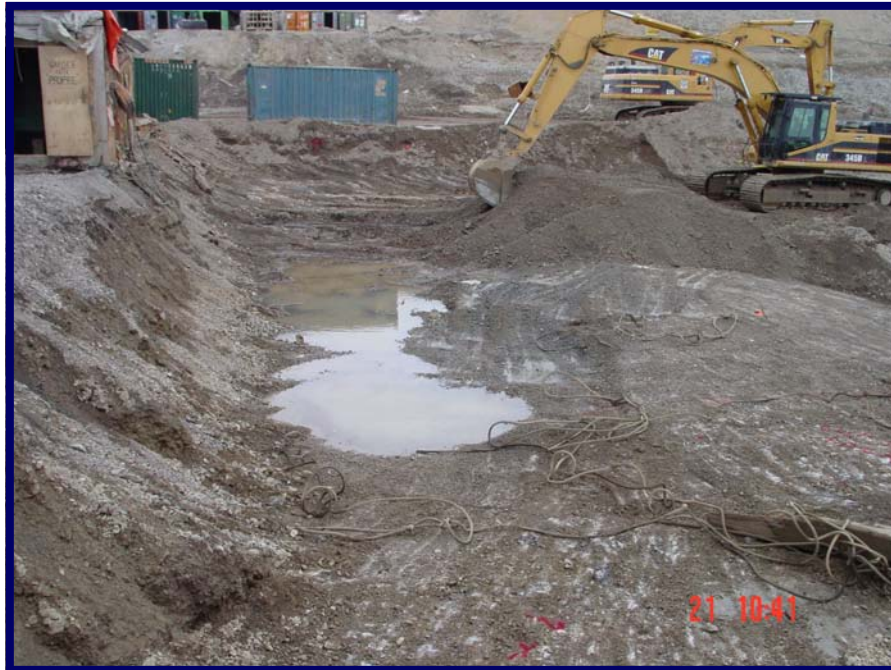
Excavation of contaminated soils down to frozen soils in footprint of south foldaway building.
