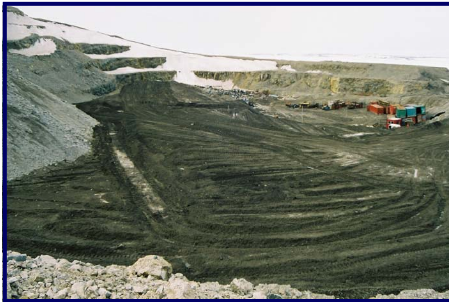
LRD quarry with cover of metals contaminated soils. Stockpiles of final cover consisting of blasted limestone visible on left.
