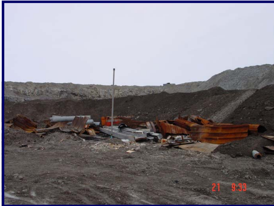
LRD quarry, large materials that remain to be cut up. Casing pipe is for installation of thermistor after quarry is closed.
