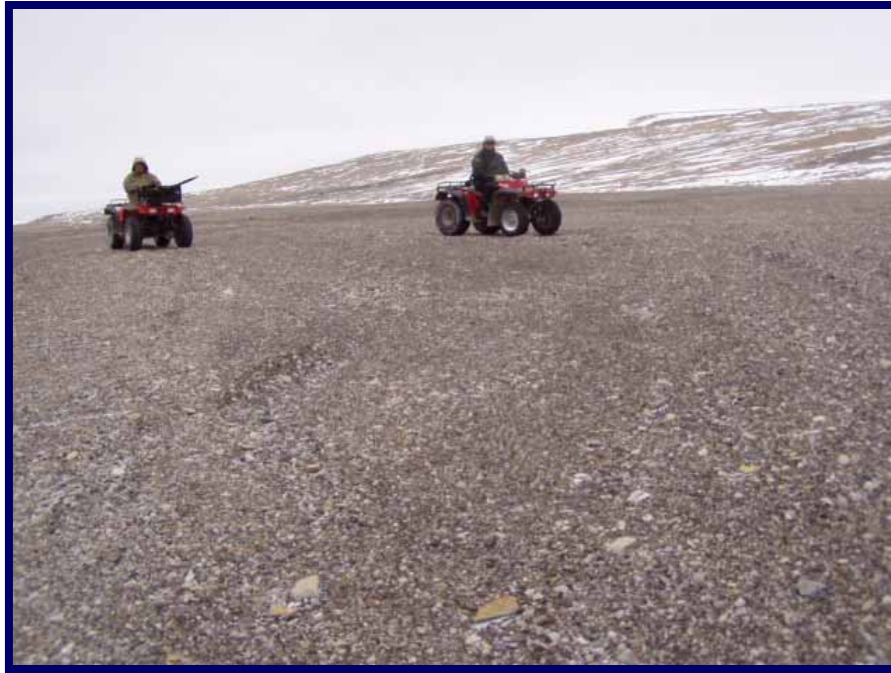
Photo 74: General view of horizontal portion of cover, near east end of landfill. This portion of the cover was supplemented by a layer of finer grained rockfill (gravel size) to fill in voids in coarse rockfill originally placed in this area during construction.
