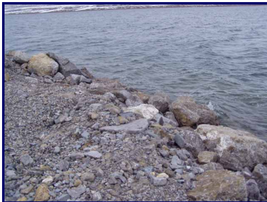
Photo 53: End of causeway, larger riprap still intact.
