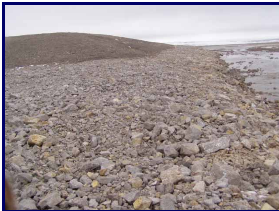
Photo 35: Looking upstream along right bank towards breached section of dam. Note riprap lined channel and flat slopes of breached cut in dam, seen in section in this photo.
