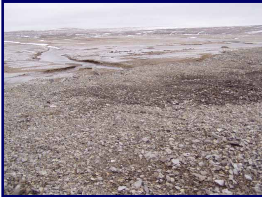
Photo 45: Seepage through the foundation along downstream side of gravel bar at east end. Note old scour channel from previous breach in this area.
