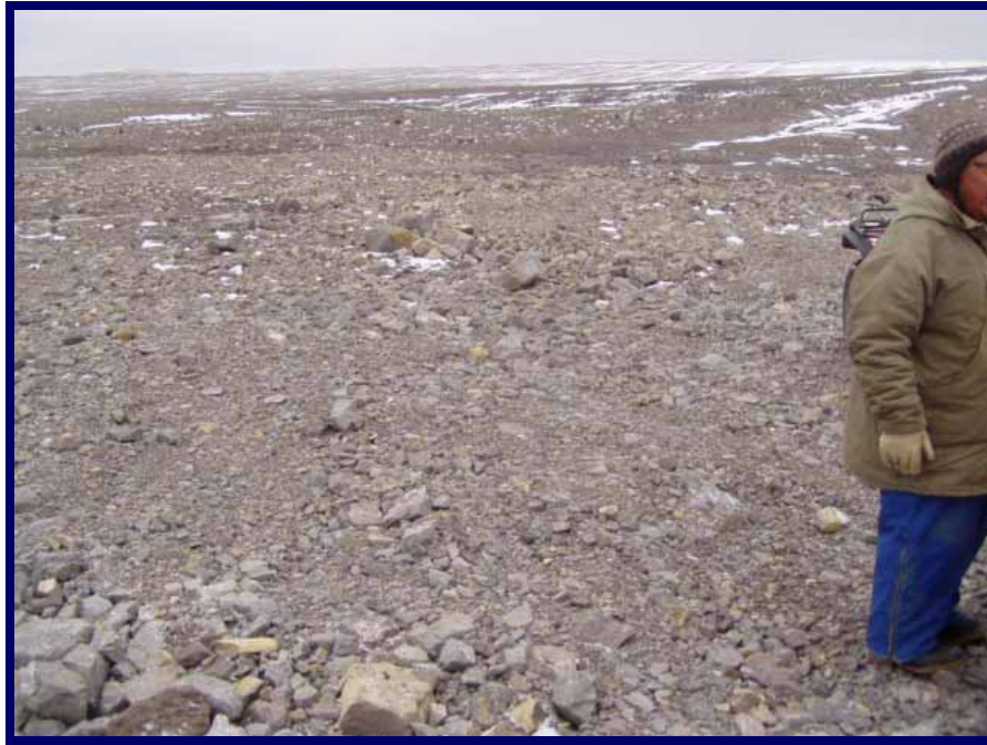
Photo 40: Erosion protection extending across top of right bank of Garrow Creek, downstream of dam.
