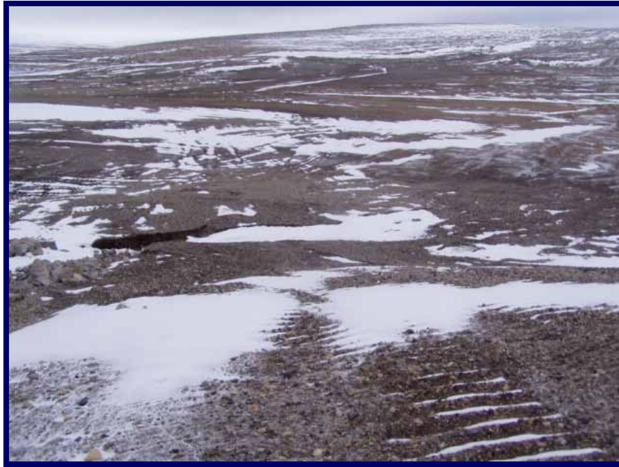
Photo 56: General view looking east, from crest of reclaimed slope on west side. A fan of eroded material can be seen at the toe of the slope on left side of photo. This material was eroded in 2006 along an ephemeral stream channel due to concentrated flow along the slope during spring melt. The channel was subsequently armoured with riprap in 2006 and is now stable.
