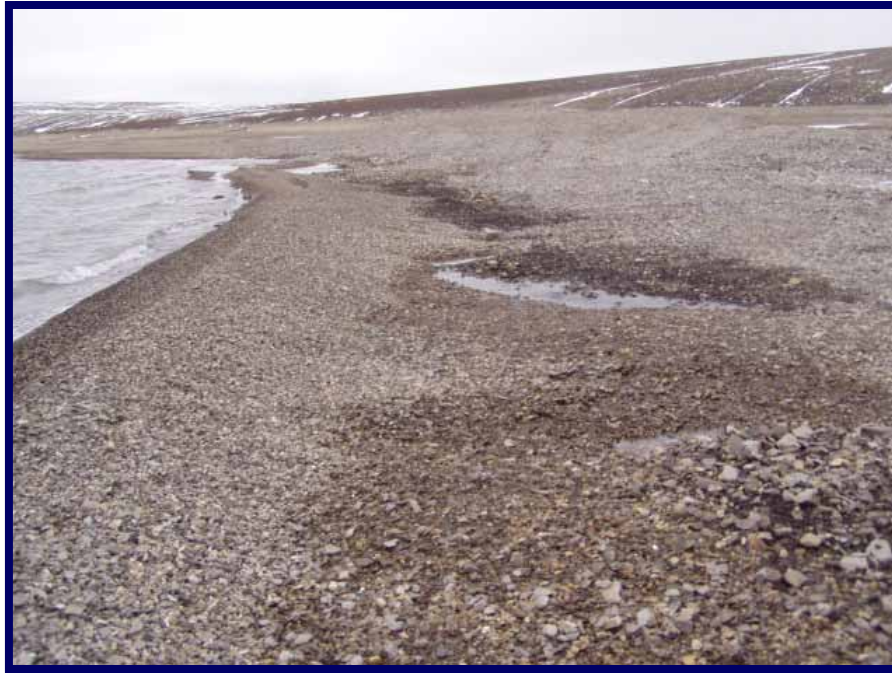
Photo 43: Looking east along downstream side of natural gravel bar across south end of Garrow Lake. Material to right is foundation footprint of former wave break structure. Note seepage exiting along toe of berm. Berm is at maximum height at this point, about 1.2 m (see
