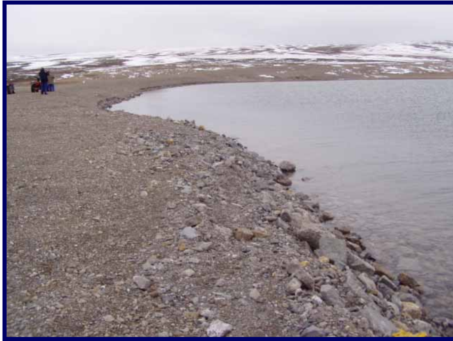
Photo 54: Leeward (south) side of causeway. Generally causeway looks in sound shape, with no real degradation or erosion.
