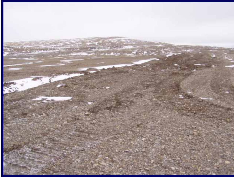
Photos 62: General view of reclaimed landscape looking north to northwest along decommissioned haul road along west side of New Quarry. Interceptor ditch leading to riprap lined channels shown in previous photos is visible along left side of road, infilled with drifting snow.
