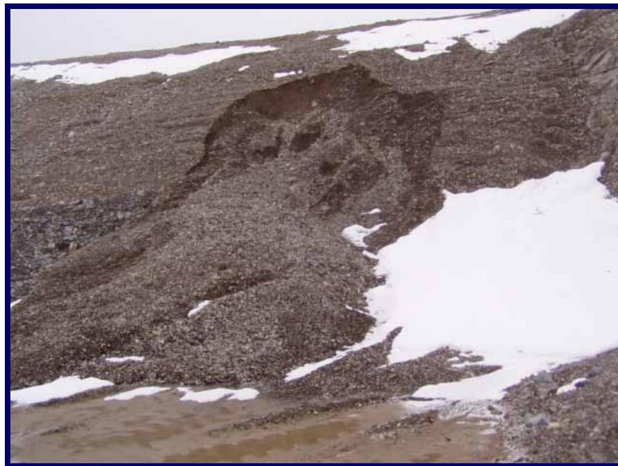
Photo 93: Close-up view of slump in Main Portal backfill. It appears this was due to backfill being placed too steeply and becoming saturated with snowmelt from a snowdrift.
