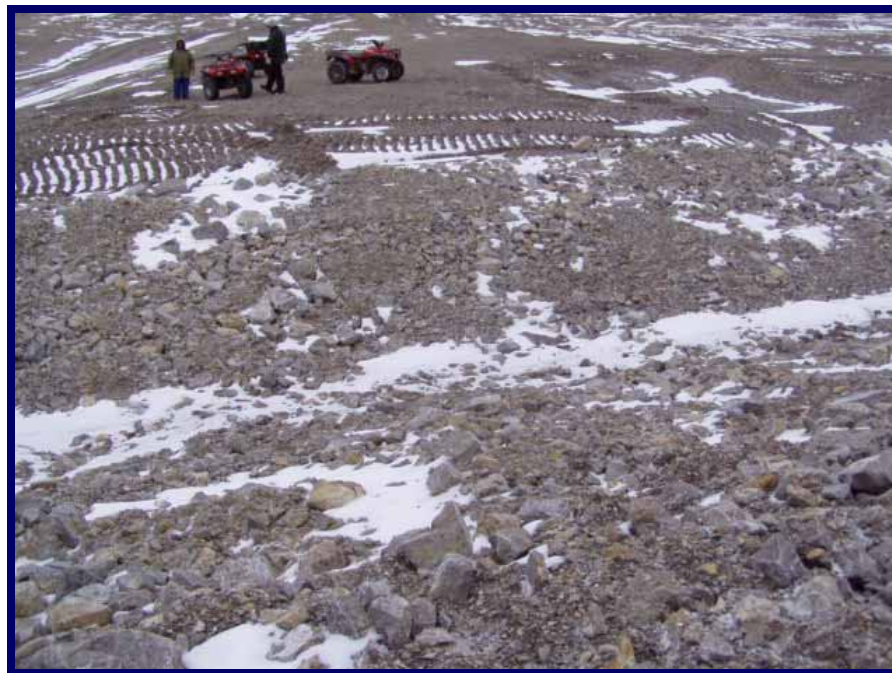
Photo 61: View of same channel as in previous photo showing riprap lining where channel cuts across decommissioned haul road. Looking south along west side of New Quarry.
