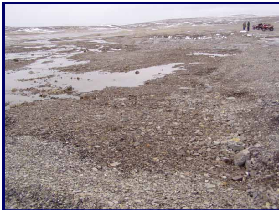
Photo Photo 42: Looking downstream from location of previous photo. Garrow Lake Dam is in distant background. Water is entirely from seepage through the natural berm or under seepage through the pervious former lakebed gravels. Surface disturbance of gravels is due to previous episode of flow when natural berm was breached by overtopping. Berm has since re-healed itself.
