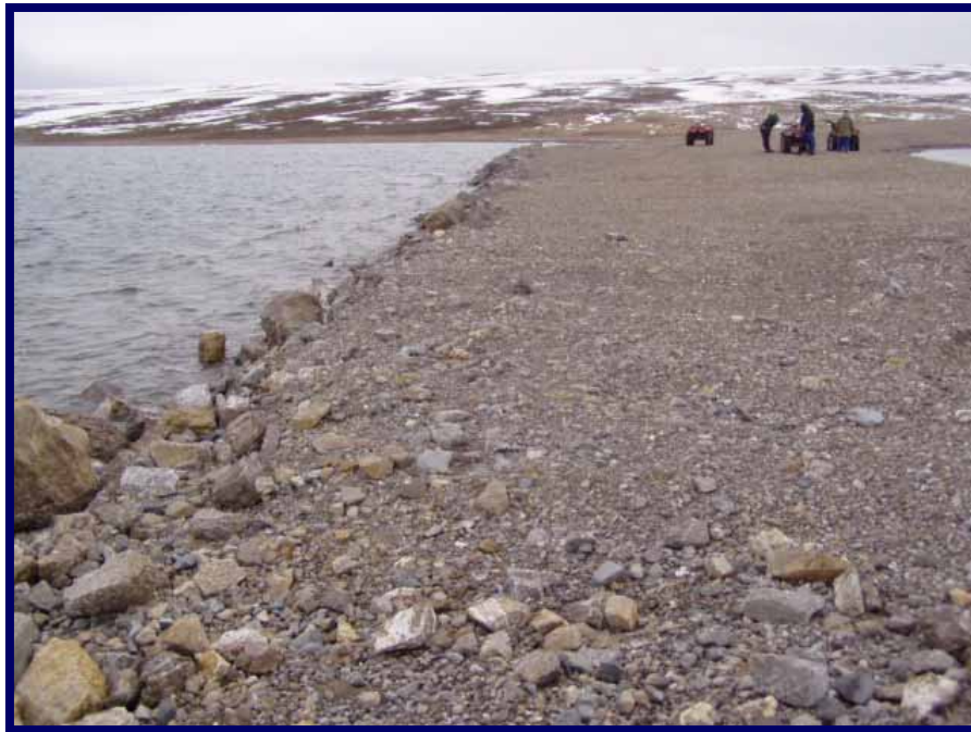
Photo 51: Wave washed windward (north) side of causeway.
