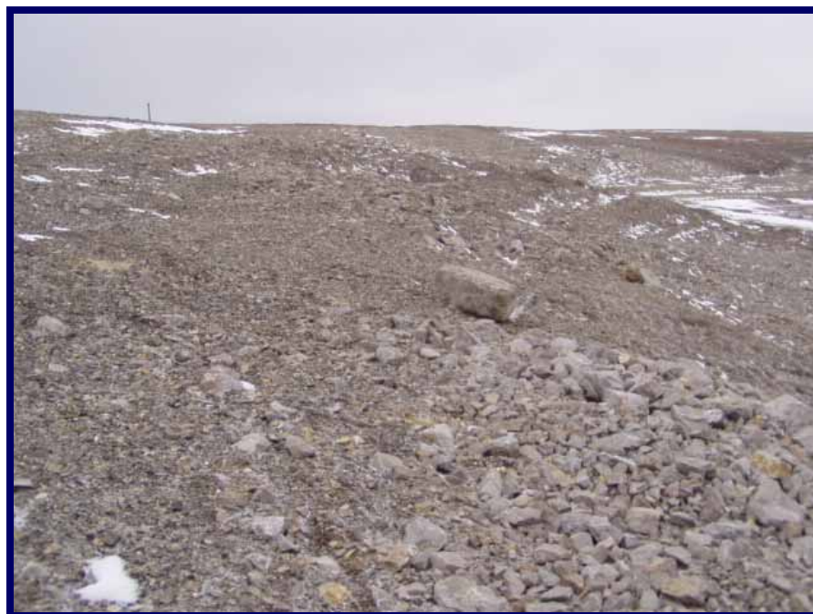
Photo 37: Upstream slope of dam on right side of Garrow Creek. Slope surface is irregular as this material was originally placed on top of snow and ice, which has since melted out and drained away.
