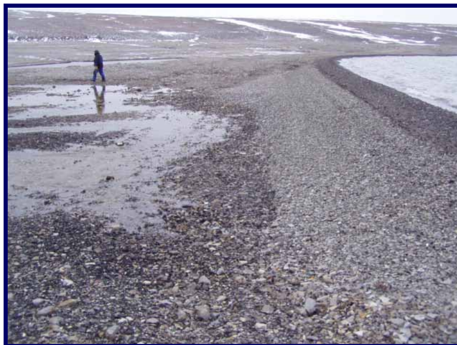
Photo 50: Seepage along downstream toe at point of maximum height.
