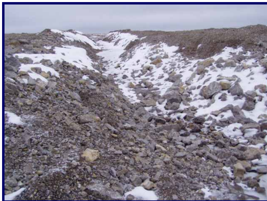
Photo 59: Same stream channel as in previous photos. This portion of channel is parallel with the crest of the slope and intercepts runoff from further upslope sources.
