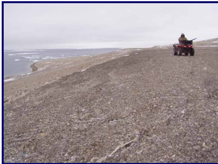
Photo 73: Looking west along south-facing slope portion of cover. No signs of any erosion, settlement or heaving.
