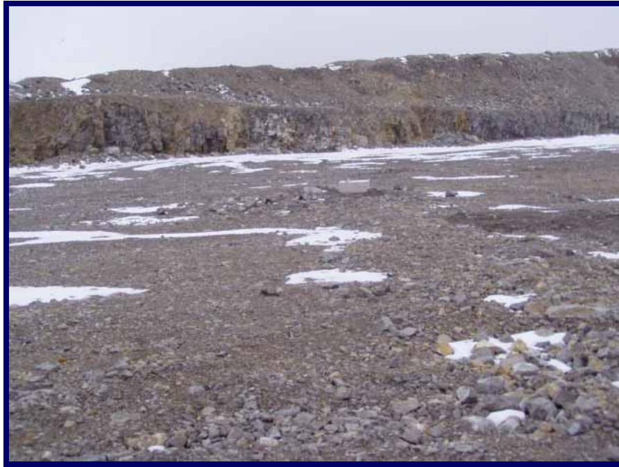
Photo 99: Looking northeast across landfill cover. In general cover looks stable with no signs of erosion, settlement or heaving.
