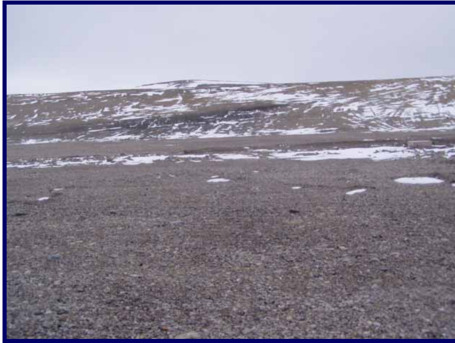
Photo 71: Looking north across horizontal portion of landfill cover. Note thermistor box on right side of photo. Cover shows no signs of erosion, settlement or heave.
