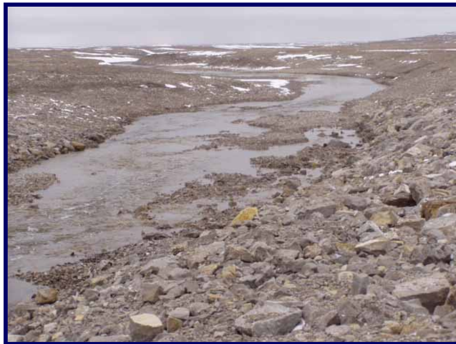
Photo 34: Garrow Creek downstream of dam, looking downstream. Note riprap on channel sides extends across top of bank on right, as shown in next photo.
