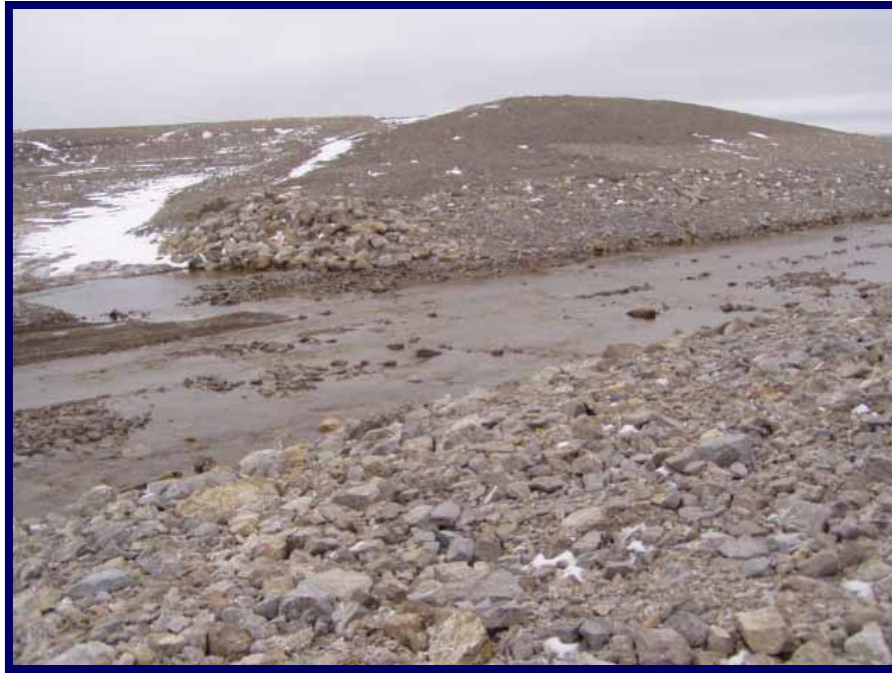
Photo 38: View across breached dam to left bank side, along upstream slope of dam.
