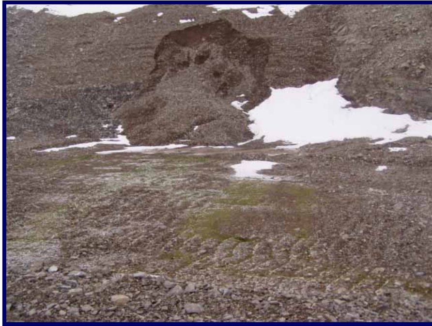
Photo 96: General view of Main Portal showing classic tongue-shaped flow slide and green zone of vegetation associated with seepage from the backfill.
