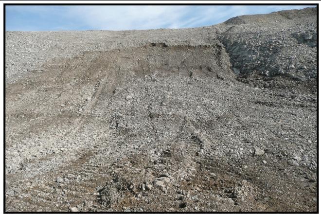
548)- Main portal backfill with lower buttress of rockfill along toe and re-grading to flatten over slope. Excavator left minor over steepened slope sections, which are expected to fail in the short term, but not expected to be detrimental to long term physical stability of backfill. Note steep rock slope along south side of fill.
