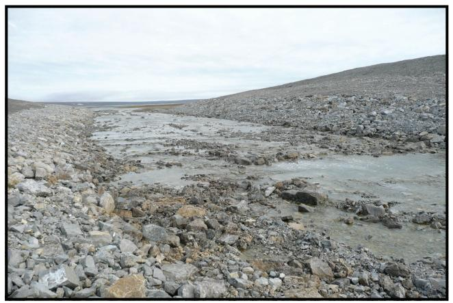
(528)- View looking upstream along Garrow Creek through breached section in dam. Creek is flowing across full width of channel, with average depth of about 150 mm.
