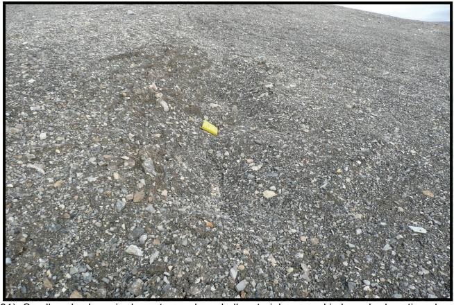
(531)- Small scale slump in downstream dam shell material exposed in breached section along west side of creek.
