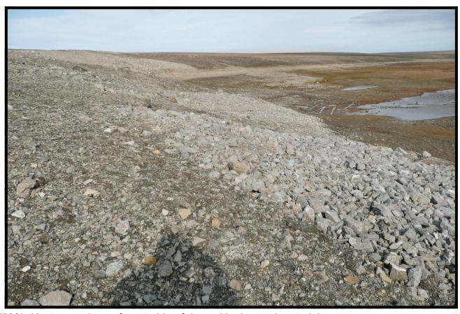
(533)- Upstream slope of west side of dam with slumped material.
