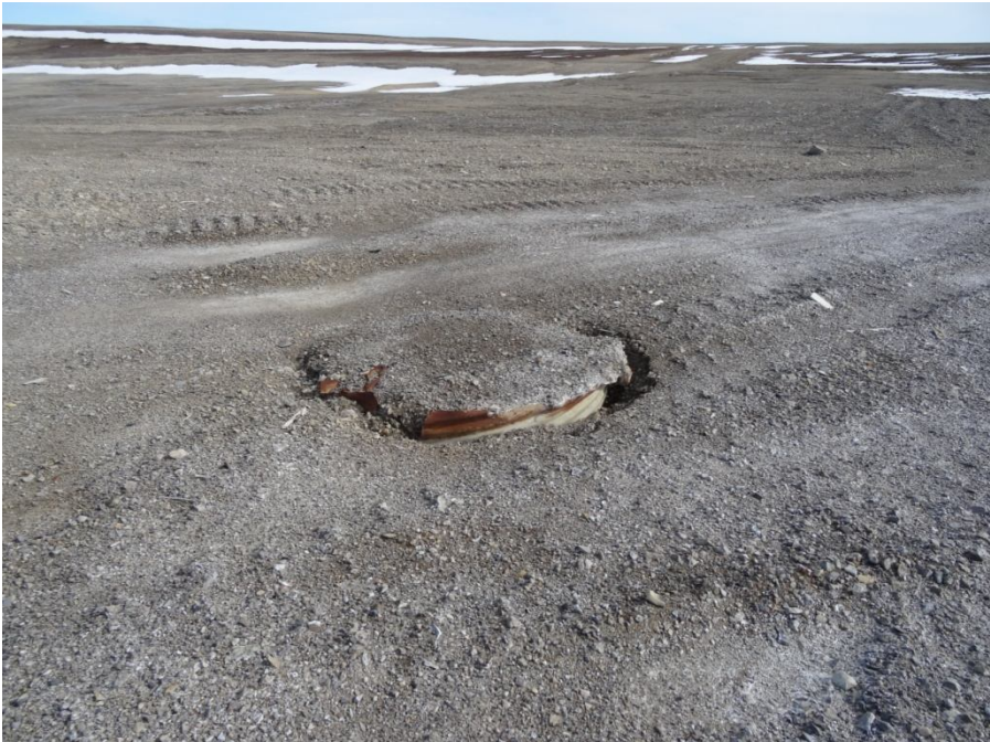
Figure 8 Vent raise - settling and subsidence
