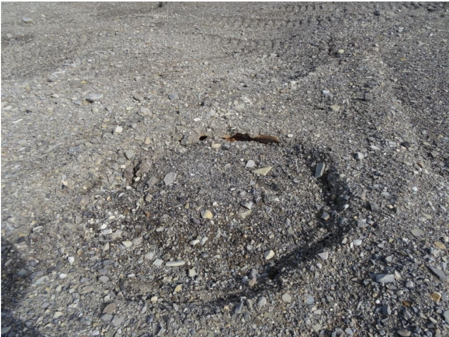
Figure 5 Vent raise .. Settling around and within the Culvert
