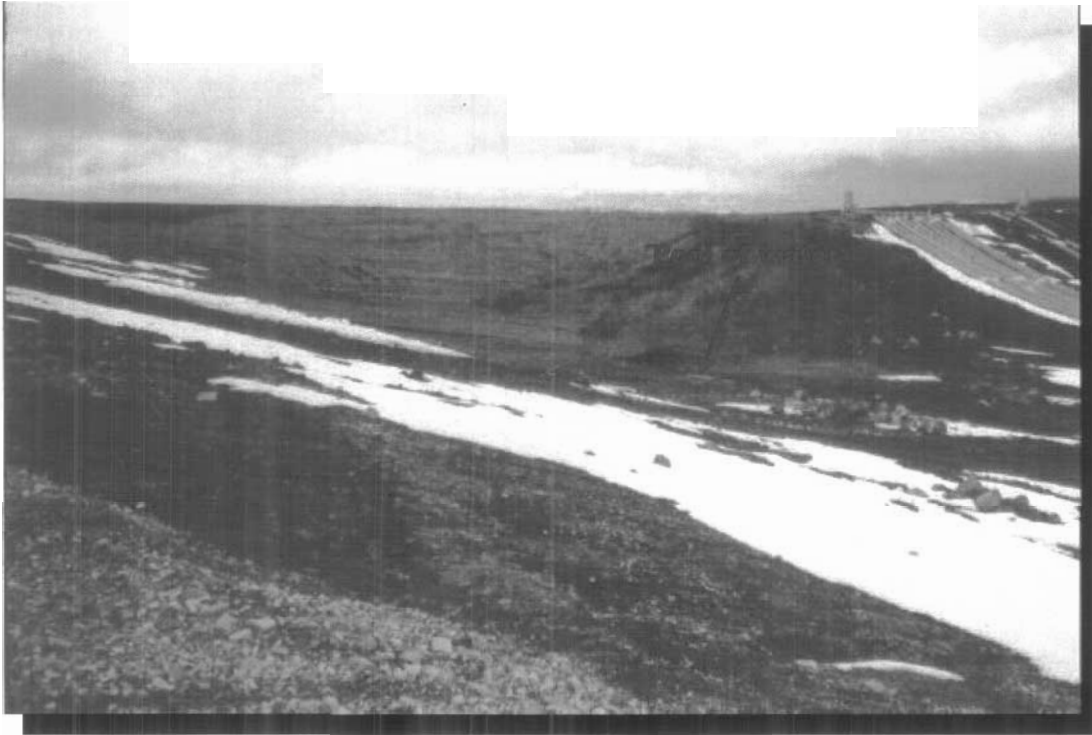
Photo 3 Downstream slope - looking east. Very little ponded water at toe of dam.
