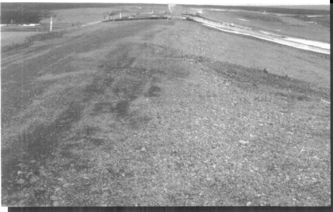
Photo 4 Dam crest - looking east.
