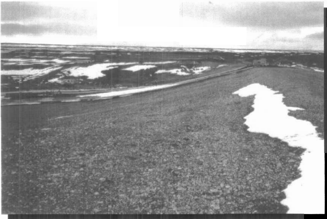
Photo 2 Downstream slope - looking west.
