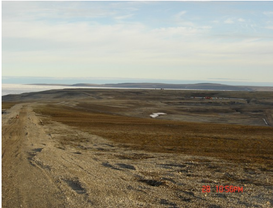
View of segment of road to Frustration Lake looking southwest towards mine site from the highest point of topography. Roadway and sideslope are in good condition, free of significant erosion features.
