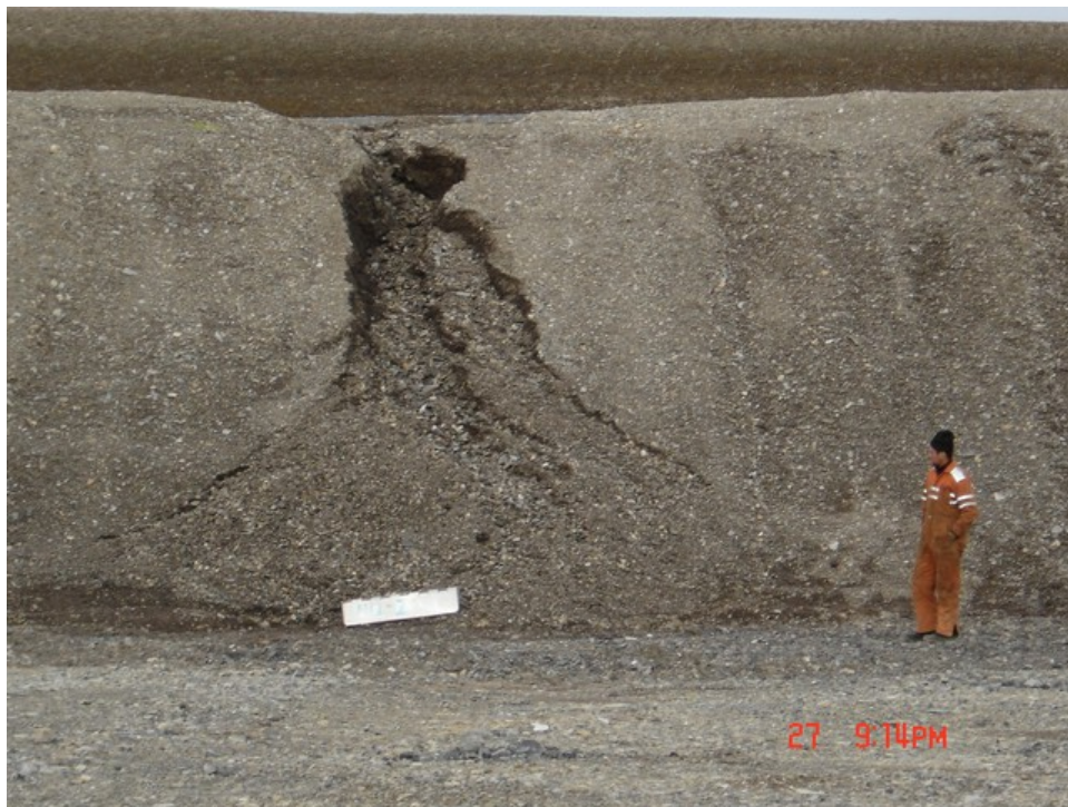
Close-up view of erosion gully at waypoint NQ2 PH1, showing relatively small width, and apparent tendency to be self-armouring.
