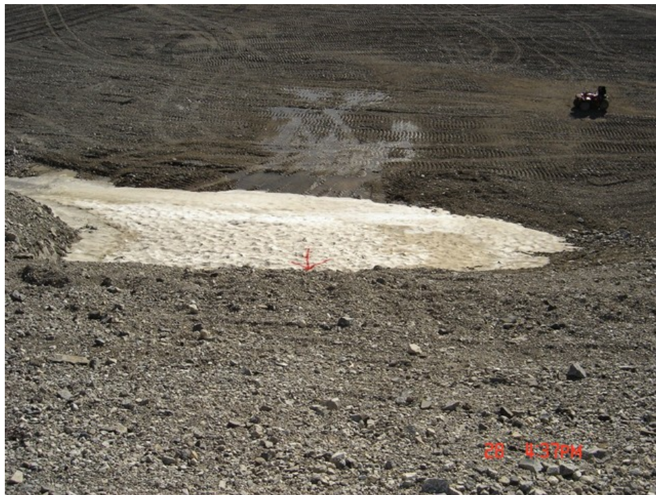
Slope above Main Portal area is inclined at about 26 degrees, locally steepening to 35 degrees. Minor slumping was observed, but not considered to present hazard to humans or wildlife.
