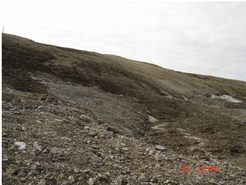
North Portal looking west across backfill. This portal accessed a decline and was frozen prior to being backfilled. Thus, the minor drainage along the toe of the cap is considered to be of a surficial nature only.
