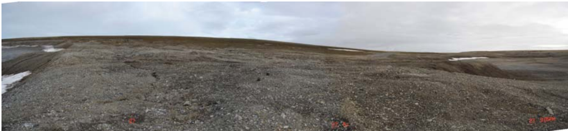
View looking up west sideslope of New Quarry Extension, where stripped organic surficial soil has been spread. Occasional cracks but no signs of mass movement presenting any hazard to humans or wildlife.
