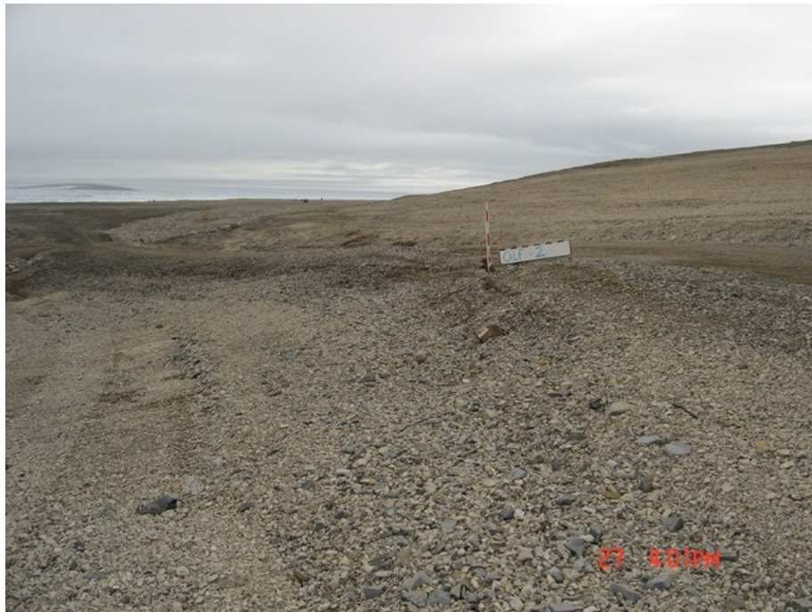
Minor almost imperceptible crack at edge of approach road to northeast end of the operational landfill, viewed from waypoint OLFPH 2. This is not associated with any other signs of settlement of instability in the slope above or below, and poses no hazard to human health or wildlife.
