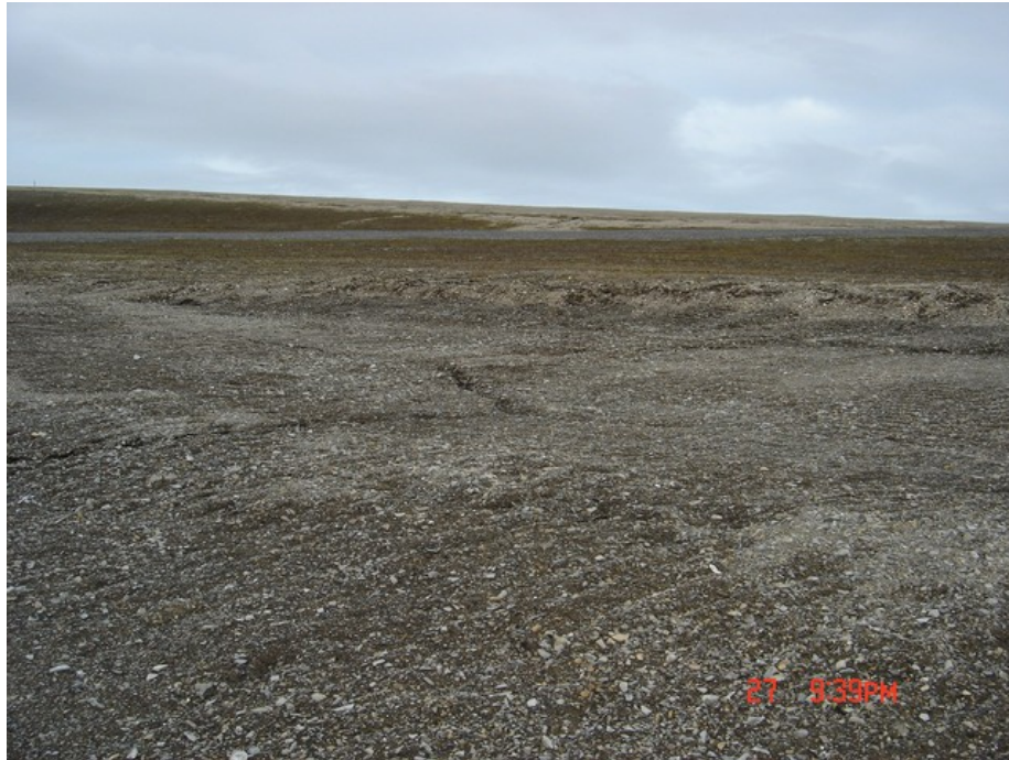
Area above waypoint NQ5 view looking northeast across area of disturbed surficial soil bordering edge of quarry sideslope. Illustrates typical pattern of surficial deformation caused by seasonal thaw of disturbed surficial soils. This poses no threat to humans or wildlife.
