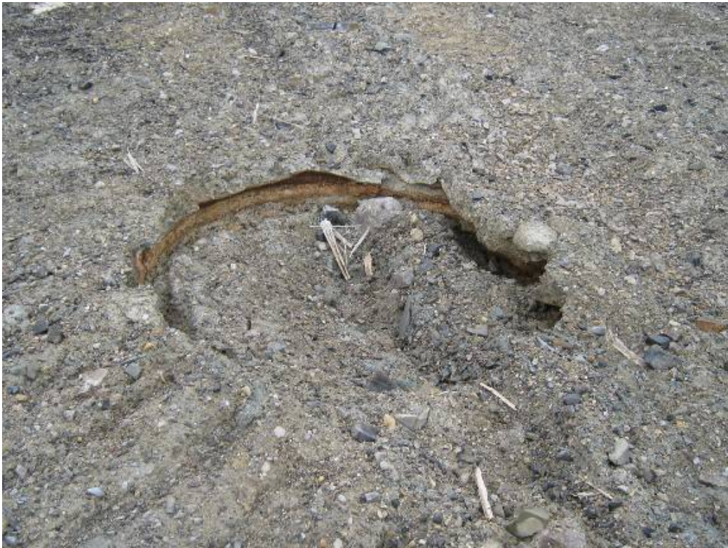
Photo 44- Northing 558151 Easting 8369131 Elevation 12 m Subsidence Area: metal vent (about 1 m diameter)
