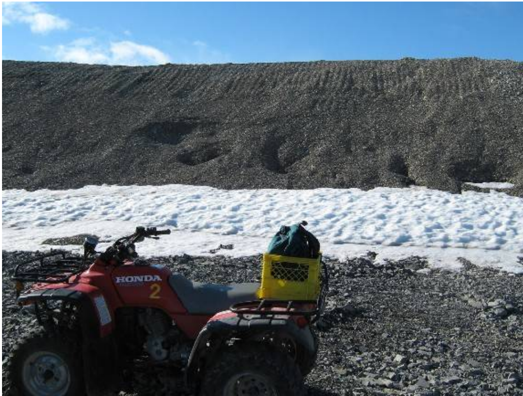
Photo 113- Northing 559027 Easting 8369443 Elevation 20 m New quarry area: sink holes on slope potentially caused by snow/ice melt.
