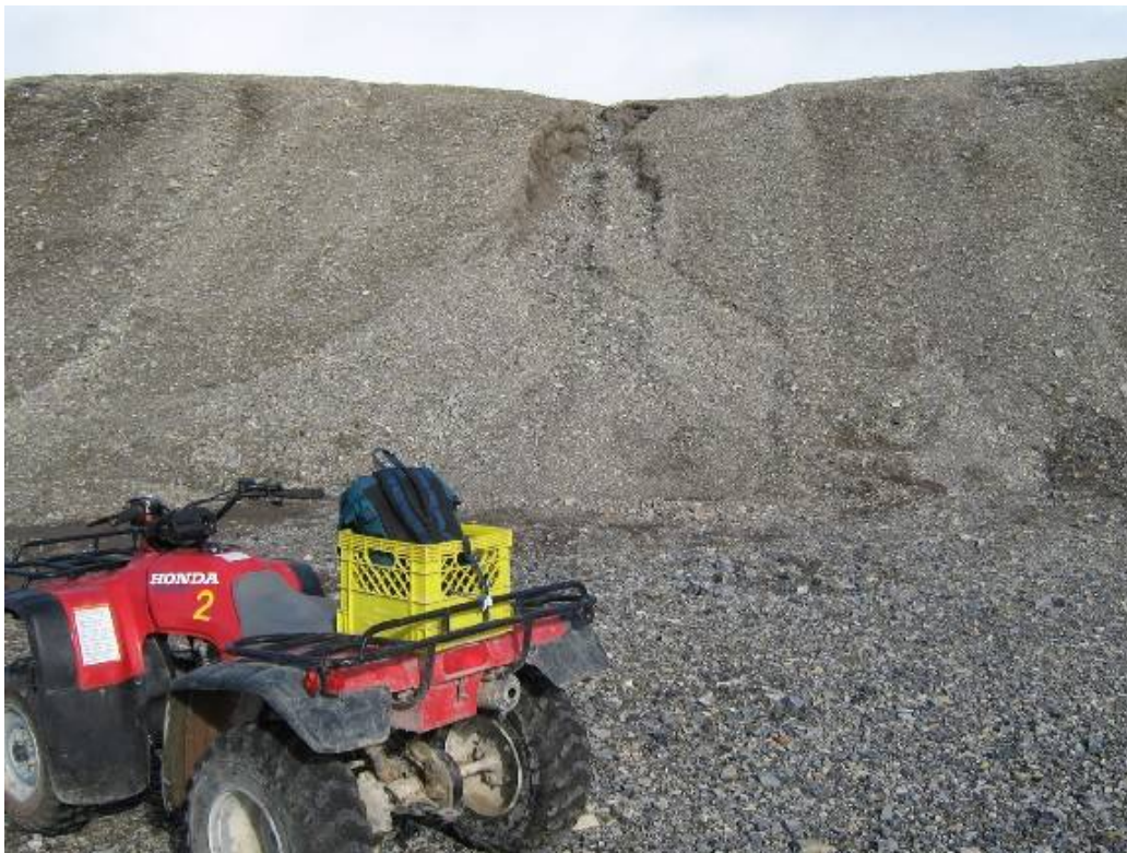
Photo 111- Northing 559086 Easting 8369039 Elevation 17 m New quarry area: erosion gully down quarry perimeter slope
