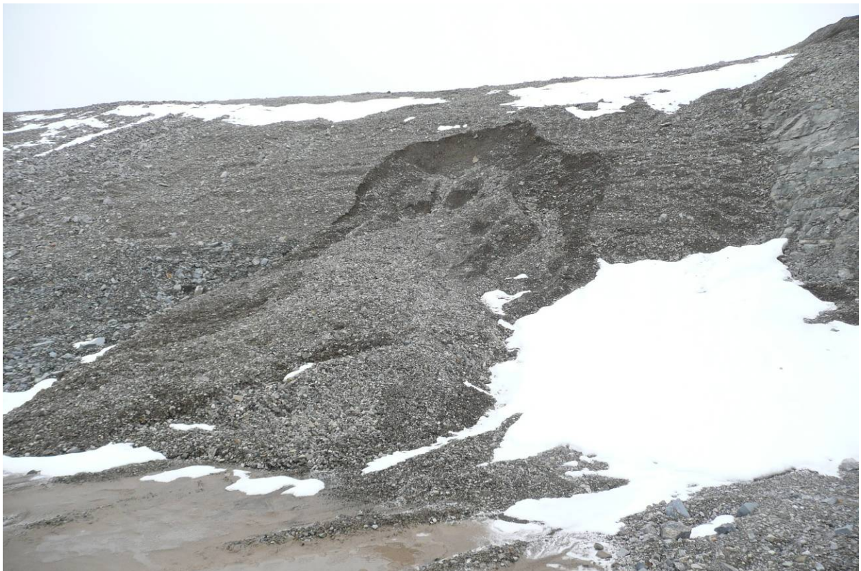
Main Portal Slope Failure (Close-up) – August 24, 2008
