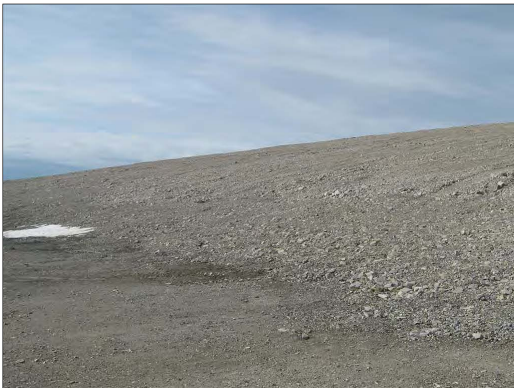
Photograph 16. Operational Landfill, East slope, view from toe ↑
