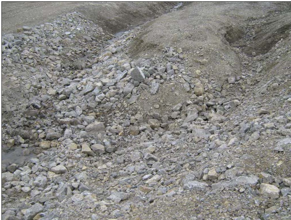
Photograph 51. Stabilized Road Drainage Ditch, South of New Quarry, above ditch ↑
