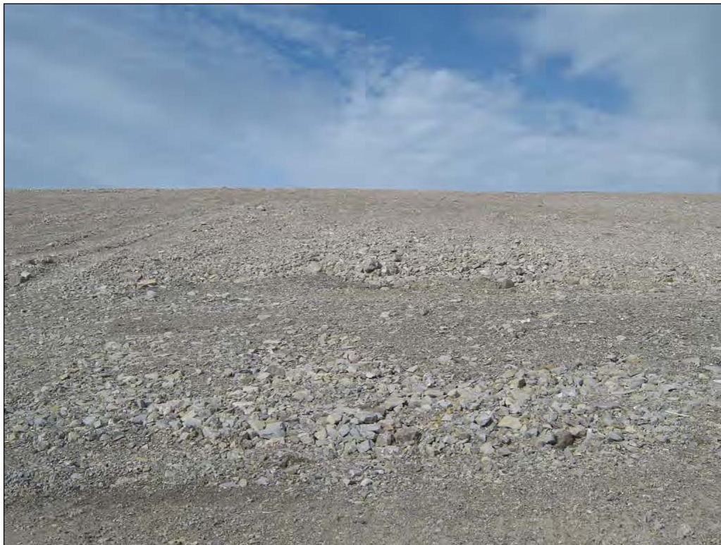
Photograph 17. Operational Landfill, East slope, view from toe ↑
