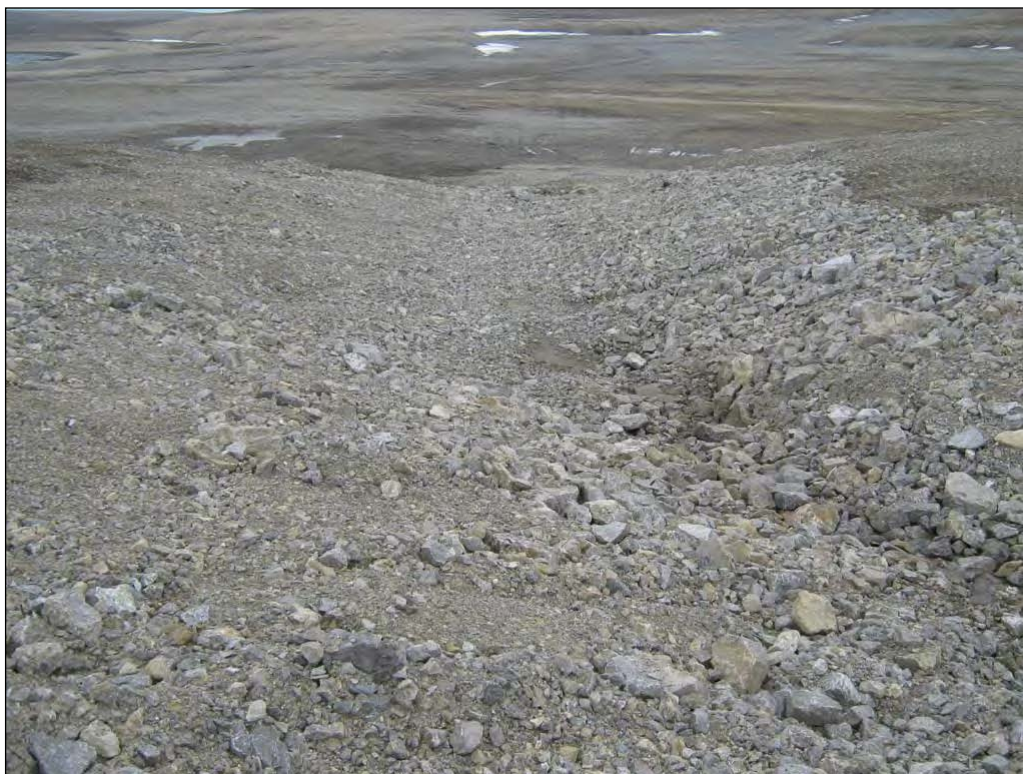
Photograph 50. Stabilized Road Drainage Ditch, South of New Quarry ↑
