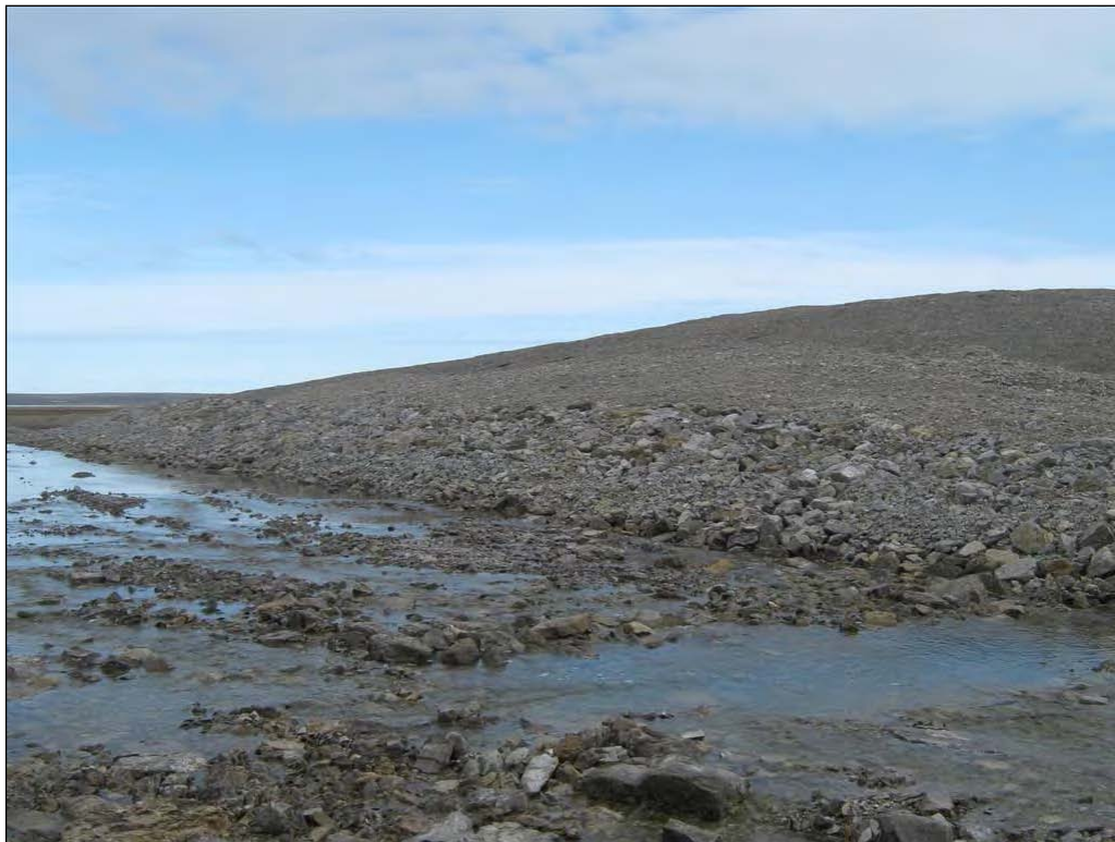
Photograph 25. Garrow Lake Dam, East Abutment ↑
