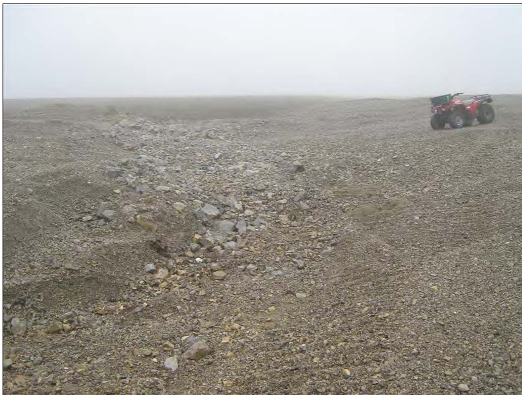
Photograph 64. Rip-Rap lined Drainage Ditch on road to Frustration Lake ↑
