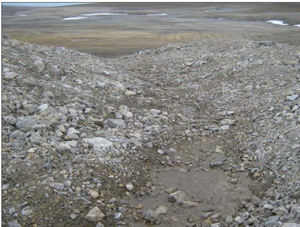
Photograph 52. Stabilized Road Drainage Ditch, South of New Quarry ↑
