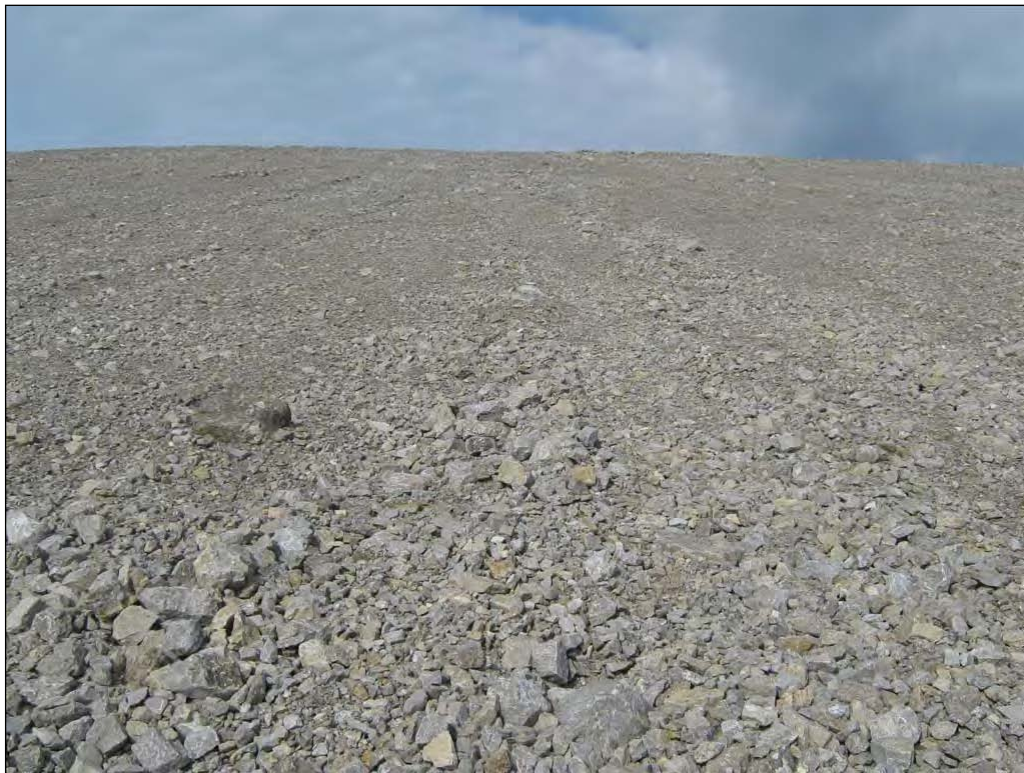
Photograph 15. Operational Landfill, self armouring rills on E slope, view from toe ↑
