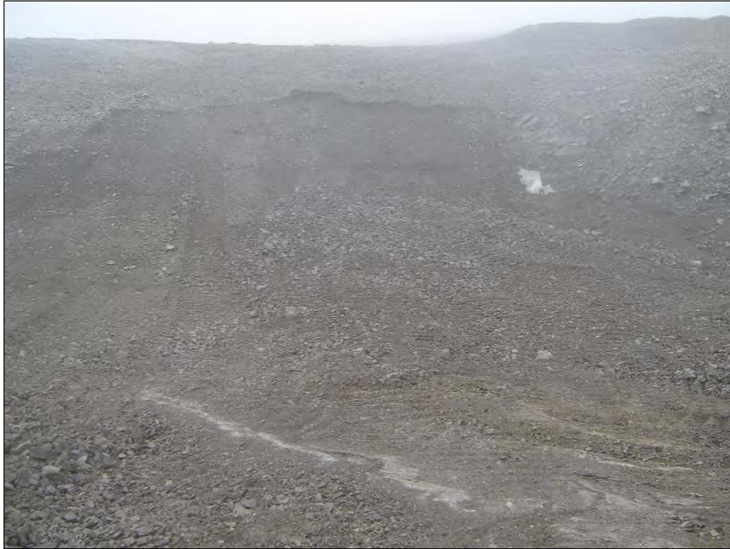
Photograph 73. Main Portal, slope repair completed (July 22/09) ↑
