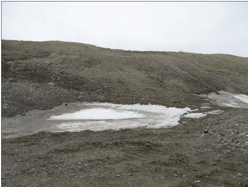
Photograph 49. North Portal, view of backfilled slope ↑
