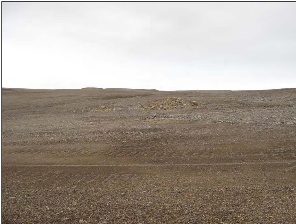
Photograph 27. Subsidence Area, facing South away from ocean ↑
