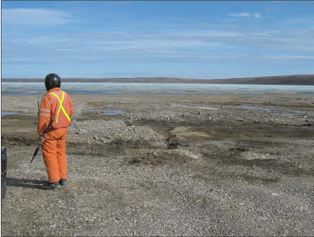
Photograph 21. Wave Break Structure, gravel berm across breached outlet in centre ↑
