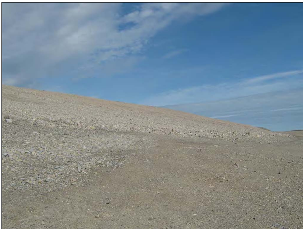
Photograph 18. Operational Landfill, East slope, view from toe ↑
