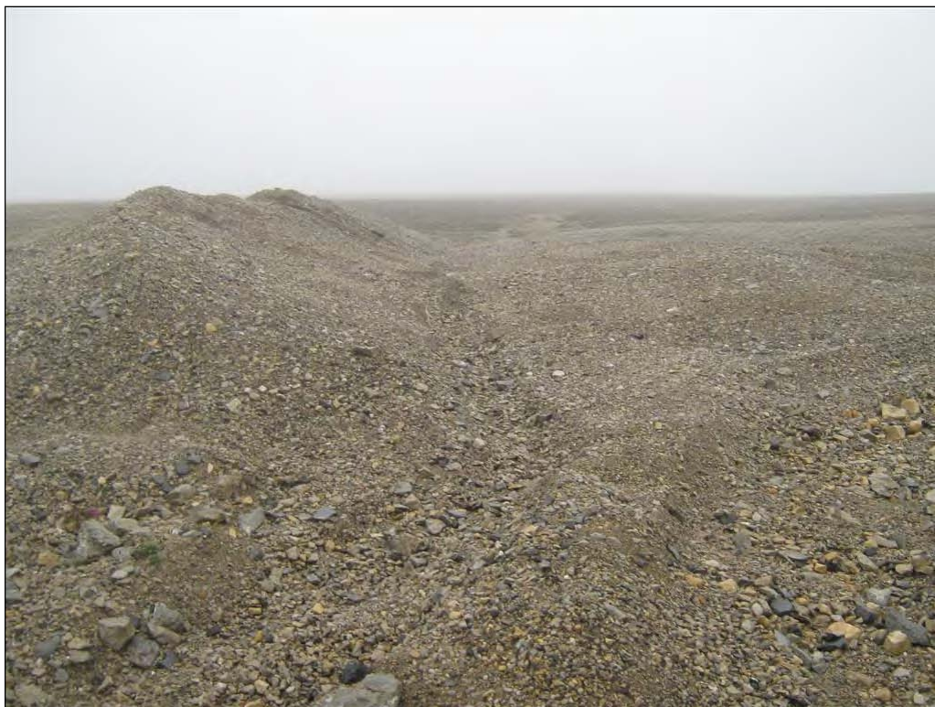
Photograph 66. Repaired Drainage Ditch and Water bar on road to Frustration Lake ↑
