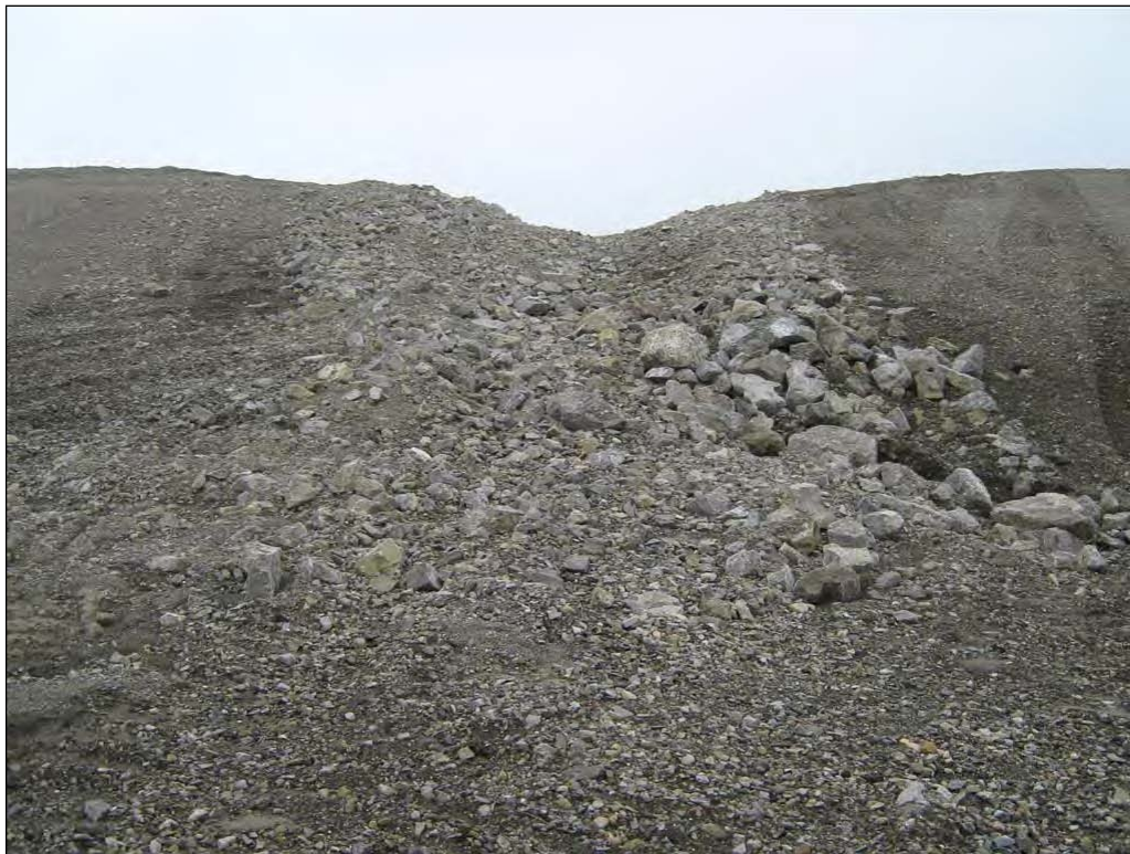
Photograph 53. Stabilized Road Drainage Ditch, South of New Quarry, slope below ditch ↑
