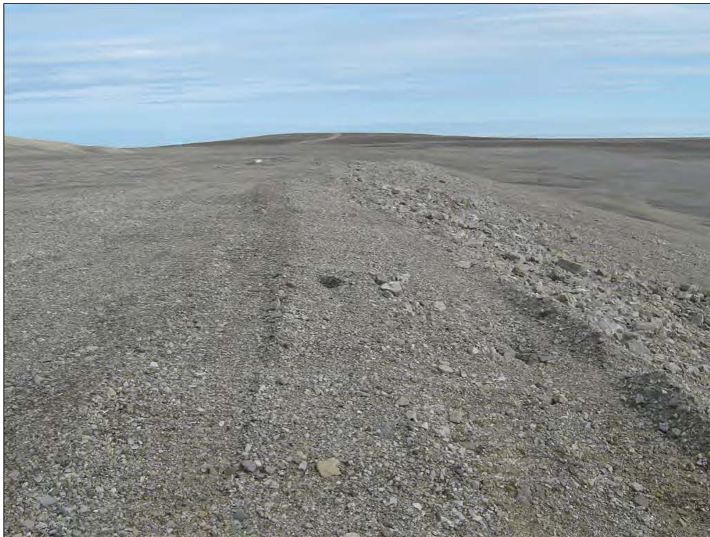
Photograph 7. Operational Landfill, East Crest, facing North along crest ↑
