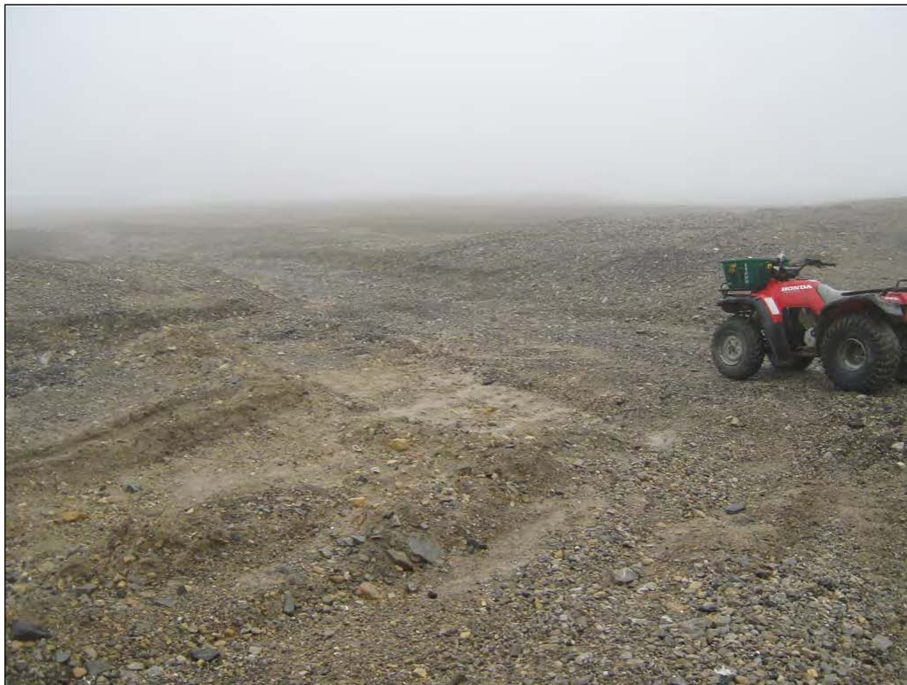
Photograph 67. Repaired Drainage Ditch on road to Frustration Lake ↑
