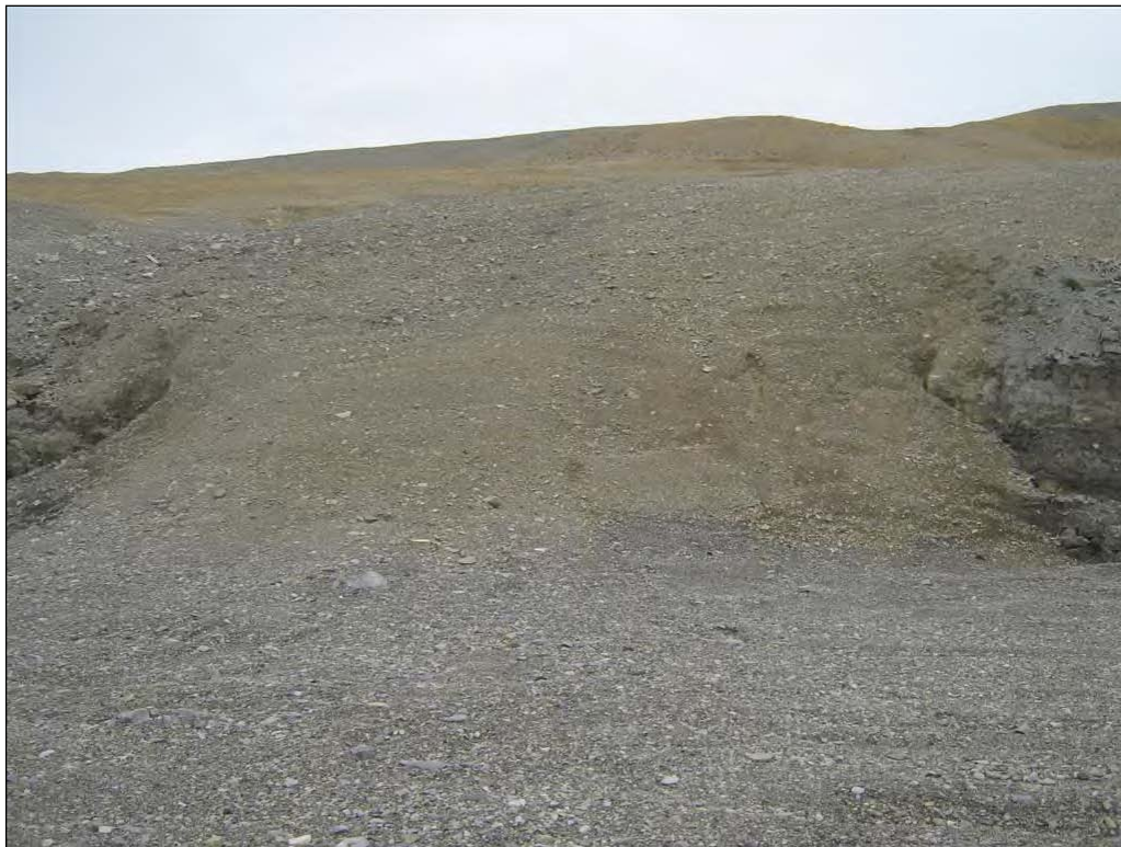
Photograph 35. Conveyor Portal, view of backfilled slope ↑
