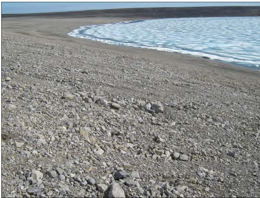
Photograph 10. Operational Landfill, SE Slope, from crest facing North down slope ↑
