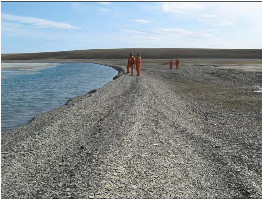
Photograph 22. Wave Break Structure, crest of gravel berm across breached outlet ↑
