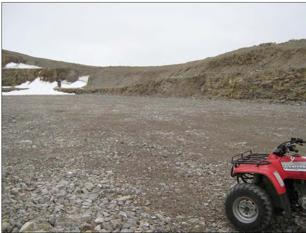
Photograph 44. Little Red Dog Quarry, rockfill cover, view from West end ↑
