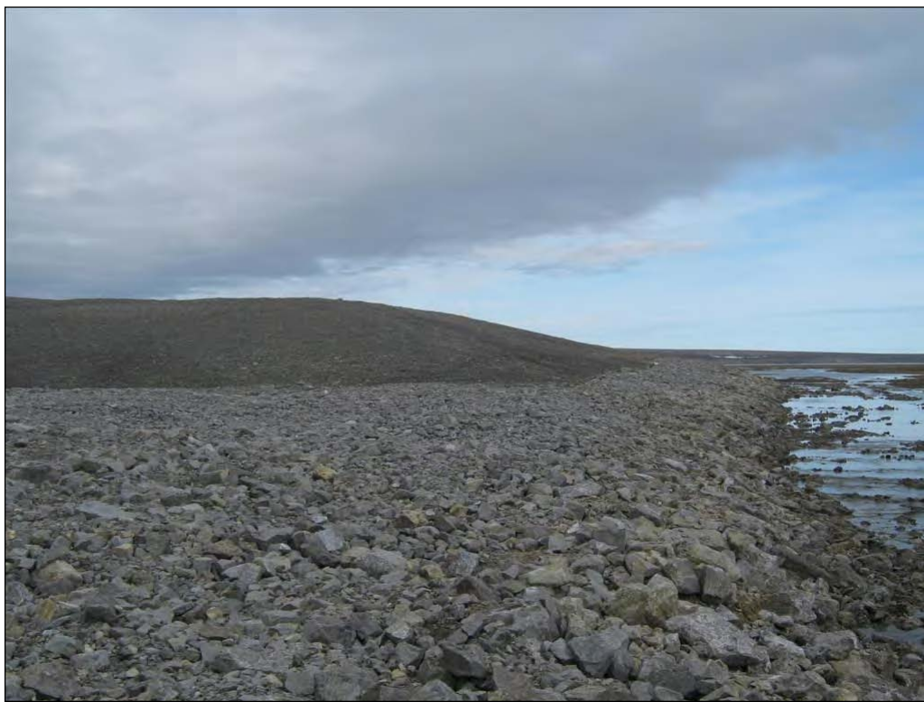
Photograph 26. Garrow Lake Dam, West Abutment ↑
