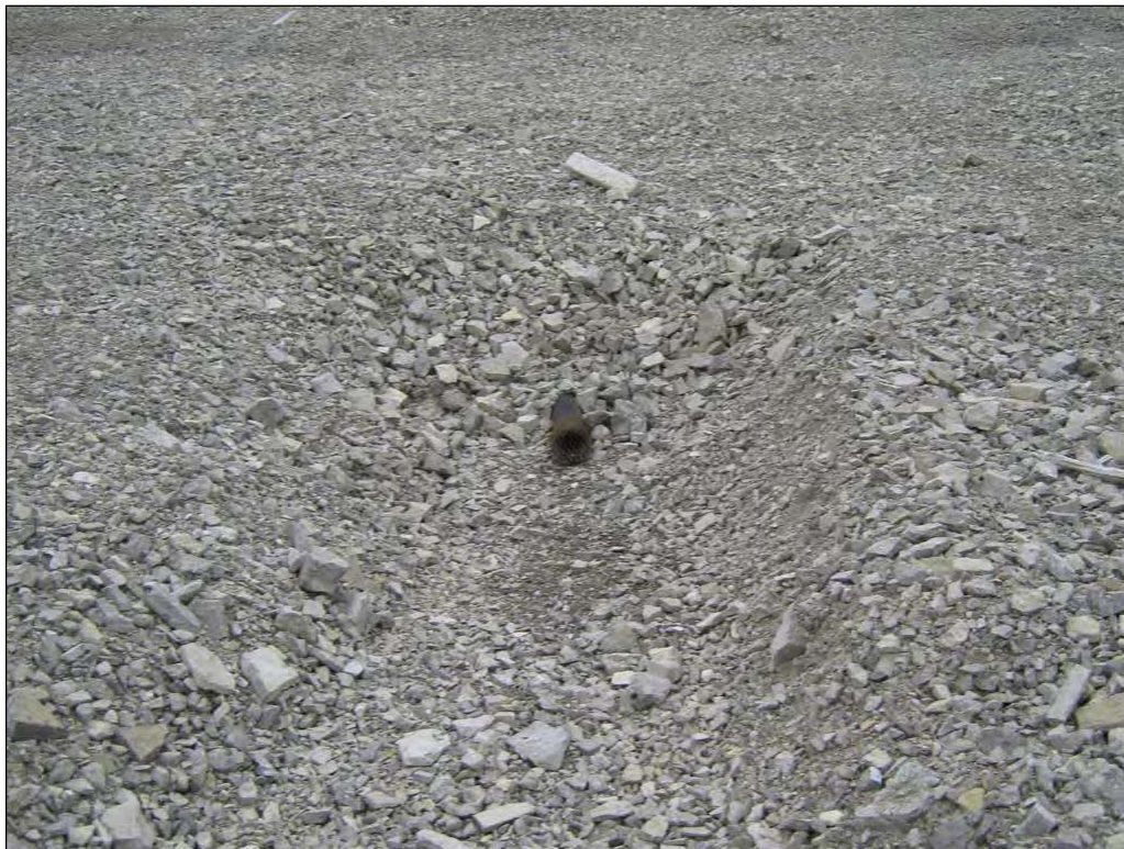
Photograph 33. Exploration Portal, view of vent pipe through backfill ↑
