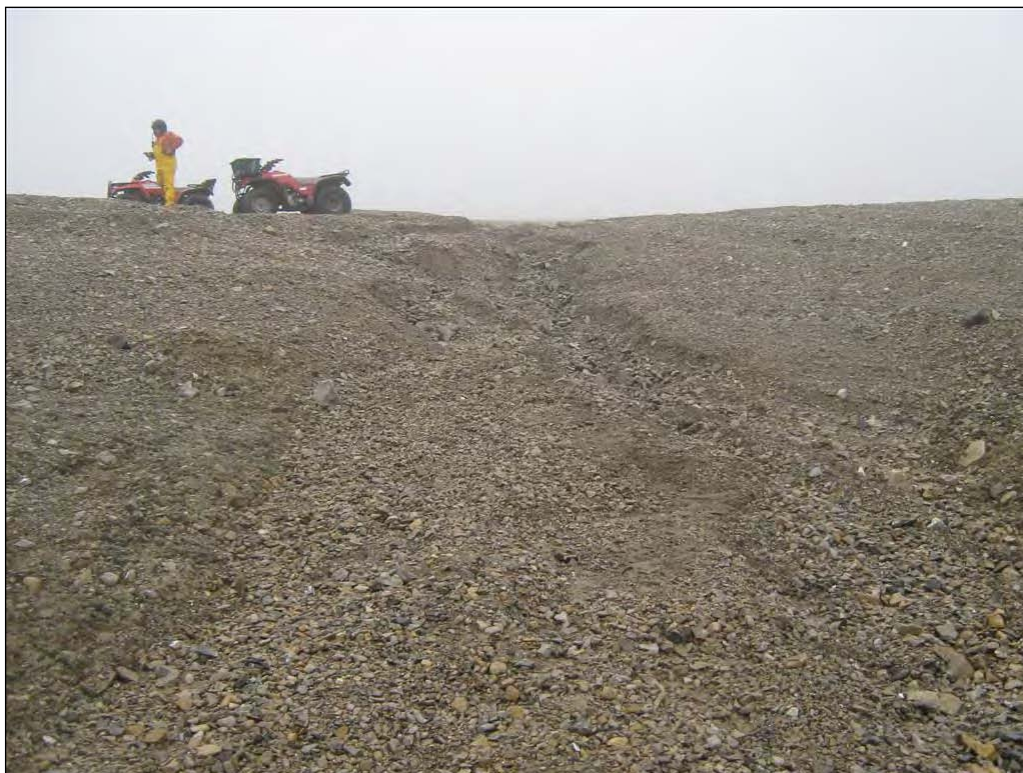
Photograph 68. Stabilized Erosion Gully on road to Frustration Lake ↑
