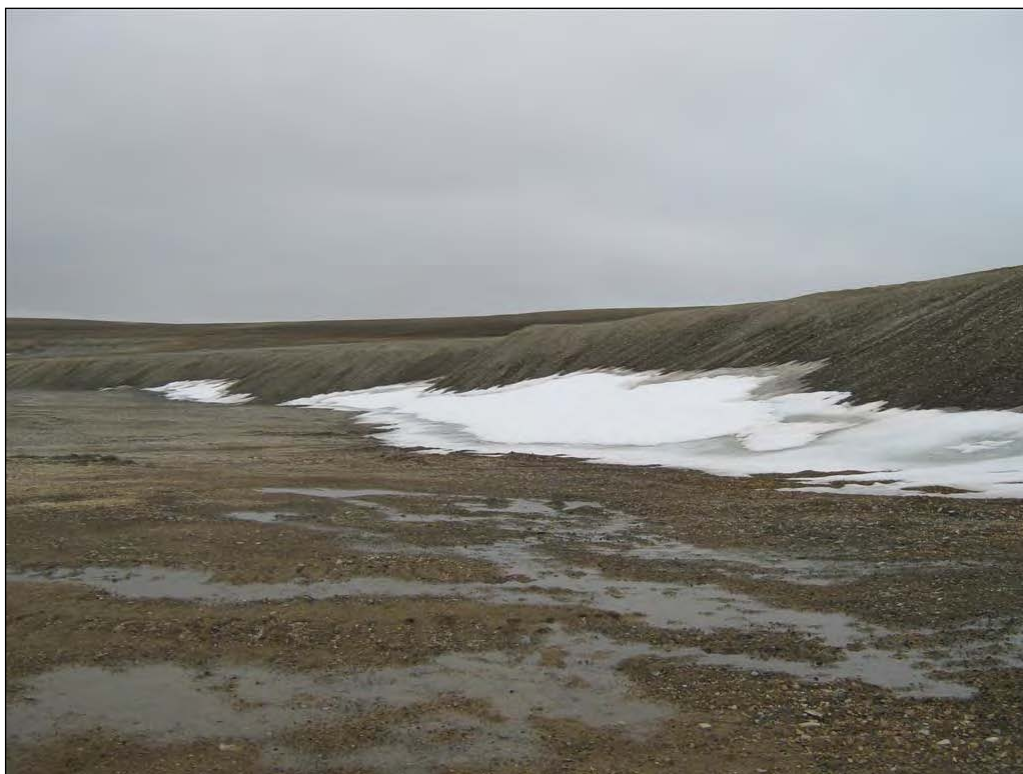
Photograph 55. New Quarry, South perimeter slope ↑
