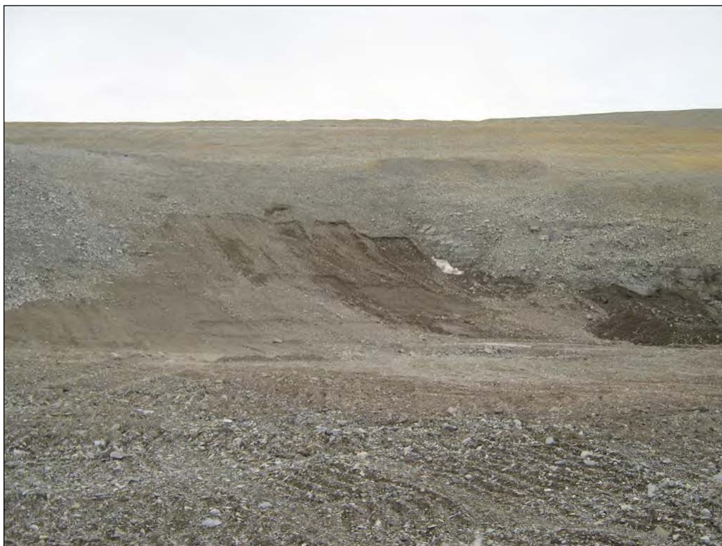
Photograph 34. Main Portal, slope repair in progress (July 21/09) ↑
