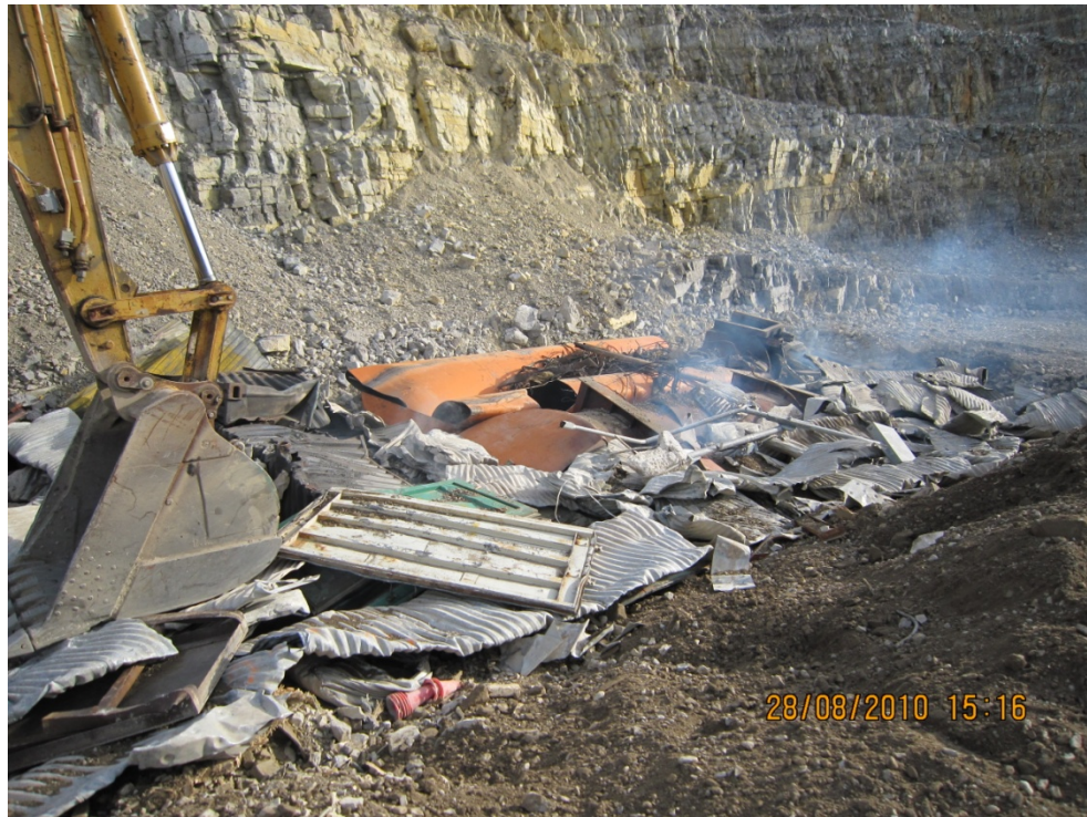
Photo #45 – Debris Being Packed into Excavation.
