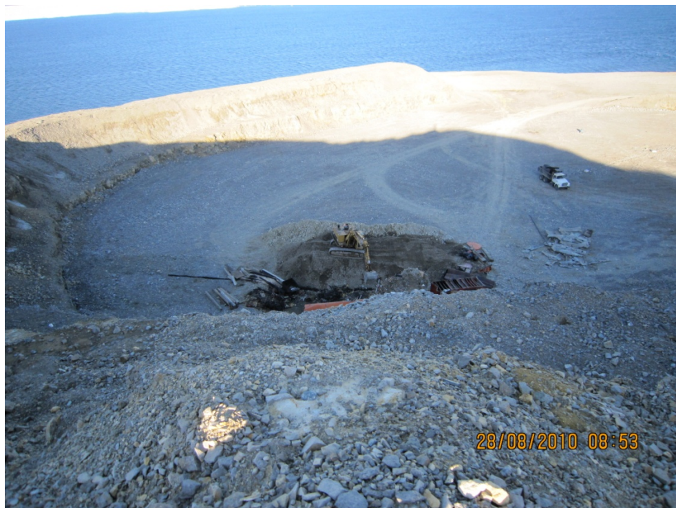
Photo #44 – Excavator On Top of Spoil Pile Placing Debris into Excavation
