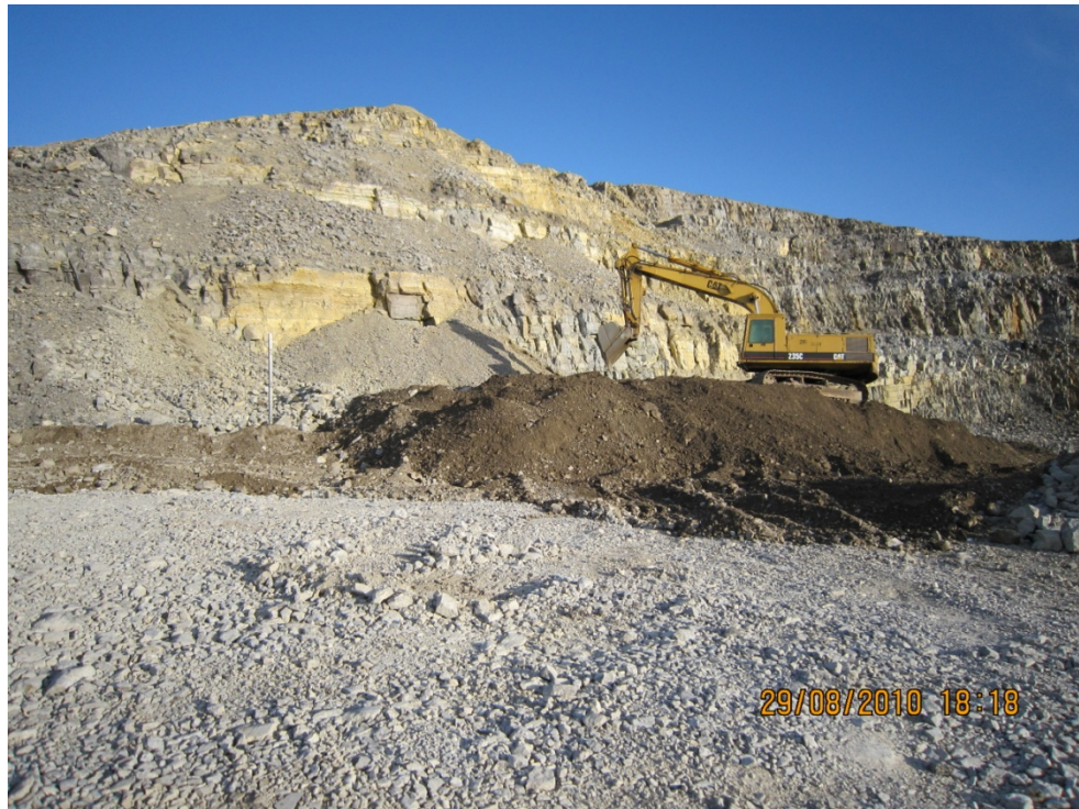
Photo #53 – Capping Process Continuing
