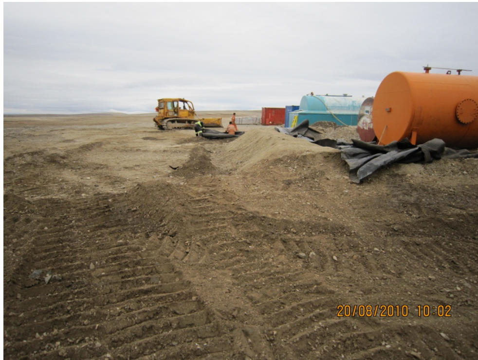
Photo #21 – Removing Liner from Top of Dirt Berm
