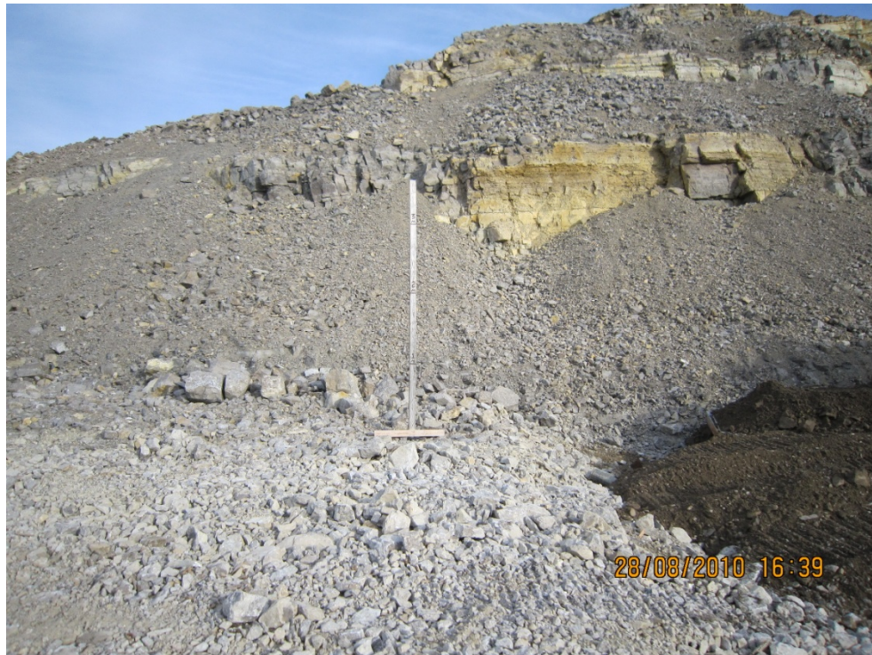
Photo #51 – North Fill Grade Stake
