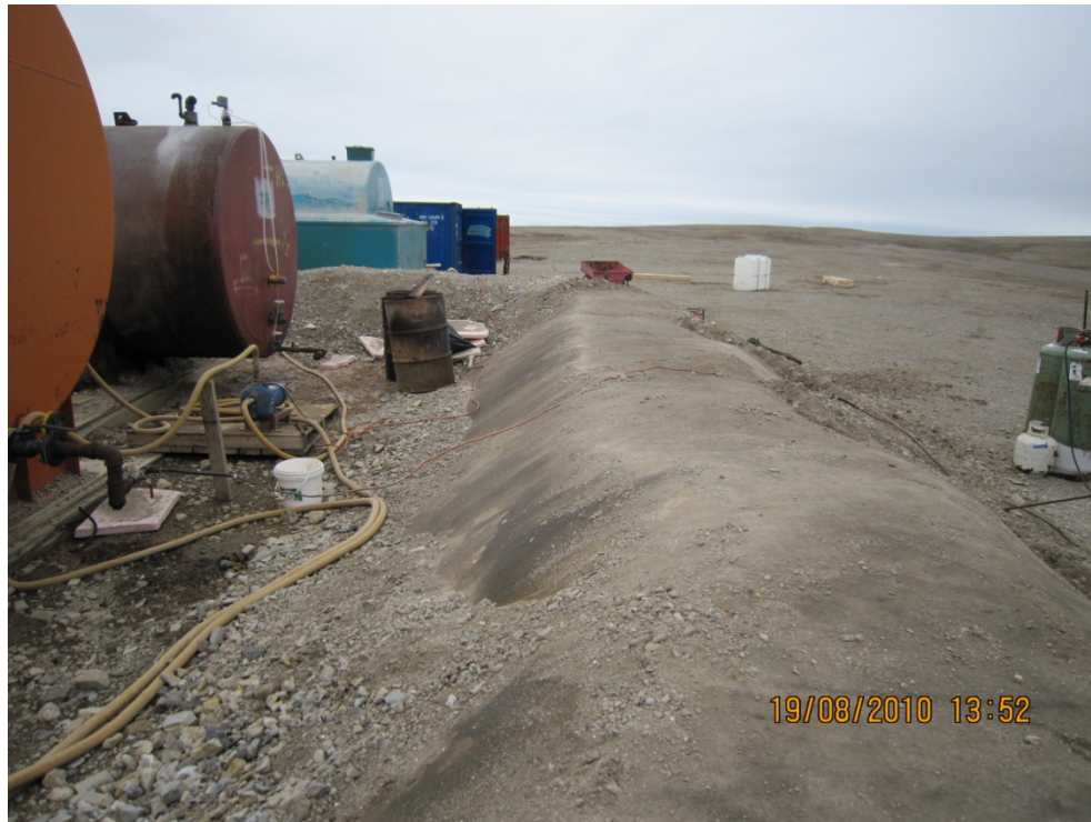
Photo #19 – Fuel Storage Spill Containment Area - Removing Dirt Cover from Liner on Berm
