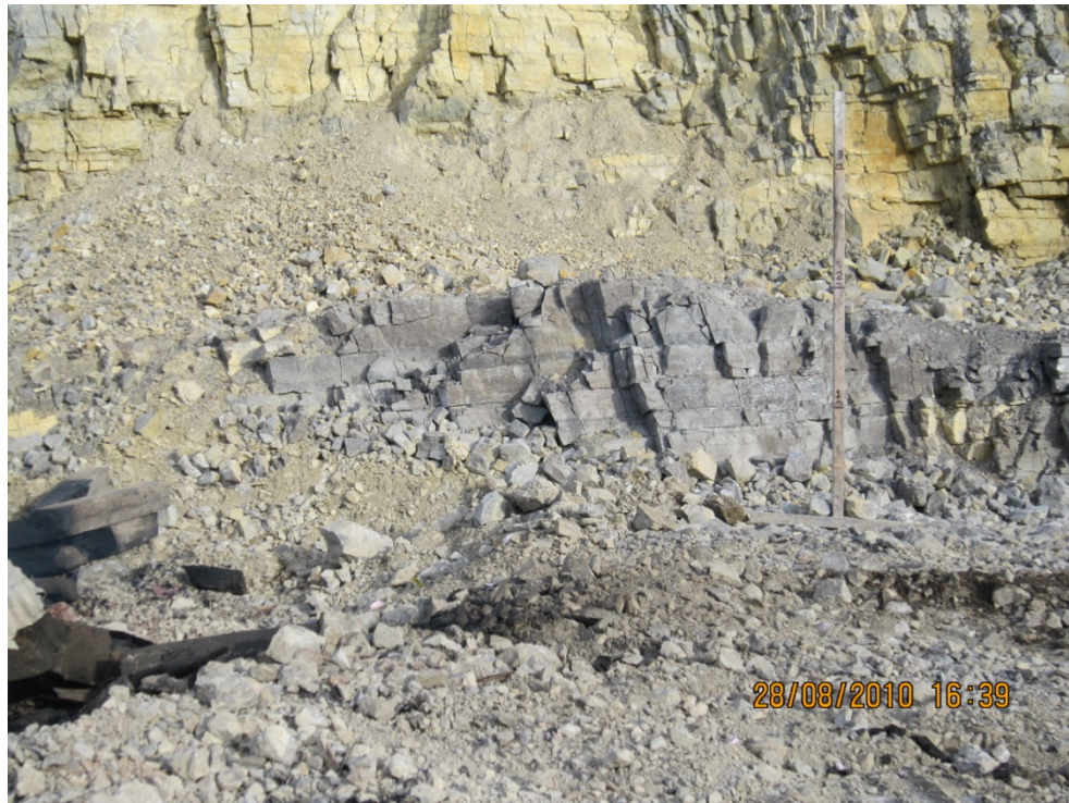
Photo #49 – South Fill Grade Stake (Marked in 1 M intervals – 3 M total)
