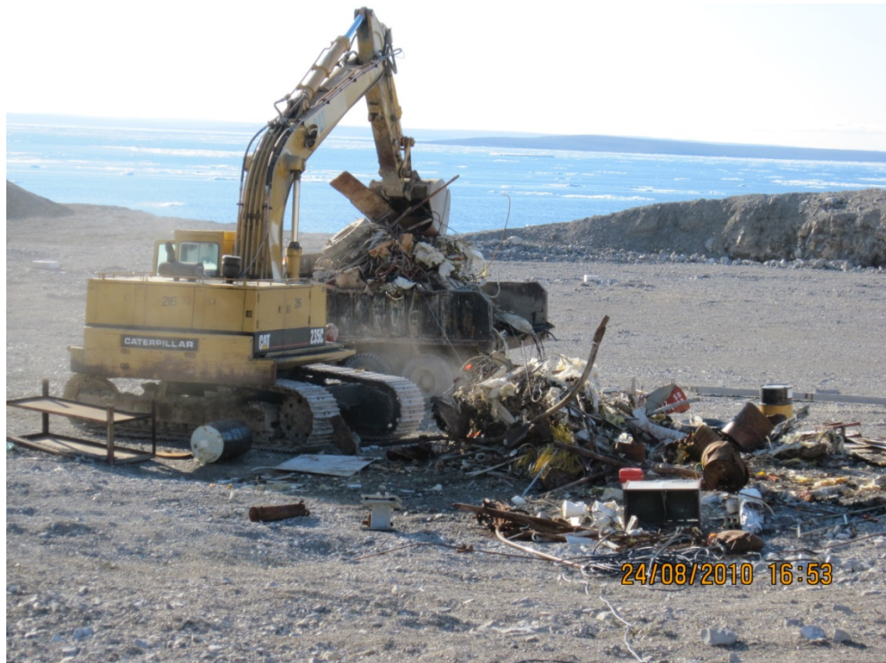
Photo #41 – Debris Collected During Annual Inspection Trips Being Hauled to Excavation
