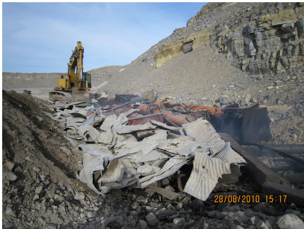
Photo #46 – Extent of Excavation and Debris Being Buried
