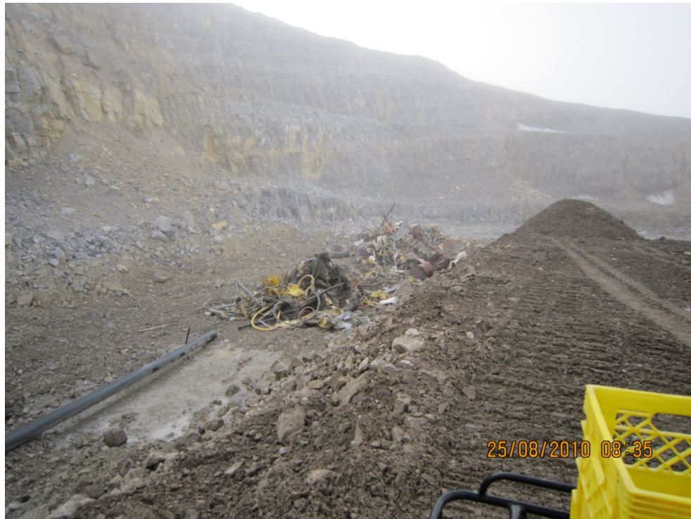
Photo #43 – Initial Debris Placed into Excavation
