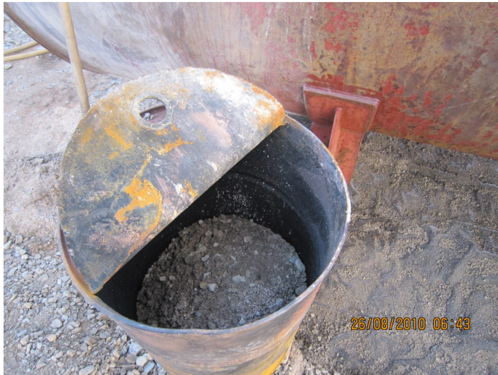
Photo #29 – Collecting Hydrocarbon Dirt From Within Fuel Storage Containment Area
