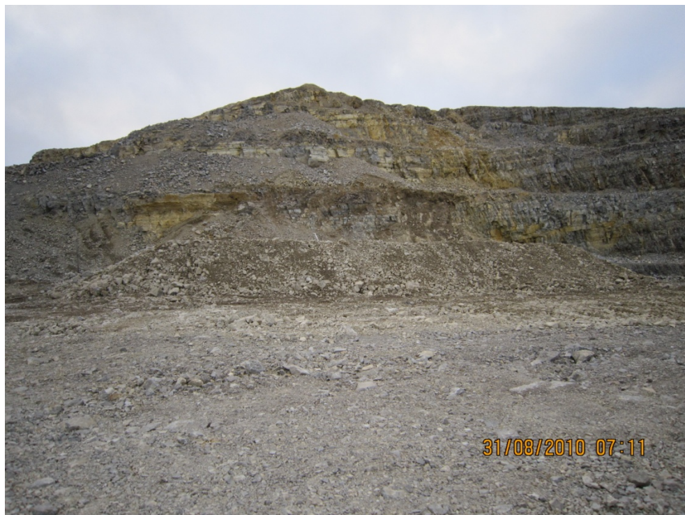
Photo #58 – View of Finished Cap
