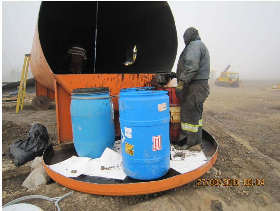
Photo #31 – Cleaning of Empty Fuel Tank
