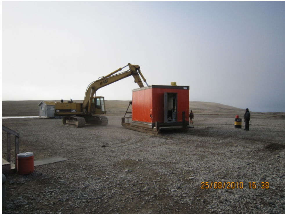
Photo #7 – Preparing Small Accommodation Trailer on Skid
