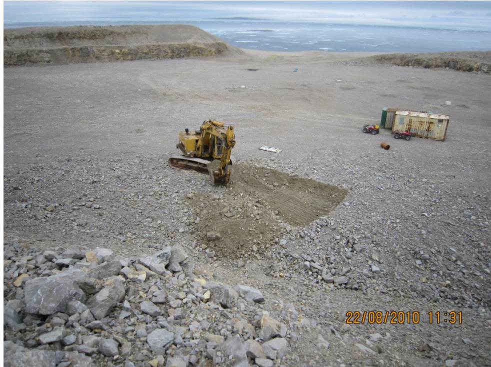
Photo #39 – Starting to Dig Cover Cap Where Final Debris Will Be Disposed
