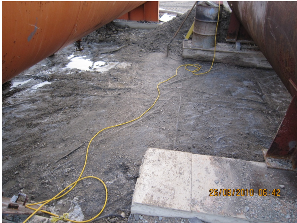
Photo #27 – Intact Liner Below Fuel Storage Tanks
