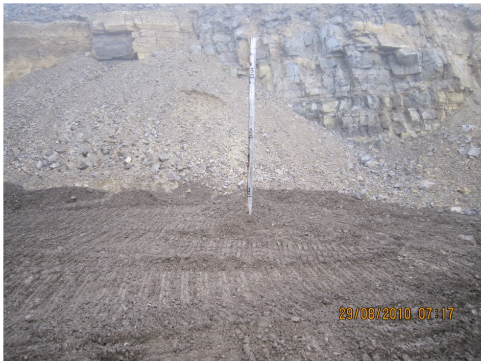
Photo #52 – Capping Continuing – Almost At 1 M Mark of Centre Fill Grade Stake
