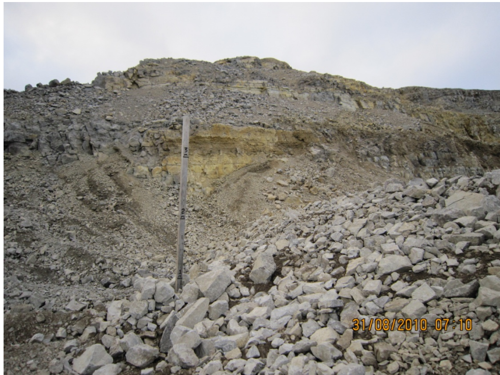
Photo #55 – North Fill Stake At Toe of North End of Cap
