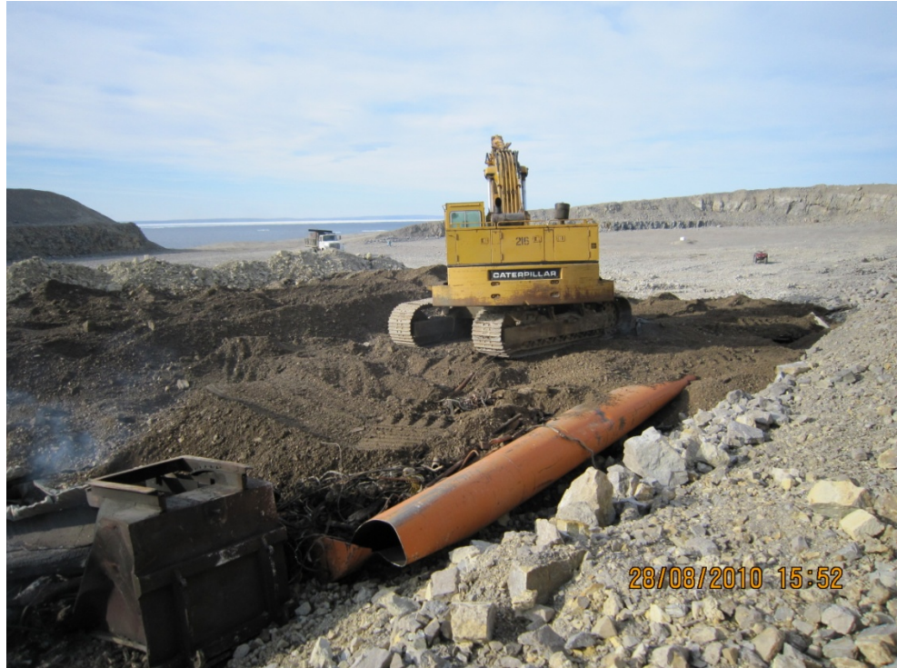
Photo #47 – Initial Fine Fill Being Placed On Top of Debris
