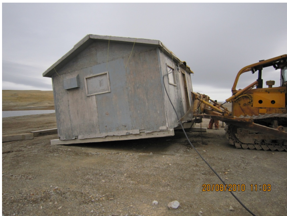
Photo #8 – Preparing Wood Accommodation Building to Move
