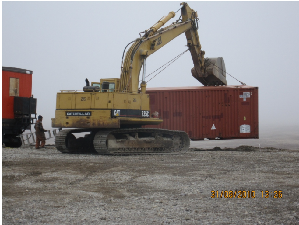
Photo #11 – Moving Sea Container to Place on Towing Skid
