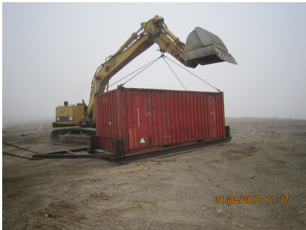
Photo #12 – Placing Sea Container on Towing Skid
