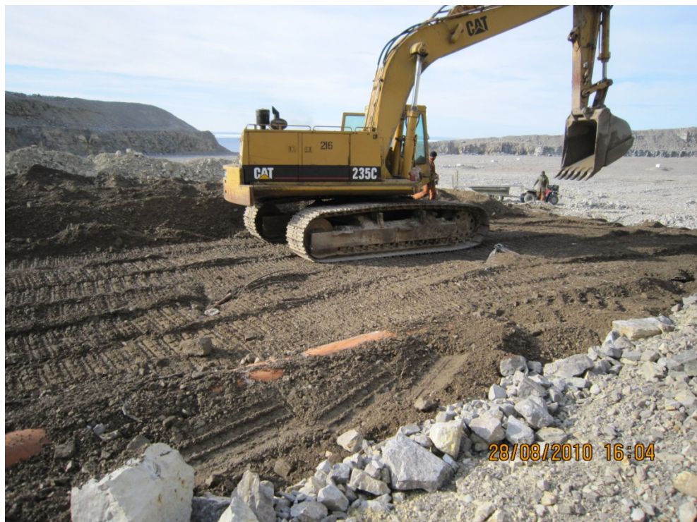
Photo #48 – Finishing Burial of Debris (0 M mark for fill stakes)
