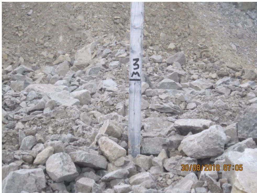
Photo #54 – Coarse Cover – Cap Now At 2.5 M Thickness (centre grade stake)
