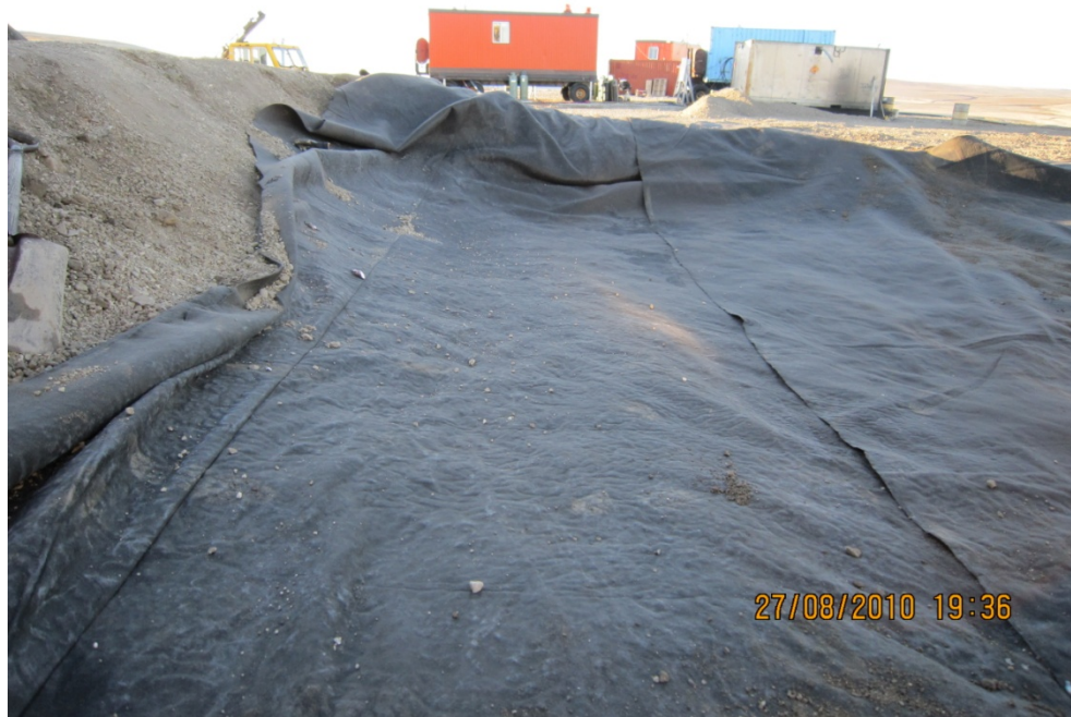
Photo #35 – Fuel Containment Liner Just Prior to Packing
