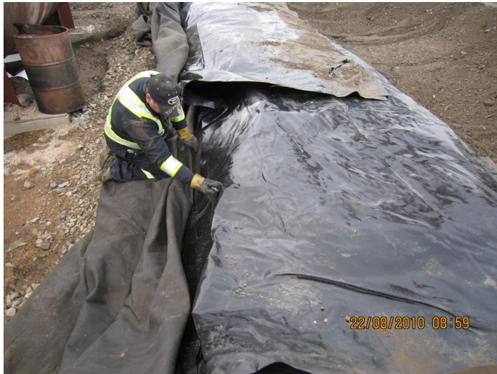
Photo #25 – Cutting Out Containment Liner Over Top of Berm (Note the integrity of the liner)
