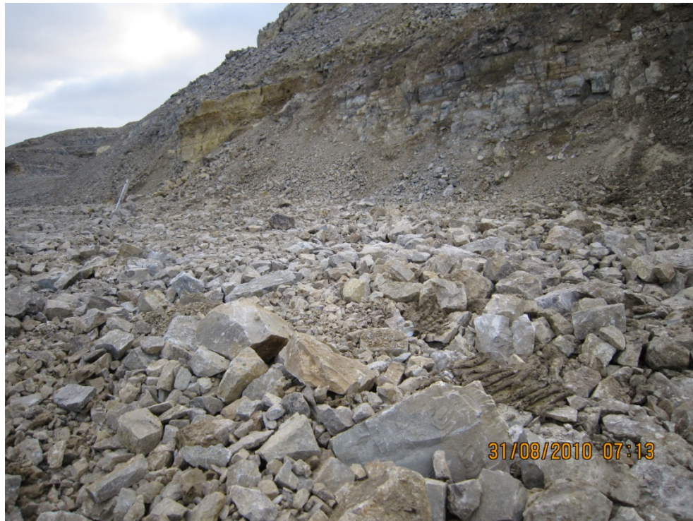
Photo #57 – Top of Cap Tied Into Pit Wall
