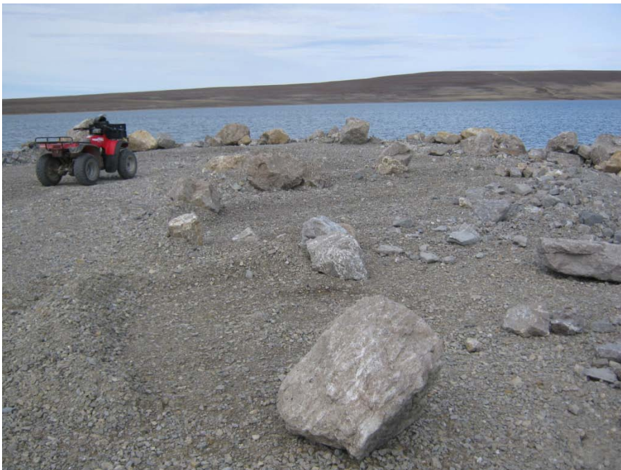
Photo 120, Frustration Lake, End of Jetty (0.5m diameter boulders pushed onto end of jetty)
