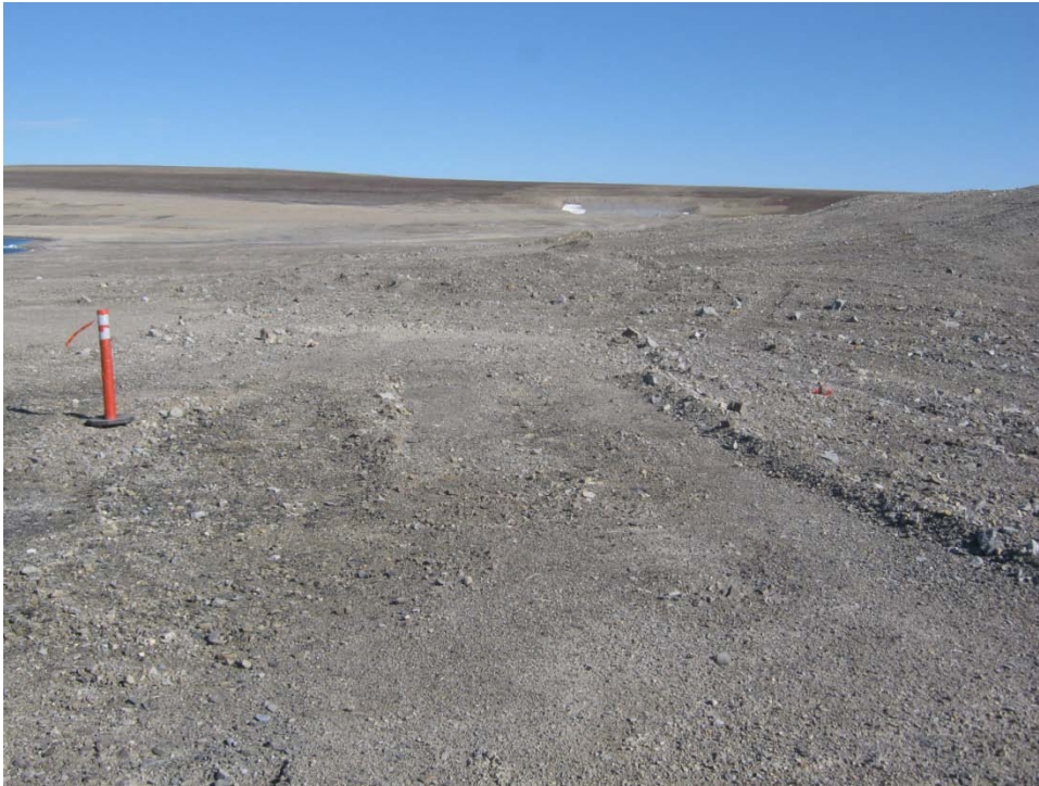
Photo 53, Subsidence Area, Northwest end, Facing East
