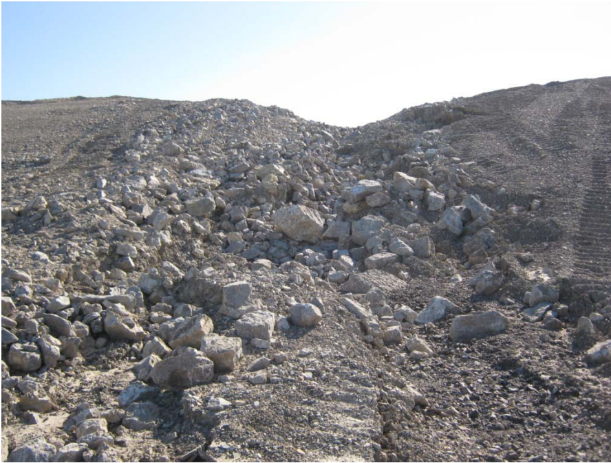
Photo 71, New Quarry, Drainage ditch at West end, Rip-Rap lined ditch facing upstream (from bottom)
