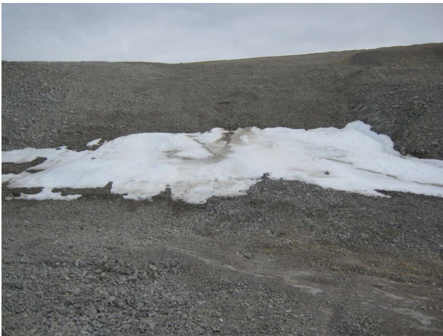
Photo 108, Mine Portals, Main Portal, Gravel backfilled slope over Main Portal
