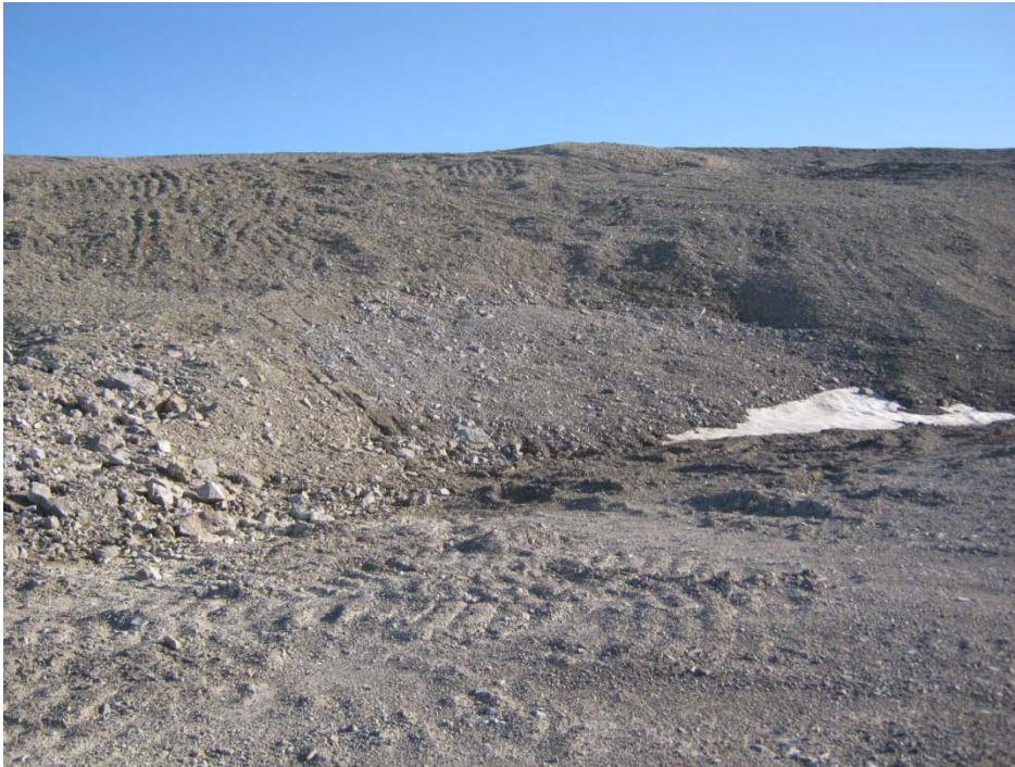
Photo 89, Mine Portals, North Portal, Gravel backfilled slope over North Portal
