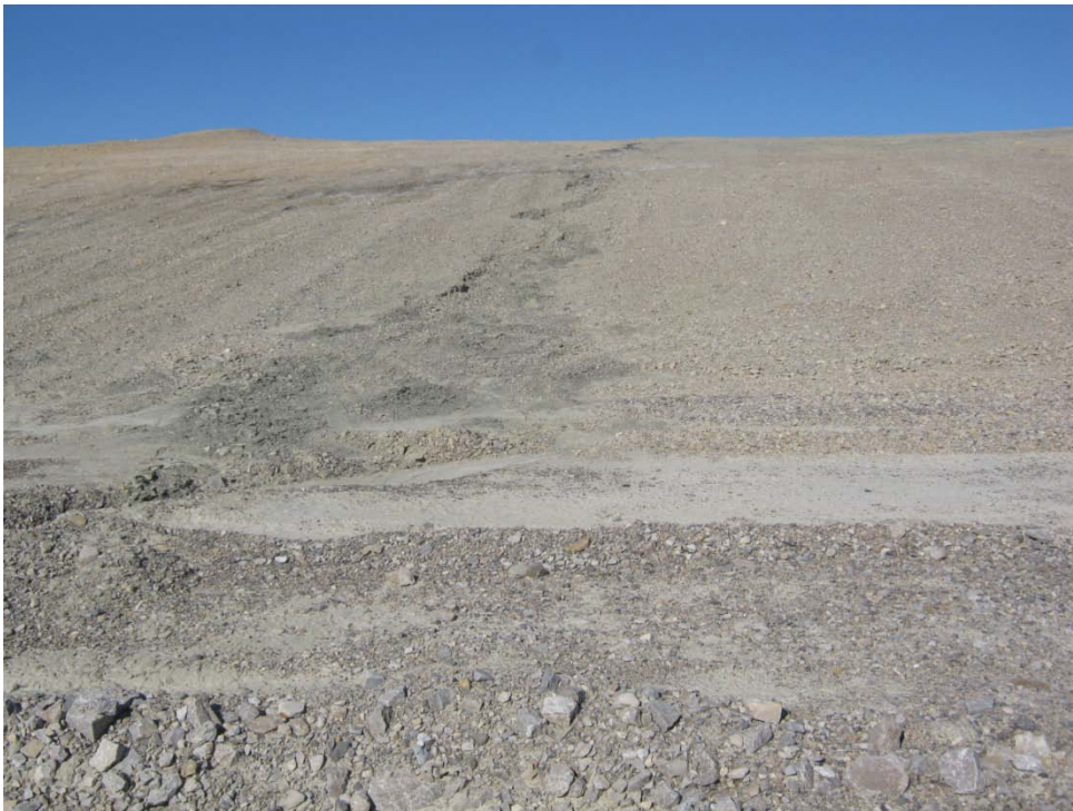
Photo 24, Operational Landfill, Back of Crest, Upslope erosion gulley above landfill
