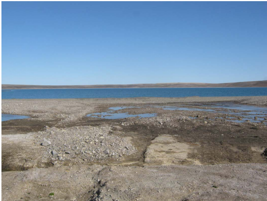
Photo 36, Garrow Lake, Downstream of Wave Break, Facing wave break structure
