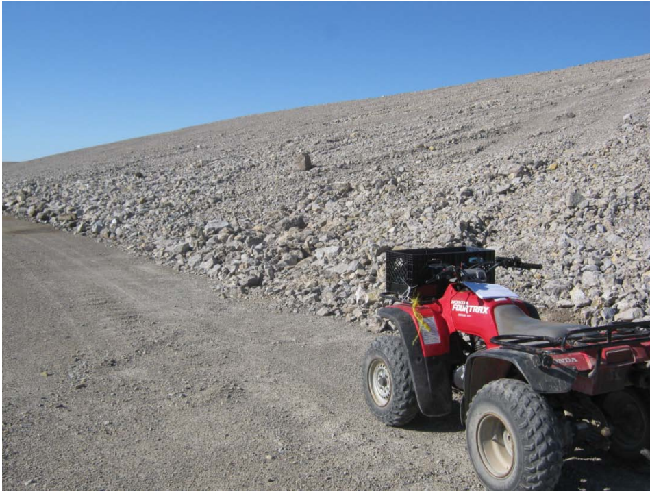
Photo 11, Operational Landfill, Northeast Toe, Facing South across slope
