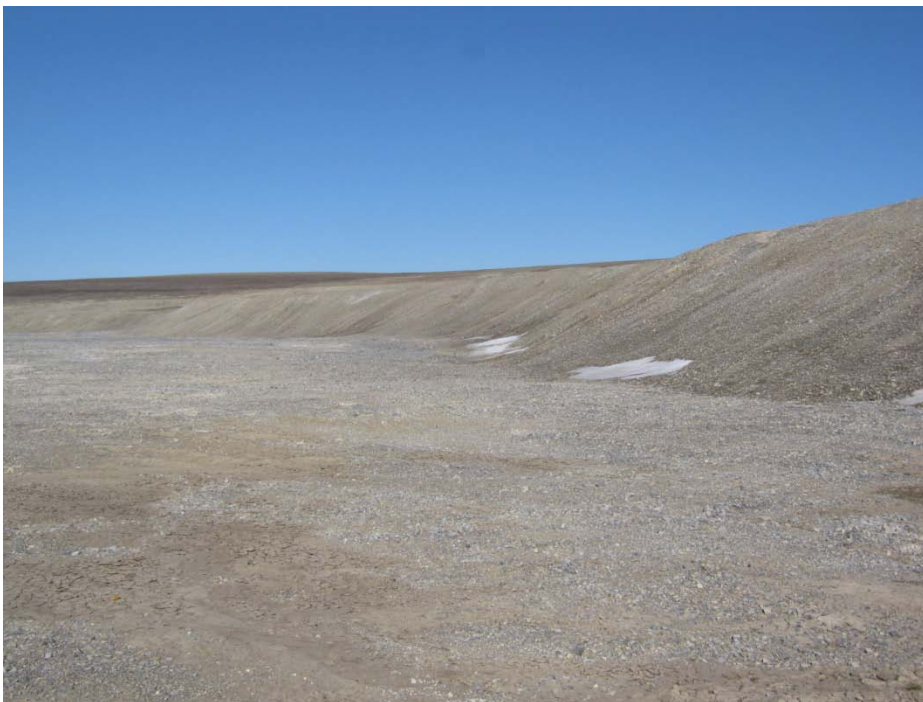
Photo 74, New Quarry, Southwest perimeter slope, Facing Southeast along the slope
