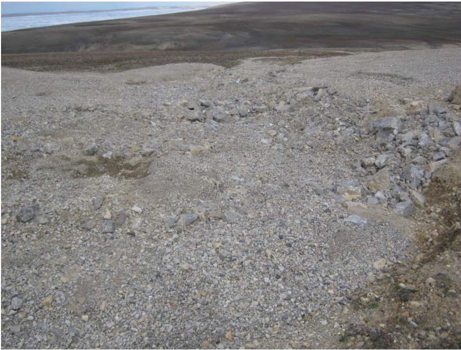
Photo 113, Frustration Lake, Rip-Rap lined drainage ditch across road
