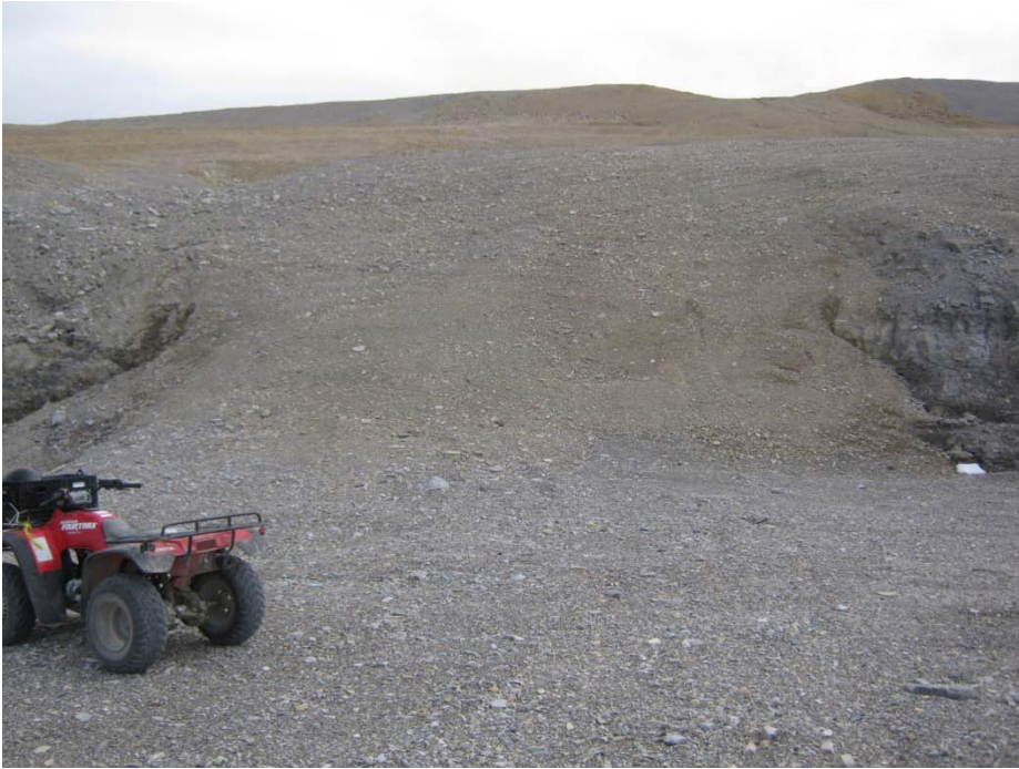
Photo 107, Mine Portals, Conveyor Portal, Gravel backfilled slope over Conveyor Portal
