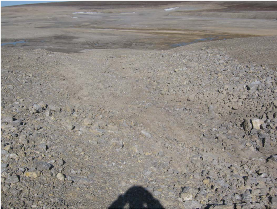
Photo 69, New Quarry, Drainage ditch at West end, Rip-Rap lined ditch facing downstream
