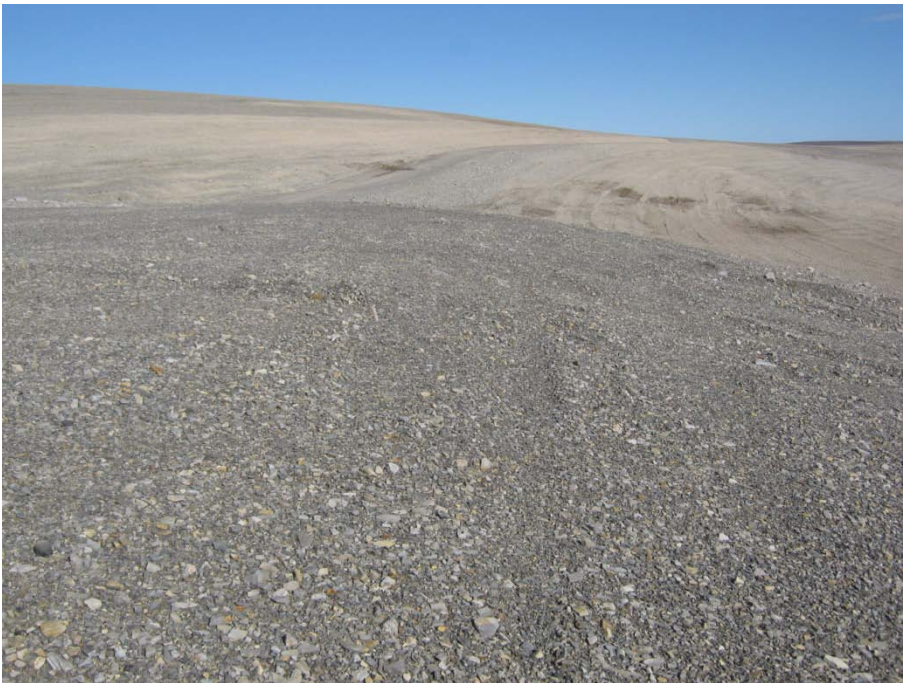
Photo 6, Operational Landfill, Northeast Crest, Facing Northwest
