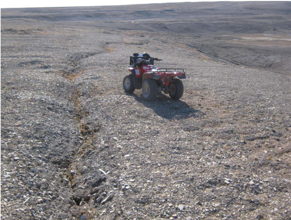
Photo 88, New Quarry, Top of Southwest slope, Old tension crack healed with erosion
