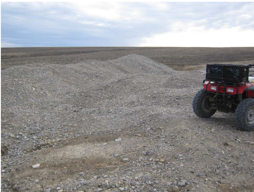
Photo 114, Frustration Lake, Water bar and self-armouring drainage ditch across road
