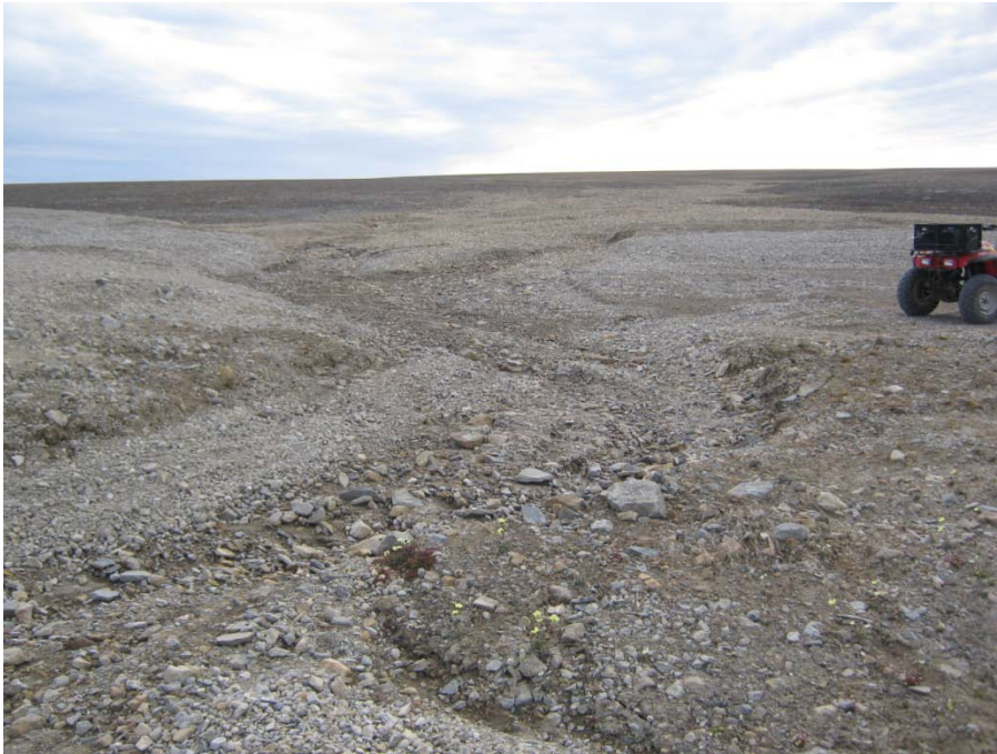
Photo 119, Frustration Lake, Self-armouring drainage ditch across road
