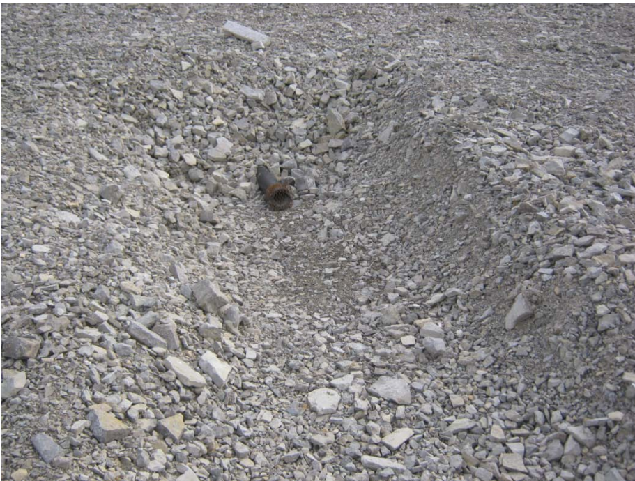
Photo 112, Mine Portals, Exploration Portal, Gravel backfilled slope (exposed ventilation pipe)
