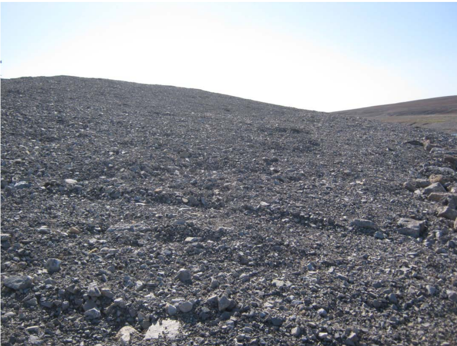
Photo 32, Garrow Lake Dam, East abutment, Upslope of East breach slope
