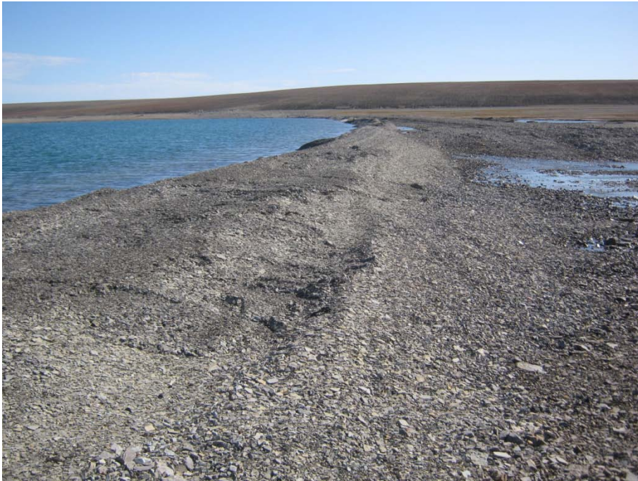
Photo 37, Garrow Lake, Wave Break Breach, Along crest of gravel berm forming at outlet
