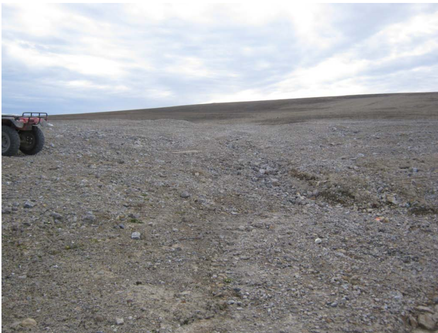
Photo 118, Frustration Lake, Self-armouring drainage ditch across road
