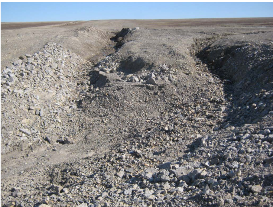
Photo 68, New Quarry, Drainage Ditch at West end, Rip-Rap lined ditch facing upstream
