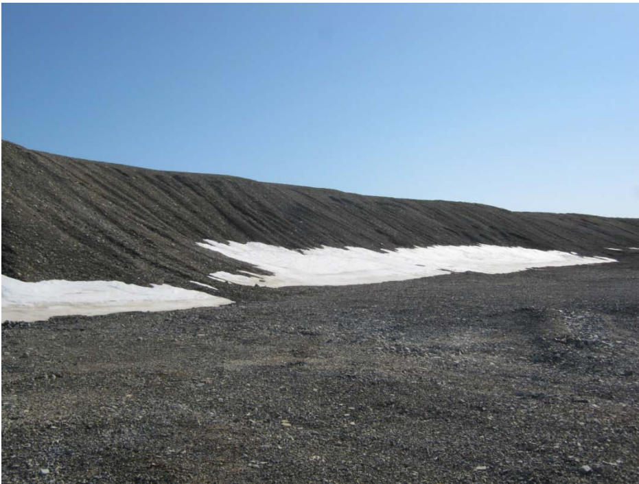
Photo 72, New Quarry, Southwest perimeter slope, Facing Southwest along slope
