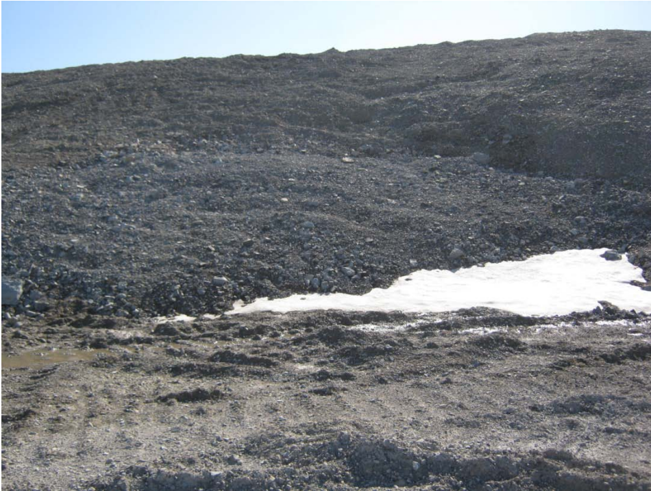
Photo 51, Mine Portals, North Portal, Gravel backfilled slope over North portal
