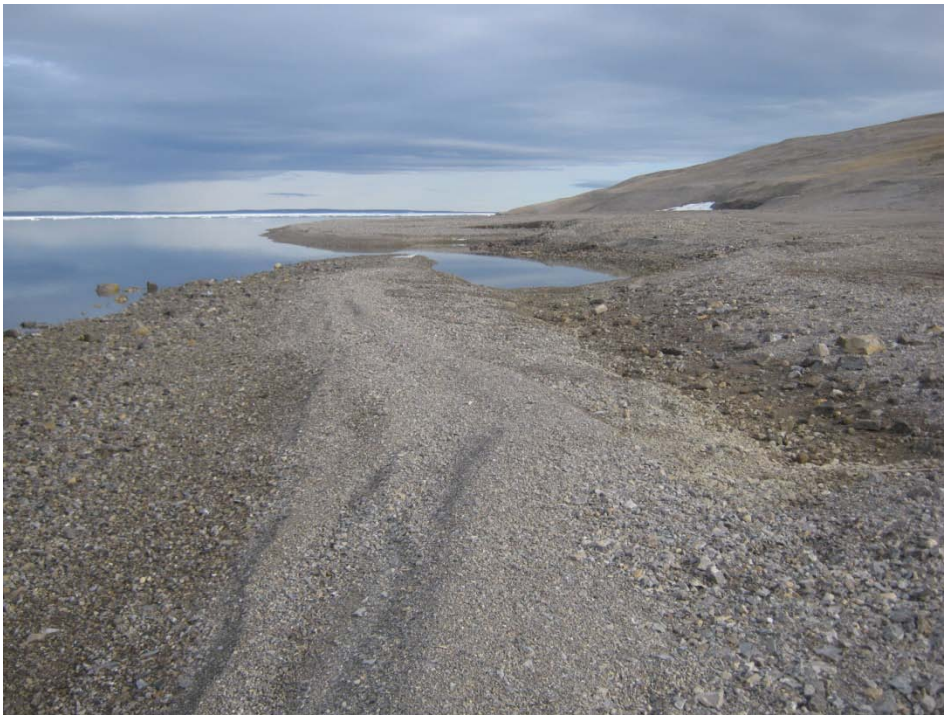
Photo 95, Foreshore, South end, Facing North along shoreline (thaw settlement)
