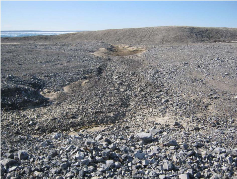
Photo 85, New Quarry, Central drainage ditch, Facing North
