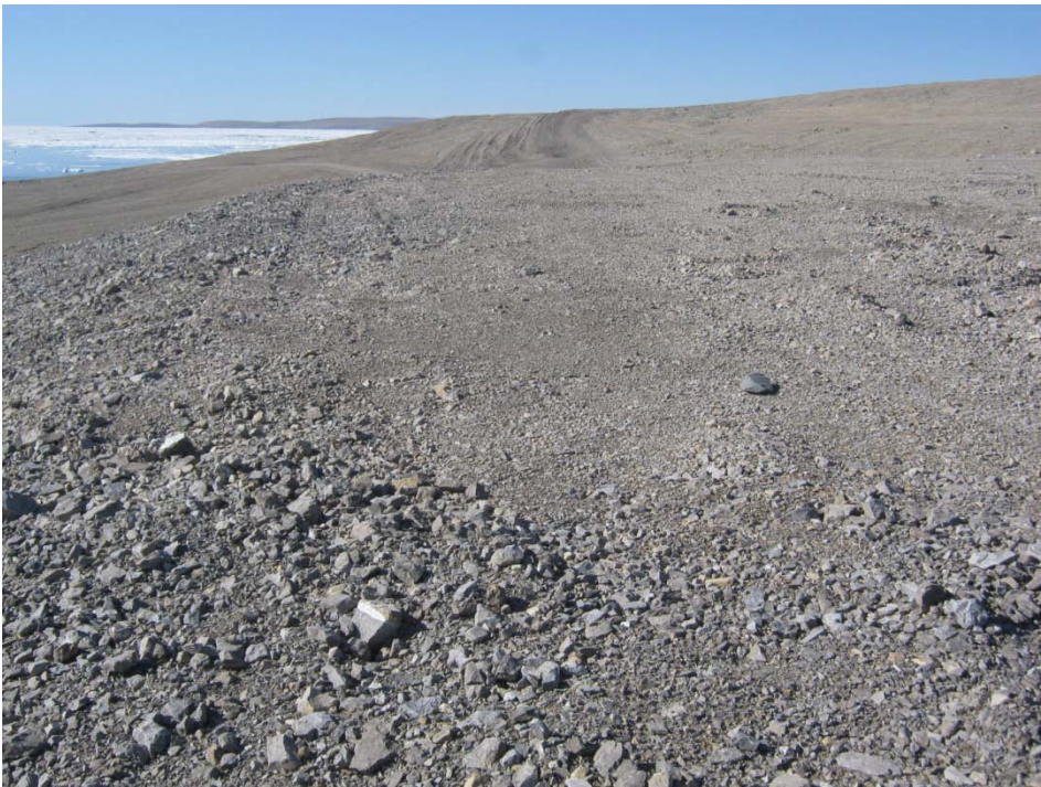
Photo 20, Operational Landfill, South Crest, Facing Southwest along crest
