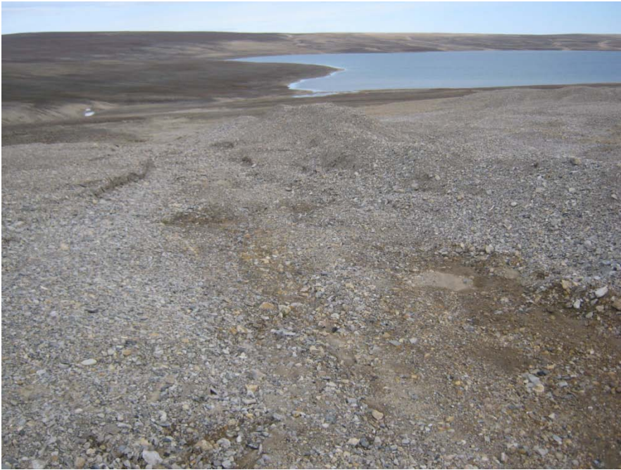
Photo 115, Frustration Lake, Water bar and self-armouring drainage ditch across road
