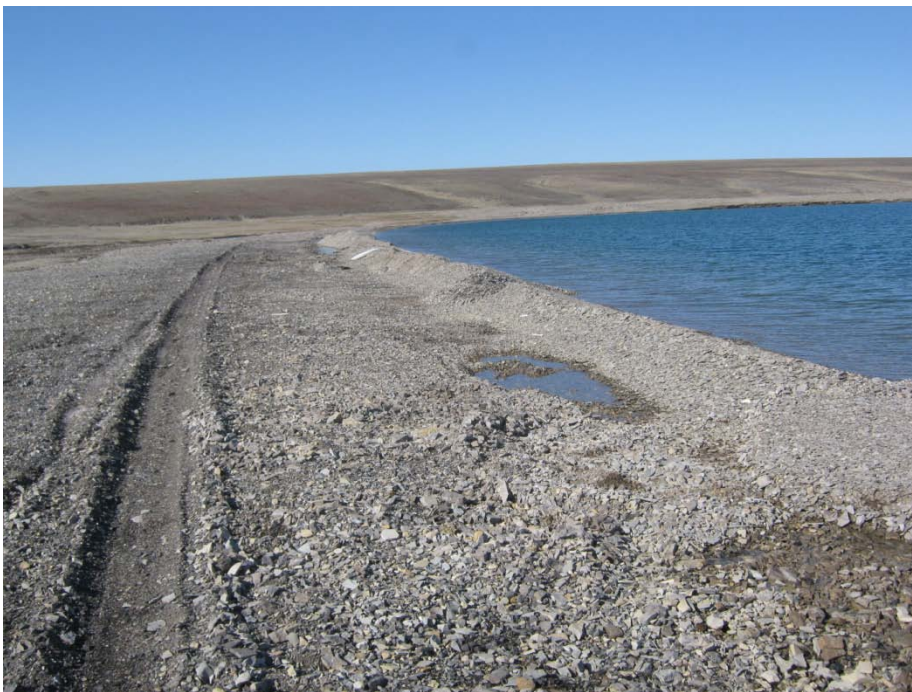
Photo 38, Garrow Lake, East end of Wave Break, Gravel berm
