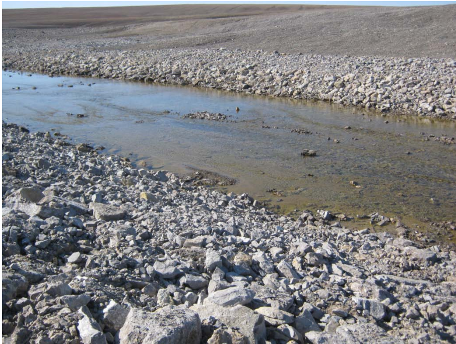
Photo 33, Garrow Lake Dam, Channel from East abutment
