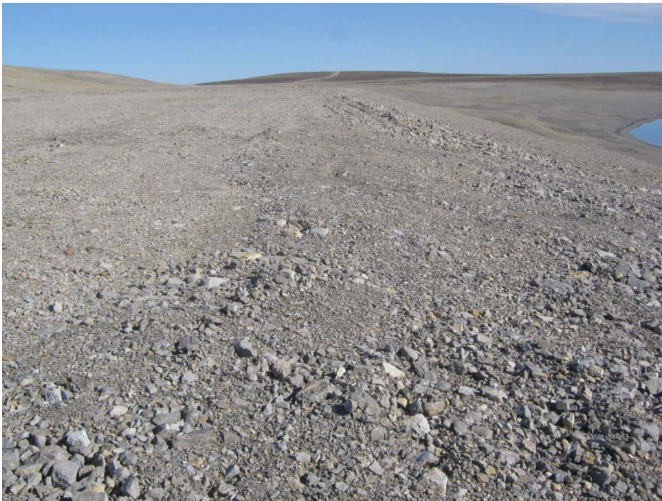
Photo 18, Operational Landfill, South Crest, Facing North along crest
