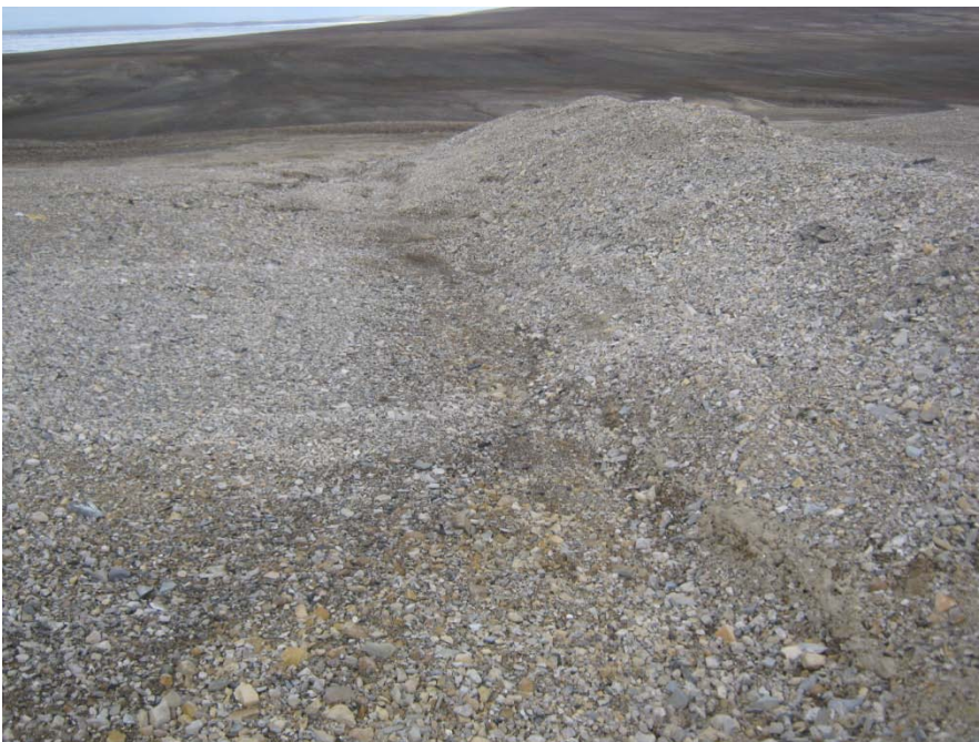
Photo 116, Frustration Lake, Water bar and self-armouring drainage ditch across road
