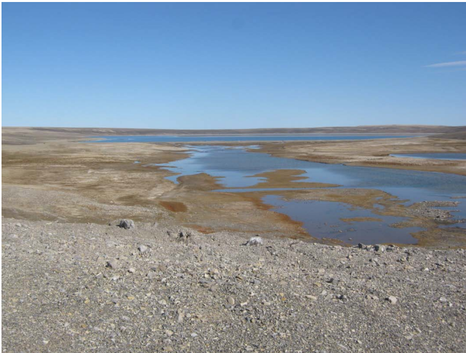
Photo 26, Garrow Lake, Facing wave break structure from West dam abutment
