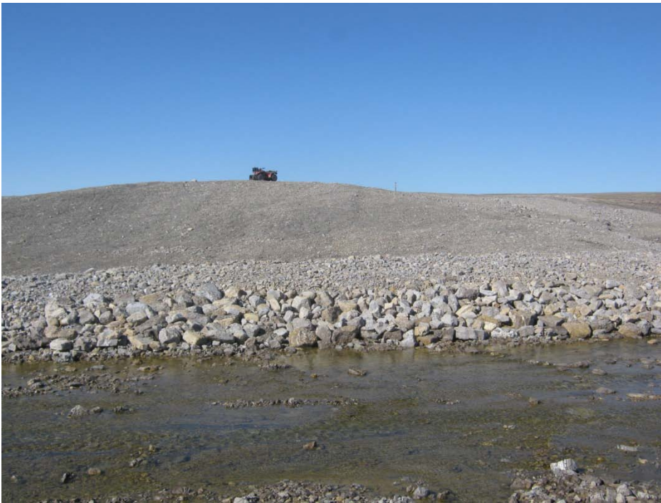
Photo 31, Garrow Lake Dam, East abutment, Facing West breach slope
