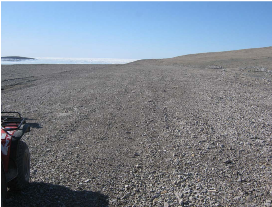
Photo 22, Operational Landfill, Back of Crest, Facing South
