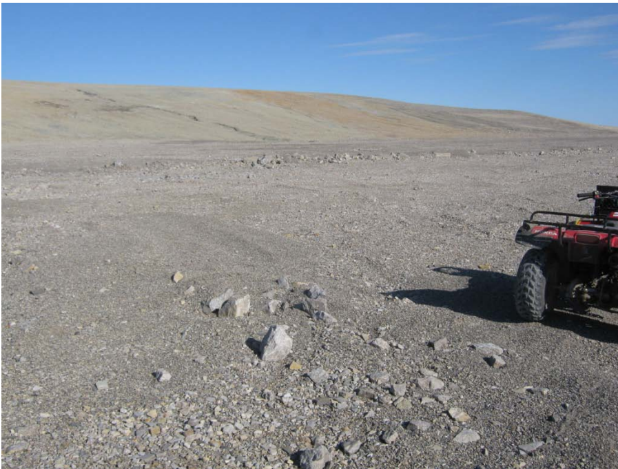
Photo 3, Operational Landfill, Central Crest, Facing Northwest
