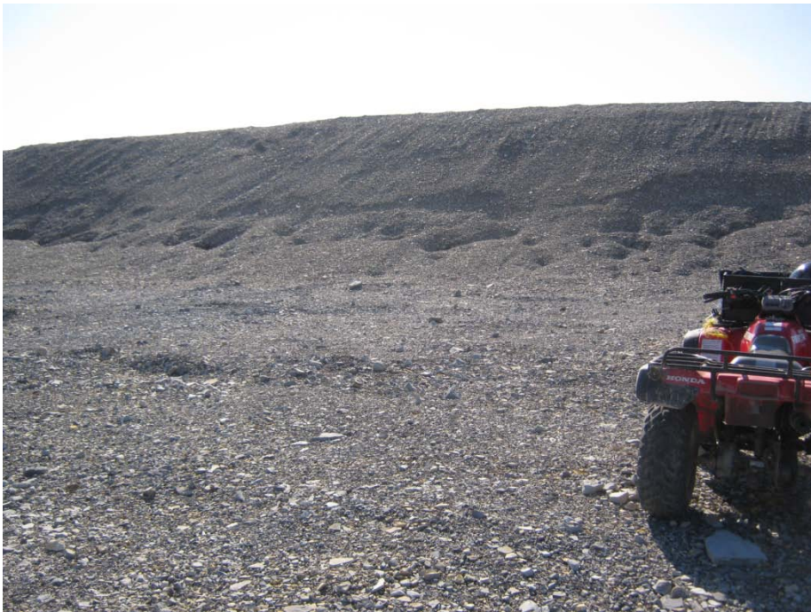
Photo 80, New Quarry, North central perimeter, Minor thaw settlement along slope bottom
