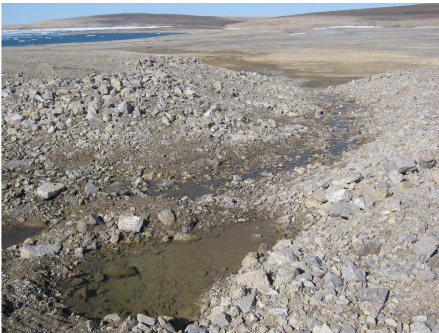
Photo 70, New Quarry, Drainage Ditch at West end, Rip-Rap lined ditch facing downstream (from top)
