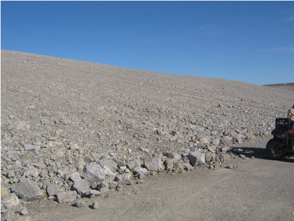
Photo 15, Operational Landfill, South Toe, Facing Northwest
