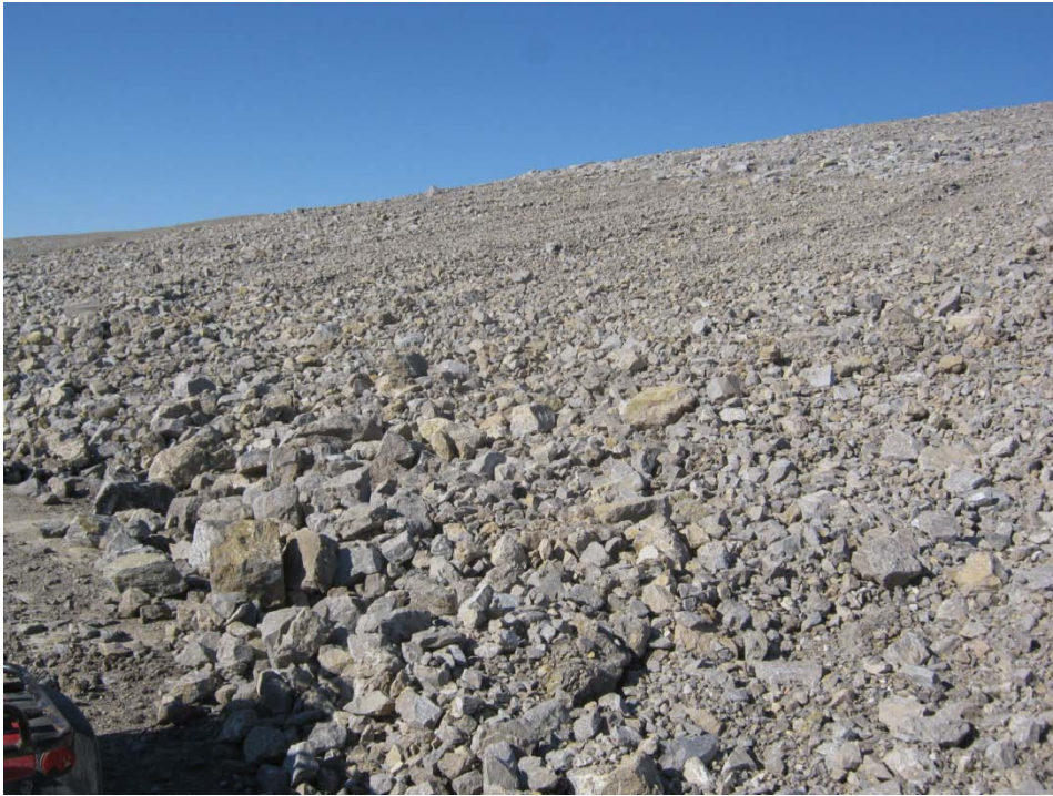
Photo 17, Operational Landfill, South Toe, Facing Southwest (undulations ~0.5m)
