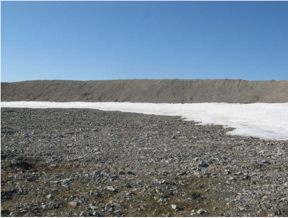
Photo 79, New Quarry, Northeast end, Typical self-amouring erosion gully, Facing Northeast
