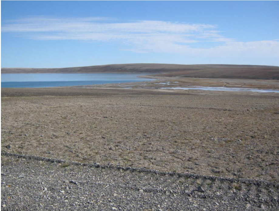
Photo 25 , Garrow Lake, View of wave break structure from access road above
