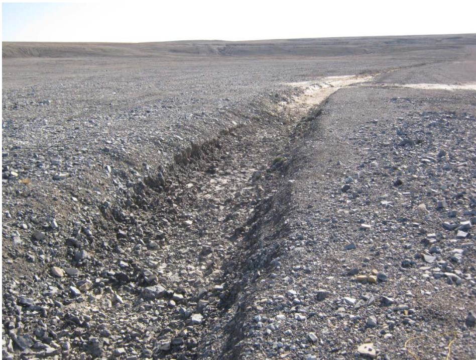
Photo 84, New Quarry, Central drainage ditch, Facing West
