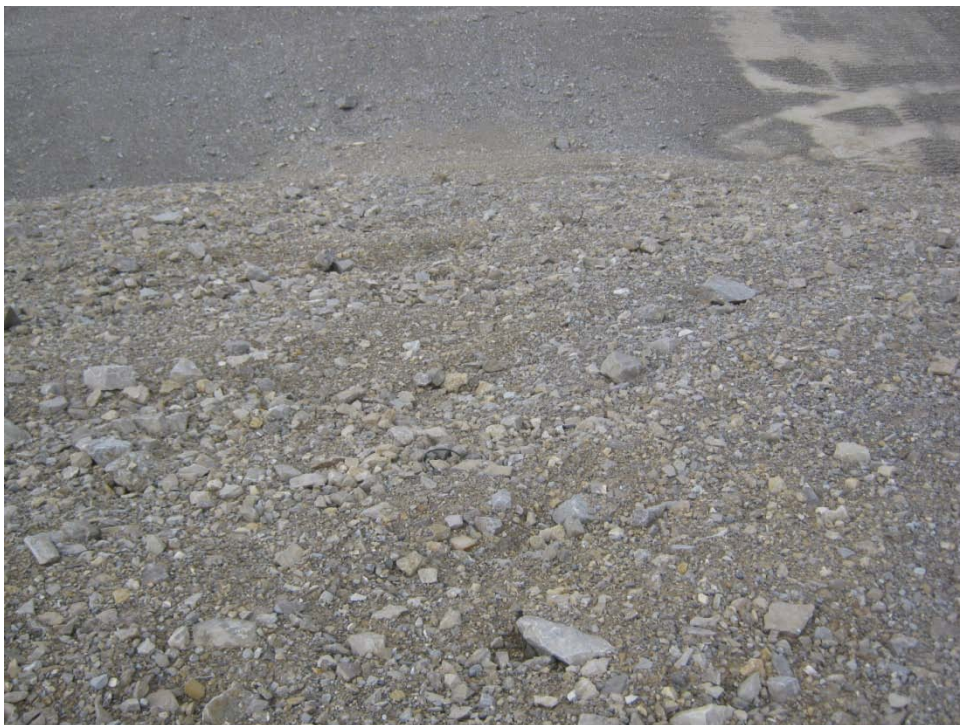
Photo 110, Mine Portals, Conveyor Portal, View from top of backfilled slope
