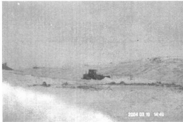
March 19, 2004 Excavating Dam
