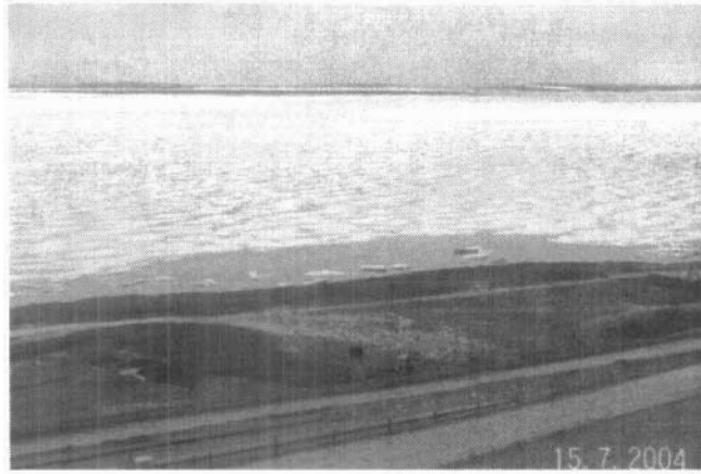
July 15, 2004 – Decommissioning of Dock Completed
