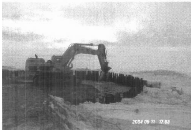
May 11, 2004 – Digging Fill From Inside Dock Sheet Piles
