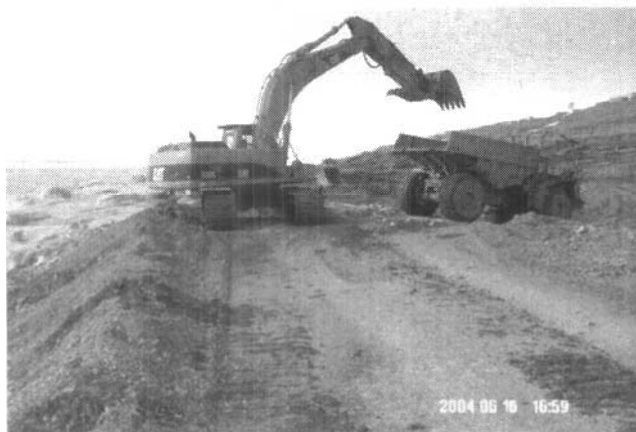
June 16, 2004 – Further South Along Shoreline, Berm Being Removed
