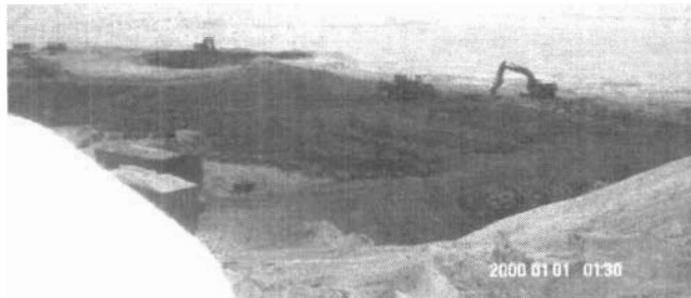
April 27, 2004 – Re-grading Area Shown Previously
