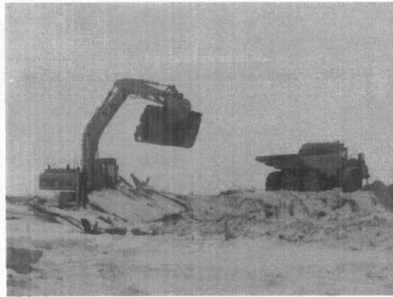
May 26, 2004 Loading Sheet Piles to be Hauled to LRD Quarry landfill
