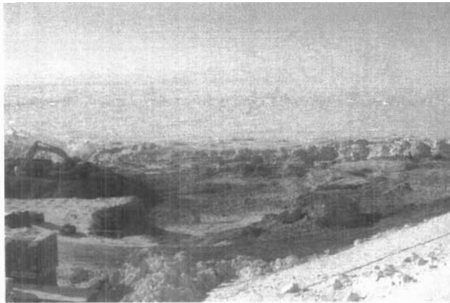
Apr 11, 2005 – Excavated Shoreline North of Previous Picture
