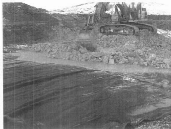
April ? – Placing Rip-Rap Onto Geotextile
