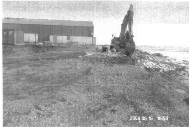
June 16, 2004 – Excavating Shoreline South Towards Foldaway Buildings
