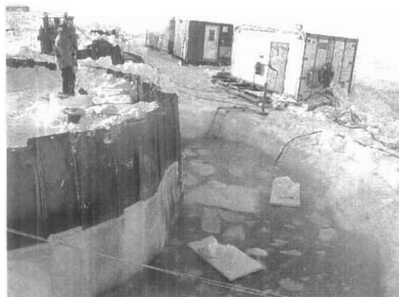
April 8, 2004 – Divers Cutting Sheet Piles
