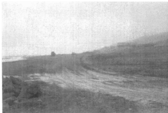
July 11, 2004 – Work Continuing on Contouring Area Above Beach
