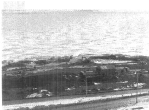
June 2, 2004 – Excavation of Dock Continuing
