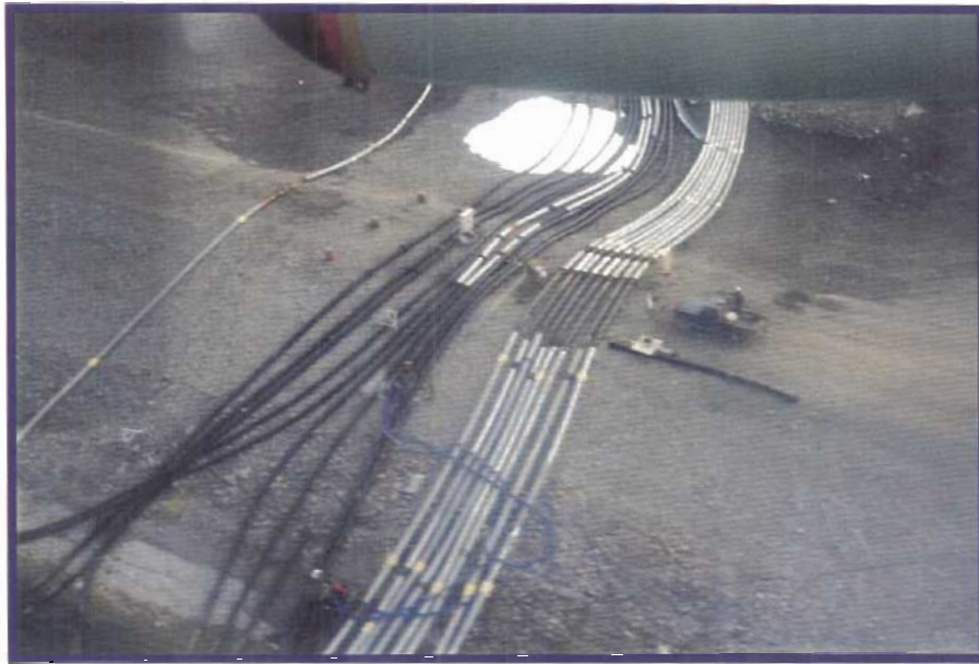
Photo 13 Aerial view of siphon pipes over Garrow Lake Dam.
