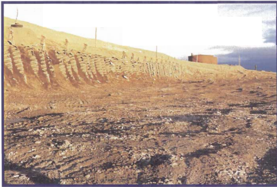
Photo 27 Partially excavated bin wall retaining wall along east side of concentrate storage shed.
