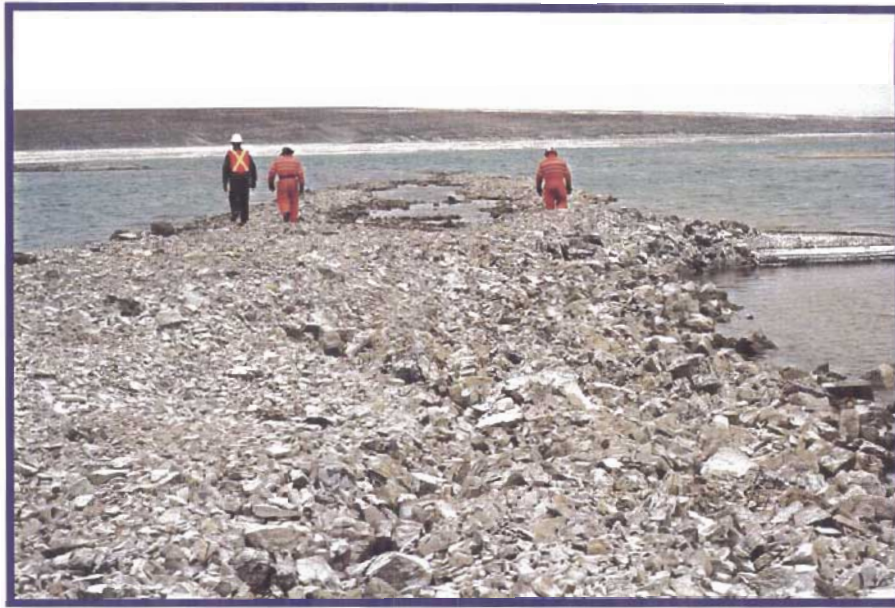
Photo 21 Top of Garrow Lake wave break structure. Open water portion is approximately 0.4 m deep and is located in vicinity of original lake outlet to Garrow Creek.
