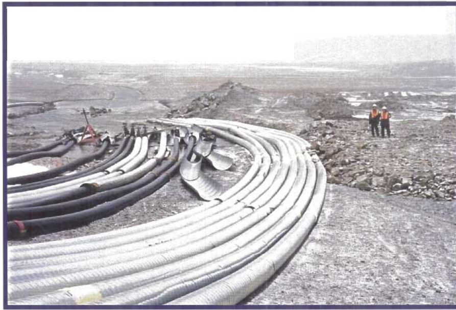
Photo 15 Discharge end of siphon pipes at downstream toe of Garrow Lake Dam. Garrow Creek flows in natural channel in background.
