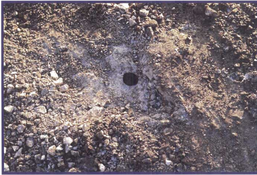
Photo 31 Close up of limestone bedrock exposed in floor of concentrate storage shed. Some 10-15 cm of rock has been removed by contractor to collect residual metals contaminated soils.
