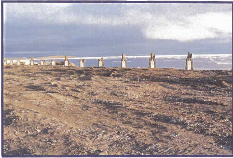
Photo 29 Lower ends of steel columns which supported the concentrate storage shed. Soil in floor of shed has been excavated to bedrock.
