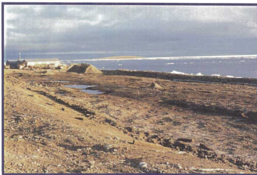
Photo 51 Foreshore area in front of concentrate storage shed. Ongoing removal of contaminated soils. Note berm along shoreline.
