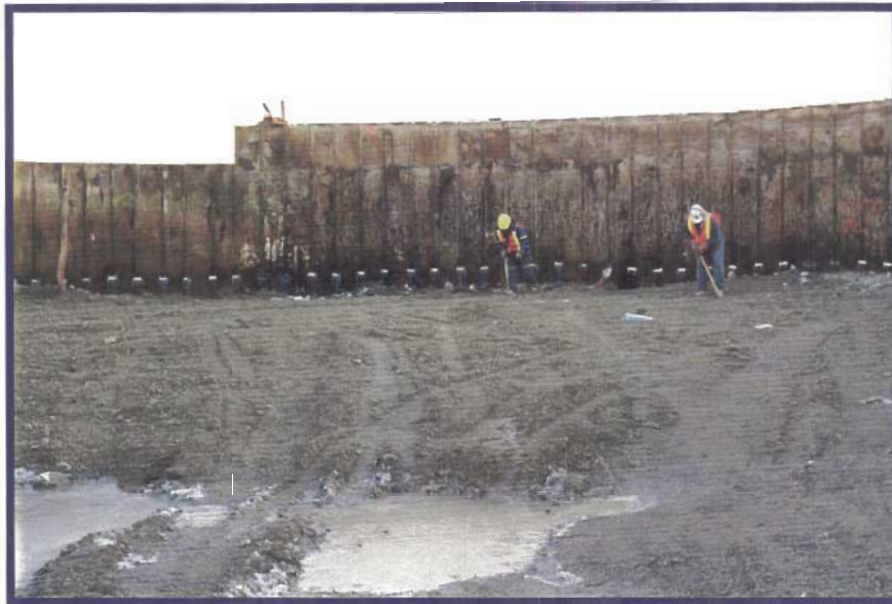
Photo 49 Workers inside dock cells exposing glycol freeze pipes by hand shovelling.
