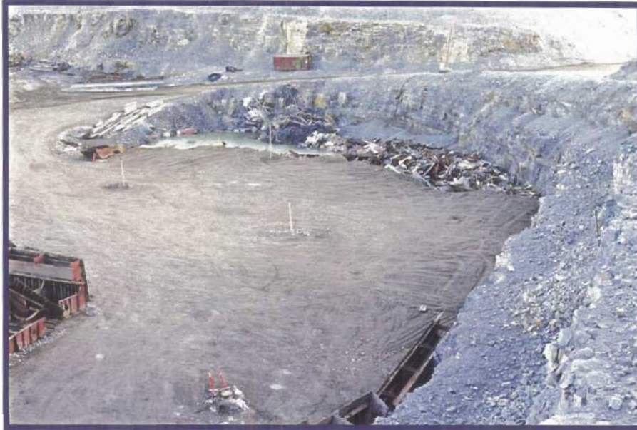
Photo 43 LRD Quarry, thermistor pipes and backfill cover, with new lift of demolition debris.
