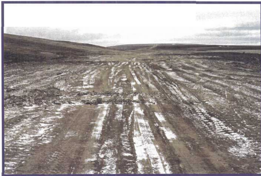
Photo 39 Top of Operational Landfill/contact zone with backslope where backfill was placed level with top of shale cover.
