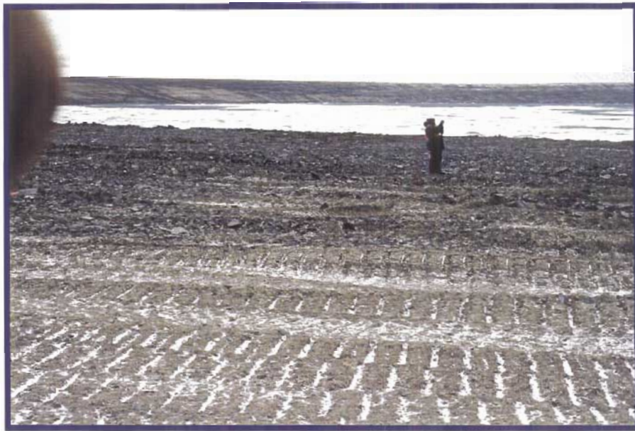
Photo 37 Surface of 1.2 m of shale cover on top of Operational Landfill.
