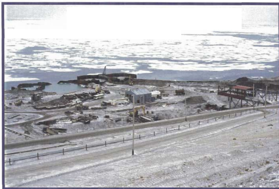
Photo 47 View of dock cell area after night of high (120 km/hr) winds. Note flooded cells with more damage to sheet piles.
