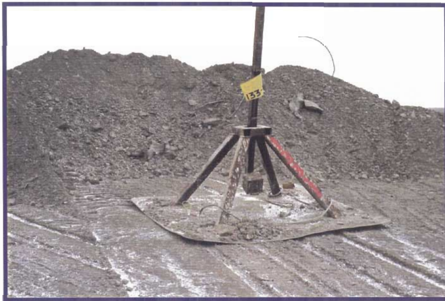
Photo 66 Protective cover over raise borehole used to drop contaminated soil into underground storage area.
