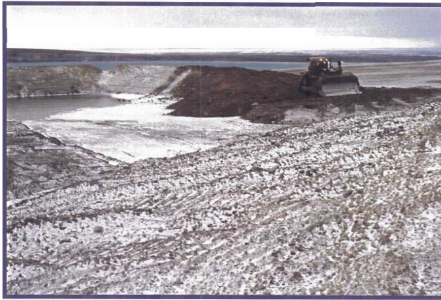
Photo 59 Tailings thickener - overflow pond dikes in process of removal.
