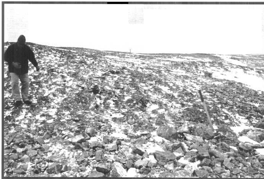
Photo 24 View along upstream face of right bank of Garrow Lake Dam. Some of the material on the slope contains entrained ice and snow and will have to be removed over the next few years as it melts and drains out .
