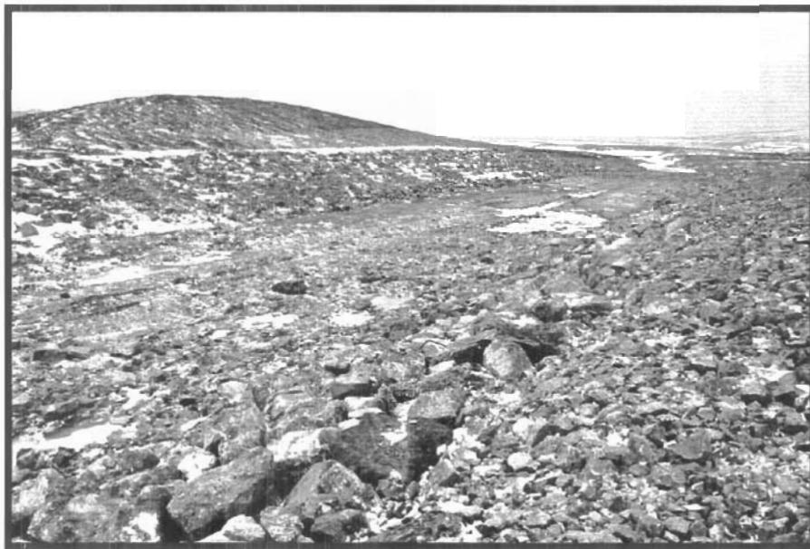
Photo 22 View looking downstream along re-established channel through Garrow Lake Dam. Note coarse rip rap lining channel. A finer grade of rip rap was added above the channel rip rap to protect the lower exposed cuts through the dam embankment against erosion.
