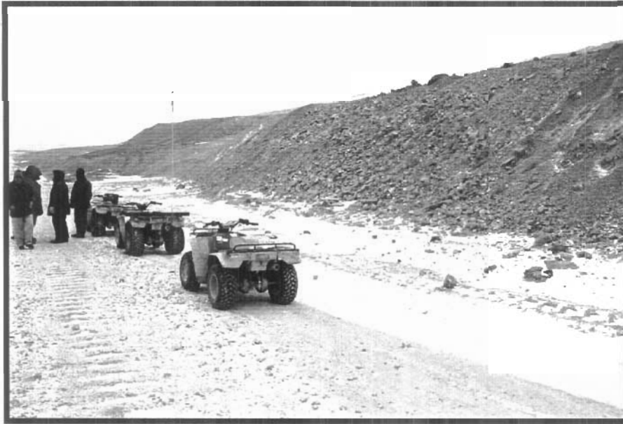
Photo 16 Slope of fill material below site of incinerator. This slope needs to be flattened.
