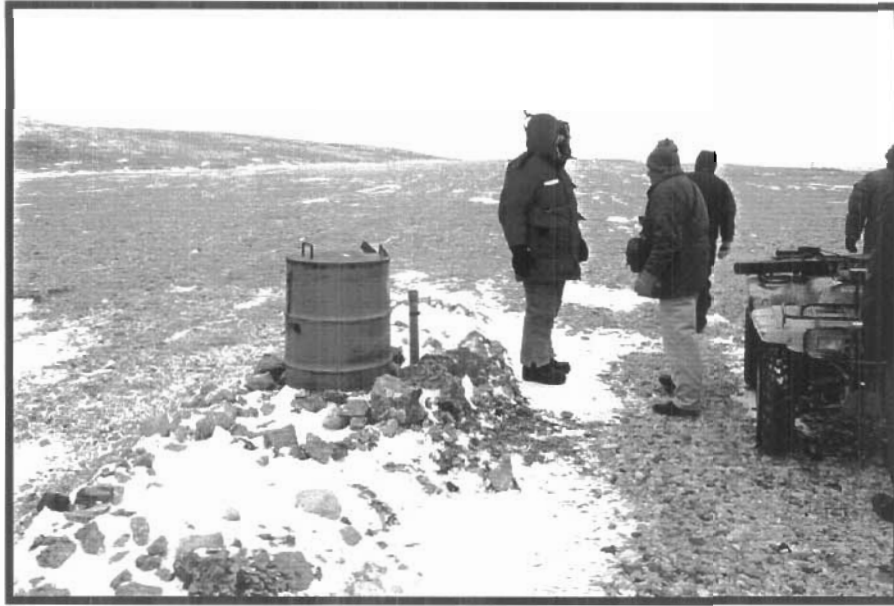
Photo 14 Operational Landfill- cover with thermistor installation.
