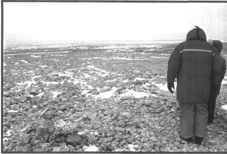
Photo 2 Rip rap cover placed on exposed erodible soils downstream of dam on right bank.
