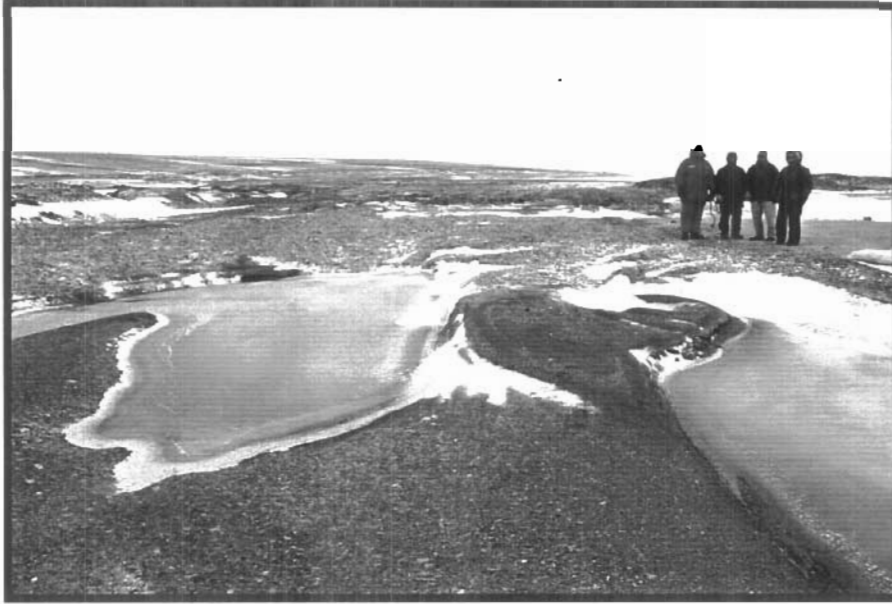
Photo 10 Looking upstream along channel excavated through wave break structure. Teck Cominco added some fill into the breach to bring water level in Garrow Lake back up to former natural level.
