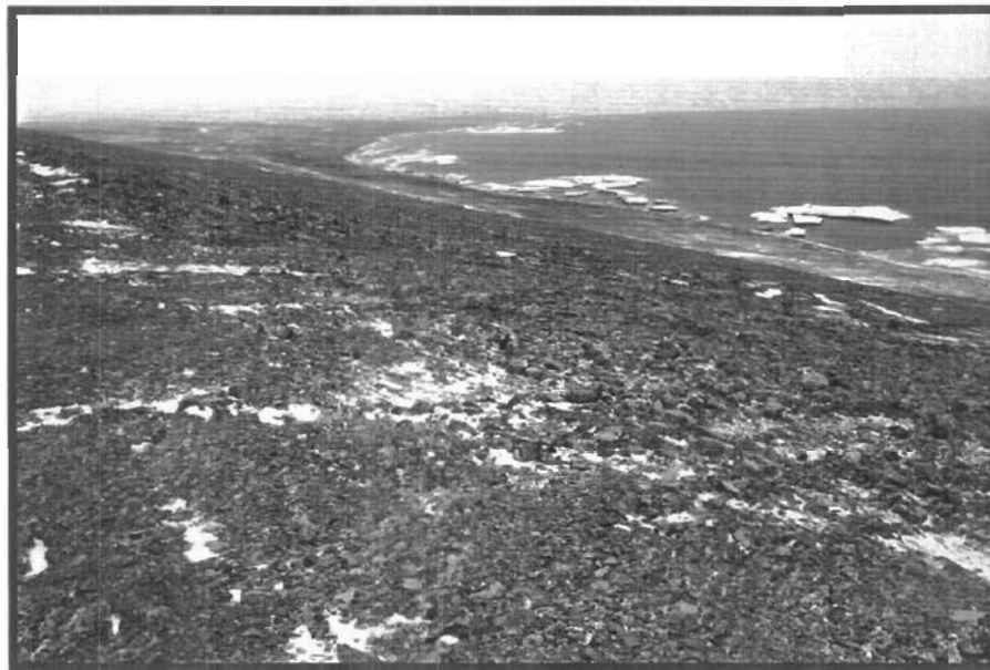
Photo 15 South slope of Operational Landfill. A 30 cm layer of finer grained cover material was placed to repair the cracks and settled areas noted in this area in the previous visit.
