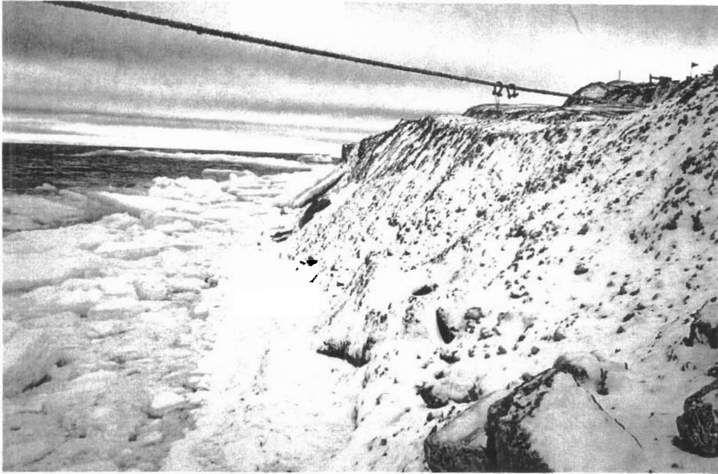
Photograph No. 10: View of shoreline looking north at Station 1500 N. The shoreline to the north of 1500 N is fill comprised of material with about 300 mm minus material. (August 19, 2000).
