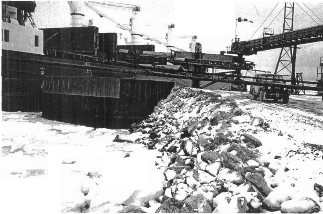
Photograph No. 12: View of shoreline looking north at Station 1300 N. New riprap has been placed in this area in the last 2 years. (August 19, 2000).
