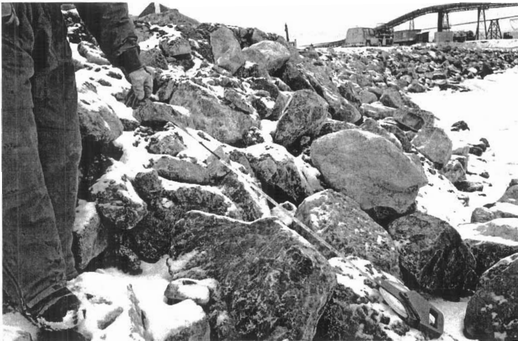
Photograph No. 11: View of shoreline looking south at Station 1500 N. The shoreline is covered with rip rap to the south of Station 1500 N, with a mean size of about 300 mm (August 19, 2000).
