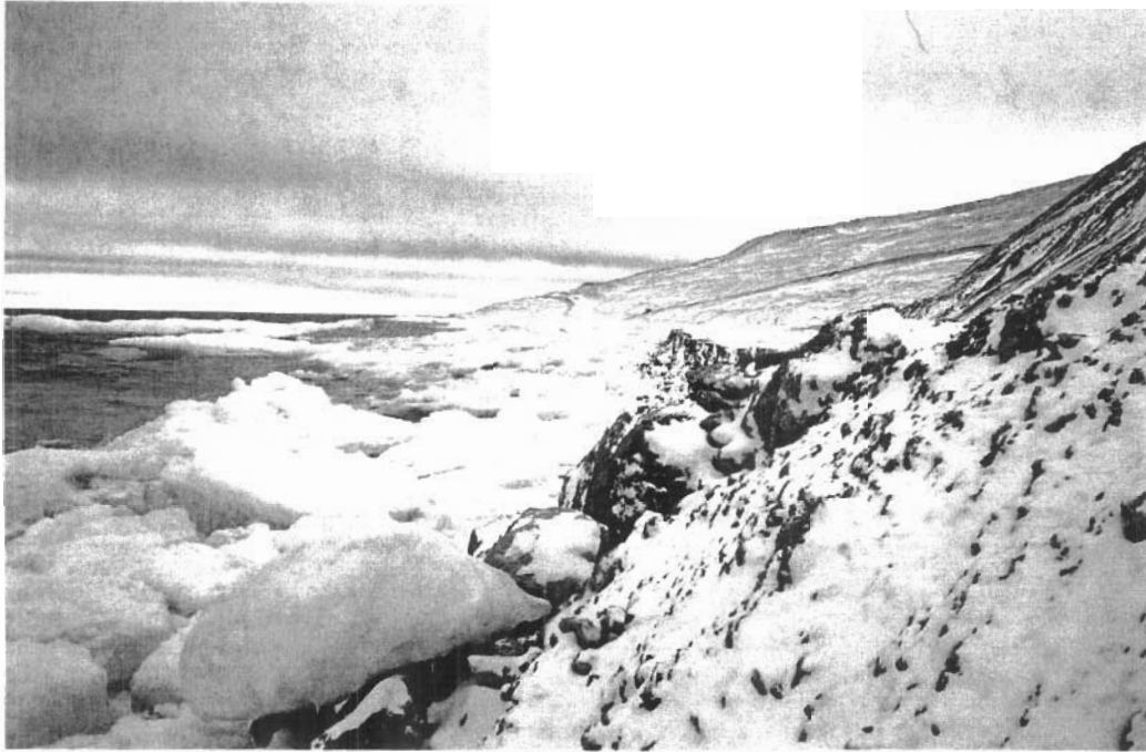
Photograph No. 8: View of shoreline looking north at Station 1600 N. The fill is about a 300 mm minus material, with a mean size of 25 mm. (August 19, 2000).
