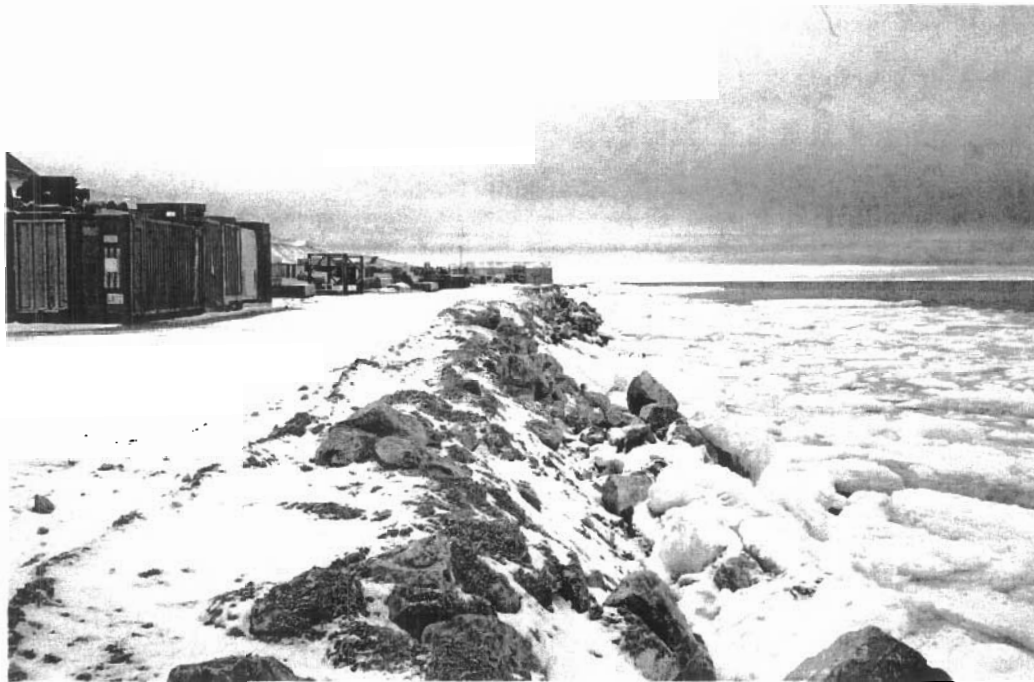
Photograph No. 15: View of shoreline looking south at Station 1200 N. It has been more than two years since riprap has been placed south of Station 1200 N. (August 19, 2000).
