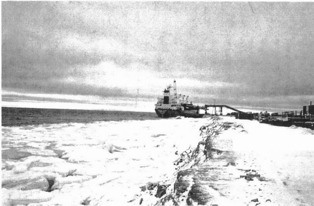
Photograph No. 18: View of shoreline looking north at Station 1000 N. Most of the riprap has slipped down the slope at this location. (August 19, 2000).
