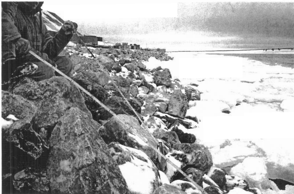
Photograph No. 13: View of shoreline looking south at Station 1300 N. This area has the largest size rock produced from the Little Red Dog Quarry and used as riprap, with a mean size in the range of about 400 mm to 500 mm. (August 19, 2000).
