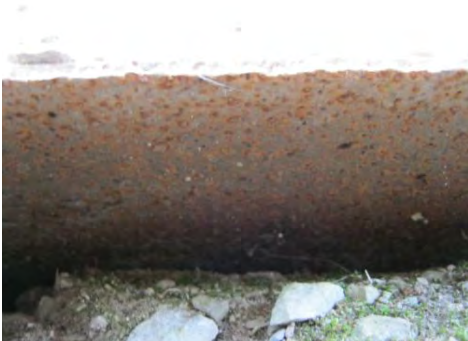
Photo 1723: View under tank bottom plate, minimal corrosion noted <0.020'' .
