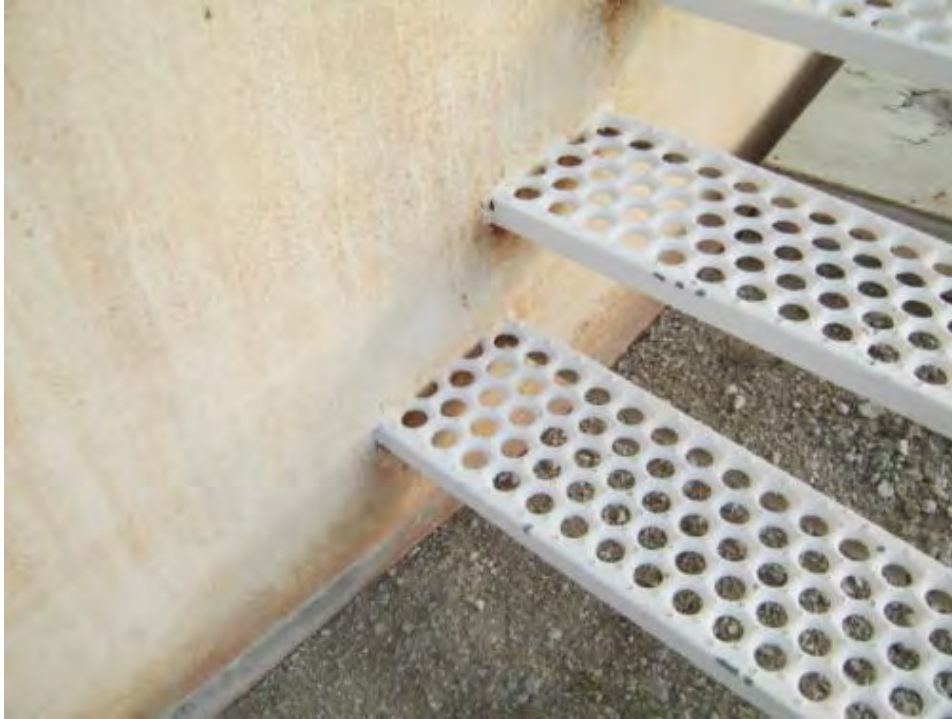
Photo 1729: Stairway attachments to tank.
