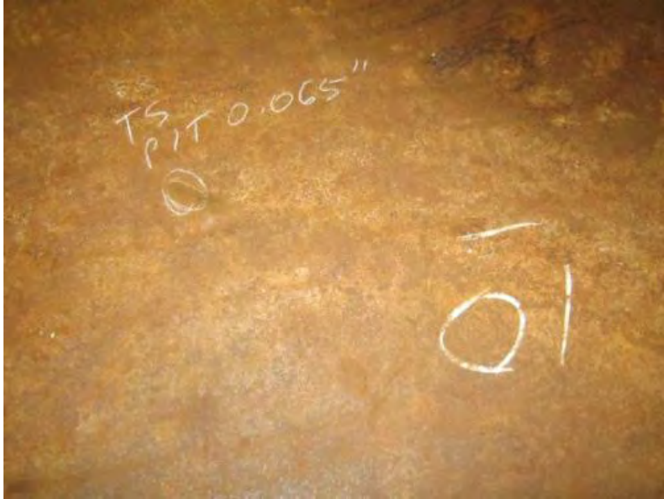
Photo 1757: Random/isolated deeper pit 0.065".
