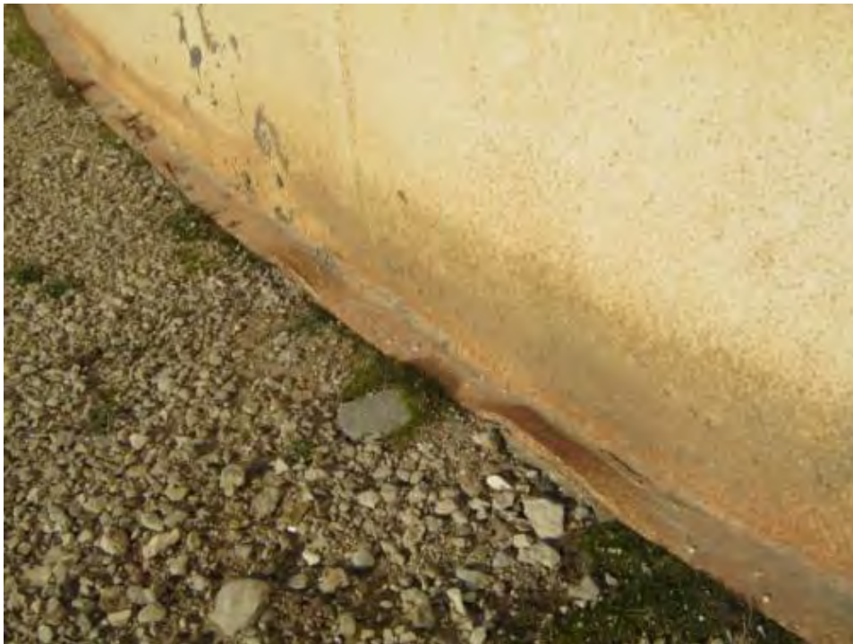
Photo 1728: Deformations at bottom plate projection at random.
