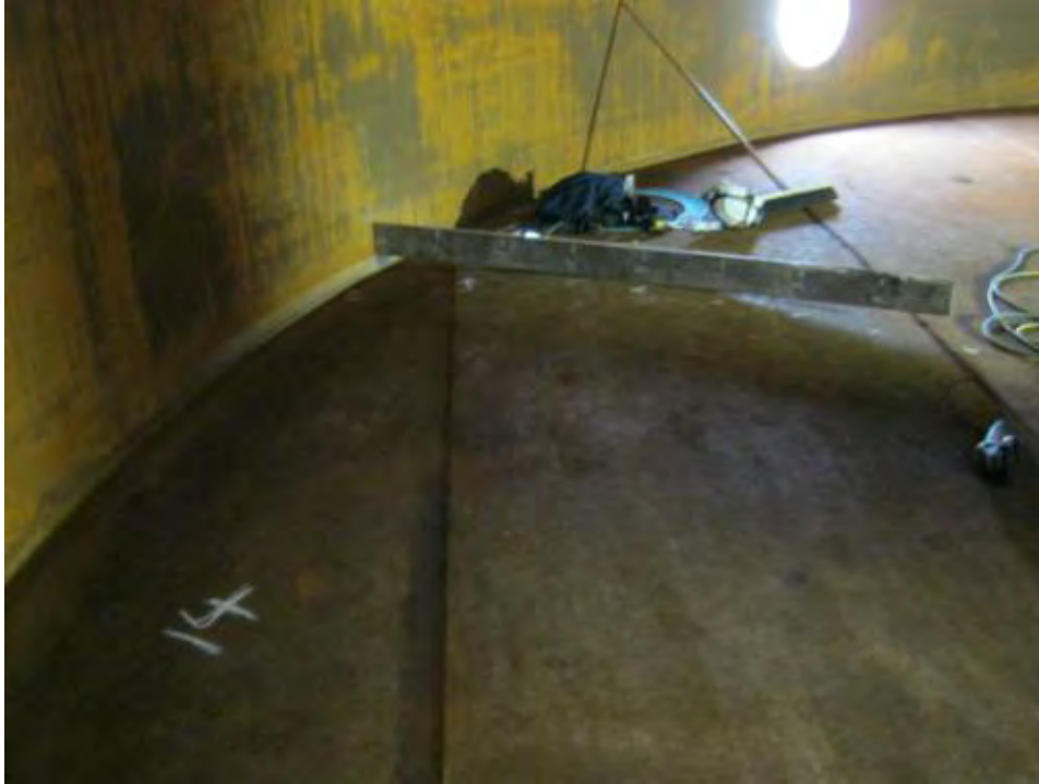
Photo 1775: Bottom/floor plate settlement distortion plate 13 and 14 area.
