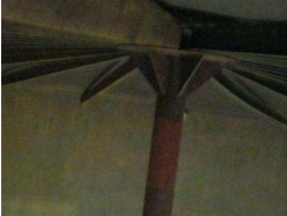
Photo 1801: View of rafters on column top plate, note roof plate not laying flat on rafters.
