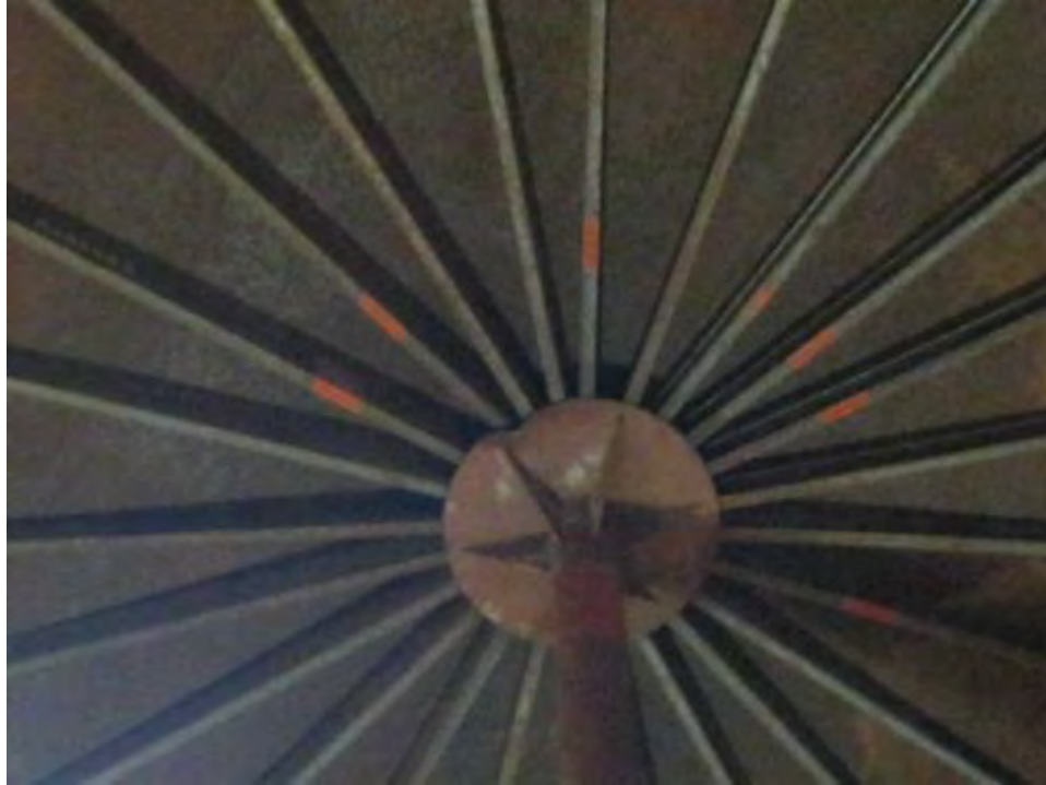
Photo 1745: Bent area at edge on column centre plate.
