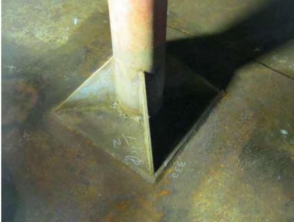
Photo 1752: Column base welded to floor, no significant settlement/heave issue noted.
