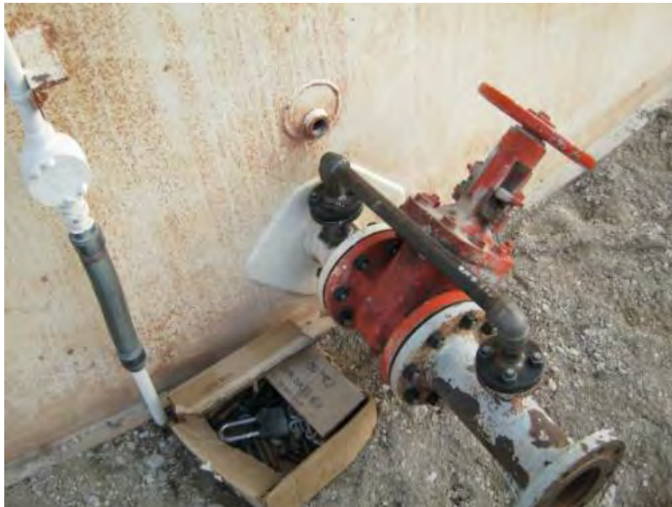
Photo 1738: Fill/discharge line nozzle, non-standard shell insert above, later cleaned and MT tested.
