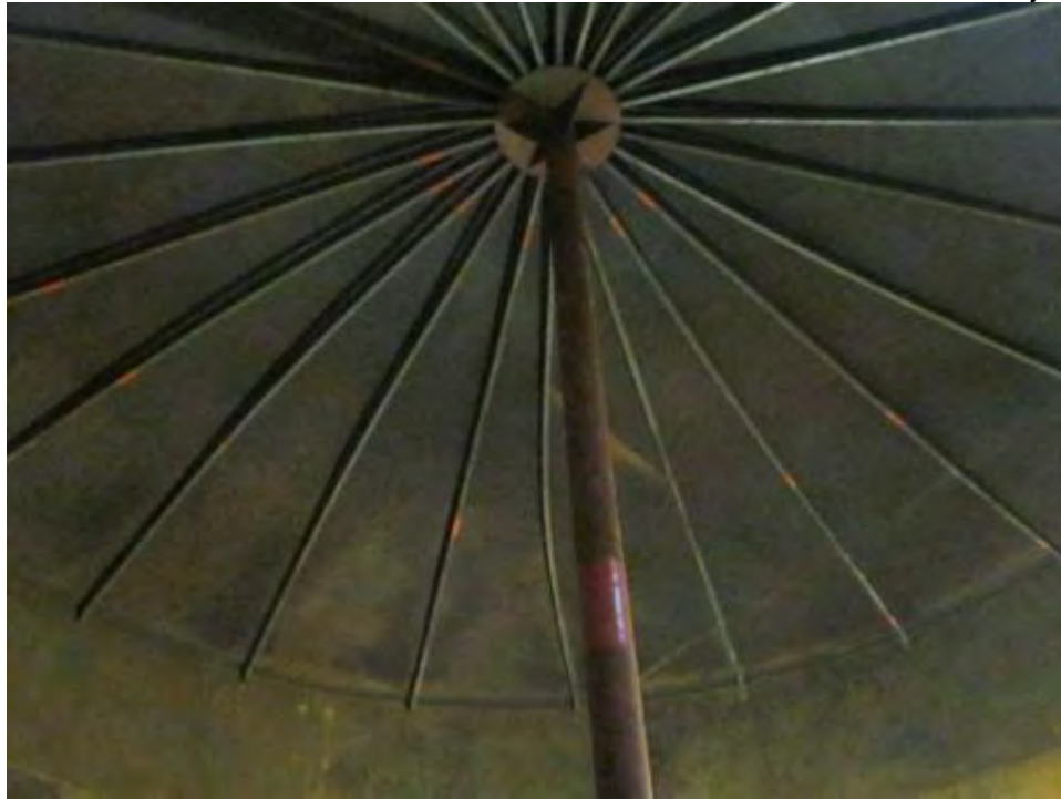
Photo 1810: View of roof rafter deformations, estimated up to 6".
