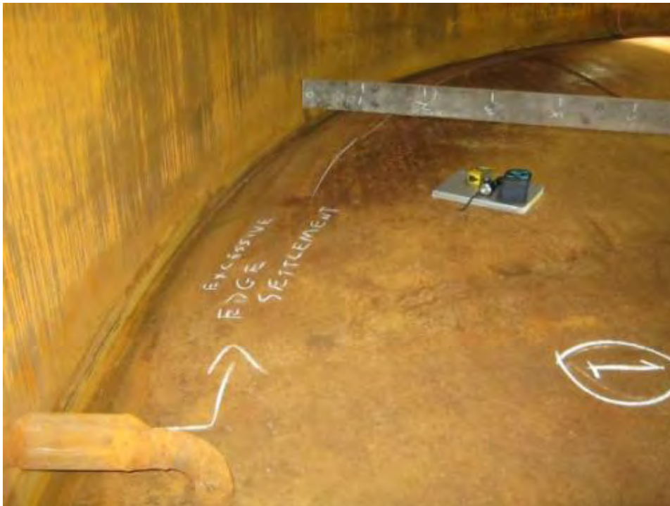
Photo 1751: Edge settlement plate 1 areas, 4'-5' first 3' from shell.
