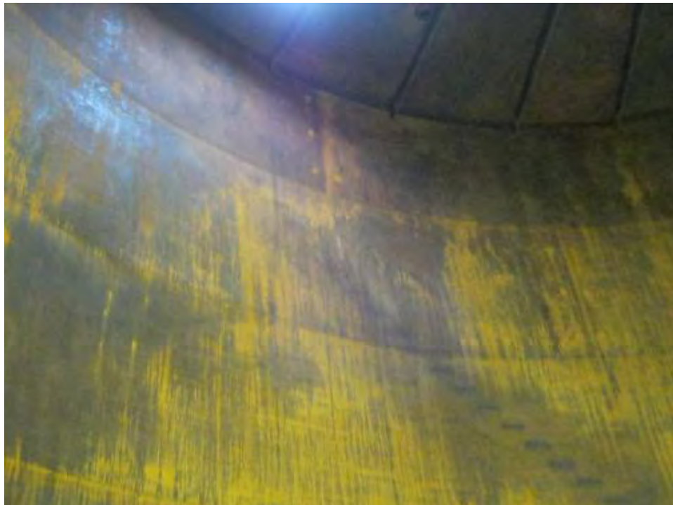
Photo 1746: Upper shell to roof, no significant corrosion noted.
