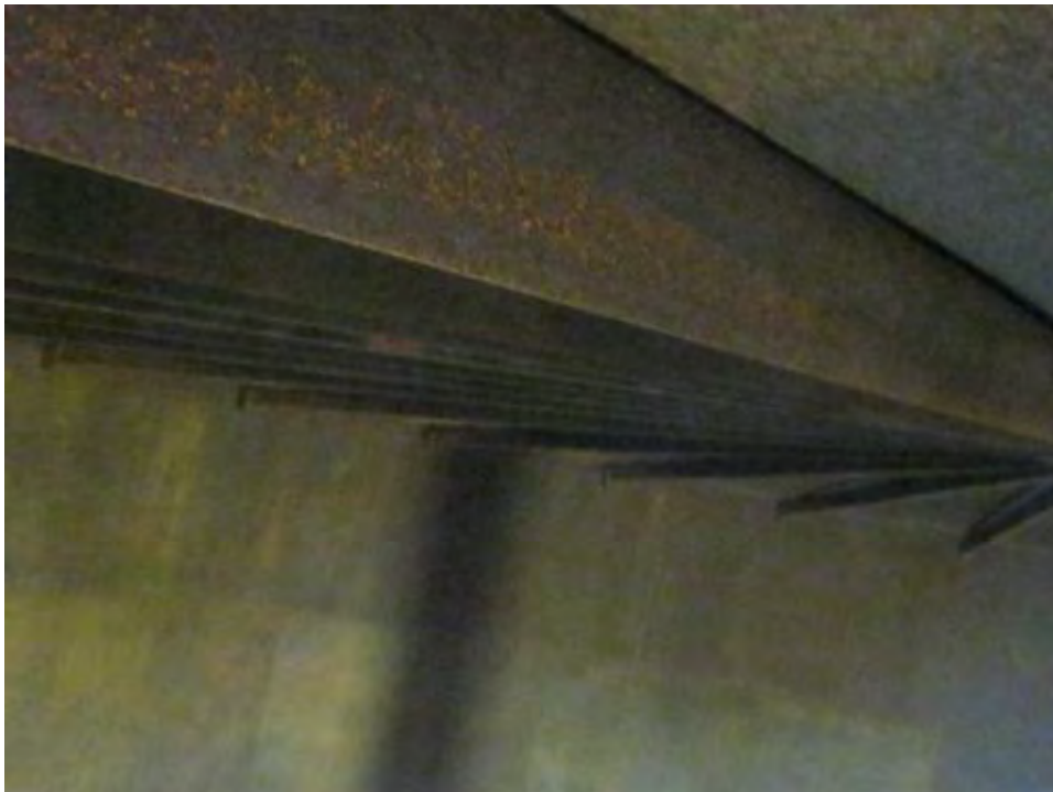
Photo 1799: Rafter close-up, no significant corrosion.
