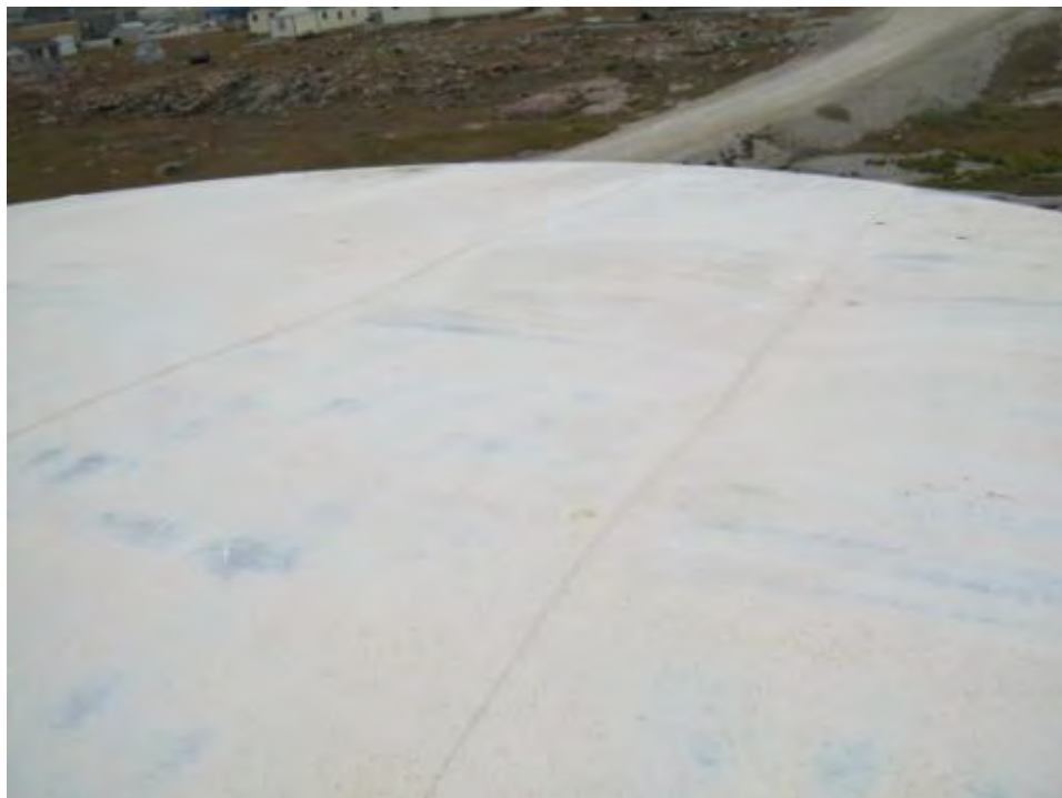
Photo 1781: Roof plate undulating not flat on rafters as noted in photo 1801.
