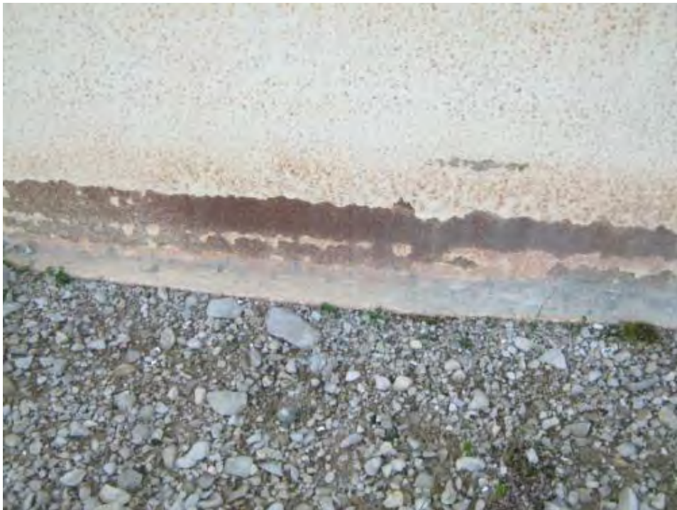
Photo 1719: Close-up of shell to bottom plate projection, coating peeling and light corrosion.
