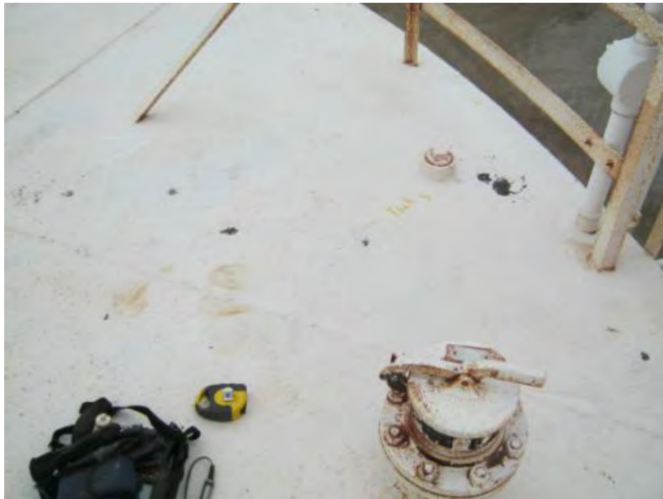
Photo 1788: Sample hatch nozzle.
