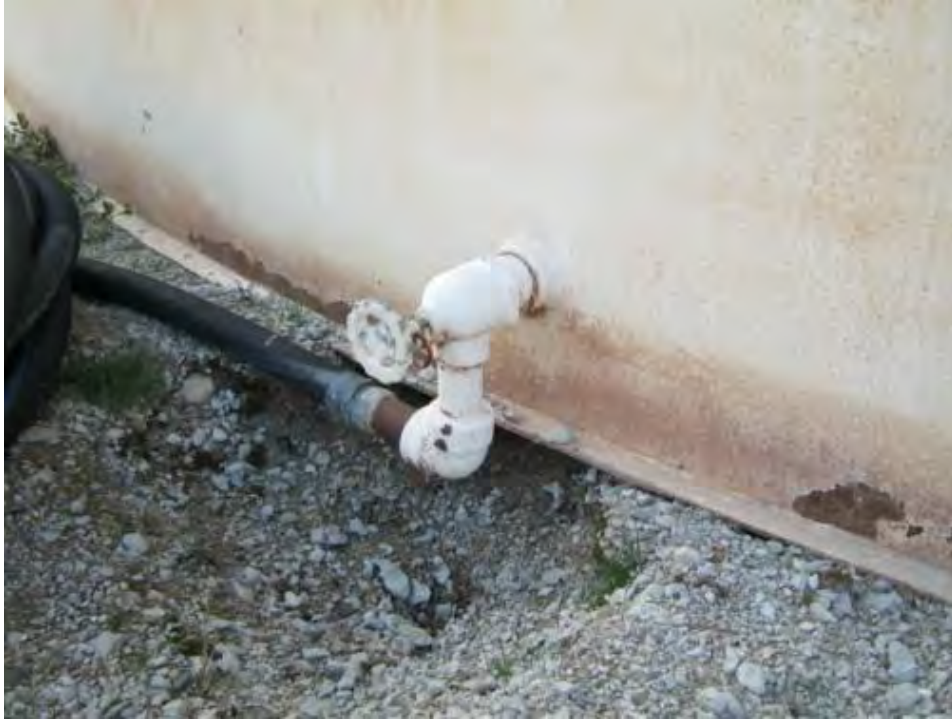
Photo 1720: Drain nozzle area excavated for draining tank
