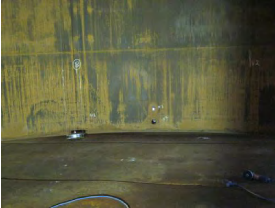
Photo 1774: Shell interior in good general condition, some minor shell denting/distortion at lower 1 foot from moving operations in the past.
