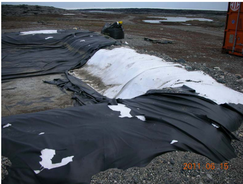
PICTURE 1: Lagoon with Torn and Missing Sections of Liner
