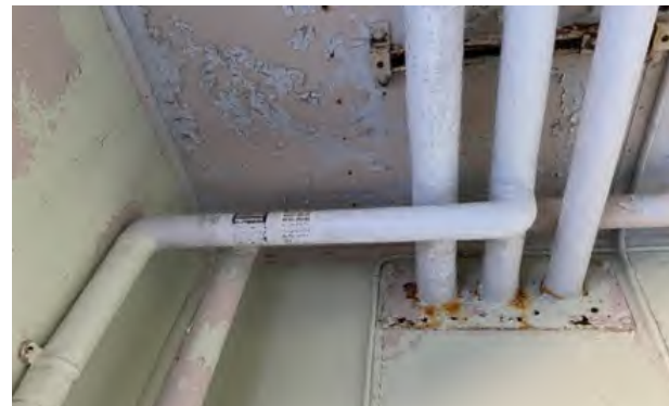
PCB painted walls and asbestos wrapped pipes.
