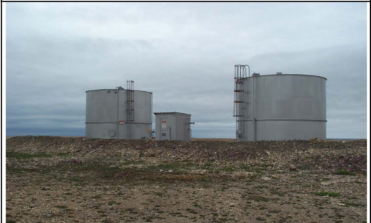
Photo 4: Station POL and pumphouse
