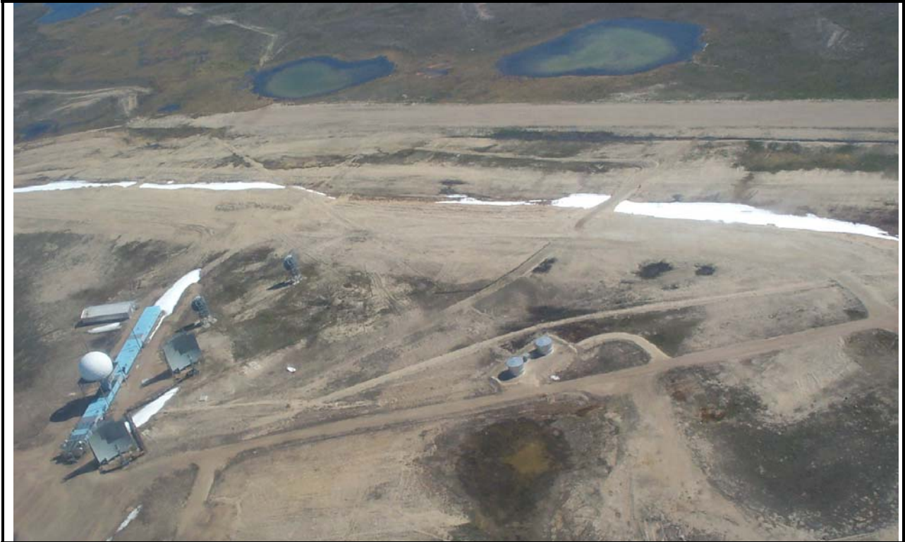
Photo 1: Station area – aerial
