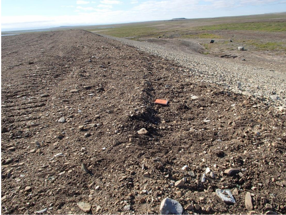
Photograph 75. Tier II Disposal Facility – low spot and ridge from construction activities on landfill. Picture P8130027 ↑
