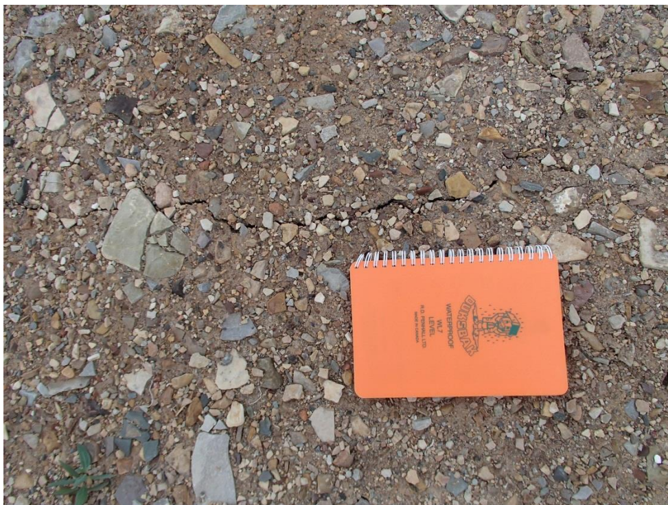
Photograph 87. Airstrip Landfill Lobe B – tension crack on east side of landfill. Picture P8150209 ↑
