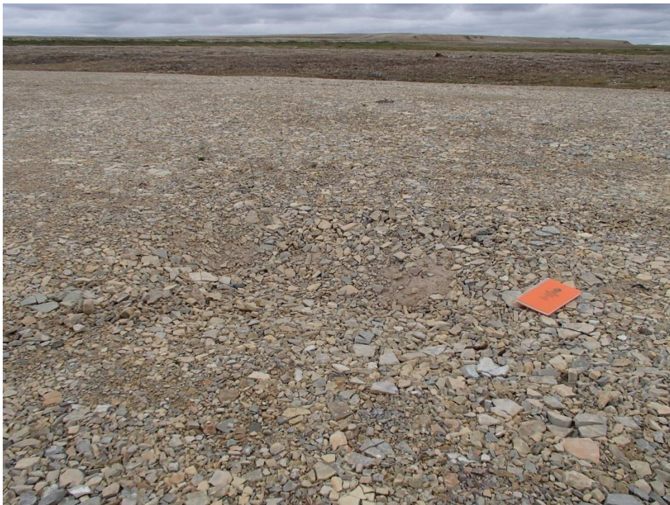
Photograph 86. Airstrip Landfill Lobe B – low spot from construction activities on landfill. Picture P8150222 ↑
