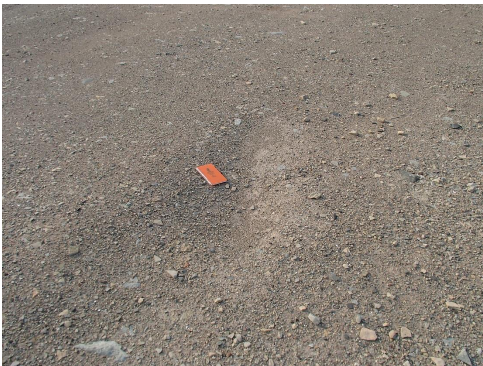
Photograph 43. Station Area Landfill Lobe A – low spot (approx. 75 mm deep) on landfill. Picture P8140163 ↑
