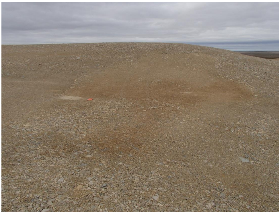
Photograph 25. North Landfill Lobe C – area of fine material on top of landfill. Picture P8150372 ↑
