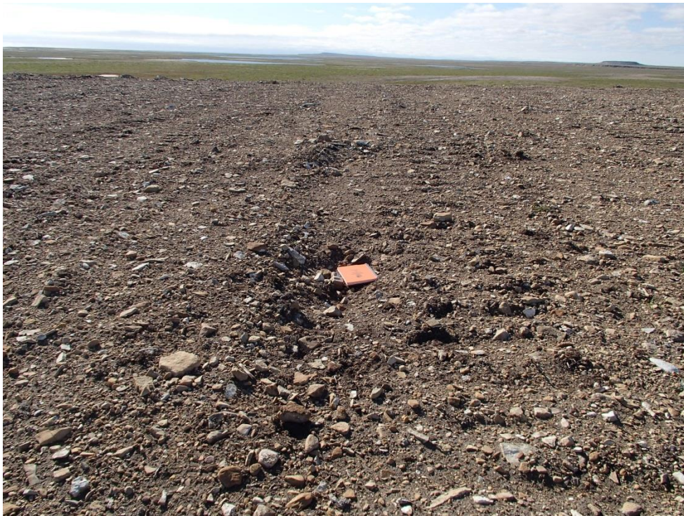
Photograph 74. Tier II Disposal Facility – low spot from construction activities on landfill. Picture P8130026 ↑
