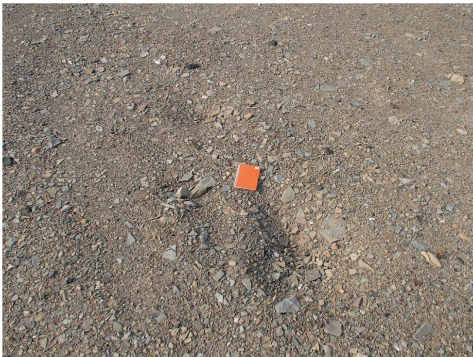
Photograph 44. Station Area Landfill Lobe A – isolated low spot (75 mm to 200 mm deep) on top of landfill. Picture P8140145 ↑
