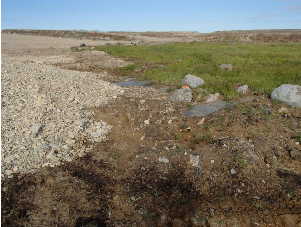
Photograph 73. Tier II Disposal Facility – wet area of ponding water near southeast corner of landfill. Picture P8130038 ↑
