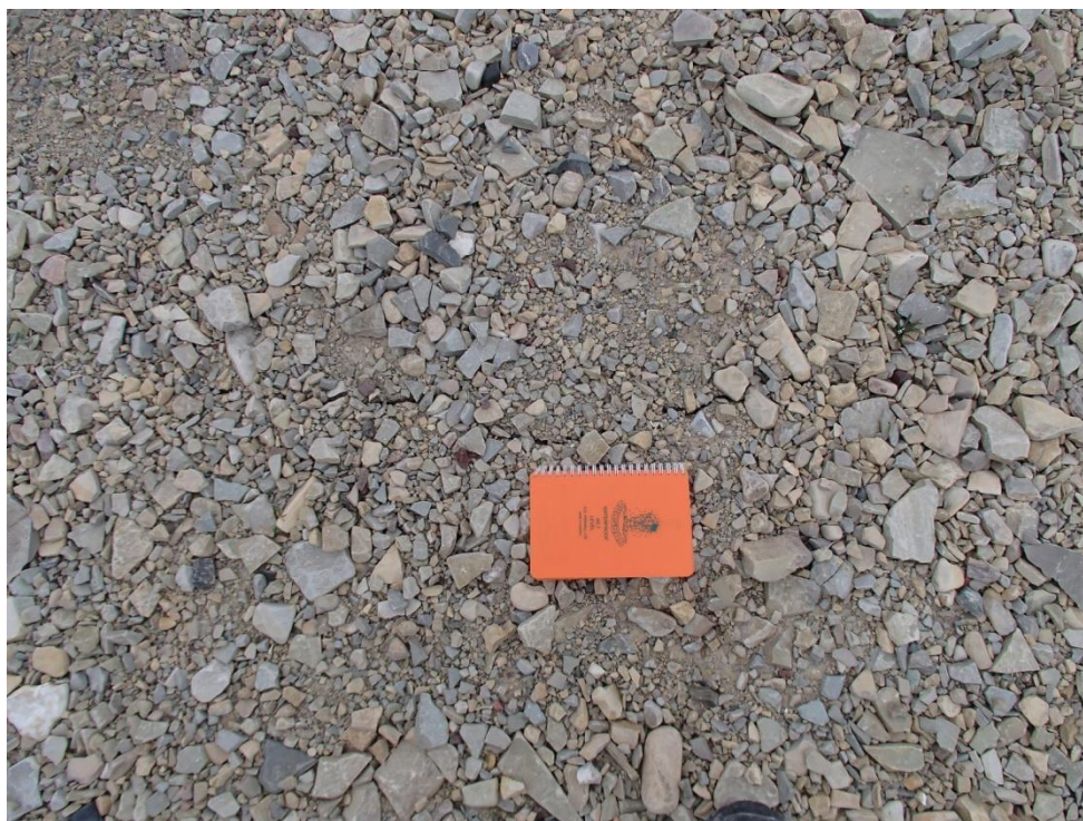
Photograph 8. Northwest Landfill Lobe D – small tension crack on top of landfill. Picture P8150288 ↑
