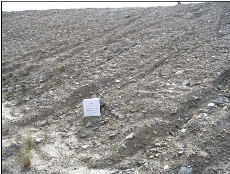
Photo MLFN-7A, Easting: 495874, Northing: 7667561, Direction: 110° Main Landfill North; looking across erosion gullies on slope Scale: photo placard dimensions are 29.4 cm wide by 27.5 cm in height
