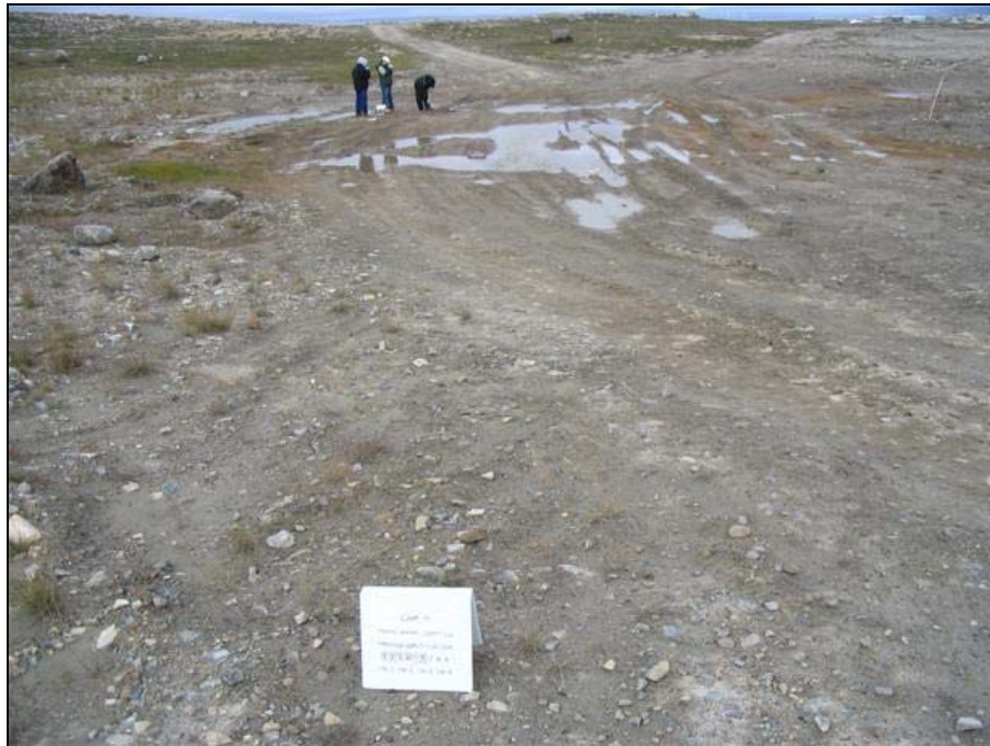
Photo SSLF-5C, Easting: 496386, Northing: 7666035, Direction: 340° South Shore Landfill; east central slope facing ponded water and seepage Scale: photo placard dimensions are 29.4 cm wide by 27.5 cm in height
