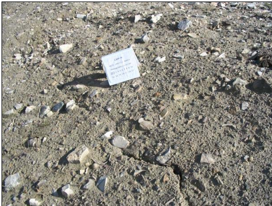
Photo MLFN-2D, Easting: 495755, Northing: 7667517, Direction: 45° Main Landfill North; close-up of crack Scale: photo placard dimensions are 29.4 cm wide by 27.5 cm in height
