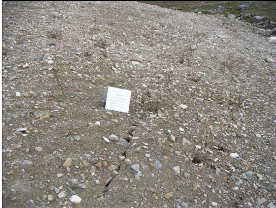
Photo SDA-3A, Easting: 494417, Northing: 7669235, Direction: 45° D.C.C. Tier II Soil Disposal Area; 40 m long crack, max. width 2.5 cm, max. depth 10 cm Scale: photo placard dimensions are 29.4 cm wide by 27.5 cm in height
