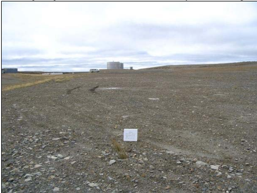
Photo SSLF-2, Easting: 496366, Northing: 7666015, Direction: 225° South Shore Landfill; minor depressions in landfill surface Scale: photo placard dimensions are 29.4 cm wide by 27.5 cm in height
