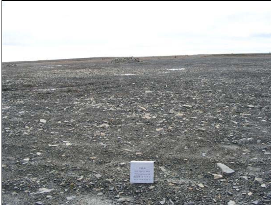
Photo MLFN-4A, Easting: 495814, Northing: 7667617, Direction: 180° Main Landfill North; Some undulations and ponded water at top of landfill Scale: photo placard dimensions are 29.4 cm wide by 27.5 cm in height
