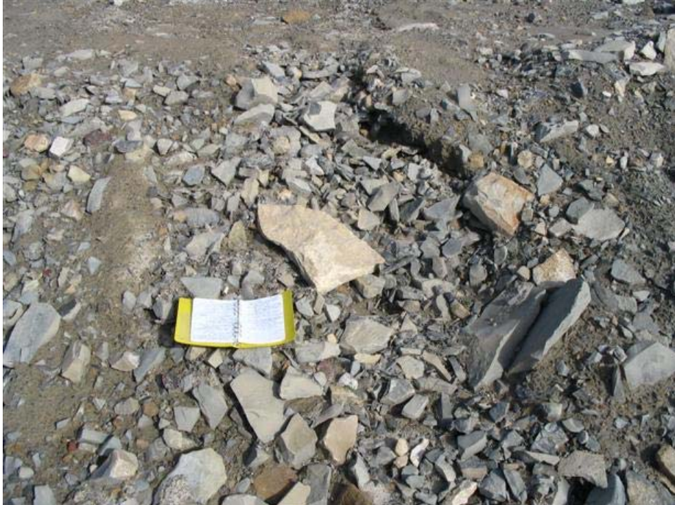
Photo MLFS-7E, Easting: 495751, Northing: 7667267, Direction: 340° Main Landfill South; close-up of erosion Scale: field book dimensions are 29.5 cm wide by 20.0 cm in height
