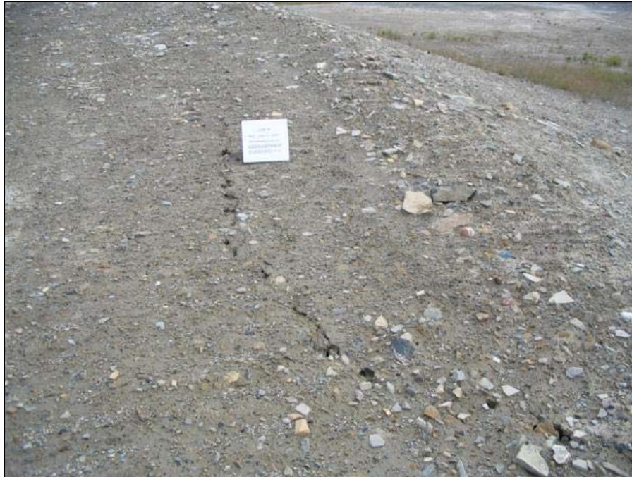
Photo MLFN-15C, Easting: 495927, Northing: 7667478, Direction: 110° Main Landfill North; tension crack along crest Scale: photo placard dimensions are 29.4 cm wide by 27.5 cm in height
