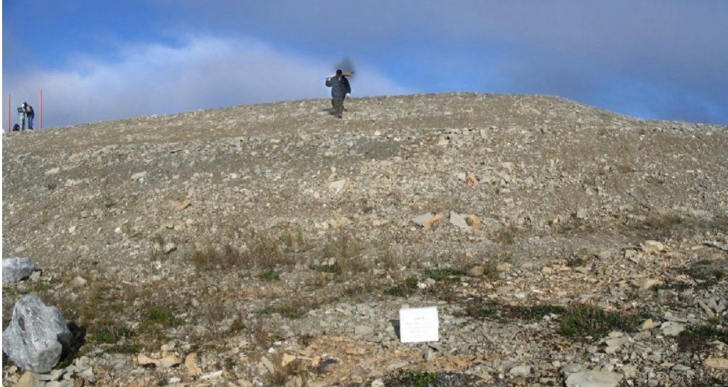
Photo MLFS-3, Easting: 495821, Northing: 7667332, Direction: 300° Main Landfill South; facing slope from toe, some orange stained rock at toe. Scale: photo placard dimensions are 29.4 cm wide by 27.5 cm in height
