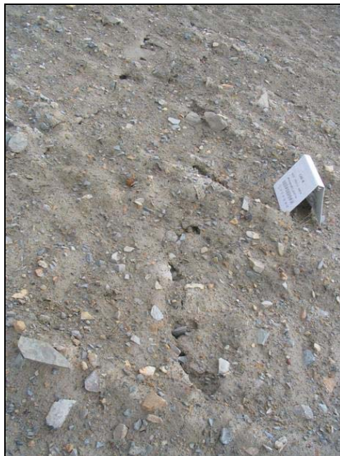
Photo MLFN-11B, Easting: 495916, Northing: 7667534 Main Landfill North; crack max width 0.1 m, max depth 0.1 m Scale: photo placard dimensions are 29.4 cm wide by 27.5 cm in height
