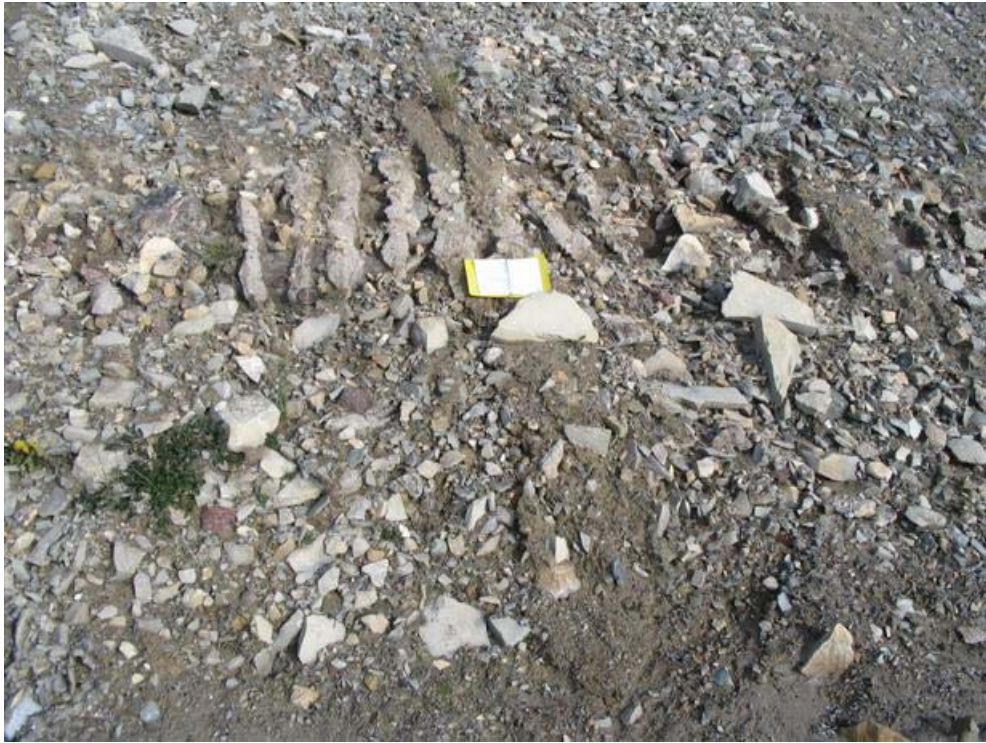
Photo MLFS-10B, Easting: 495657, Northing: 7667274, Direction: 340° Main Landfill South; close-up of erosion Scale: field book dimensions are 29.5 cm wide by 20.0 cm in height
