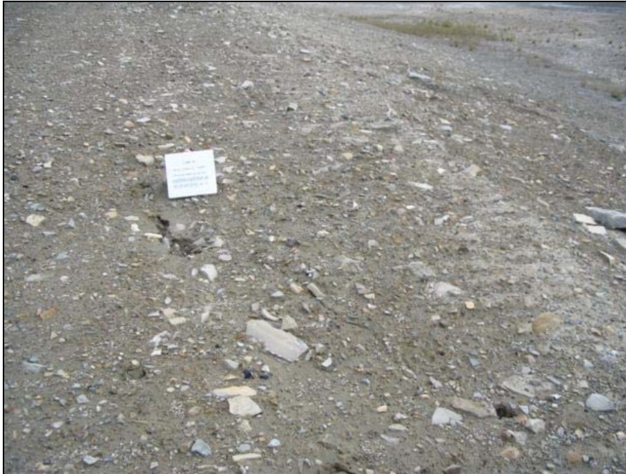
Photo MLFN-15A, Easting: 495927, Northing: 7667478, Direction: 110° Main Landfill North; tension crack along crest, west end Scale: photo placard dimensions are 29.4 cm wide by 27.5 cm in height
