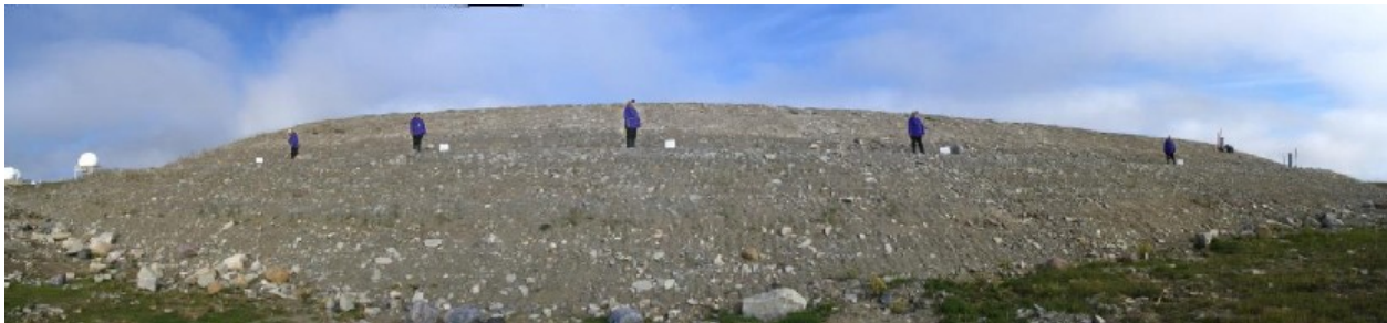
Photo MLFS-10A, Easting: 495657, Northing: 7667274, Direction: 340° Main Landfill South; minor erosion on south slope Scale: photo placard dimensions are 29.4 cm wide by 27.5 cm in height
