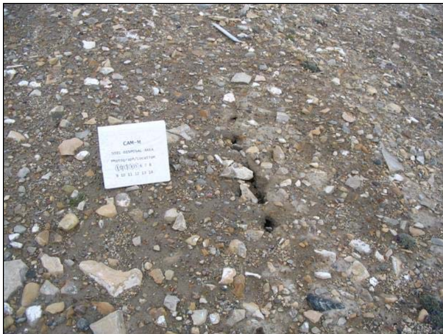
Photo SDA-5C, Easting: 494413, Northing: 7669256, Direction: 315° D.C.C. Tier II Soil Disposal Area; close up of tension crack along north crest Scale: photo placard dimensions are 29.4 cm wide by 27.5 cm in height
