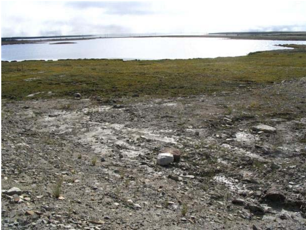
Photo MLFS-10E, Easting: 495657, Northing: 7667274, Direction: 90° Main Landfill South; eroded fines below ITS2 and VT5
