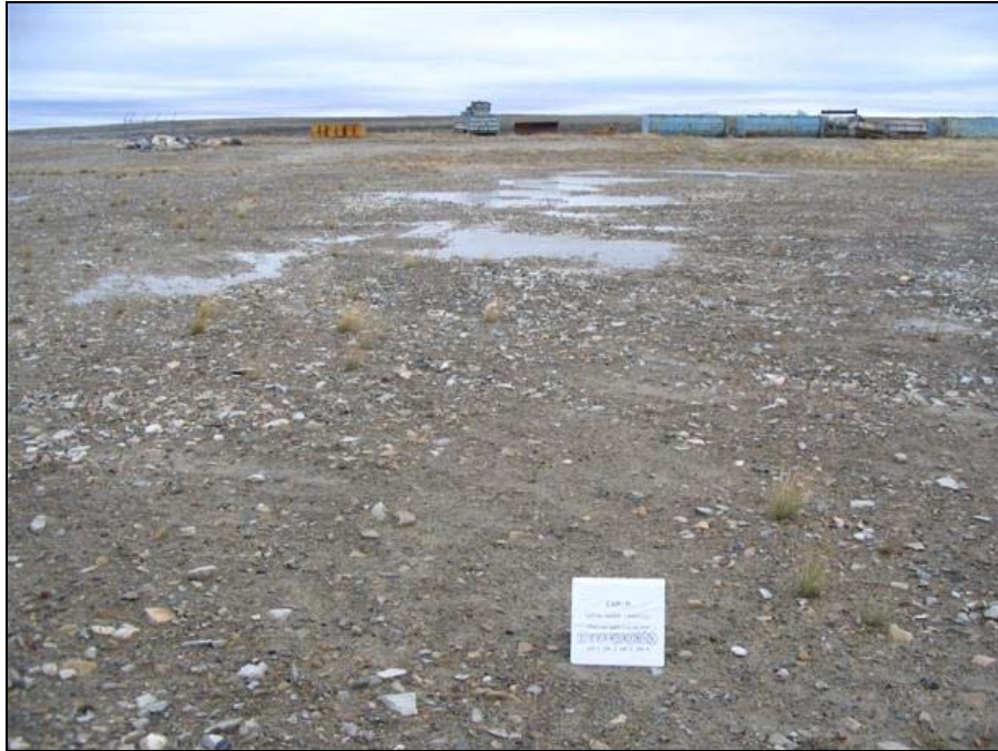
Photo SSLF-11A, Easting: 496274, Northing: 7665993, Direction: 160° South Shore Landfill; facing south to ponded water depressions Scale: photo placard dimensions are 29.4 cm wide by 27.5 cm in height
