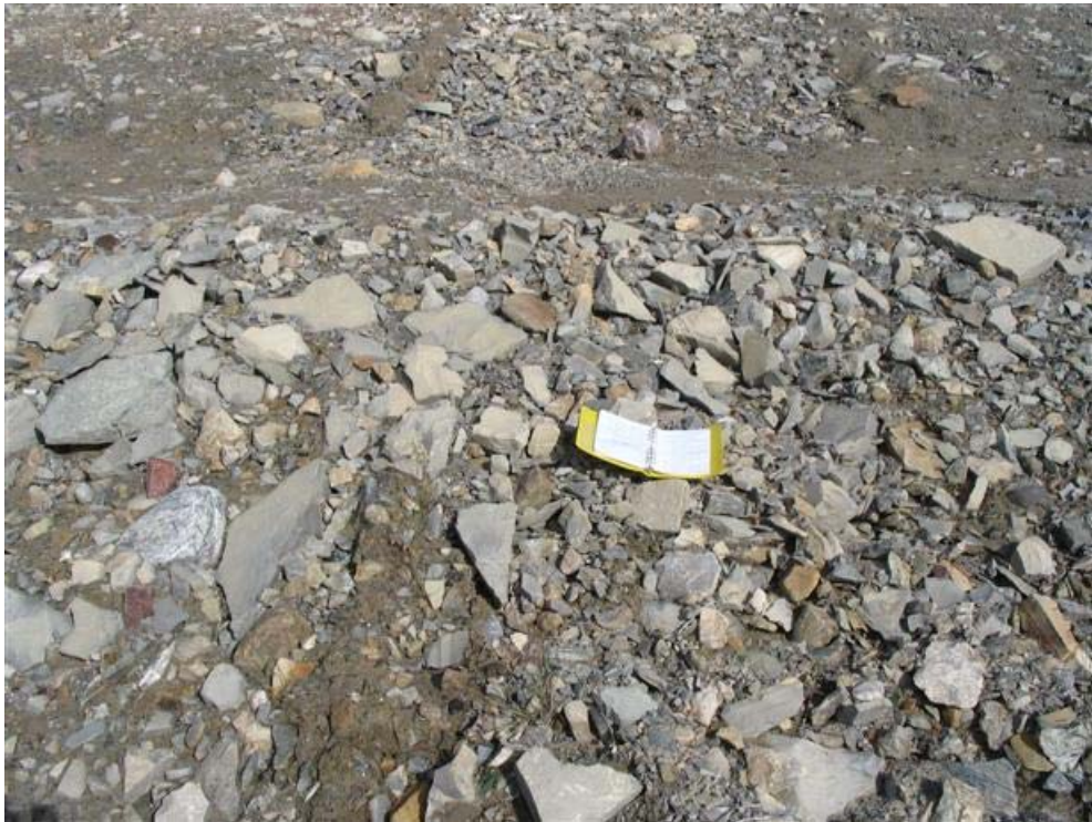
Photo MLFS-10C, Easting: 495657, Northing: 7667274, Direction: 340° Main Landfill South; close-up of erosion Scale: field book dimensions are 29.5 cm wide by 20.0 cm in height
