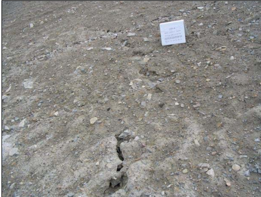
Photo MLFN-11G, Easting: 495916, Northing: 7667534 Main Landfill North; east end of crack along toe of slope Scale: photo placard dimensions are 29.4 cm wide by 27.5 cm in height
