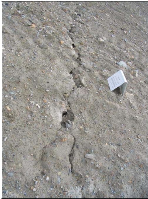
Photo MLFN-11C, Easting: 495916, Northing: 7667534 Main Landfill North; crack along toe of slope Scale: photo placard dimensions are 29.4 cm wide by 27.5 cm in height
