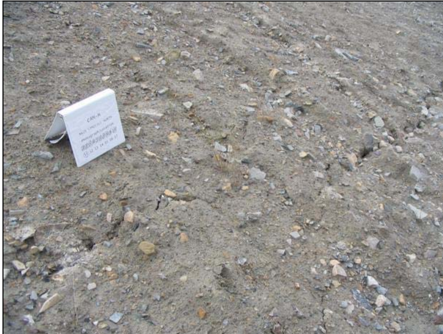
Photo MLFN-11D, Easting: 495916, Northing: 7667534 Main Landfill North; crack along toe of slope Scale: photo placard dimensions are 29.4 cm wide by 27.5 cm in height
