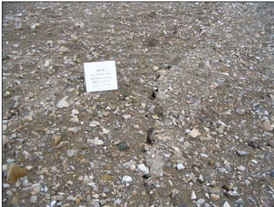
Photo SDA-3B, Easting: 494417, Northing: 7669235, Direction: 45° D.C.C. Tier II Soil Disposal Area; close-up of crack
