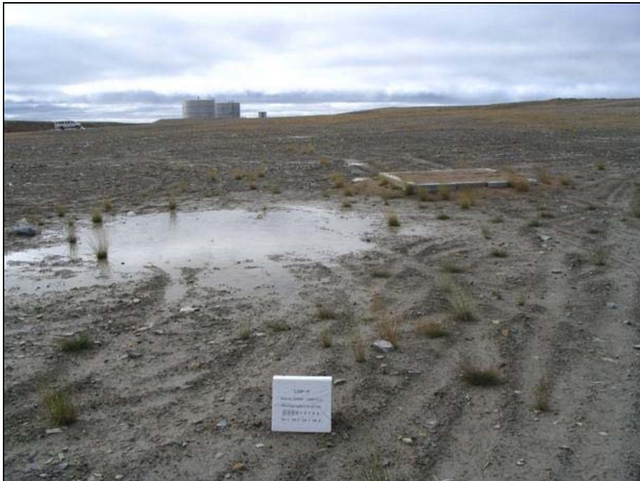
Photo SSLF-4, Easting: 496341, Northing: 7666056, Direction: 240° South Shore Landfill; view near golf tee of shallow depression with ponded water Scale: photo placard dimensions are 29.4 cm wide by 27.5 cm in height
