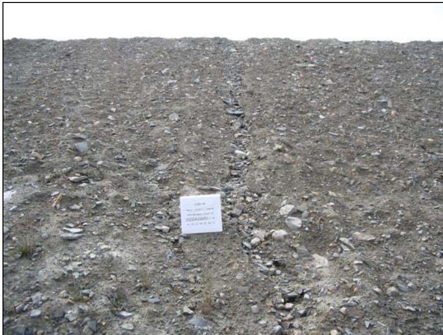
Photo MLFN-8, Easting: 495874, Northing: 7667564; Direction: 200° Main Landfill North; looking up erosion channel West of ITN2 about 0.3 m wide and 0.1 m deep Scale: photo placard dimensions are 29.4 cm wide by 27.5 cm in height
