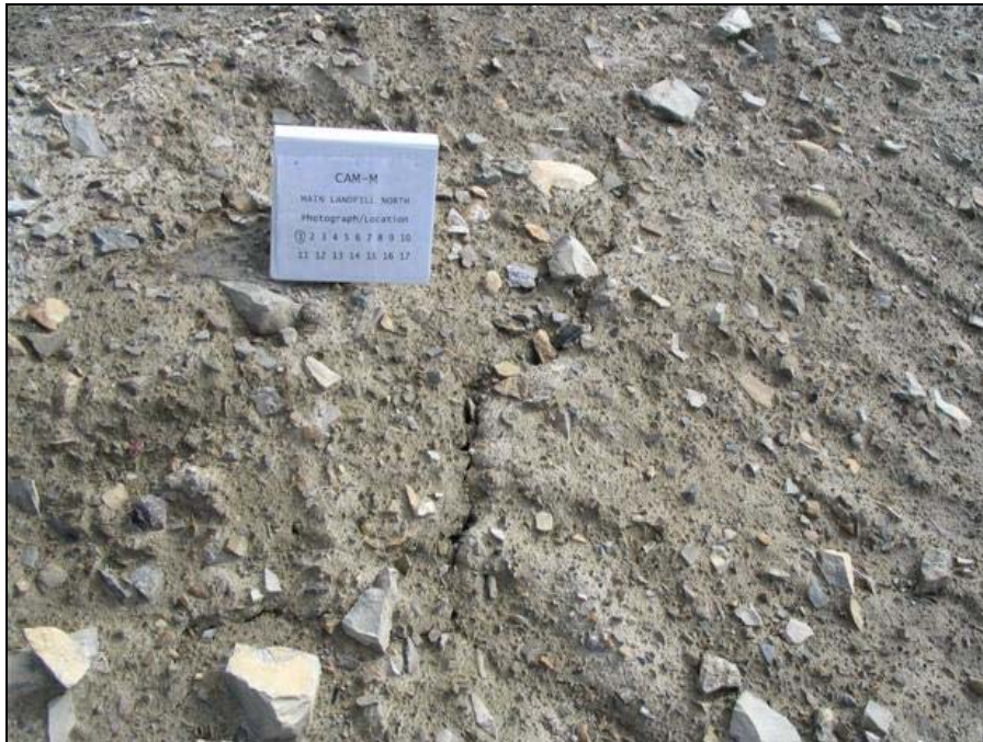
Photo MLFN-1B, Easting: 495755, Northing: 7667517, Direction: 110° Main Landfill North; 2.5 cm wide by 2.5 cm deep by 4 meters long crack on south slope Scale: photo placard dimensions are 29.4 cm wide by 27.5 cm in height
