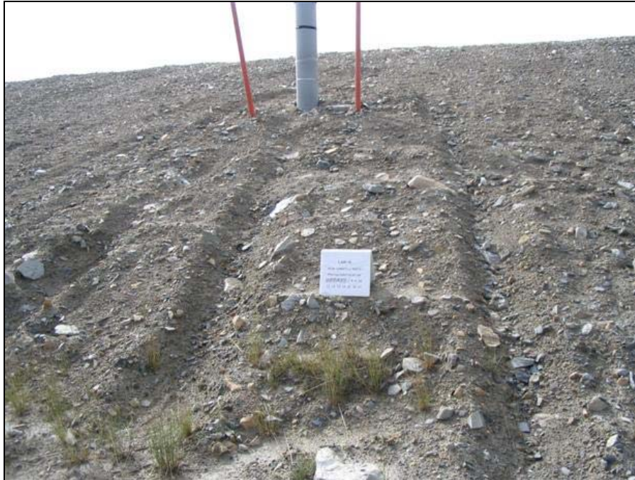
Photo MLFN-6, Easting: 495814, Northing: 7667617, Direction: 225° Main Landfill North; Erosion gullies about 0.3 m wide and 0.2 m deep spaced approximately 2 – 3 m apart Scale: photo placard dimensions are 29.4 cm wide by 27.5 cm in height
