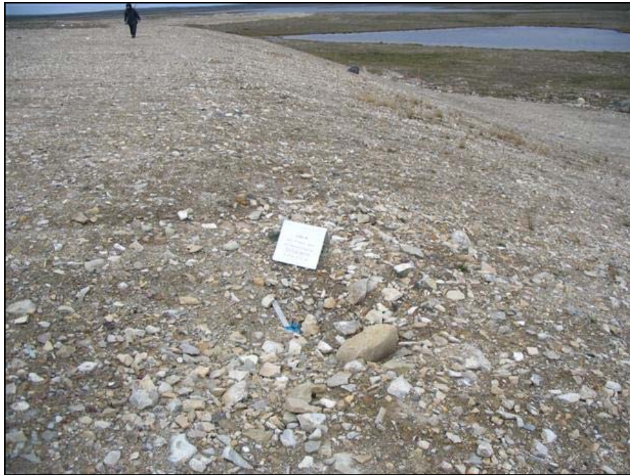
Photo SDA-8A, Easting: 494371, Northing: 7669282, Direction: 315° D.C.C. Tier II Soil Disposal Area; small settlement area at crest, 0.5 m diameter, 0.2 m deep Scale: photo placard dimensions are 29.4 cm wide by 27.5 cm in height
