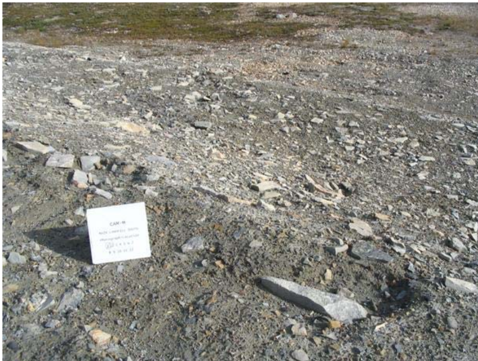
Photo MLFS-2B, Easting: 495807, Northing: 7667351, Direction: 45° Main Landfill South; close-up of north slope where self-armouring erosion has occurred
