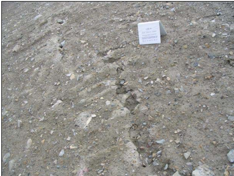
Photo MLFN-11F, Easting: 495916, Northing: 7667534 Main Landfill North; crack along toe of slope Scale: photo placard dimensions are 29.4 cm wide by 27.5 cm in height
