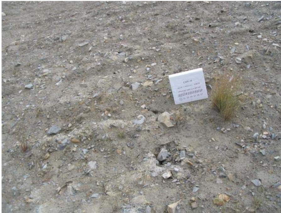
Photo MLFN-11A, Easting: 495916, Northing: 7667534 Main Landfill North; west end of crack along toe of slope Scale: photo placard dimensions are 29.4 cm wide by 27.5 cm in height
