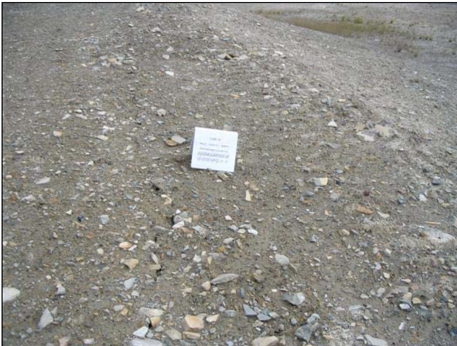
Photo MLFN-15B, Easting: 495927, Northing: 7667478, Direction: 110° Main Landfill North; tension crack along crest Scale: photo placard dimensions are 29.4 cm wide by 27.5 cm in height
