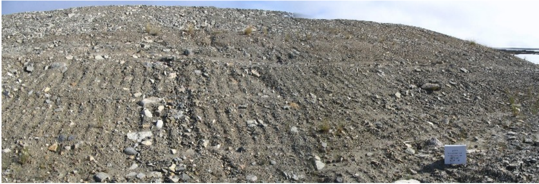
Photo MLFS-9, Easting: 495737, Northing: 7667296, Direction: 45° Main Landfill South; west slope with minor erosion Scale: photo placard dimensions are 29.4 cm wide by 27.5 cm in height
