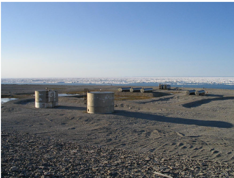
Photo : 45 Description : View north at beach area, including 2-65,000 US gal diesel tanks and 5-18,300 US ga. JP-4 tanks.
