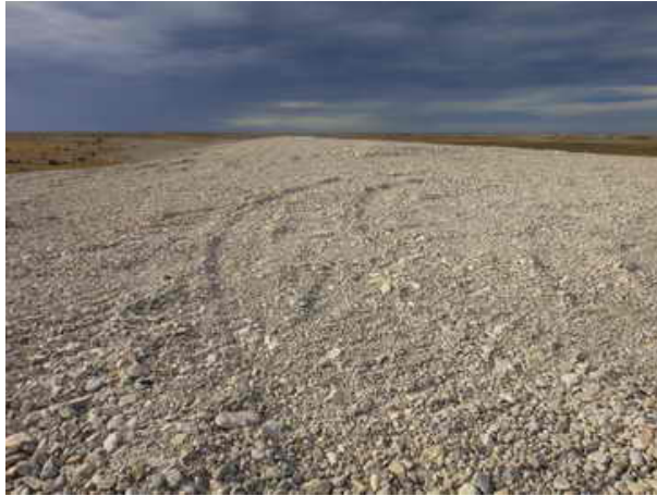
SWLF-12: View of vehicle tracks on south cover (4-8 m L, 0.3 m W, 0.05 m D) - FEATURE A
