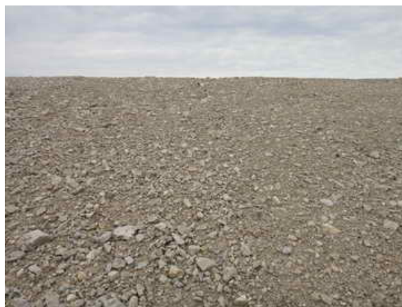
Tier II-42: (left) View south-southwest at minor erosion on southwest side slope (25 m L, 0.3-0.5 m W, 0.02-0.05 m D) - FEATURE B
