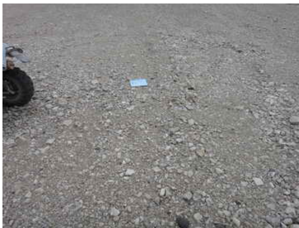
SLE-19: View southeast at minor erosion on central cover area (7m L, 0.1m W, 0.02-0.05m D) - FEATURE B
