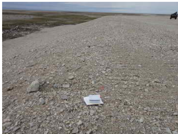
Tier II-45 (left): View south at minor depression on southwest crest (0.25 m L, 0.25 m W, 0.15 m D) - FEATURE A Tier II-47: (right) View northwest at linear depression on southwest crest (1 m L, 0.2 m W, 0.1 m D) - FEATURE A
