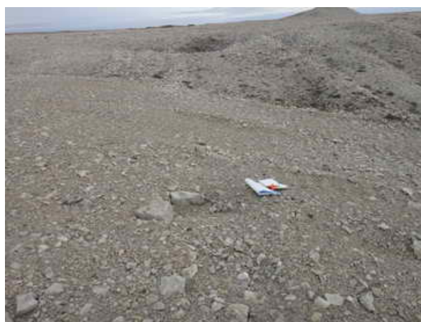
SBLF-3: (left) View west at minor depression on north side slope (0.5m L, 0.5m W, 0.1m D) - FEATURE A SBLF-21: (right) View west at localized pothole on east crest (0.6 m L, 0.25 m W, 0.1 m D) - FEATURE A
