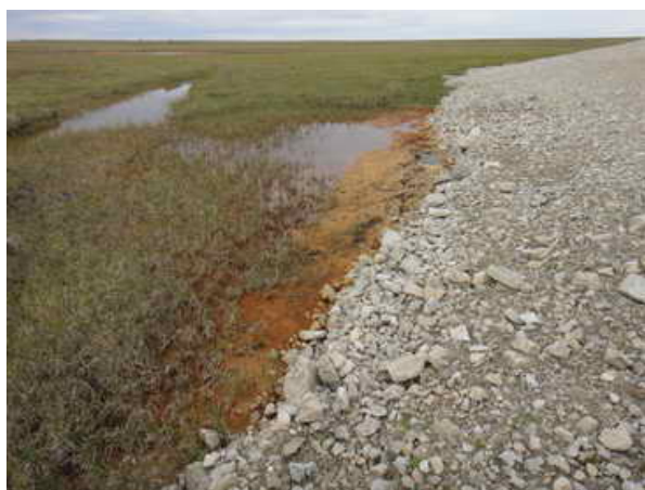
SBLF-15: (left) View northwest at staining in ponded area on southwest corner (10 m L, 0.2-1 m W) - FEATURE B SBLF-16: (right) View of non-hydrocarbon sheen on water at southwest toe (10 m L, 0.2-1 m W) - FEATURE B
