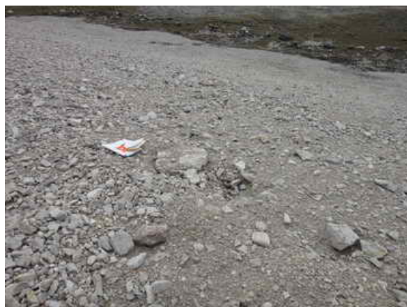
Tier II-45 (left): View south at minor depression on southwest crest (0.25 m L, 0.25 m W, 0.15 m D) - FEATURE A Tier II-47: (right) View northwest at linear depression on southwest crest (1 m L, 0.2 m W, 0.1 m D) - FEATURE A
