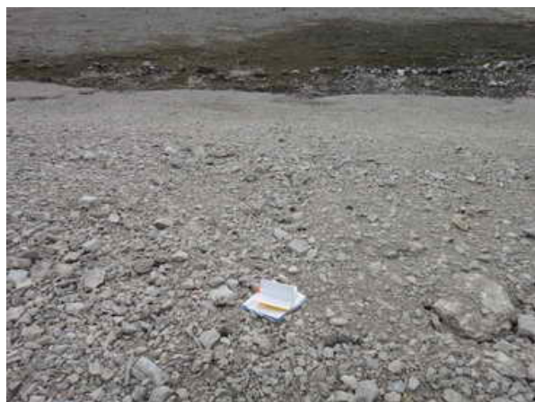
Tier II-42: (left) View south-southwest at minor erosion on southwest side slope (25 m L, 0.3-0.5 m W, 0.02-0.05 m D) - FEATURE B
