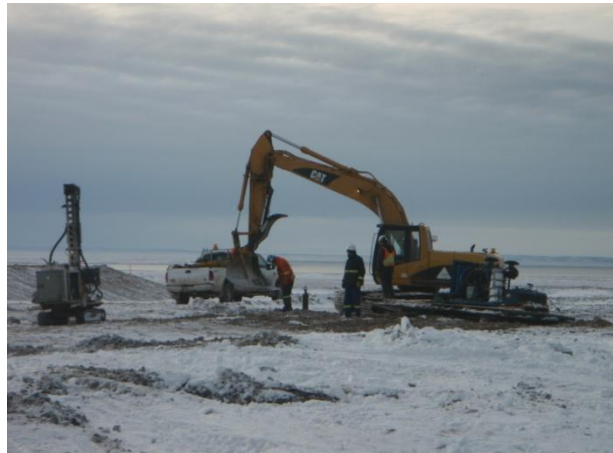
Photograph 4 ↑ Monitoring well installation
