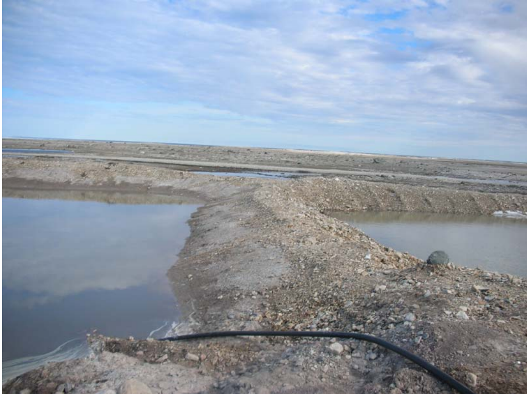
Photo 1 (DSCN 3935): Berm between sewage cells, secondary cell seen at right of photo, taken facing south.
