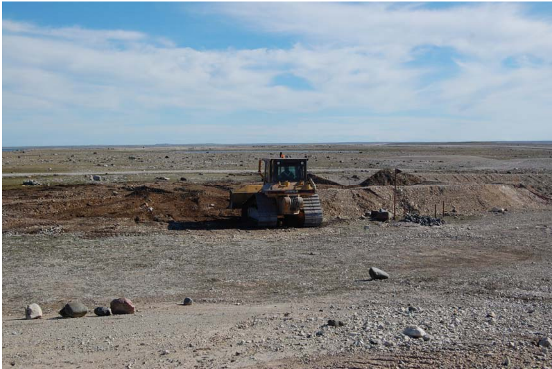
Photo 3 (Sewage Lagoon Closure – Aug.01.2011): Sewage lagoon with backfilling in progress, photo taken facing east.
