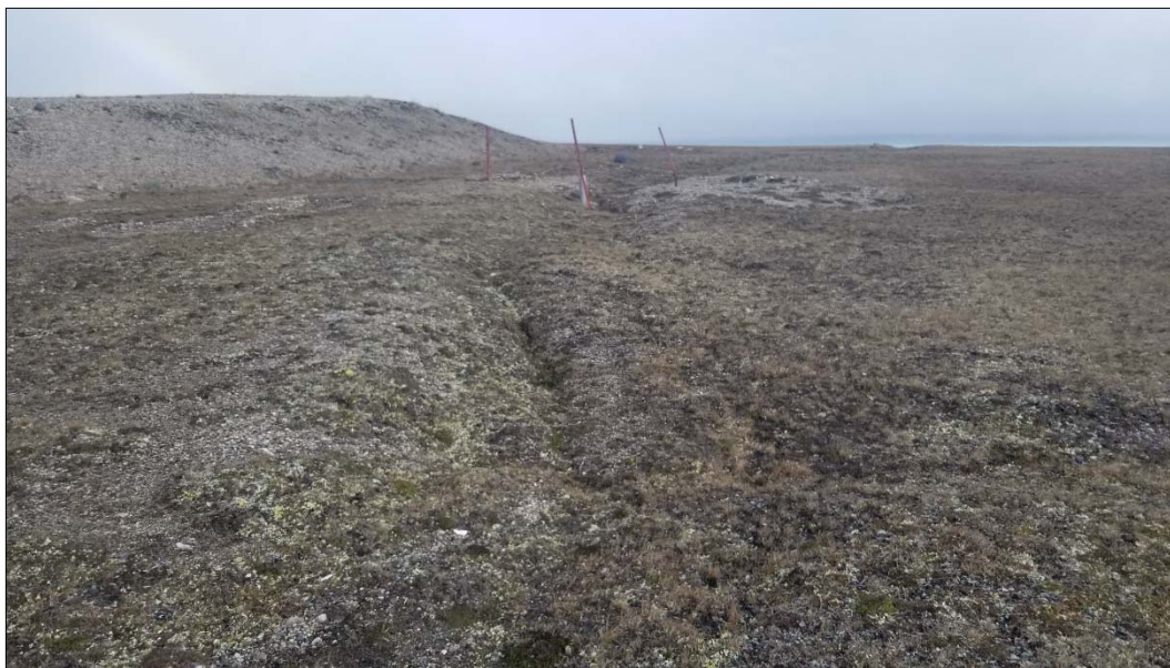
Photo 12: Drainage Pathway on Southeast Side of NHWL, Viewpoint 93
