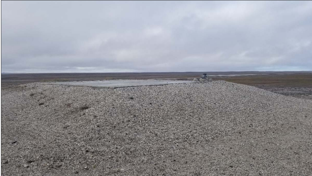
Photo 13 : Concrete Pad at Main Station Area, Viewpoint 110
