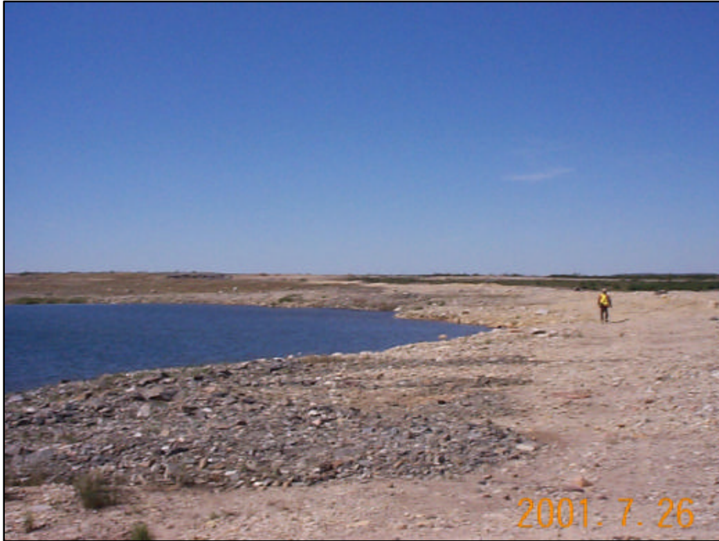
Photo 3: Dam No. 1 - looking along crest
