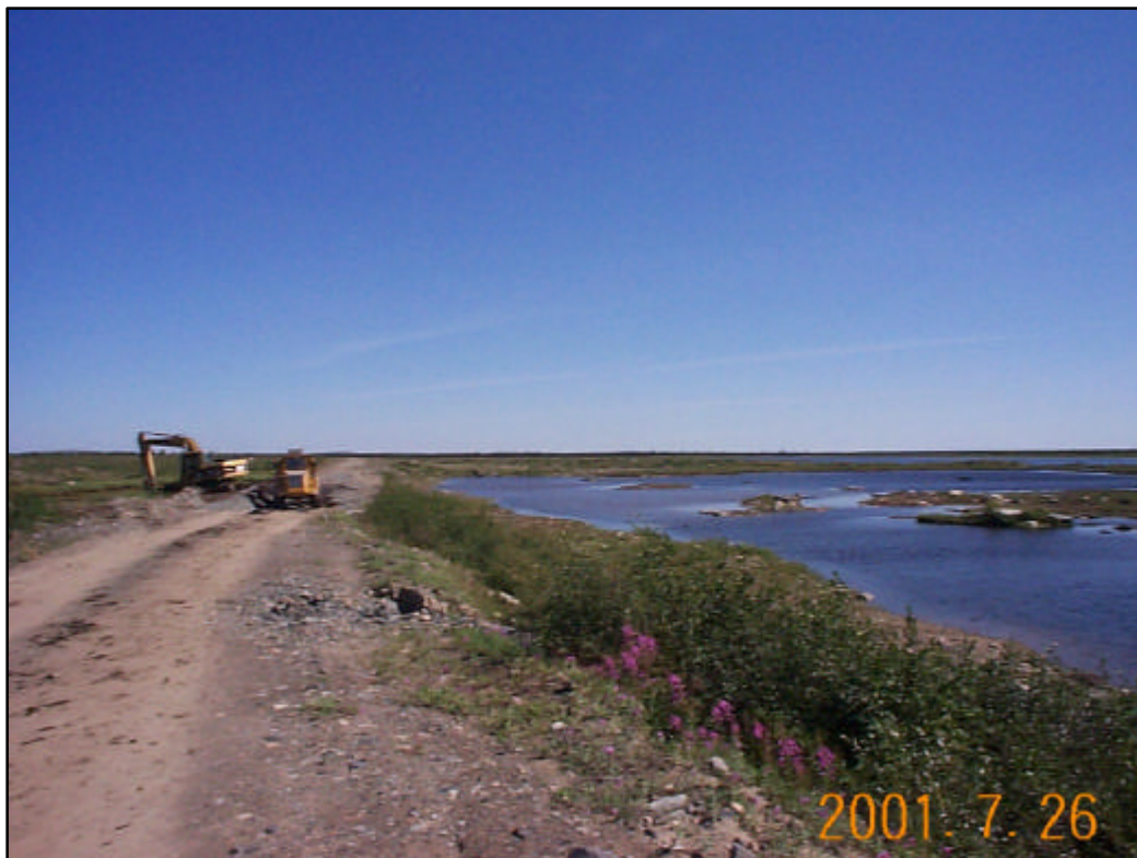
Photo 8: Dam No. 2 – looking south-southeast
