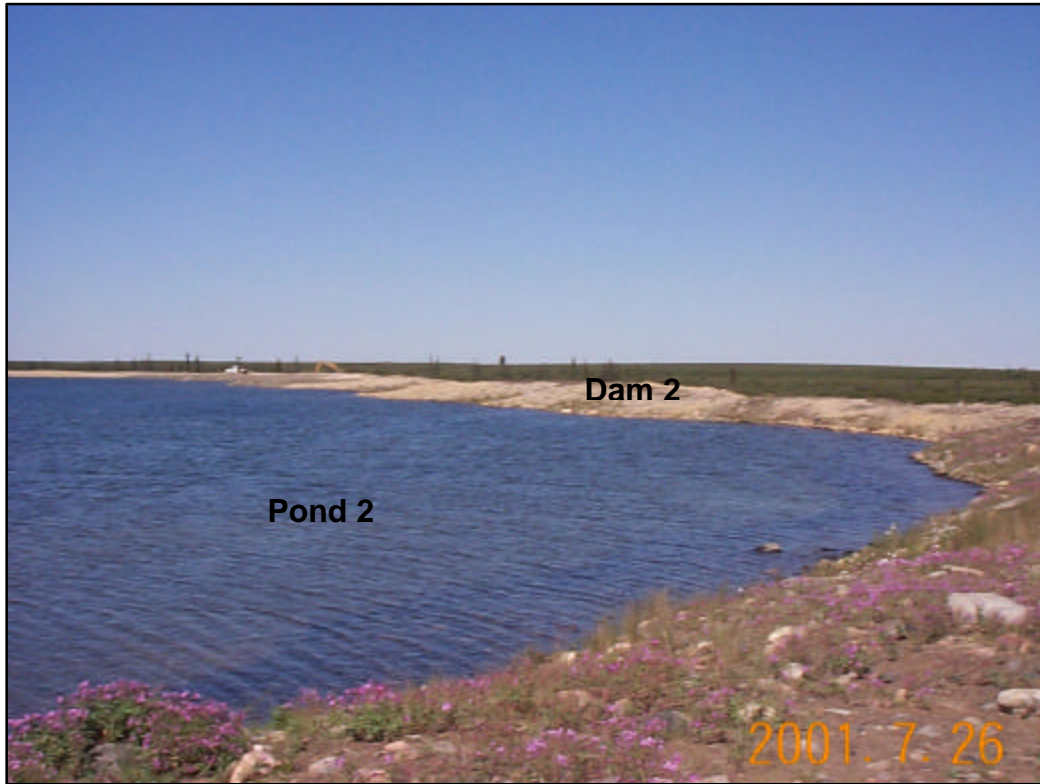
Photo 7: Dam No. 2 – looking north-northwest
