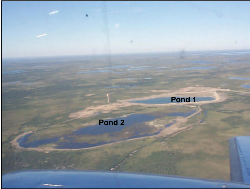
Photo 1: Cullaton Lake Tailings Facility – looking west
