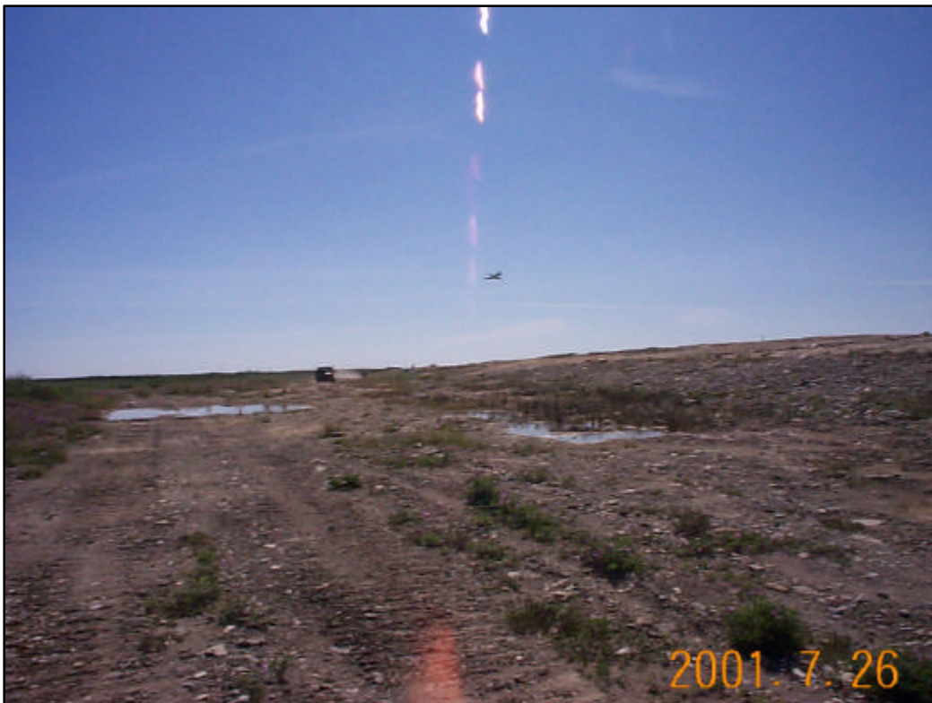
Photo 4: Dam No. 1 – looking south on downstream side
