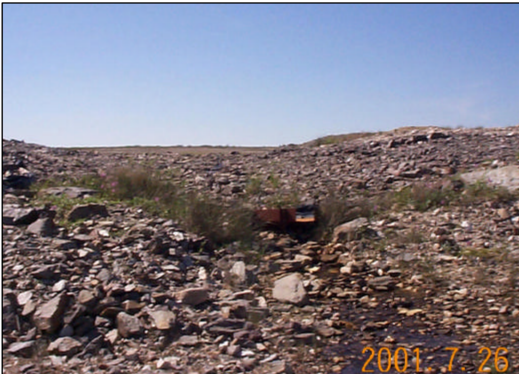
Photo 6: Dam No. 1 spillway channel and weir - looking upstream
