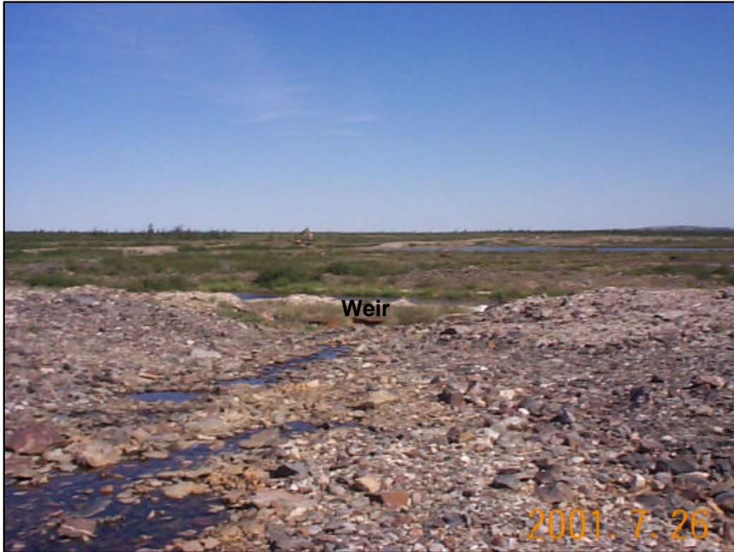
Photo 5: Dam No. 1 spillway channel – looking downstream to Pond 2
