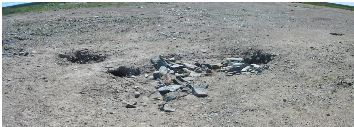
Photograph 5-12. Settlement areas in southeast corner of quarry pit cover (July 2007)
