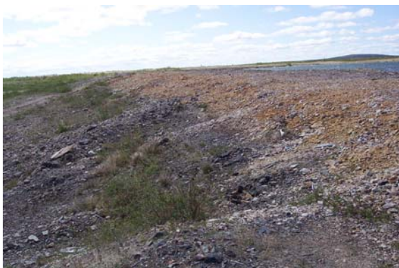
Photo 4. Photo of tailings dam, southeast end, note constructed of meta-volcanics (below) and quartzite (orange, above).
