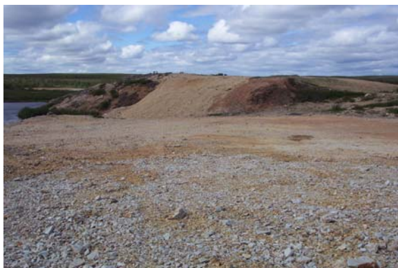
Photo 32. Overview of backfilled Shear zone portal (note backfill is pyritic quartzite).
