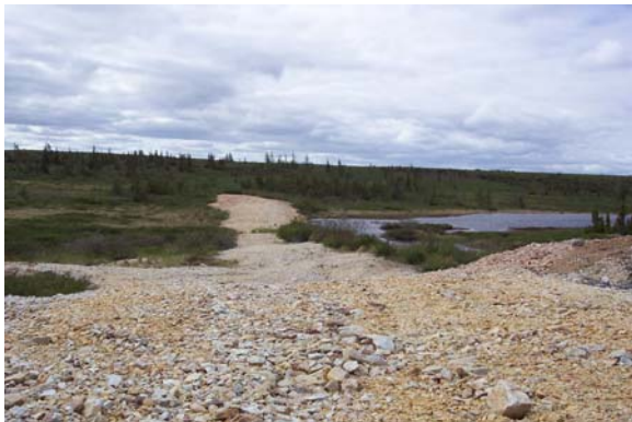
Photo 29. Dam in north end of Shear Lake constructed of pyritic quartzite.
