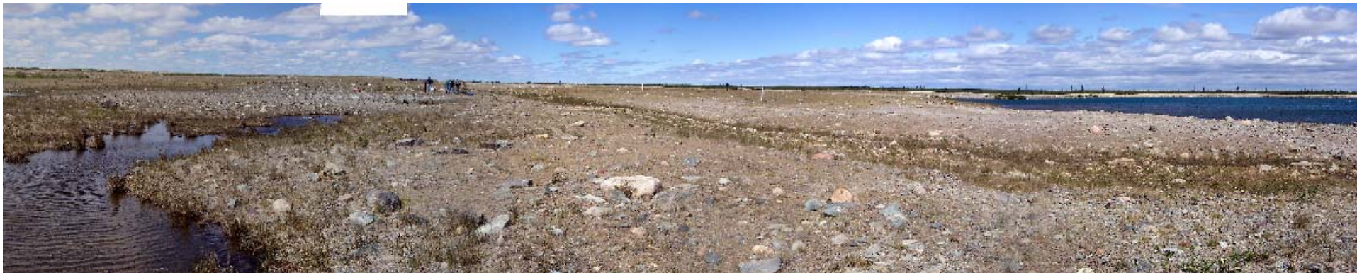
Photo 12. Panoramic photo of till covered tailings in TSF taken from central location of beach near water – till cover transition zone. Standing ponded water on top of till cover ranged in pH from 8.2 to 8.4 and EC ranged from 3.9 to 4.6 mS/cm.
