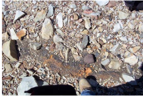
Photo 8. Exposed tailings along upstream side of north end of dam
