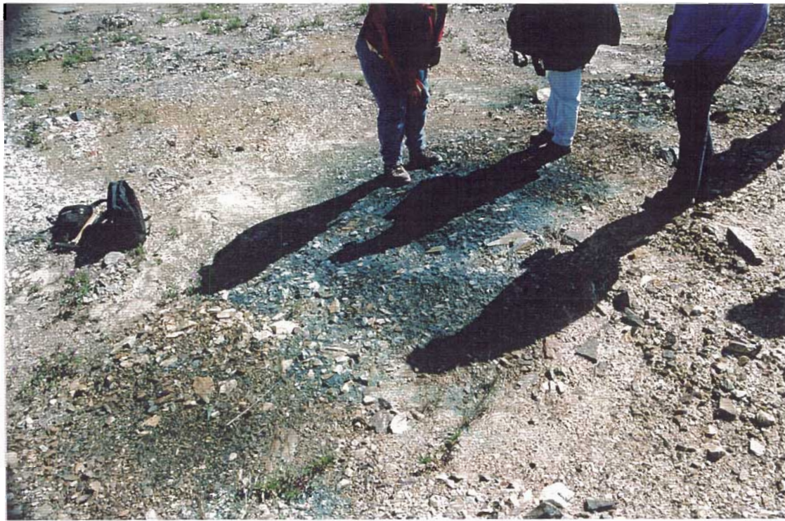
Blue stained area along downstream side of tailings dike on north side.
