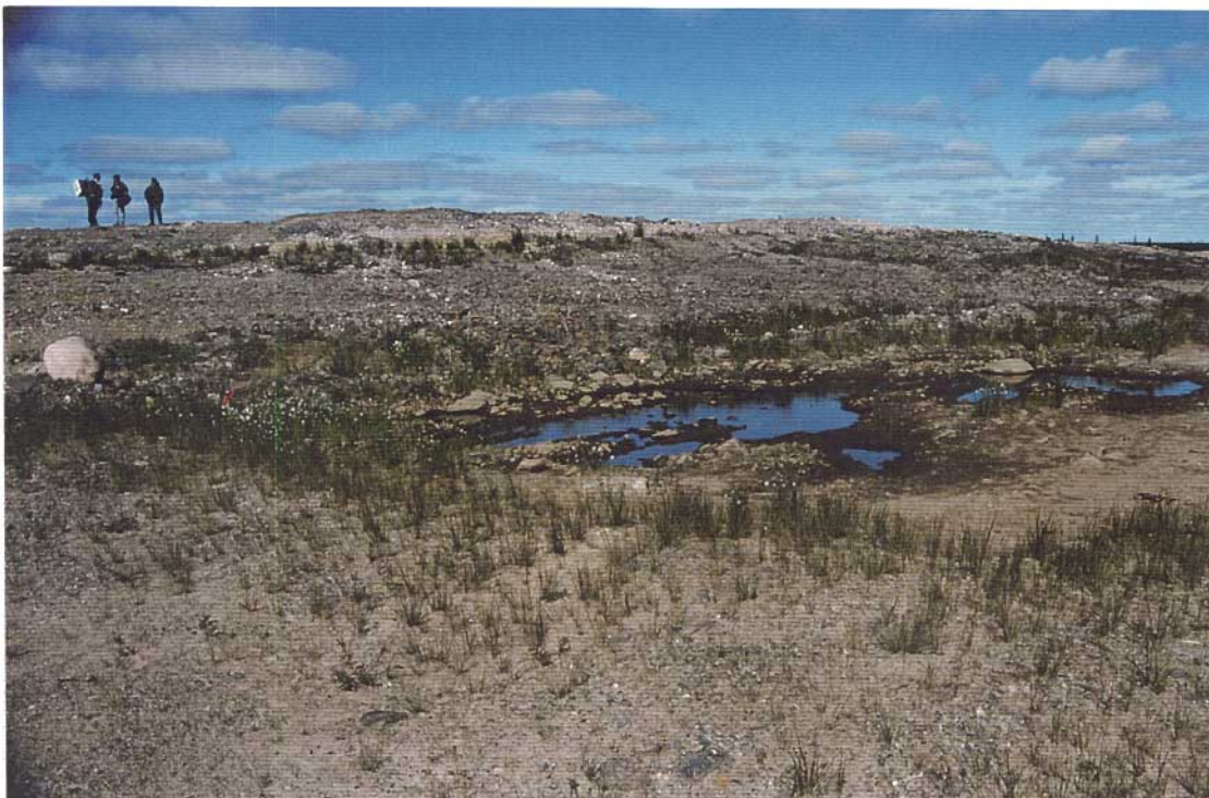
Seepage zone through #1 tailings dike near south abutment. Water sampling point.
