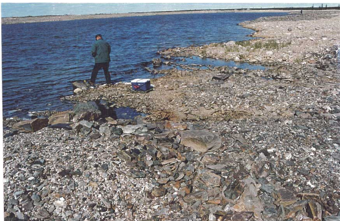
Seepage zone through #1 tailings dike near south abutment. Water sampling point.
