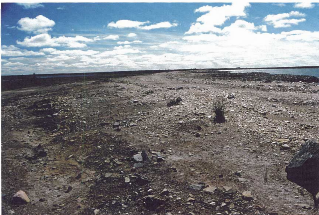
Area of oxidized sulphide bearing waste rock and blue stained patches on north side of Tailings Pond #1.
