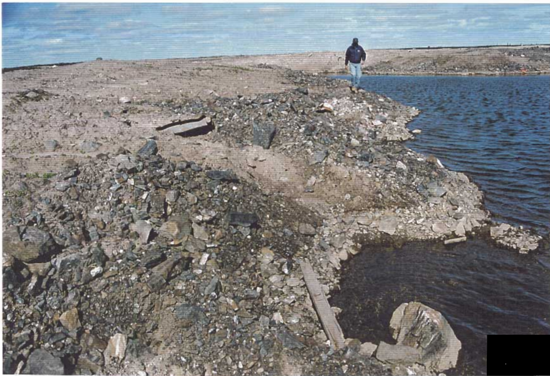
Protruding pieces of metal demolition debris buried in landfill area in quarry.
