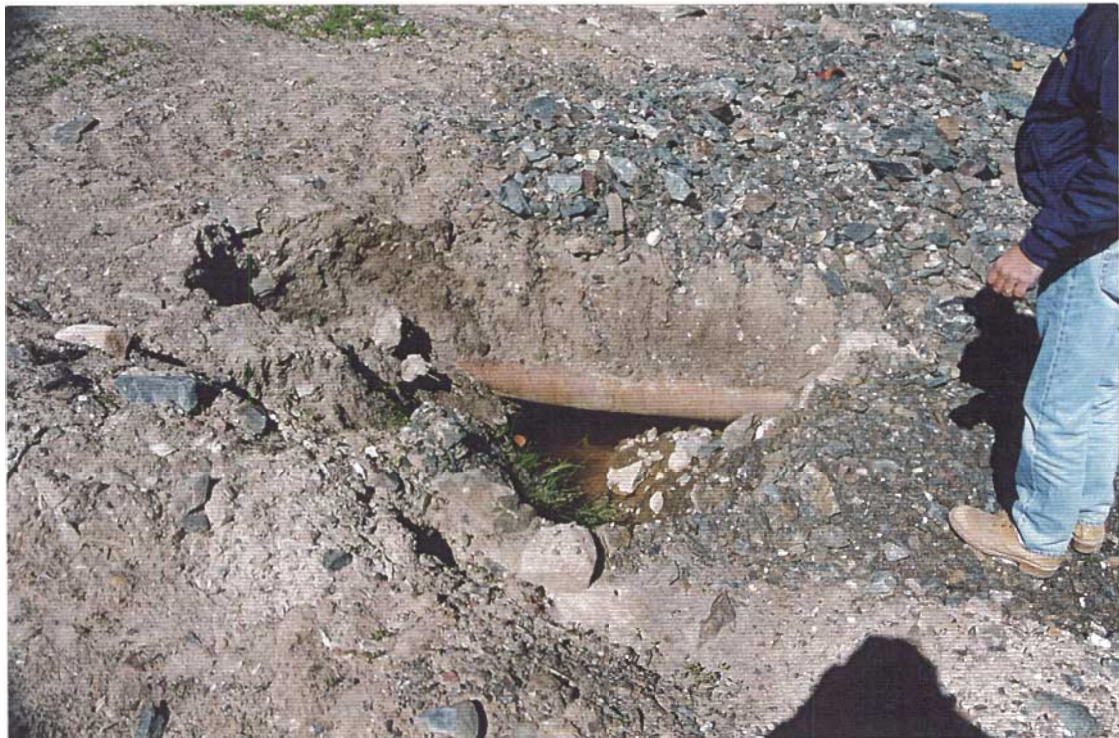
Collapse of till cover over demolition debris along west shoreline of Quarry.
