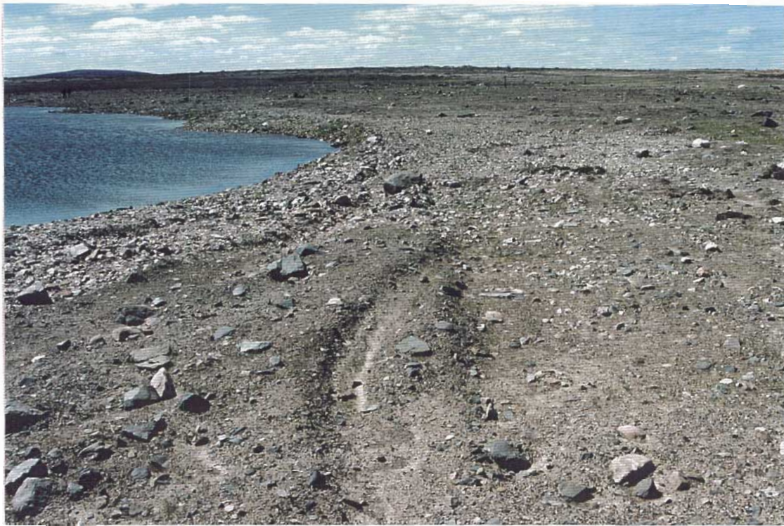
Till covered tailings area. Black pipes visible in background contain piezometers and thermistors.
