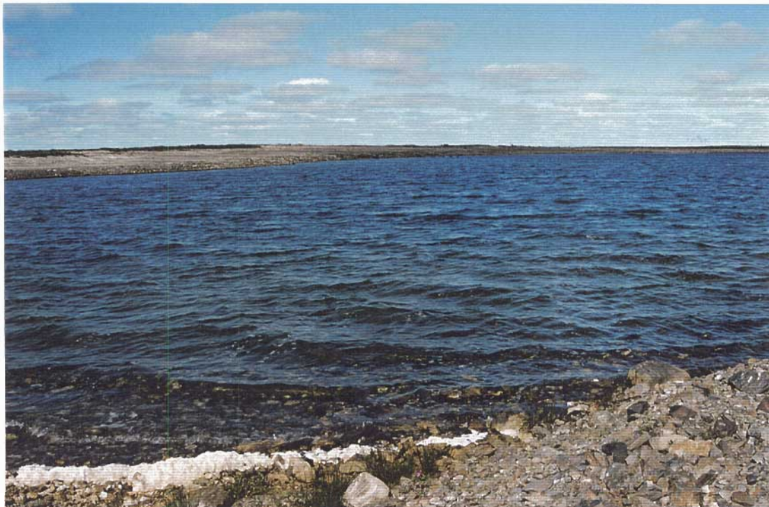
Tailings pond #1, looking north from south end. Distant shoreline contains tailings above water line, capped by till.
