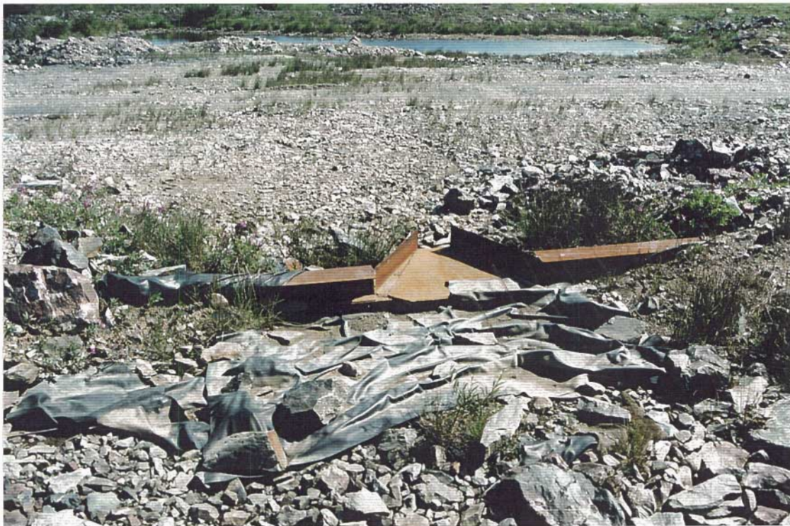
Spillway breach in #1 Tailings Pond dike – approximately 1m deep below crest level. Partially exposed HDPE liner on right.
