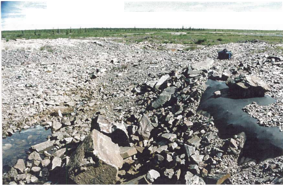
Spillway breach in #1 Tailings Pond dike – approximately 1m deep below crest level. Partially exposed HDPE liner on right.
