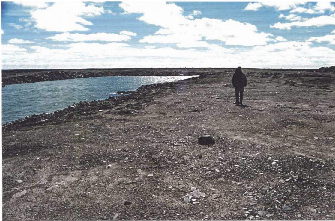
Quarry site, located south east of Tailings Pond #1. Used for disposal of demolition debris from mine and mill buildings. Covered with till. Rockfill along shoreline.
