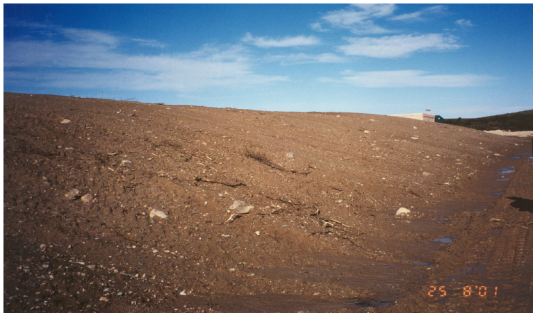
Photo 35. East slope of the new waste rock pile. Photo shows the northern portion of the pile, where capping materials contain more silt (silt till).
