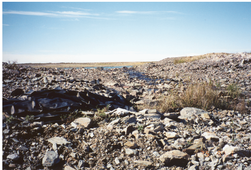
Photo 68. Spillway channel. Photo is looking upstream, showing water flow from the pond. Note the exposed piece of geomembrane. The steel weir formerly located in this area had been removed.
