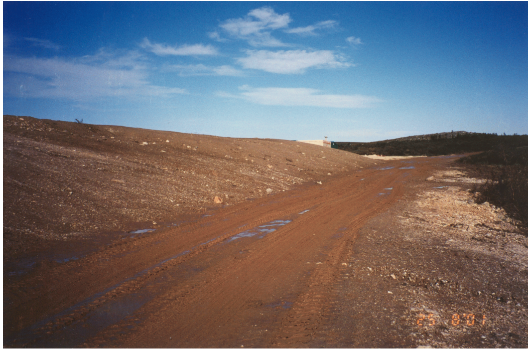
Photo 29. Newly built waste rock pile. The pile was capped with till fill materials. Photo is looking to the north, with access road separating the location of the new and old waste rock stockpiles. Part of the camp can be seen at the middle right side of the photo.
