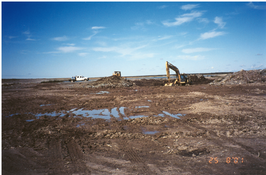
Photo 51. A portion of the Quarry Pit was used to bury crushed, inert waste materials, such as concrete rubble, steel plates, steel structures, etc. The backhoe was utilized to bury the last pieces of waste materials : an old bus and a burn box.
