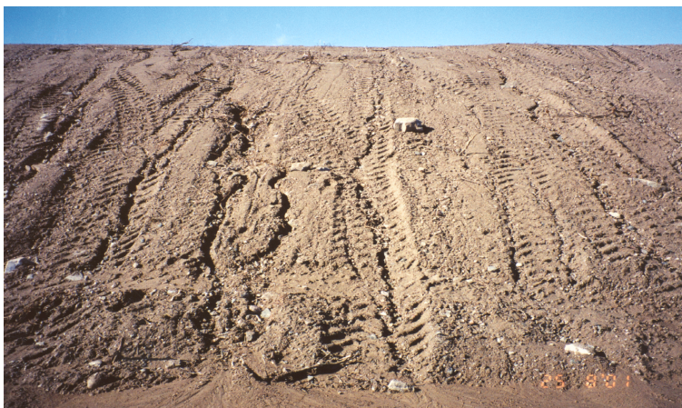
Photo 36. Close up view of the silt till capping materials. Note the degree of compaction, and some erosion from the water runoff.
