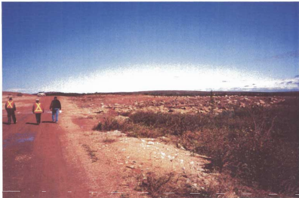
Photo 25. Old waste stock pile (right side - east of the road). Photo is looking north. Waste rock has been removed to the east side of the road. Note that some natural boulders were left at the old site.
