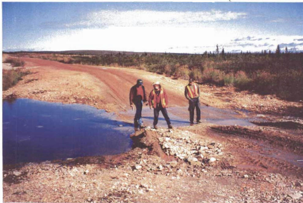
Photo 21. Another view of the creek which crosses the access road. The water level was relatively high due to recent rainfall. Usually water crosses under the access road through three to four 6in. dia. culvert pipes.
