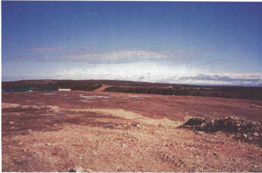
Photo 31. A view of the crest of the capped waste rock pile. Photo is looking to the north/northeast. Notice the contact between the new fill (darker brown) and the rock outcrop in the foreground.
