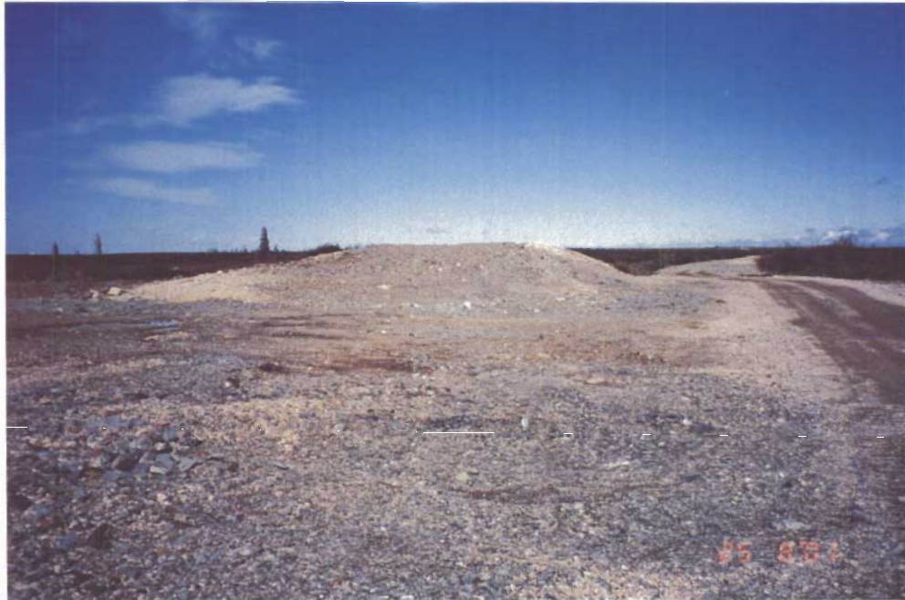
Photo 44. Close up view of one of the two “berms”. The ventilation outlet has been blocked, backfilled with granular materials and contoured.
