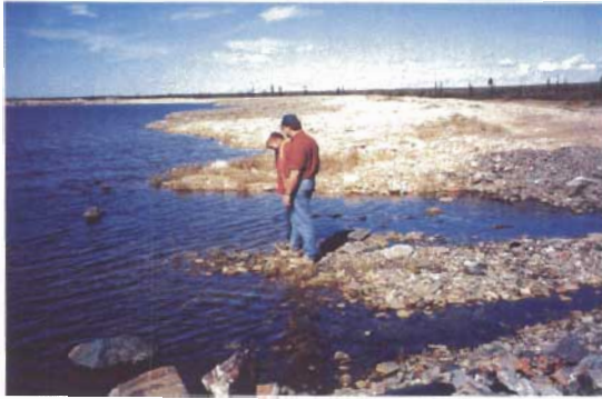
Photo 64. Water entering the spillway at the upstream side of Tailings Pond No. 1
