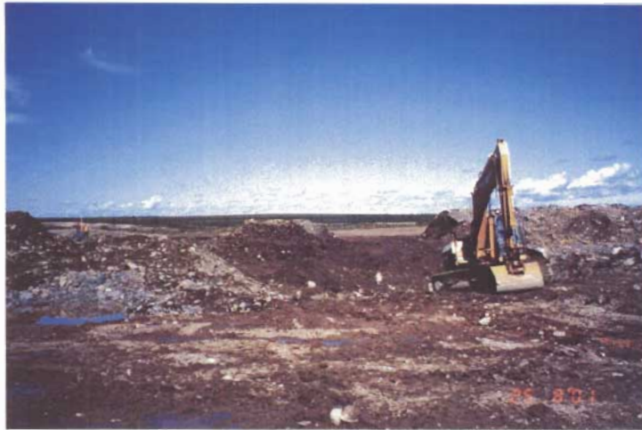
Photo 54. Burial of inert waste materials in the southern portion of the Quarry Pit.
