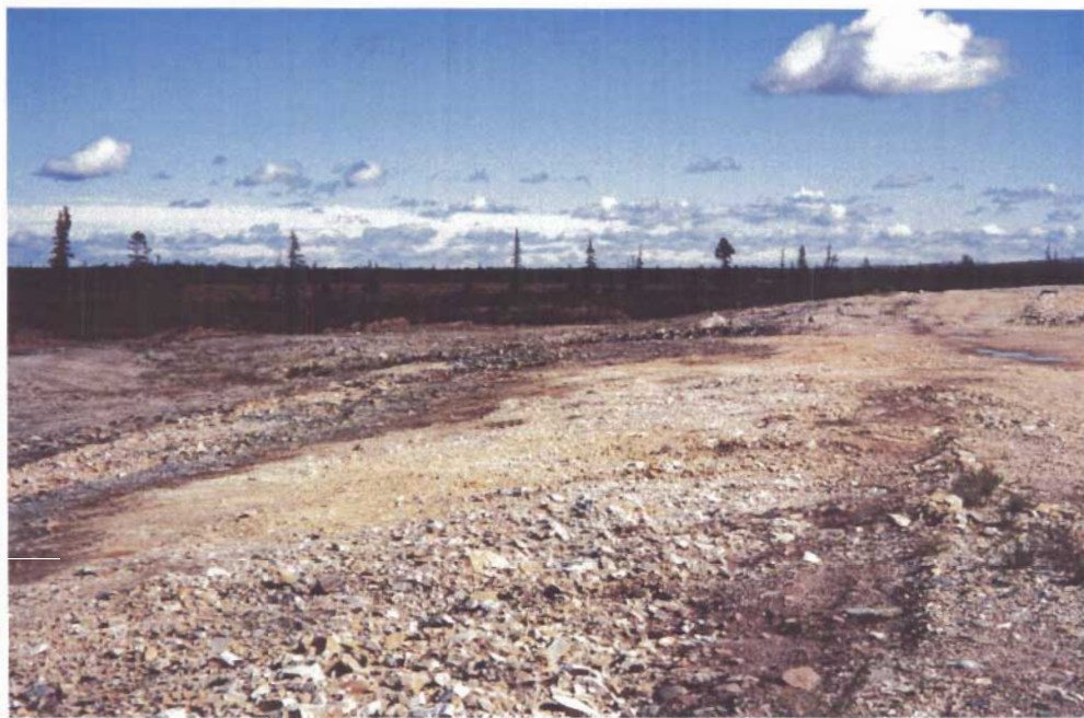
Photo 63. Another view of the downstream slope of Tailings pond No.1 dam. The crest of the dam was generally wide, and the downstream slope was relatively flat.
