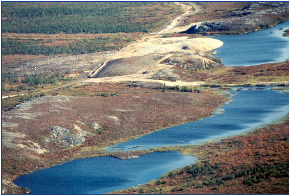
PHOTO 1: Aerial view of completed capped Shear Lake waste rock pile (center), with Shear Lake to the right. Note toe berm ringing the pile. View looking south.
