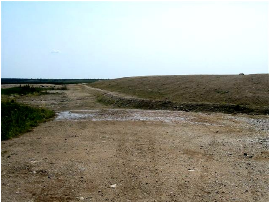
Photo 2: Area of seepage at northeast corner of encapsulated waste rock, July 7, 2004
