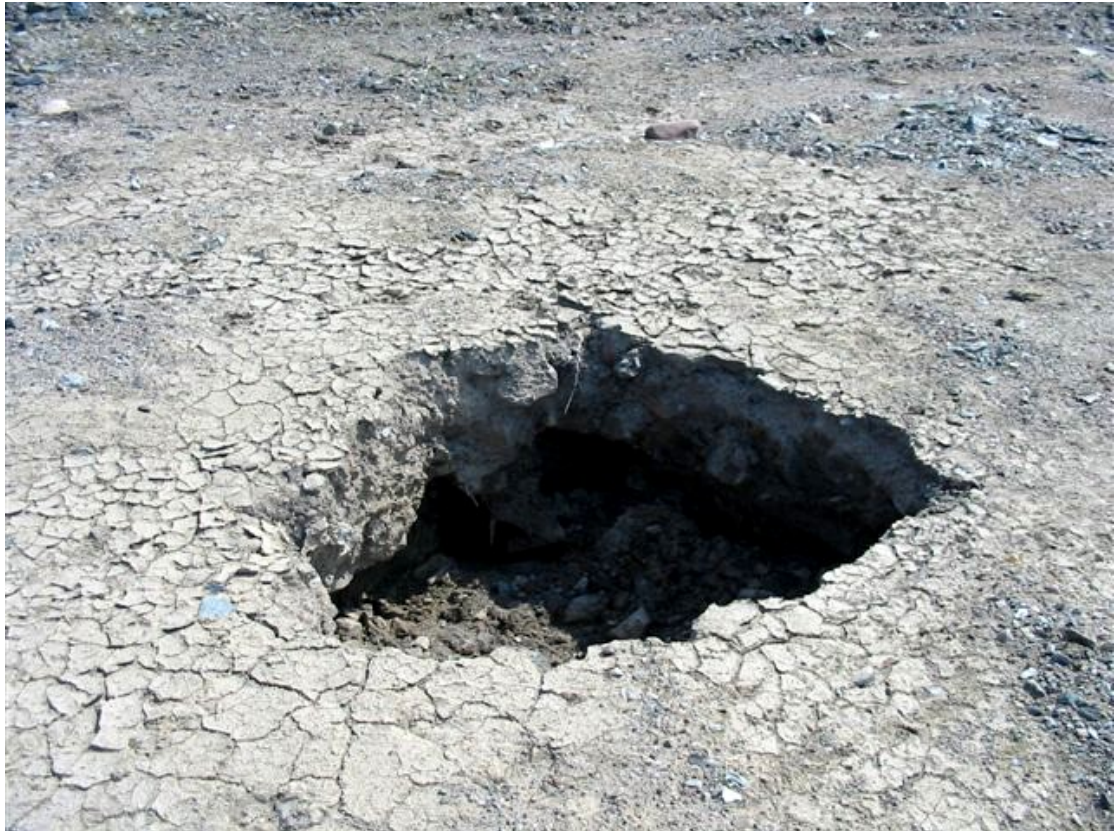
Photo 3: Minor settlement in quarry pit cover, July 7, 2004
