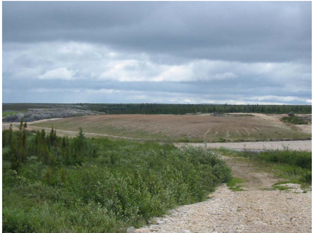
Photo 8: Encapsulated Waste Rock at Shear Lake following the application of additional seed and fertilizer. The erosion scars are visible in the foreground due to being filled in with lighter coloured granular road material.
