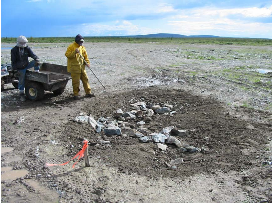
Photo 9: Minor settlement in quarry pit cover filled in August 4, 2005
