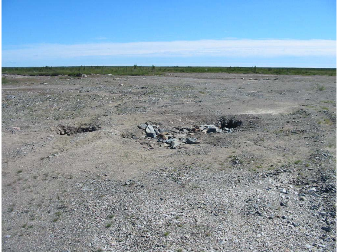
Photo 9: Minor settlement in quarry pit cover 1 year after being filled in on August 4, 2005
