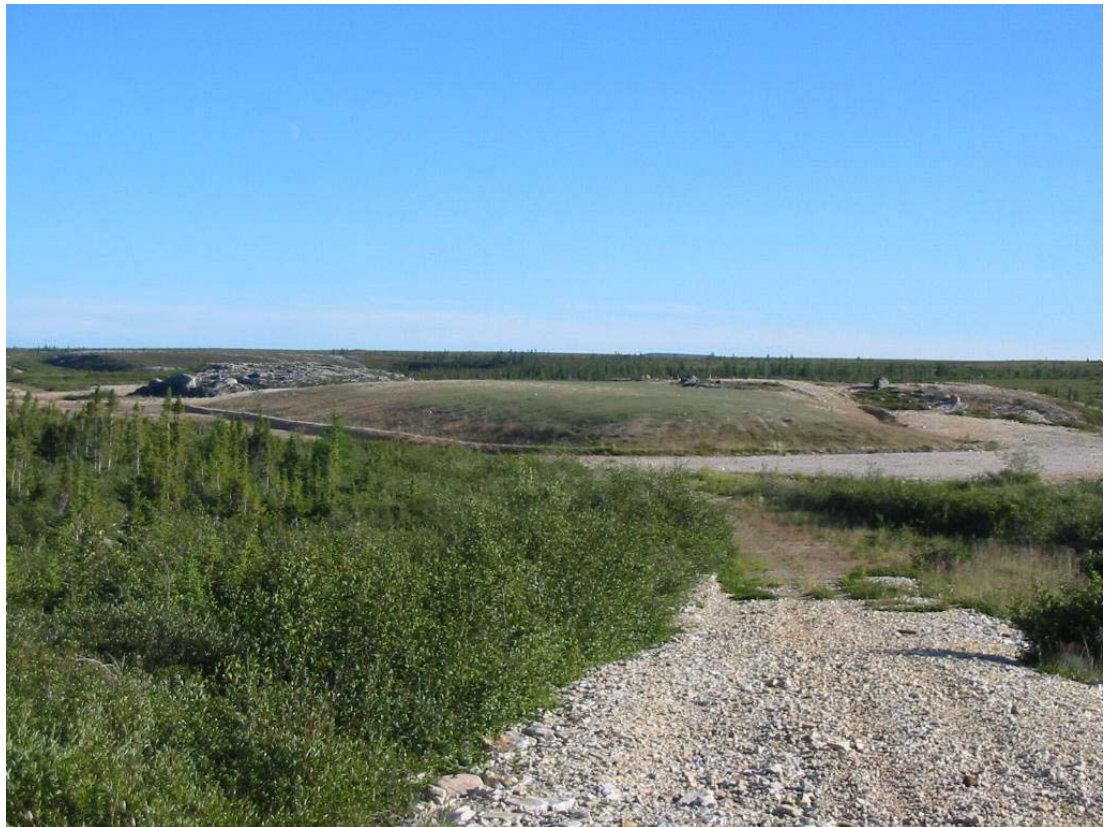
Photo 8: Encapsulated Waste Rock at Shear Lake 1 year after the application of additional seed and fertilizer. Erosion scars are visible due to being filled in with lighter coloured granular road material.
