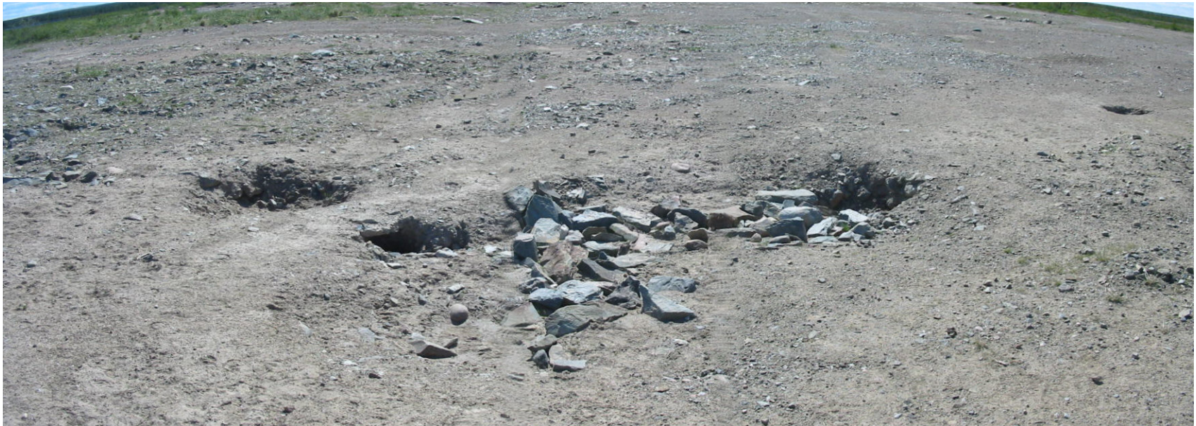
Photo 9: Minor settlement in quarry pit cover on July 5, 2007, 2 years after being filled in August, 2005.
