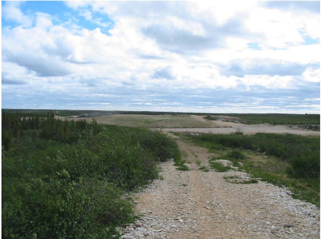
Photo 8: Encapsulated Waste Rock at Shear Lake 2 years after the application of additional seed and fertilizer. Erosion scars are visible due to being filled in with lighter coloured granular road material.
