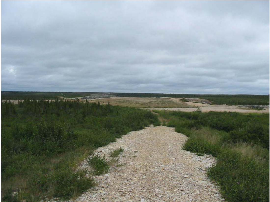
Photo 7: Encapsulated Waste Rock at Shear Lake 3 years after the application of additional seed and fertilizer. Erosion scars are visible due to being filled in with lighter coloured granular road material.
