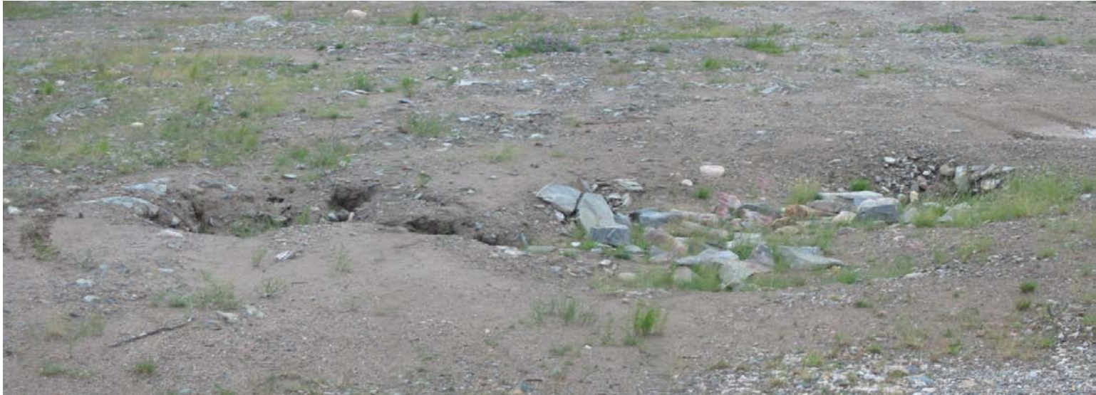
Photo 10: Minor settlement in quarry pit cover on August 3, 2008, 3 years after being filled in August, 2005.
